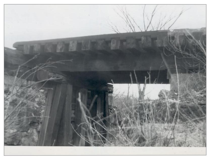
Small Bridge Between 1st and 2nd curve north of North Bennington 4/21/1962 Bridge Cribbing Installed to Support 90 Class Locomotives
