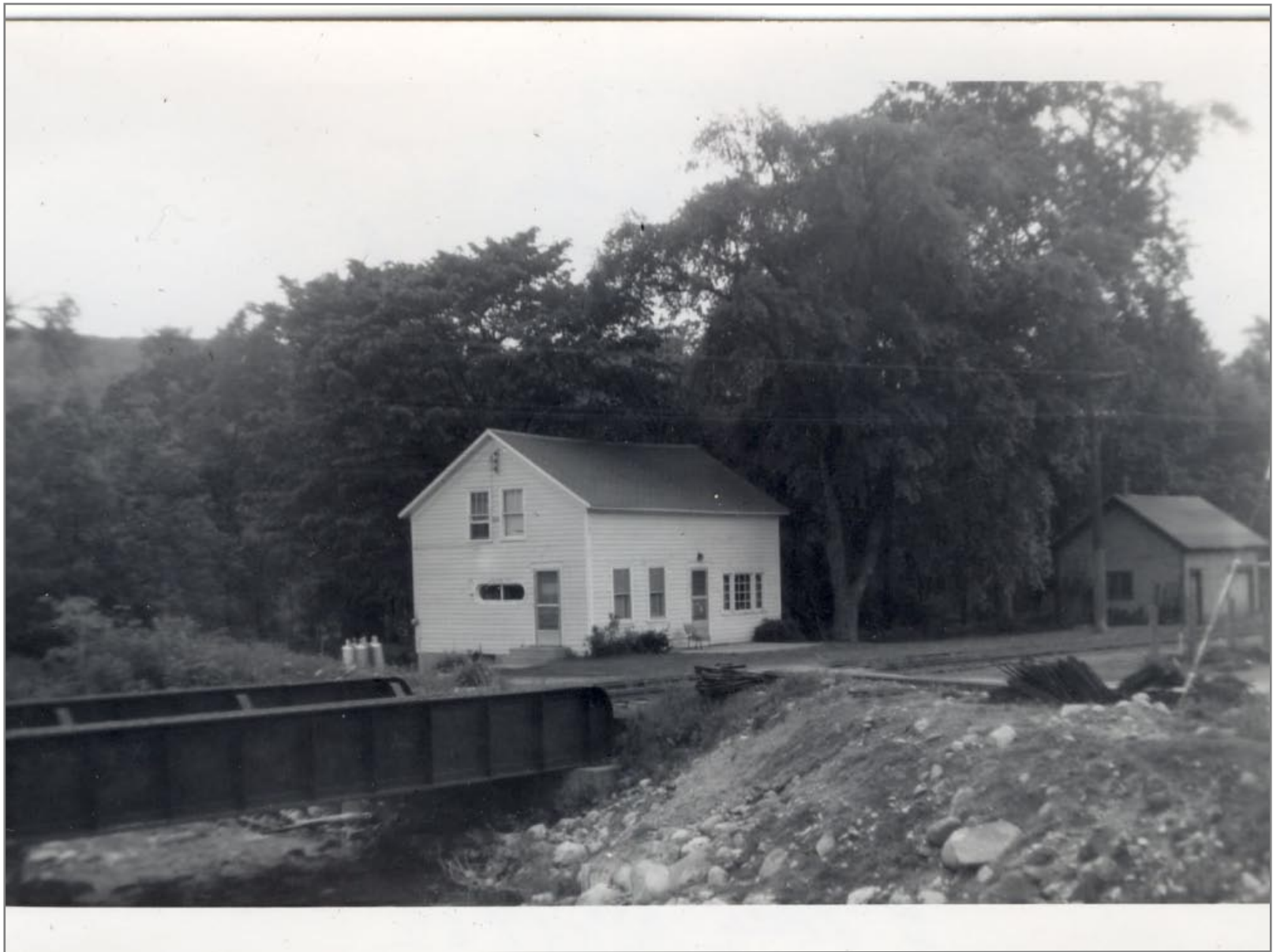
Bridge 91 Wallingford - Section House on Right 5/30/1962
