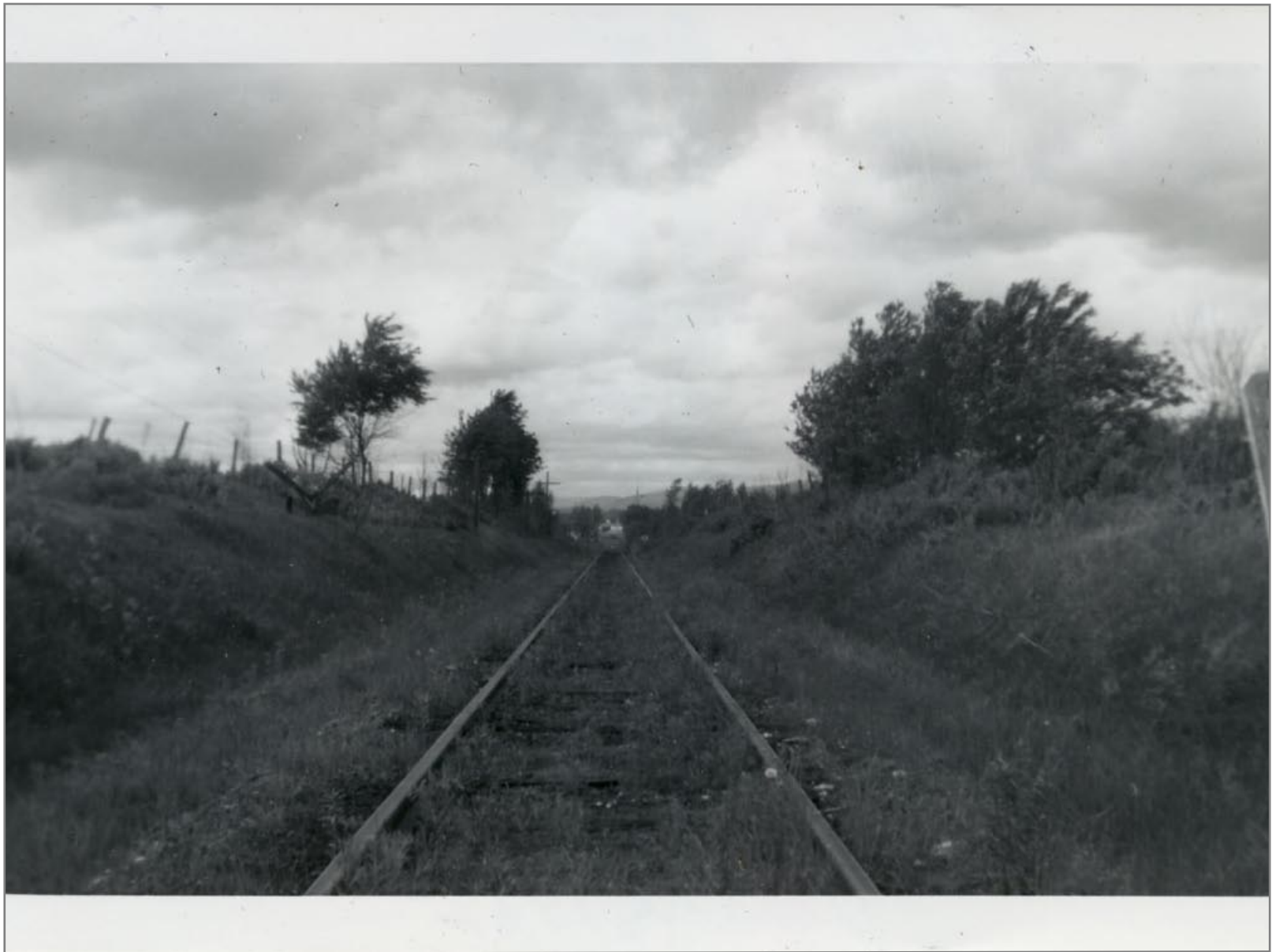
MP 53 Northbound 6/2/1962 Rutland Yard Limit Sign Distant Right 6/2/1962
