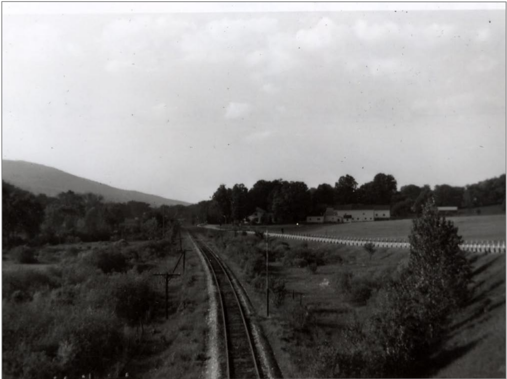
Northbound From Route 7 Bridge Looking to Wallingford 5/30/1962
