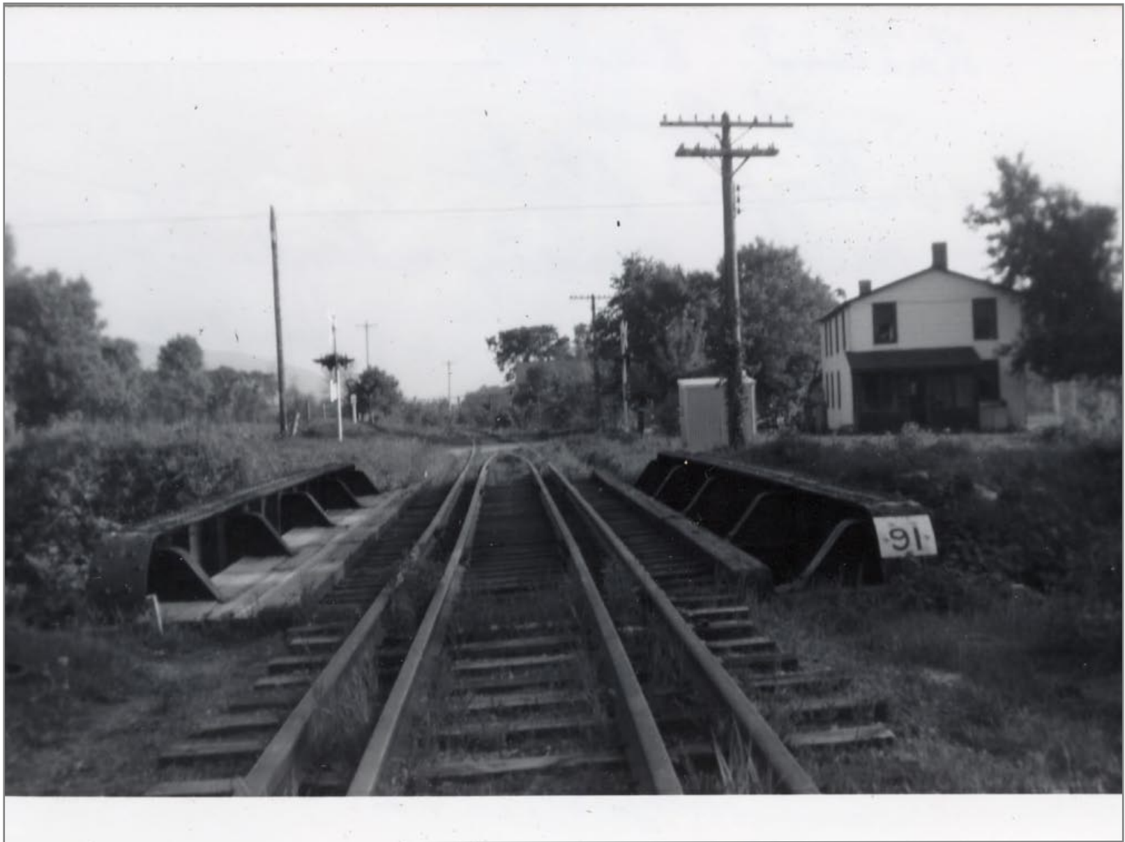
Suthbound thru bridge 91 Wallingford 5/30/1962
