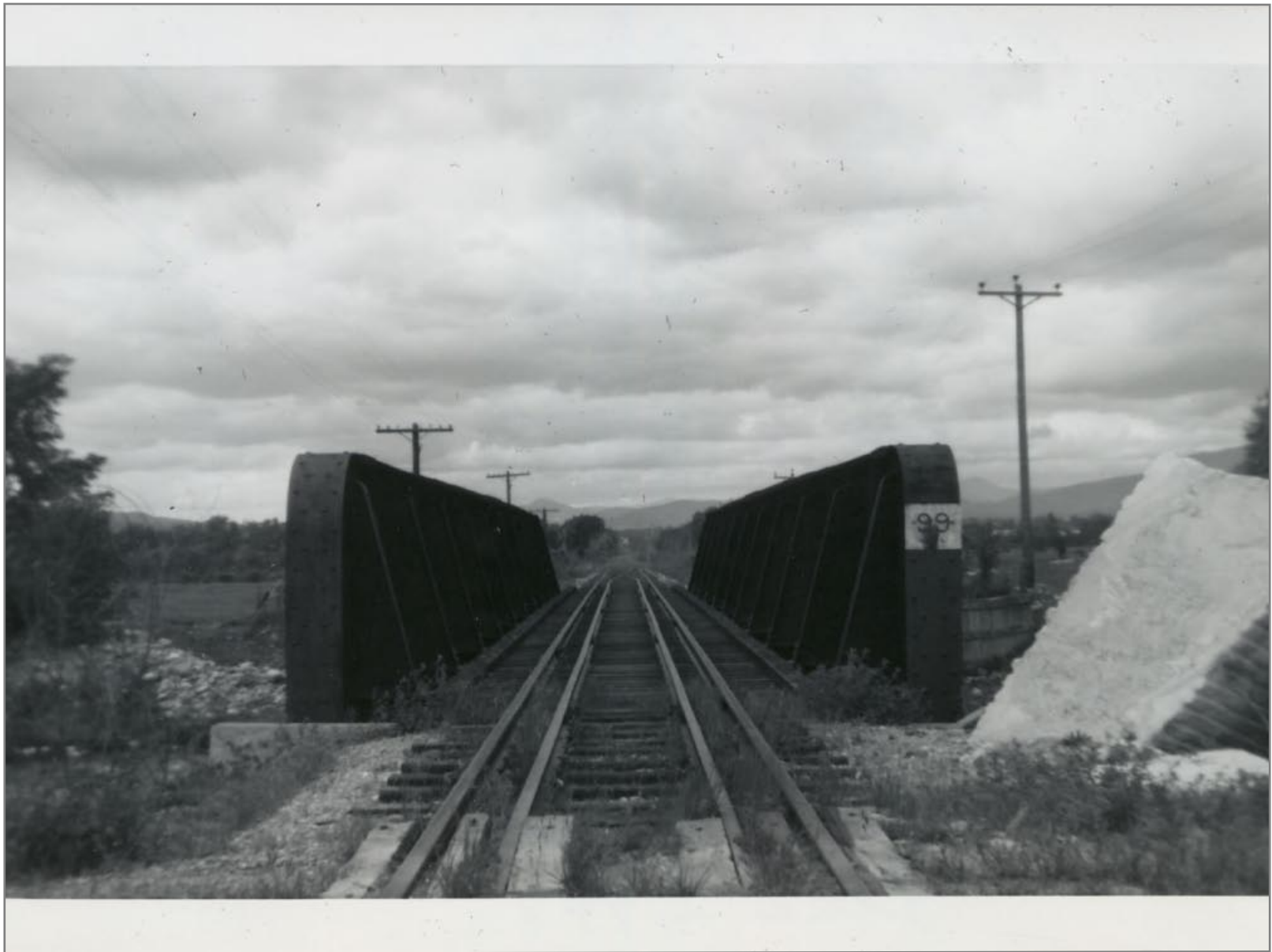
Bridge 99 Northbound American Bridge 1902 6/2/1962
