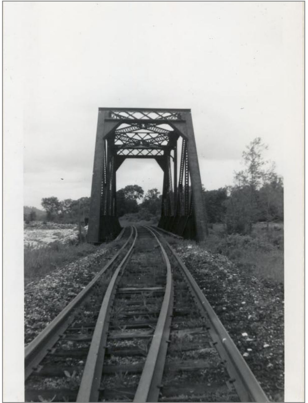
Northbound @ Bridge 93 American Bridge Company BLT 1902
