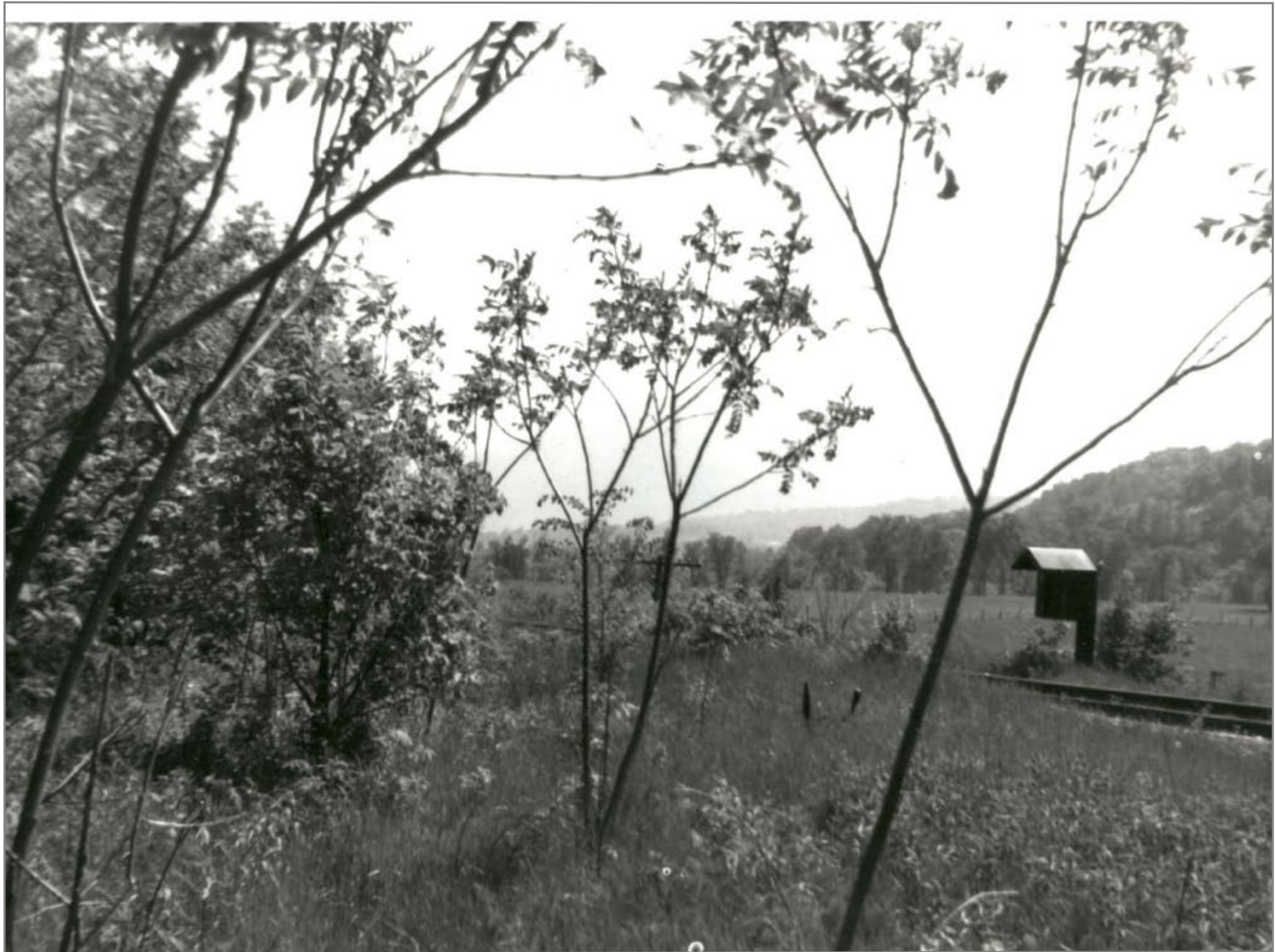
South End of Siding to Gravel Pit 5/30/1962
