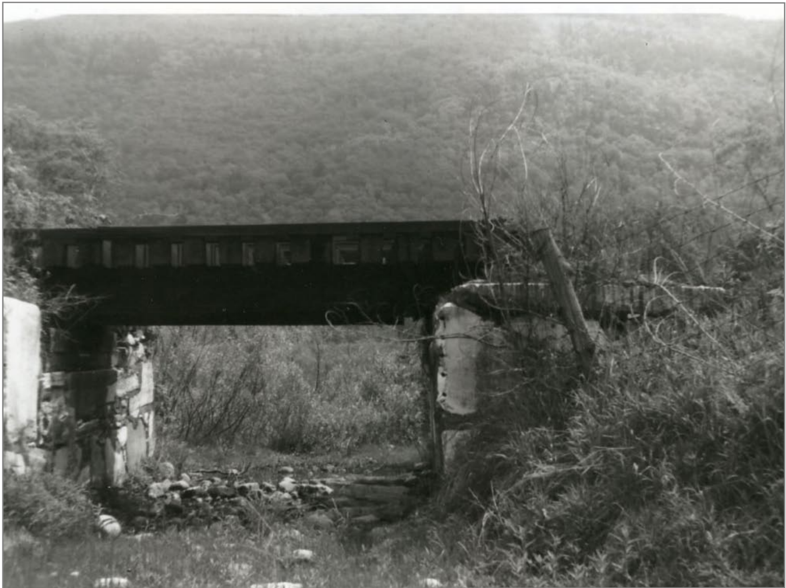
Small Bridge North of Bridge 85 5/30/1962
