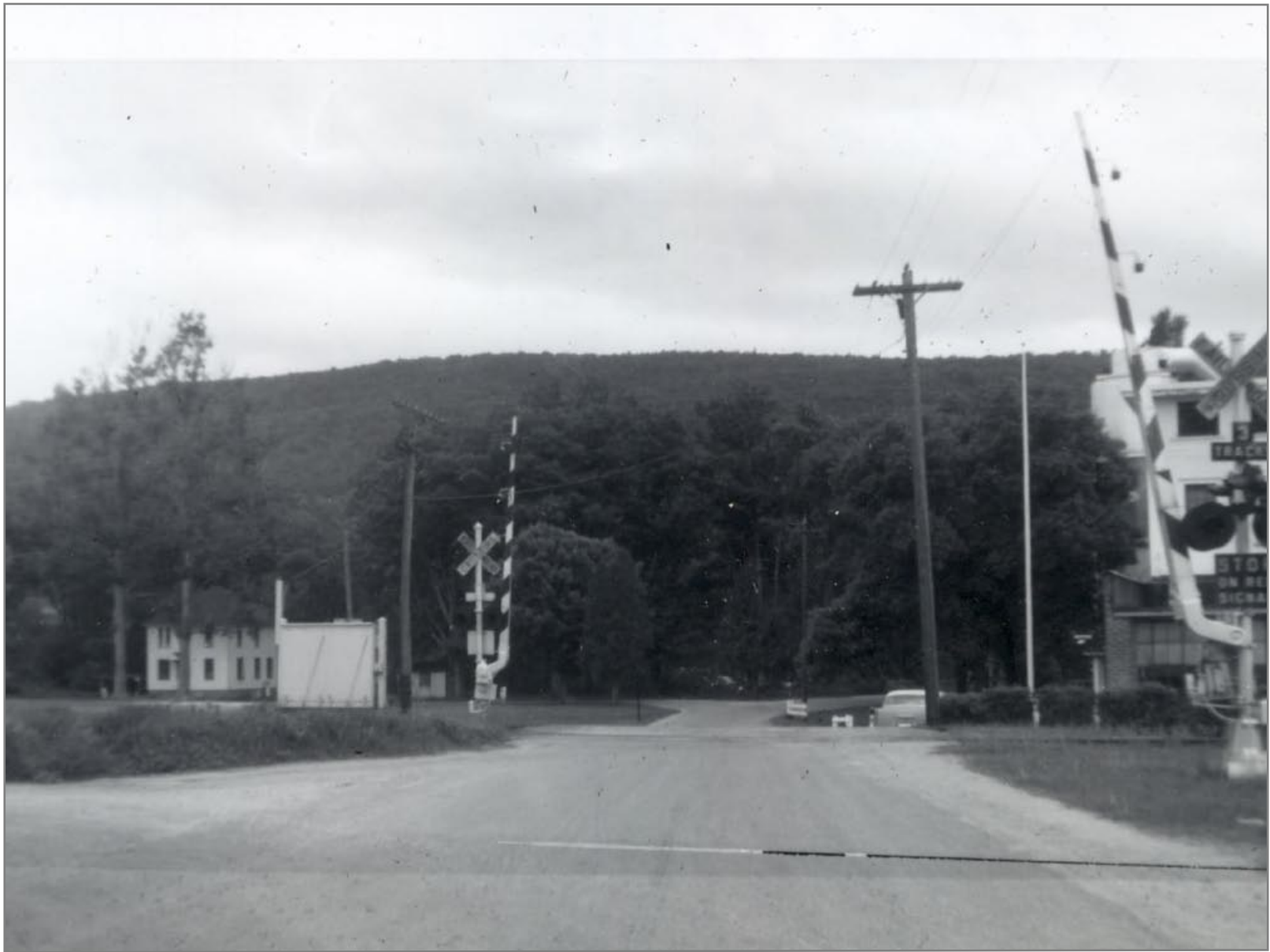
2nd crossing North of Wallingford Station 6/2/1962
