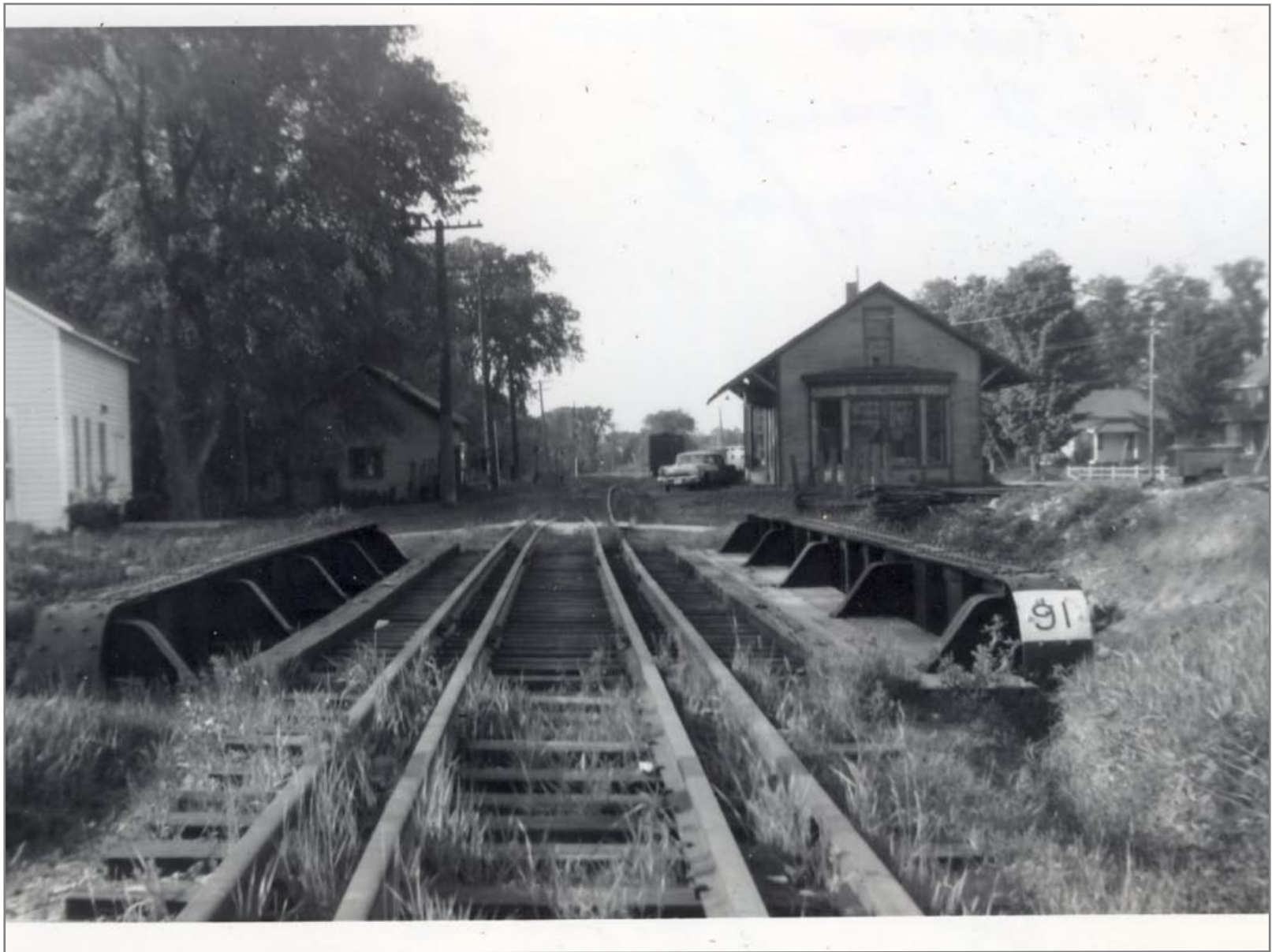
Bridge 91 South of Wallingford Station 5/30/1962
