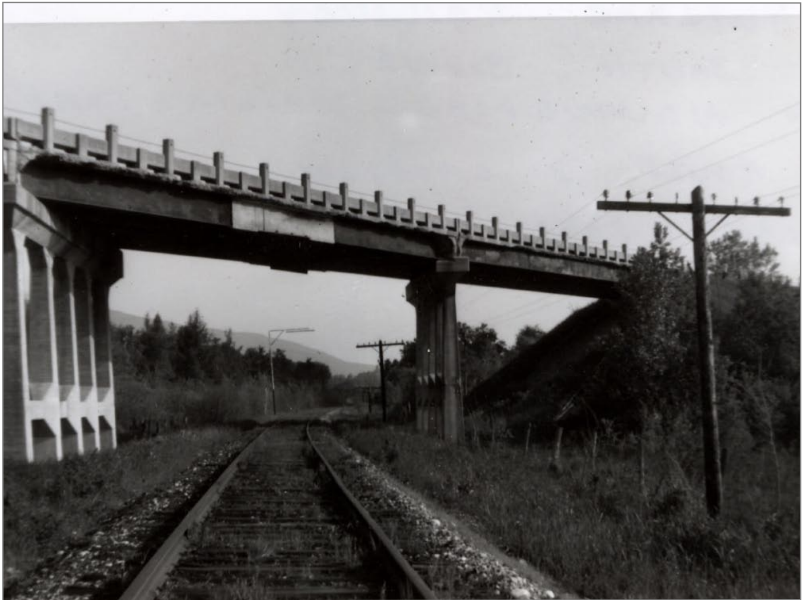
Southbound Looking Under Route 7 Bridge #350 BLT, 1937 5/30/1962
