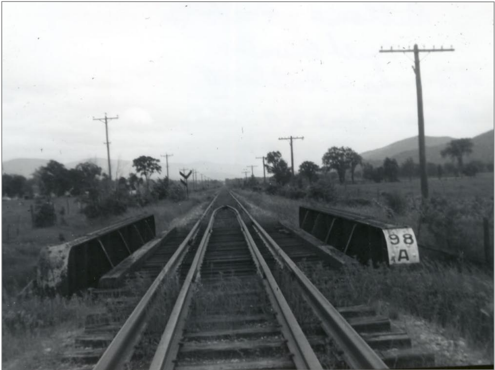
Bridge 98A Southbound Bethlehem Steel Company 1927
