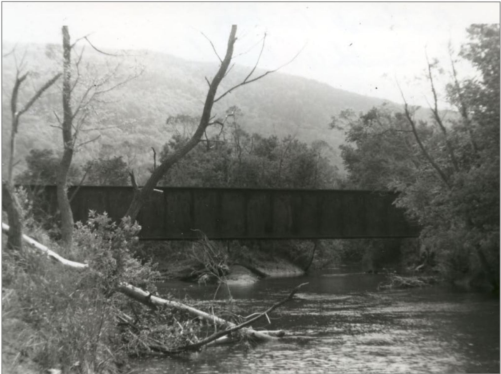
Bridge 85 American Bridge Company 1903 5/30/1962
