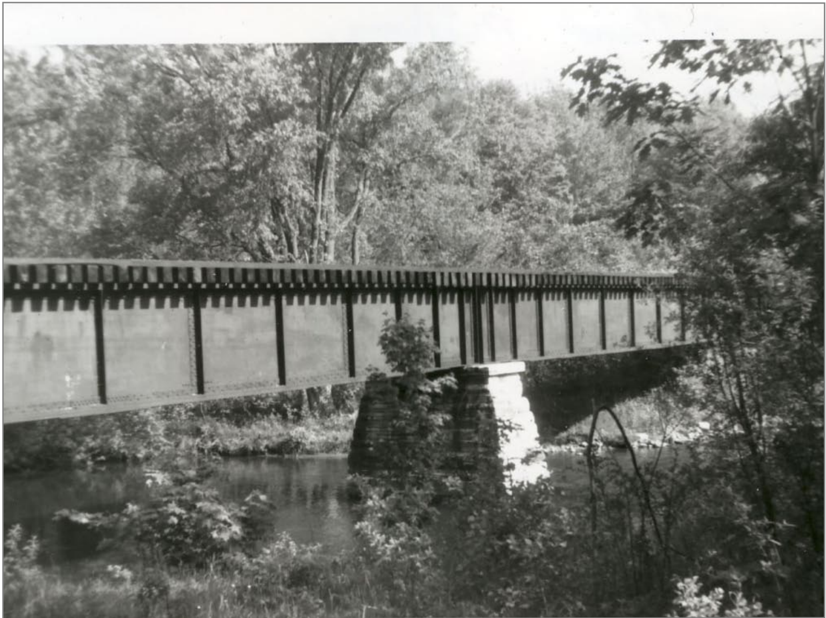
Bridge North of South Wallingford 5/30/1962
