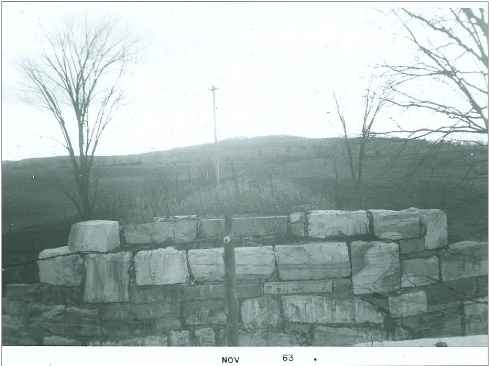
Baldwin Dry Bridge Westbound at Whinting/Shoreham Town Line
