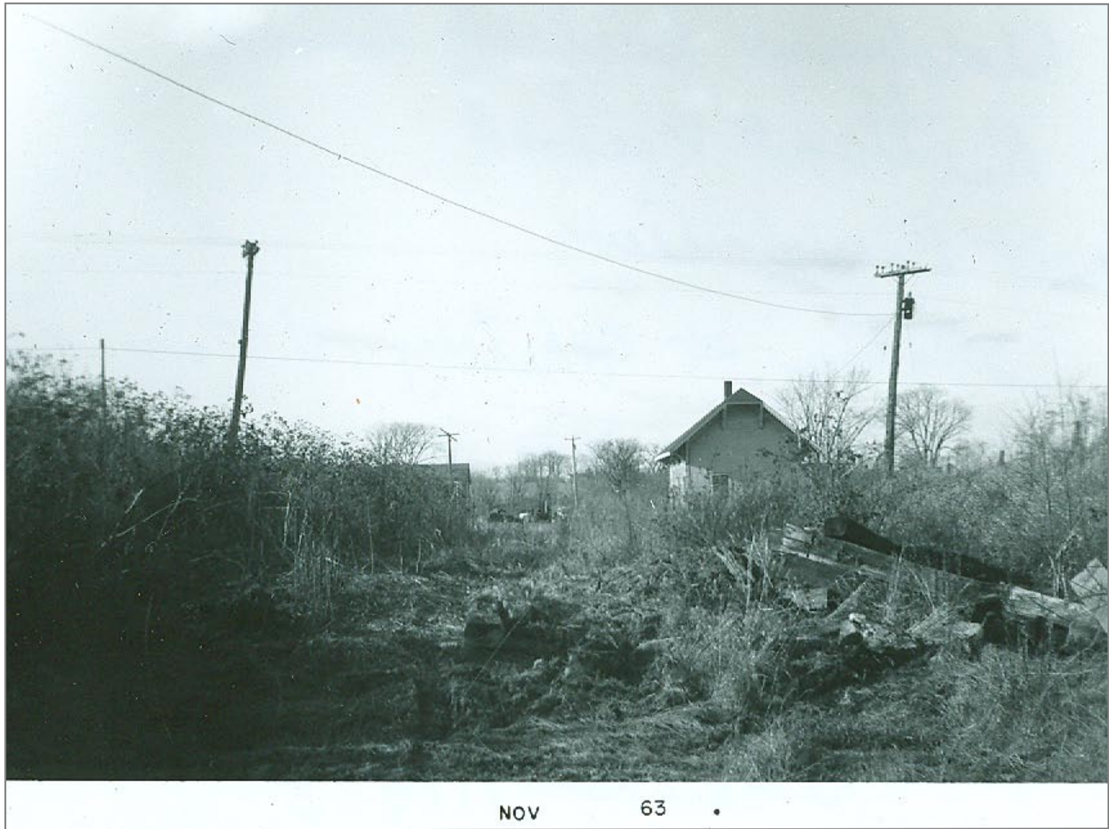
Whiting Station on right westbound
