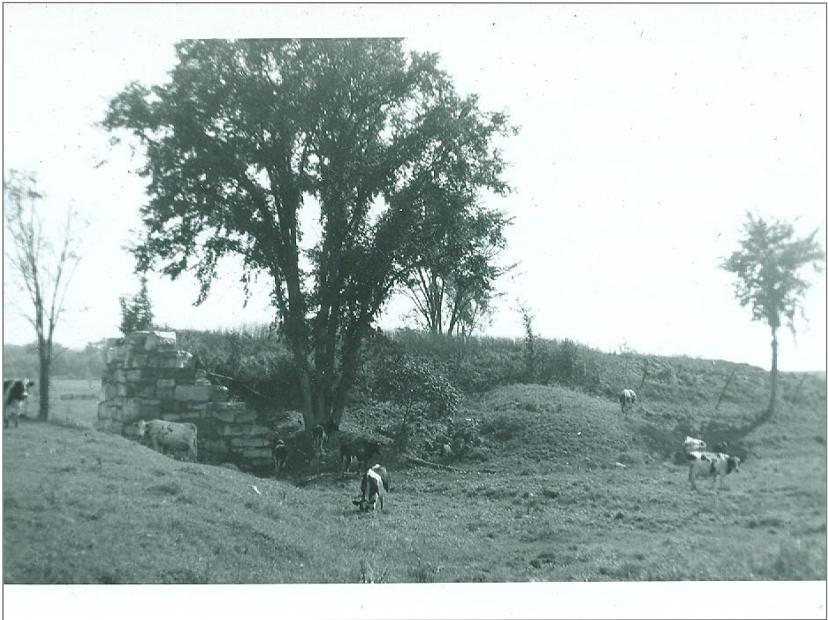
Shoreham Farm Road Crossing
