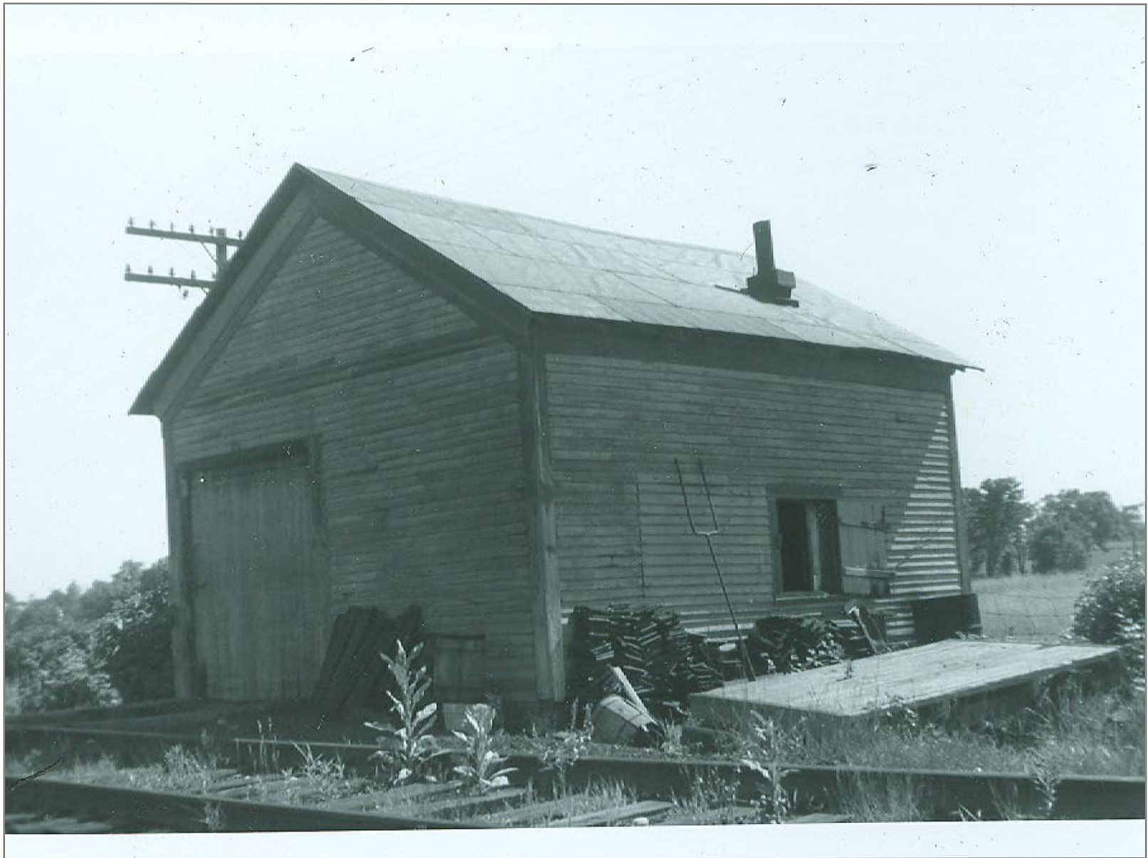
Vergennes Section House 1963
