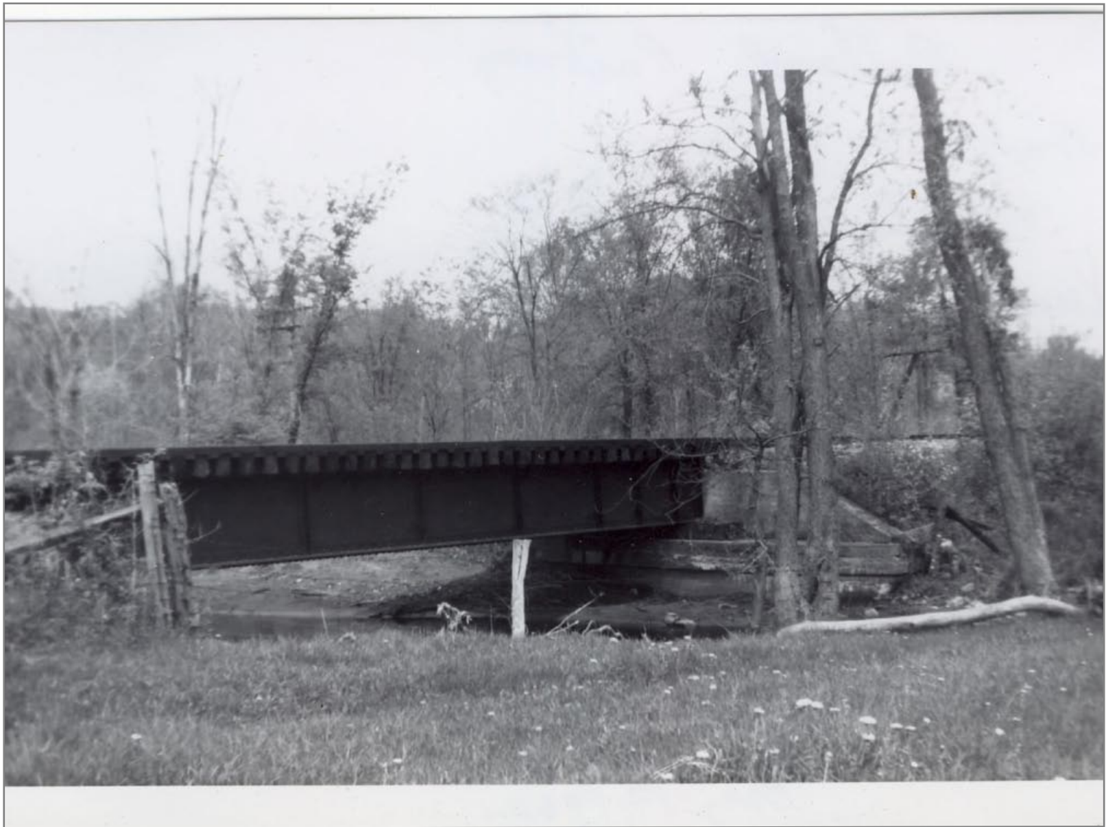
Bridge 67 Looking West 5/20/1962
