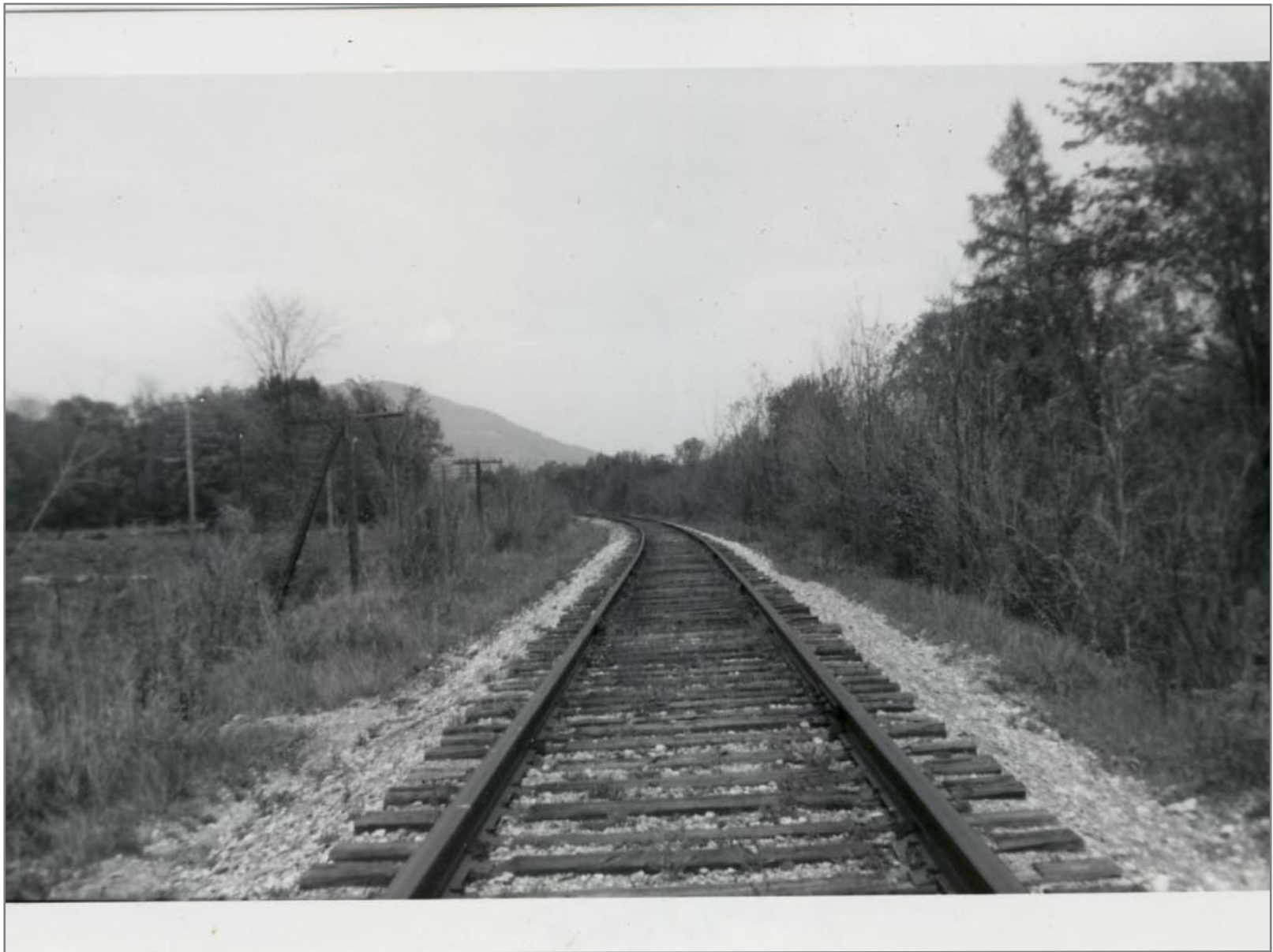
Northbound by MP 22 5/20/1962
