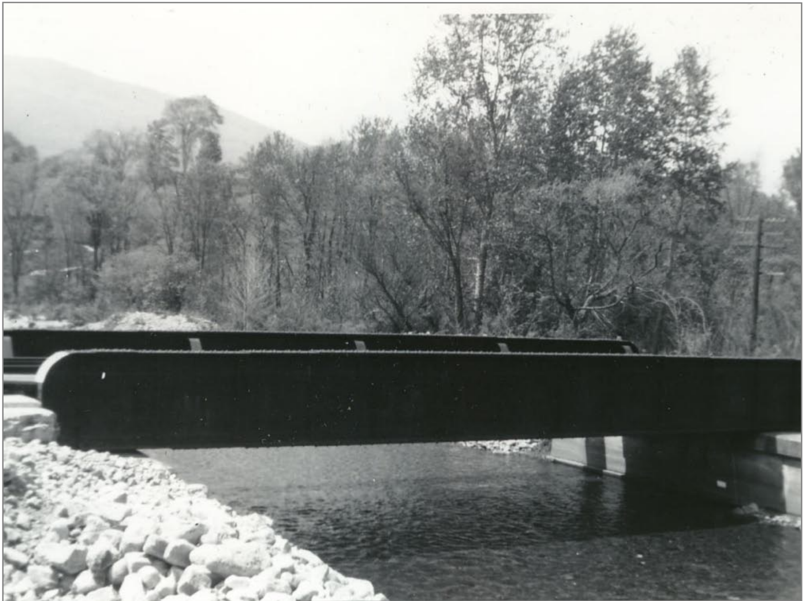
Bridge 69 Looking West 5/20/1962
