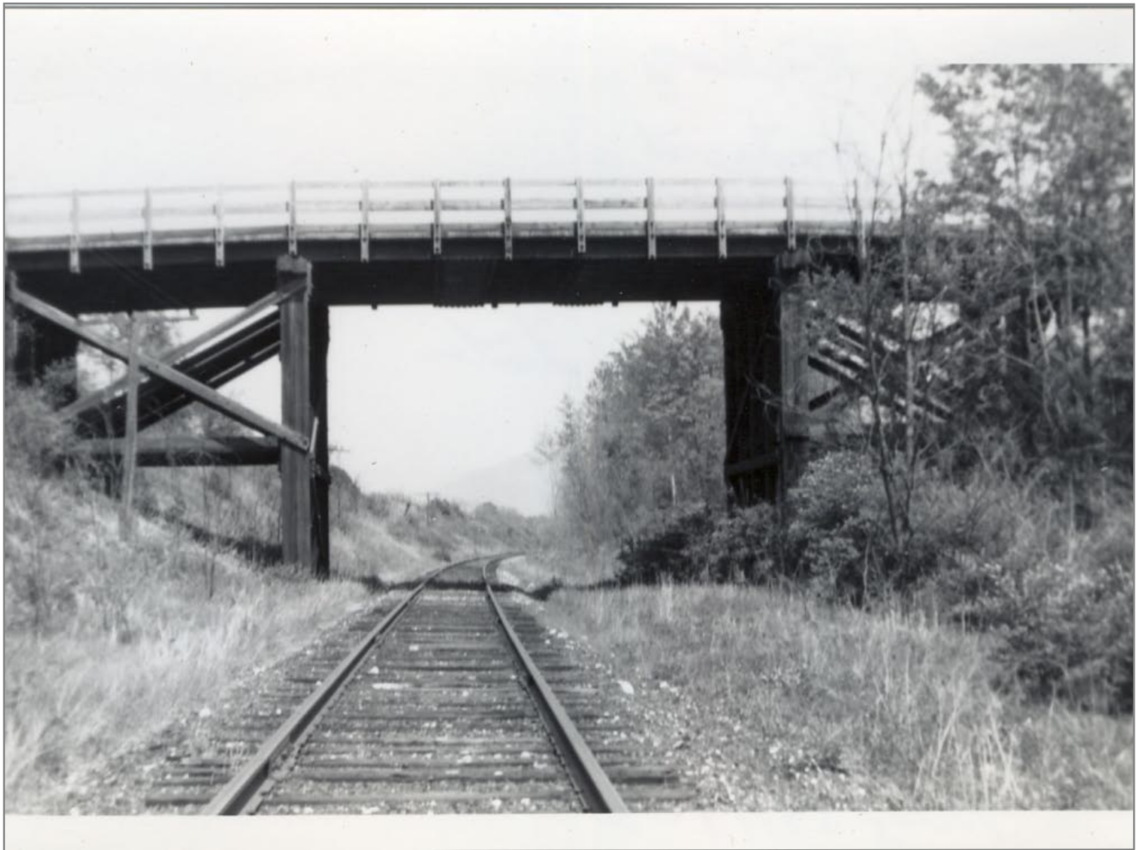
Sunderland Highway Overpass 5/19/1962
