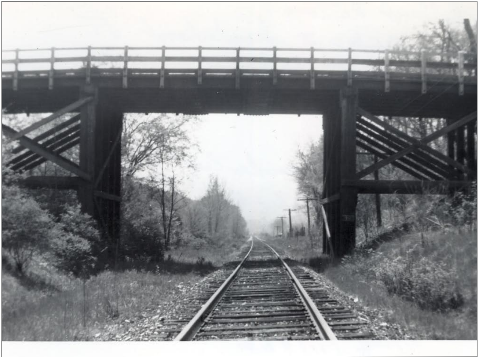
Sunderland Highway Bridge Built 1932 Looking Southbound Bridge #62A 5/19/1962
