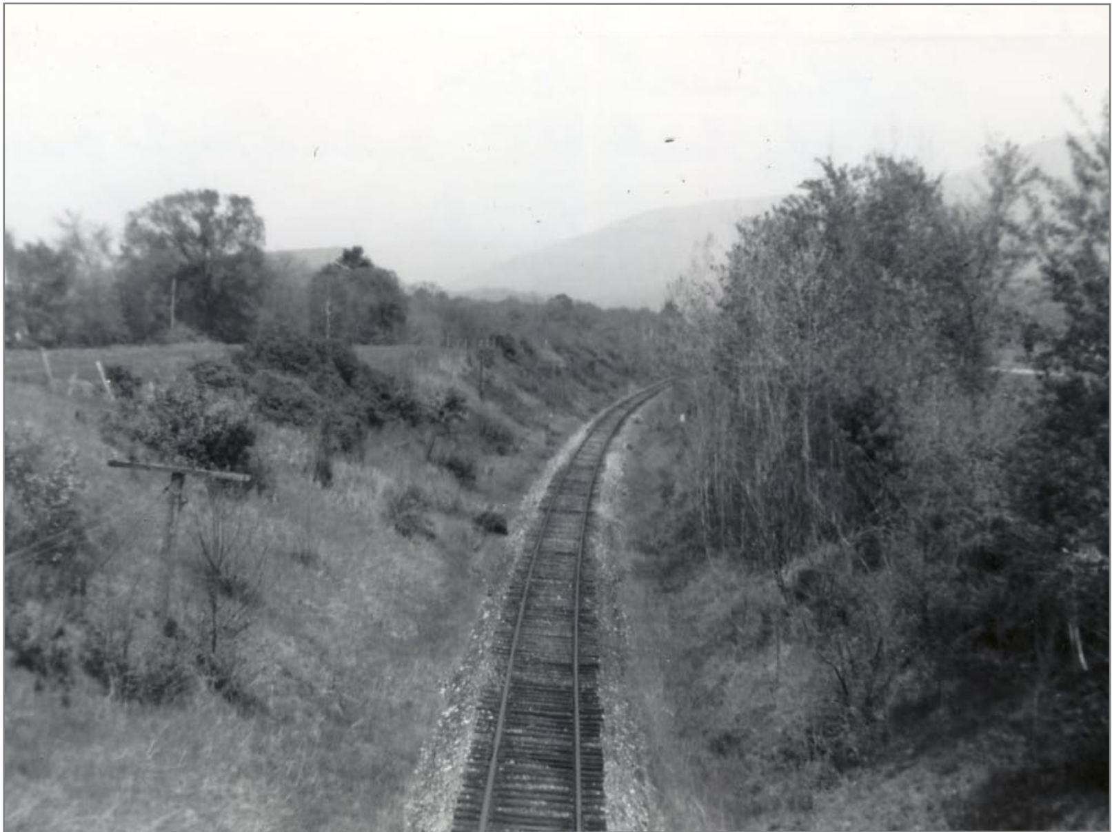
Northbound From Highway Overpass Toward MP 17 on Right 5/19/1962
