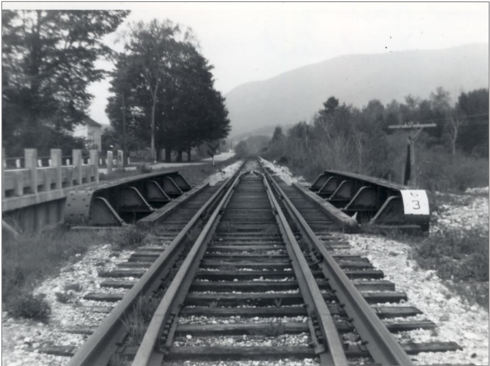
Bridge #63 Southbound Over Mill Stream Built By American Bridge Company 1903 5/19/1962
