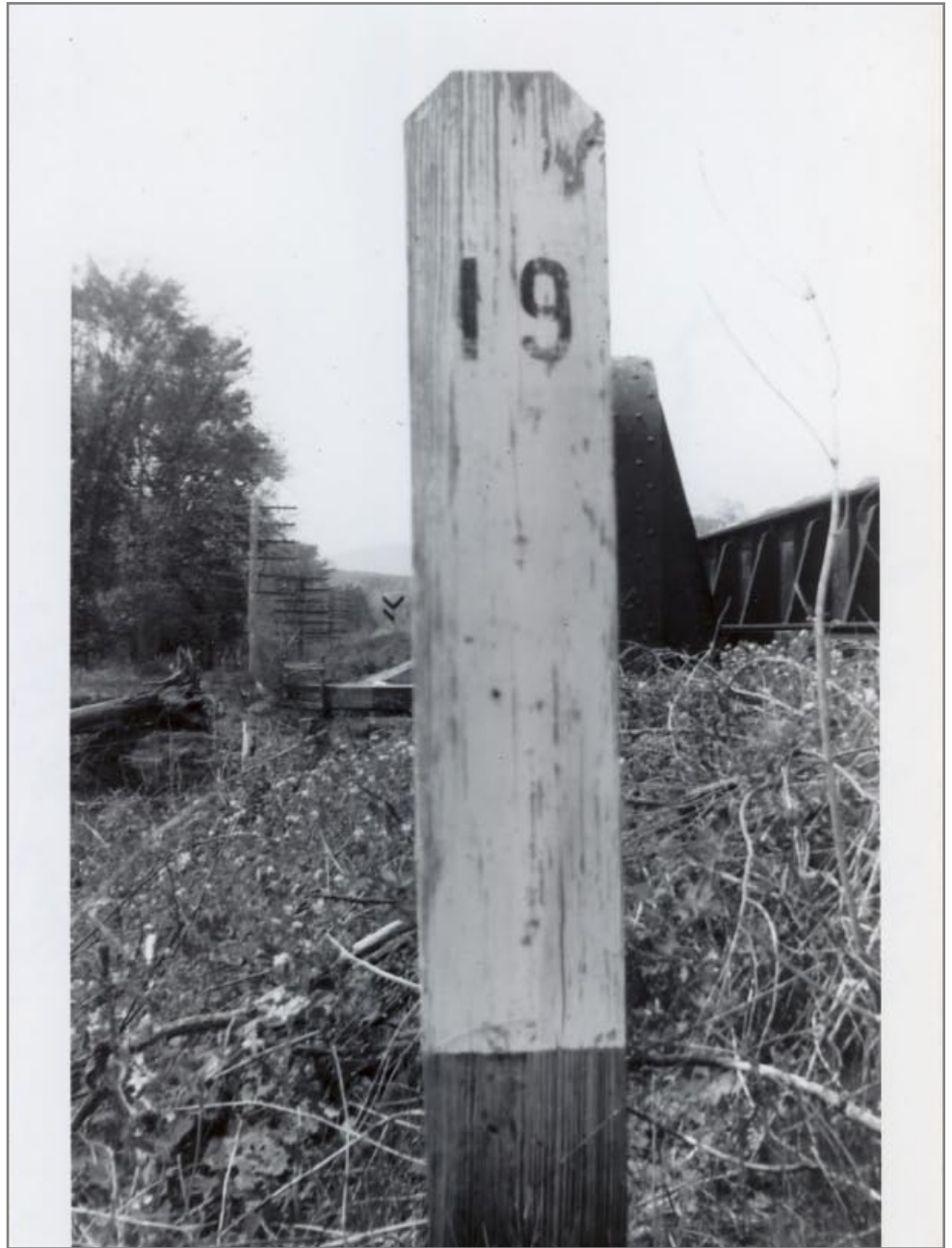
Milepost 19 w/ Bridge 65 in Background 5/20/1962
