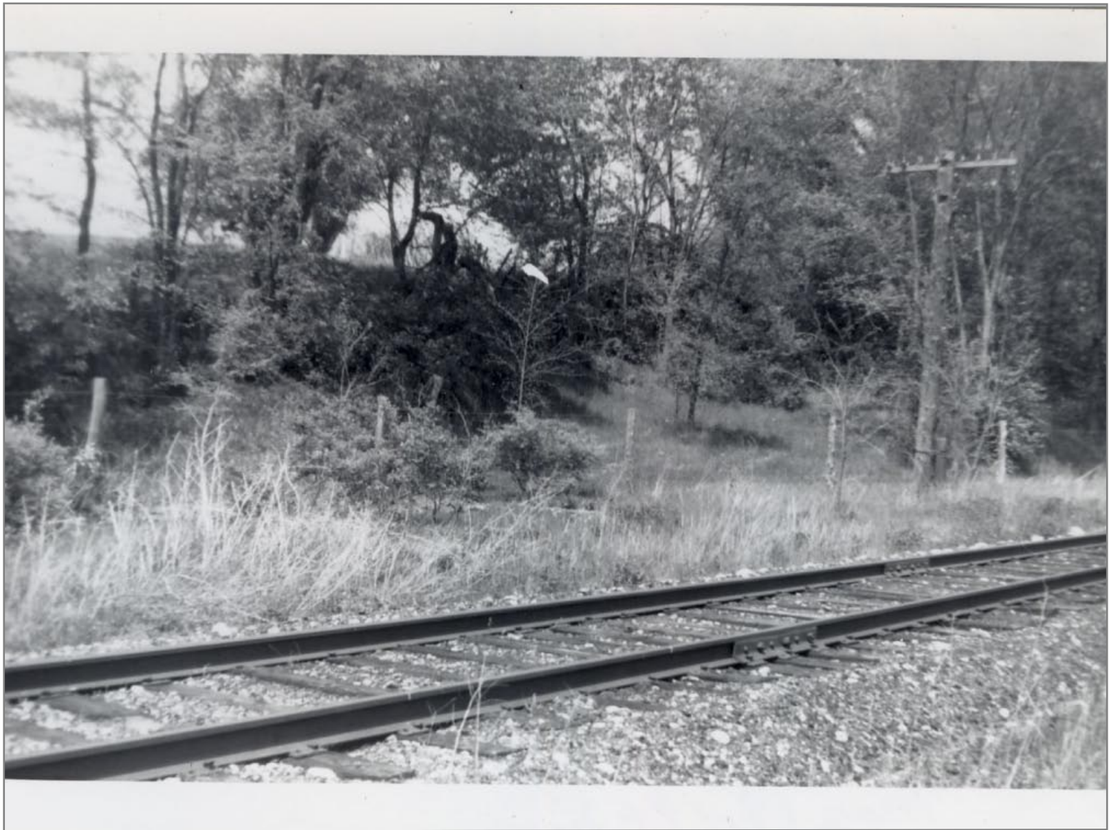
Site of Station Just South of Highway Overpass Looking Northbound 5/19/1962
