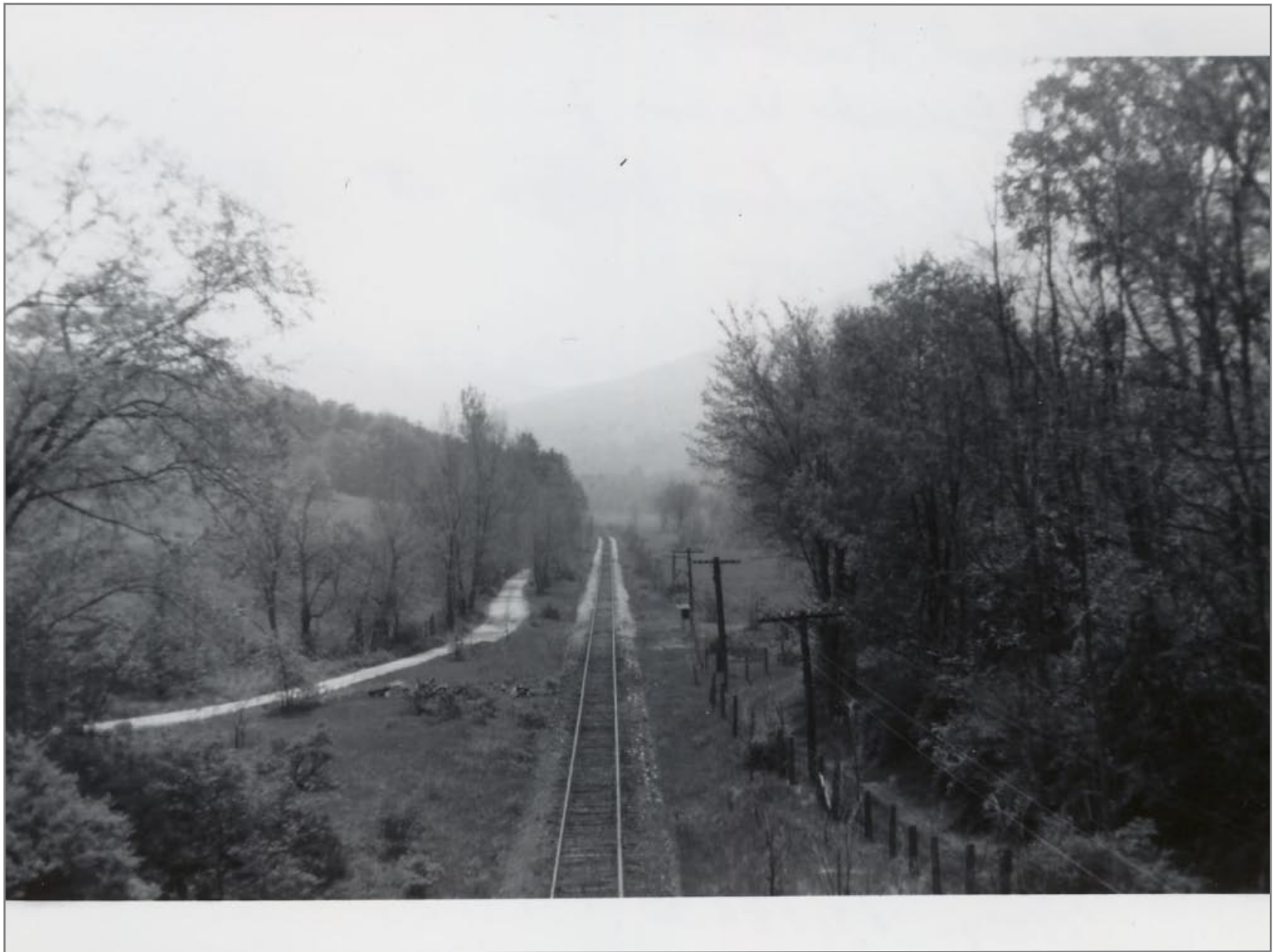
Looking Southbound From Highway Overpass Sunderland Station on Right Near Telephone Box 5/19/1962
