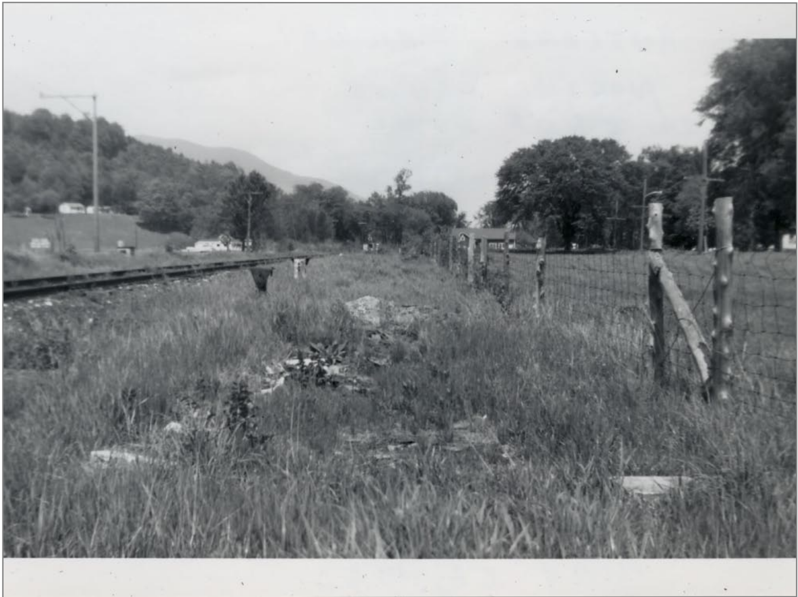
Northbound 5/26/1962 Note Rail Storage Rack on Right
