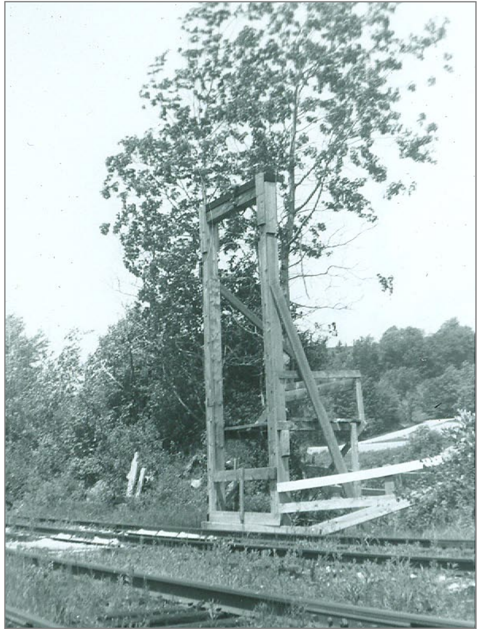
Loading Platform for Stone and Gravel @ Summit
