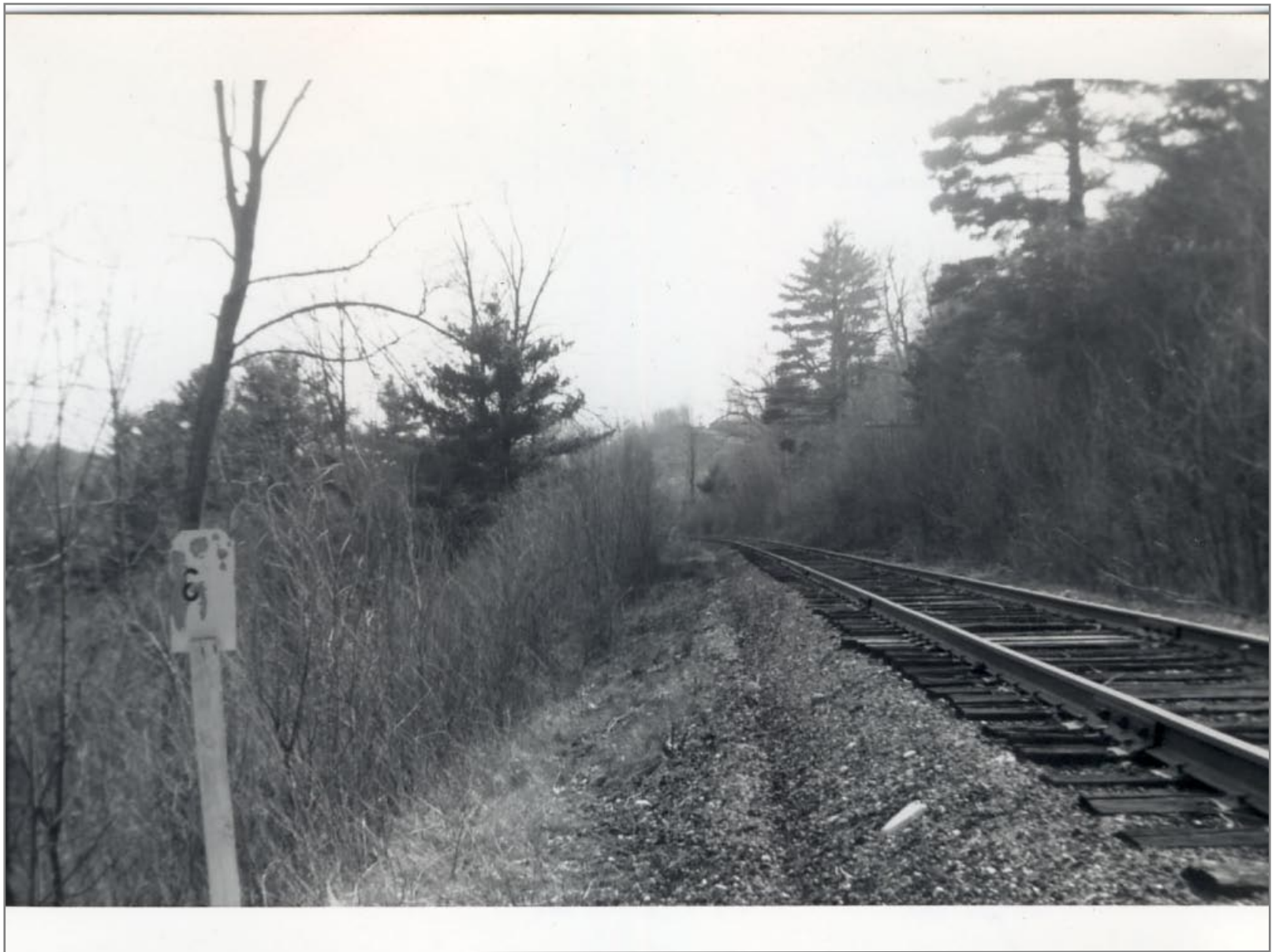
Milepost 6 Looking Southbound 4/21/1962
