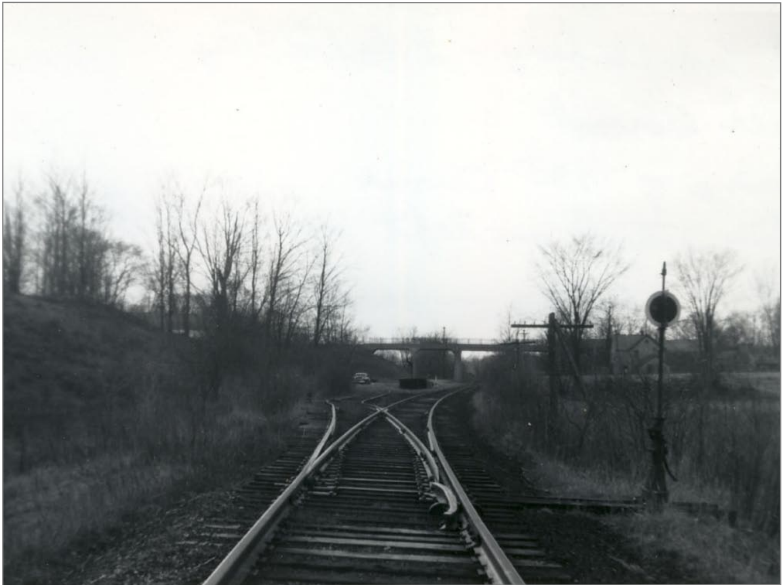
South Shaftsbury Looking South at Route 7 Bridge 4/21/1962
