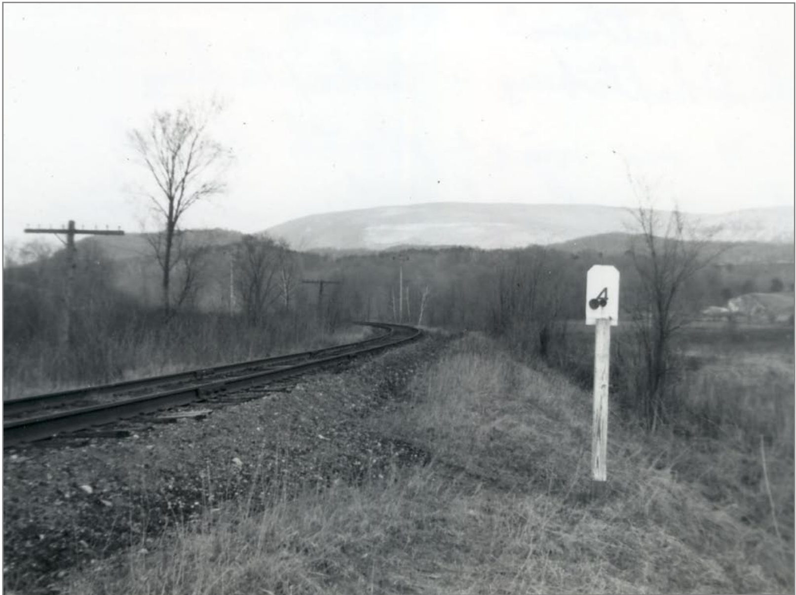
South Shaftsbury Northbound MP #4 4/21/1962
