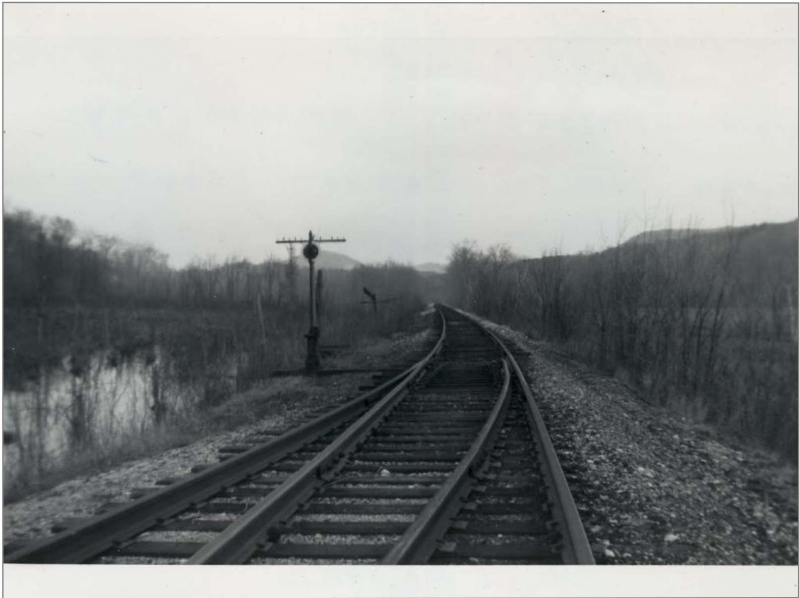
Northbound - Switch into W.E. Dailey Concrete Plant 4/21/1962
