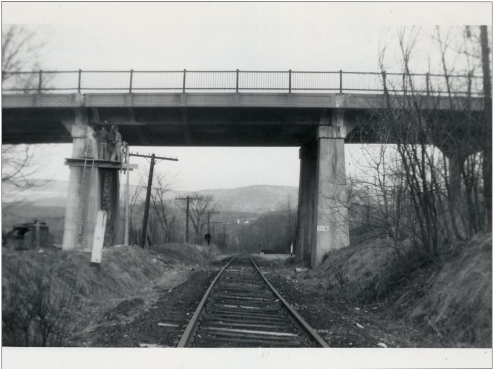
Route 7 Overpass in South Shaftsbury Northbound Bridge #59B 4/21/1962
