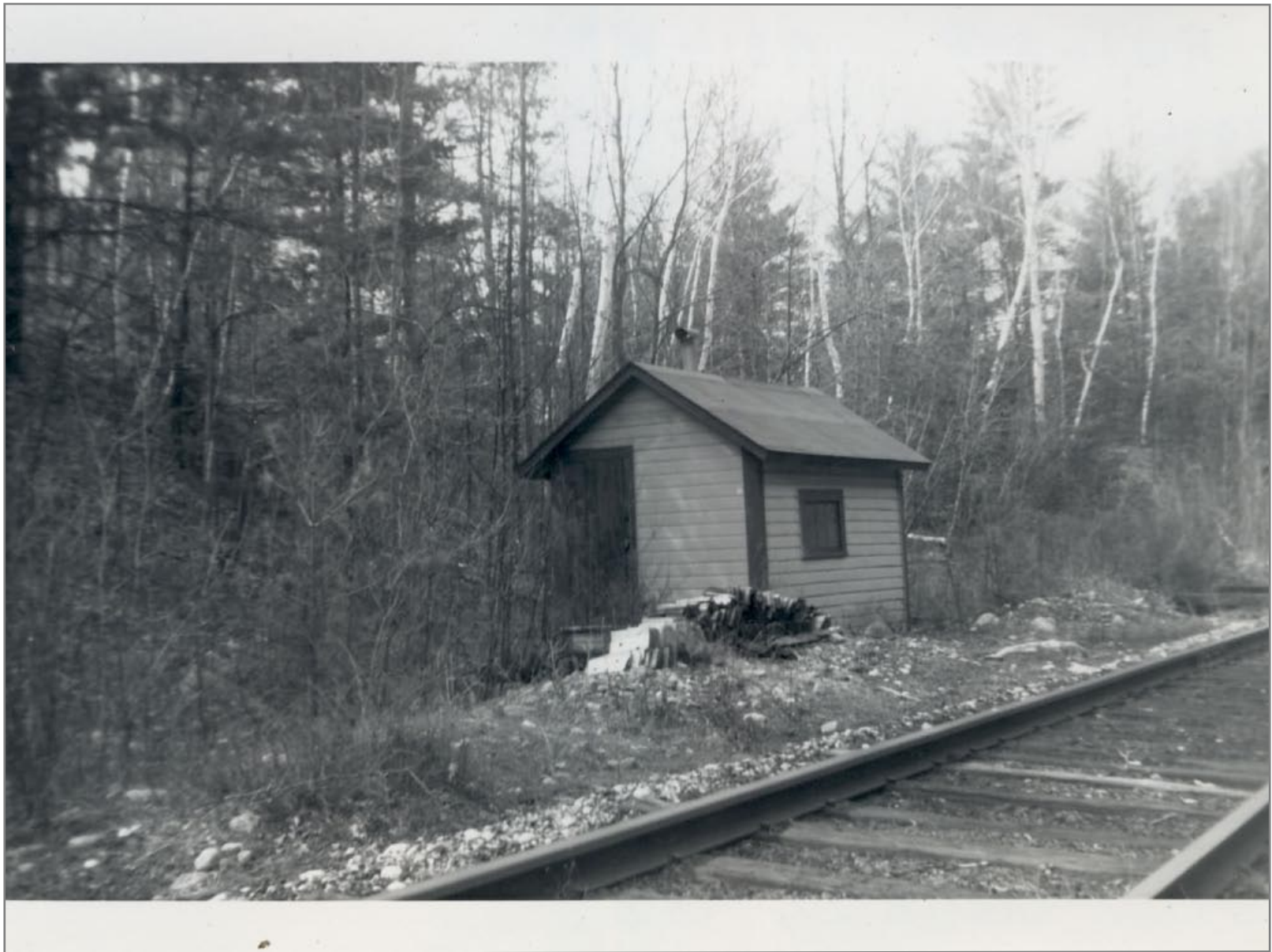
Tool House Between MP 7 & 8 Between South Shaftsbury and Shaftsbury 4/21/1962
