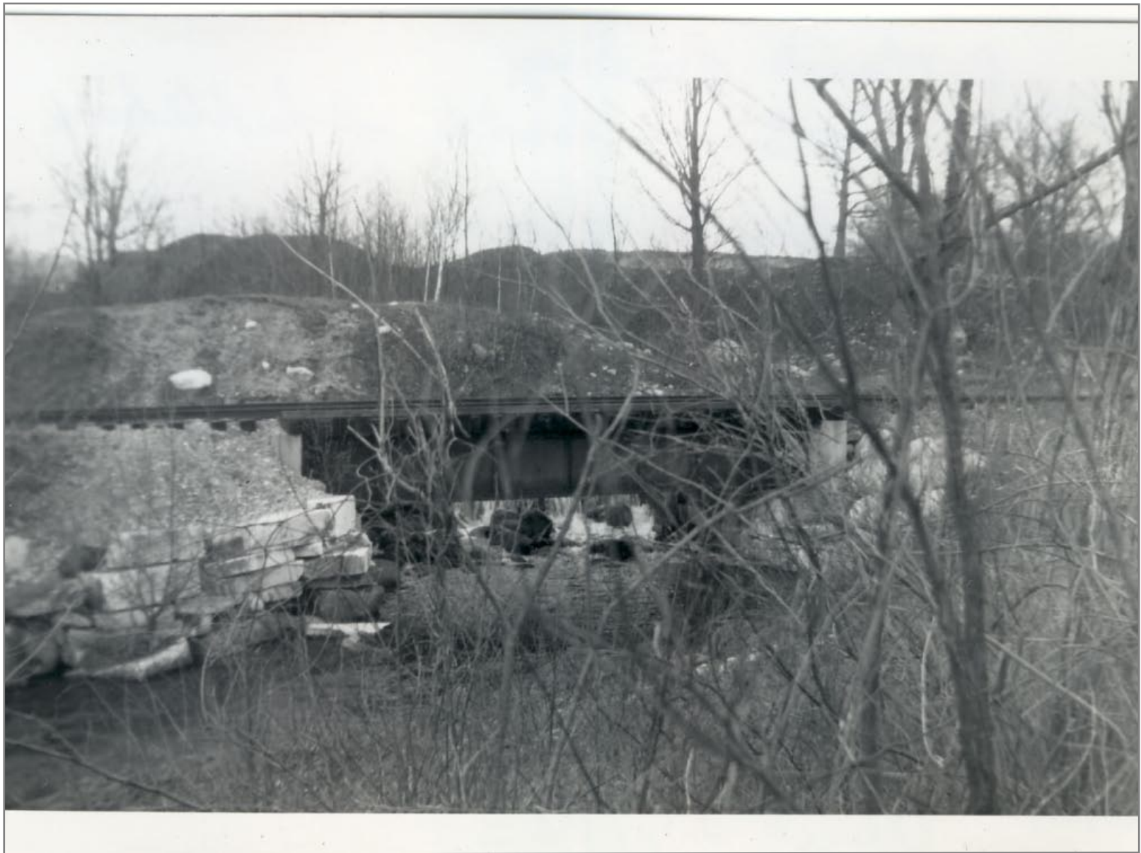
Small Bridge on Spur to Concrete Plant 4/21/1962
