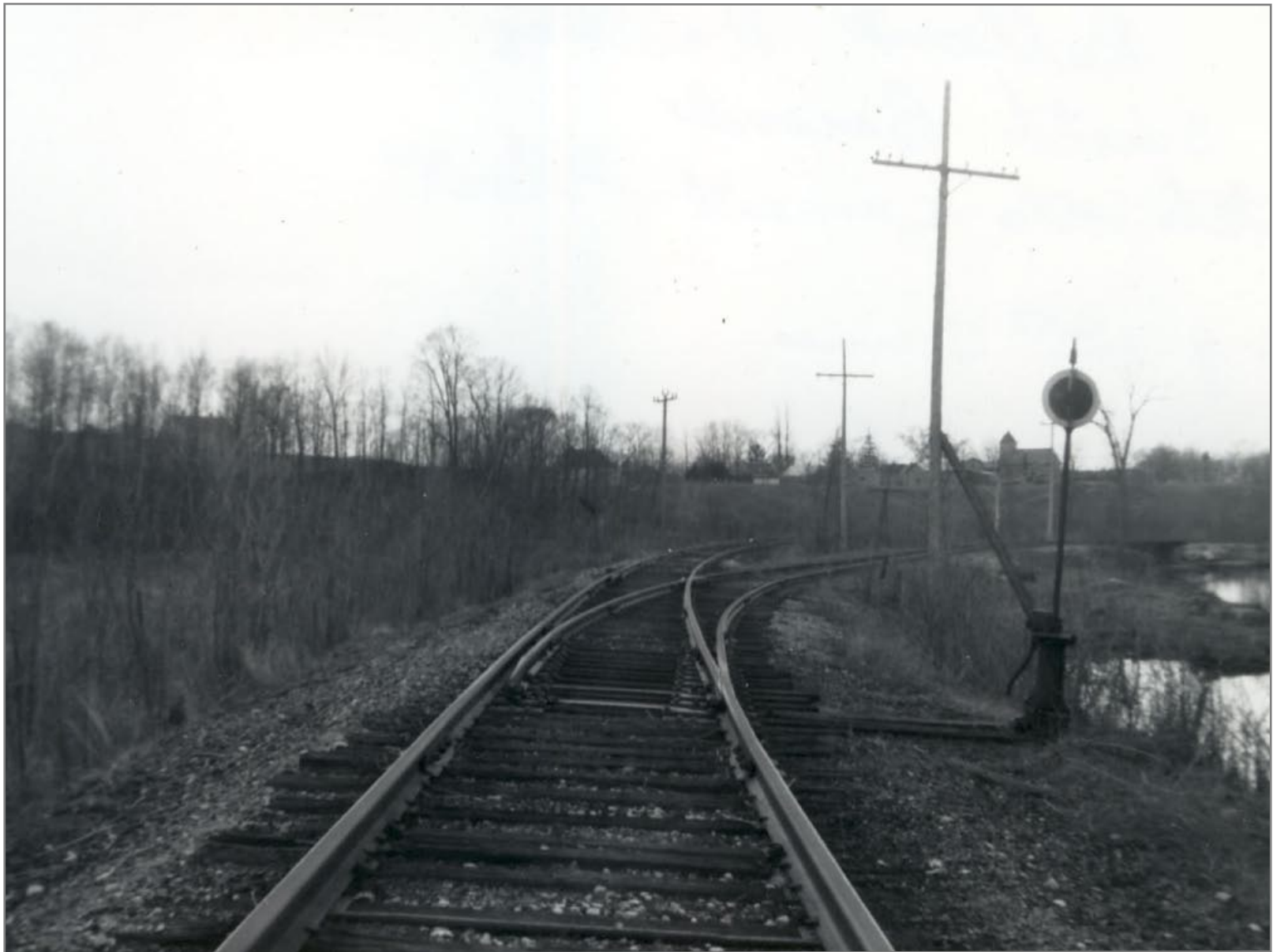
Southbound Looking at Switch into Concrete Plant - Note Small Bridge on Spur 4/21/1962
