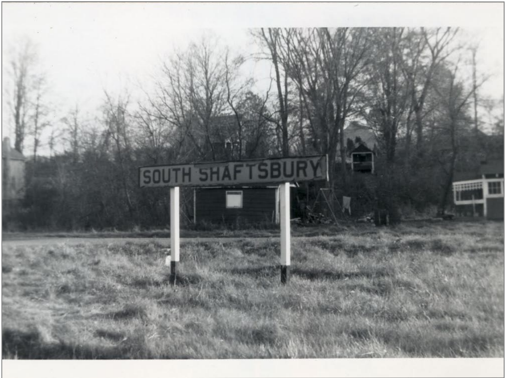
South Shaftsbury Station Site 11/12/1961
