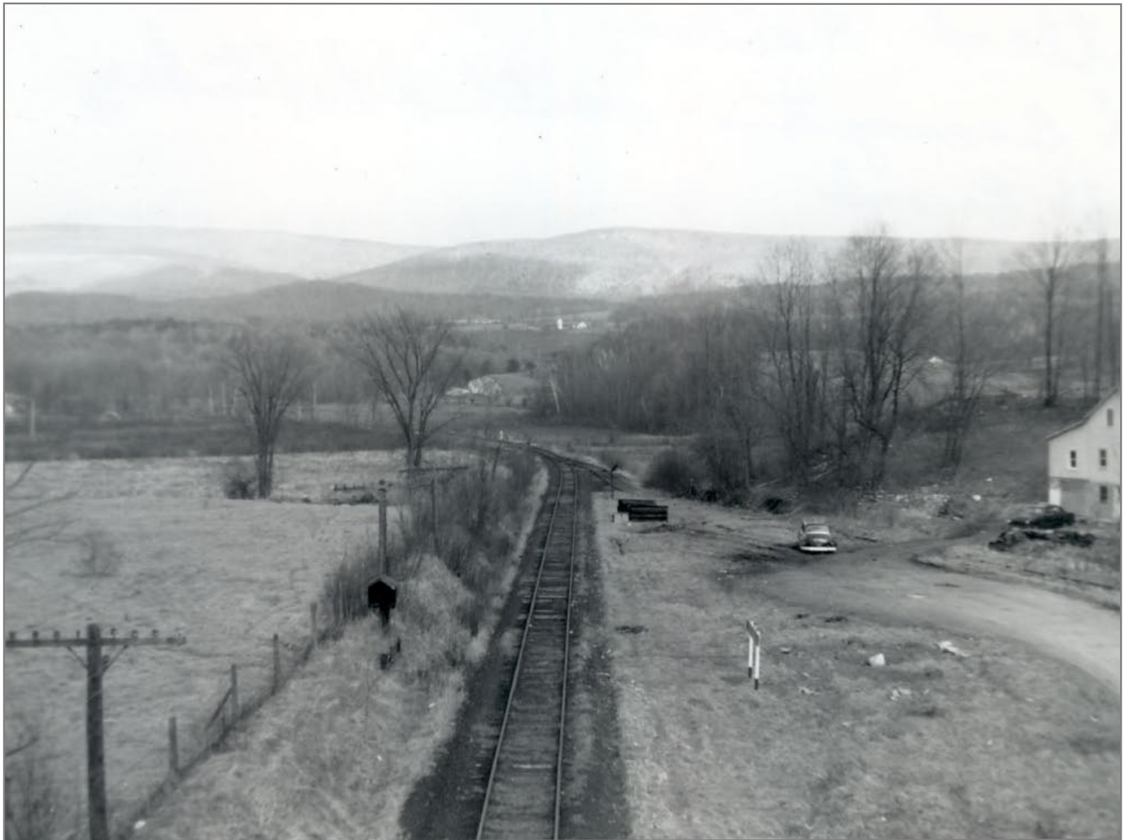
Northbound From Route 7 Bridge - South Shaftsbury Station Site on Right 4/21/1962
