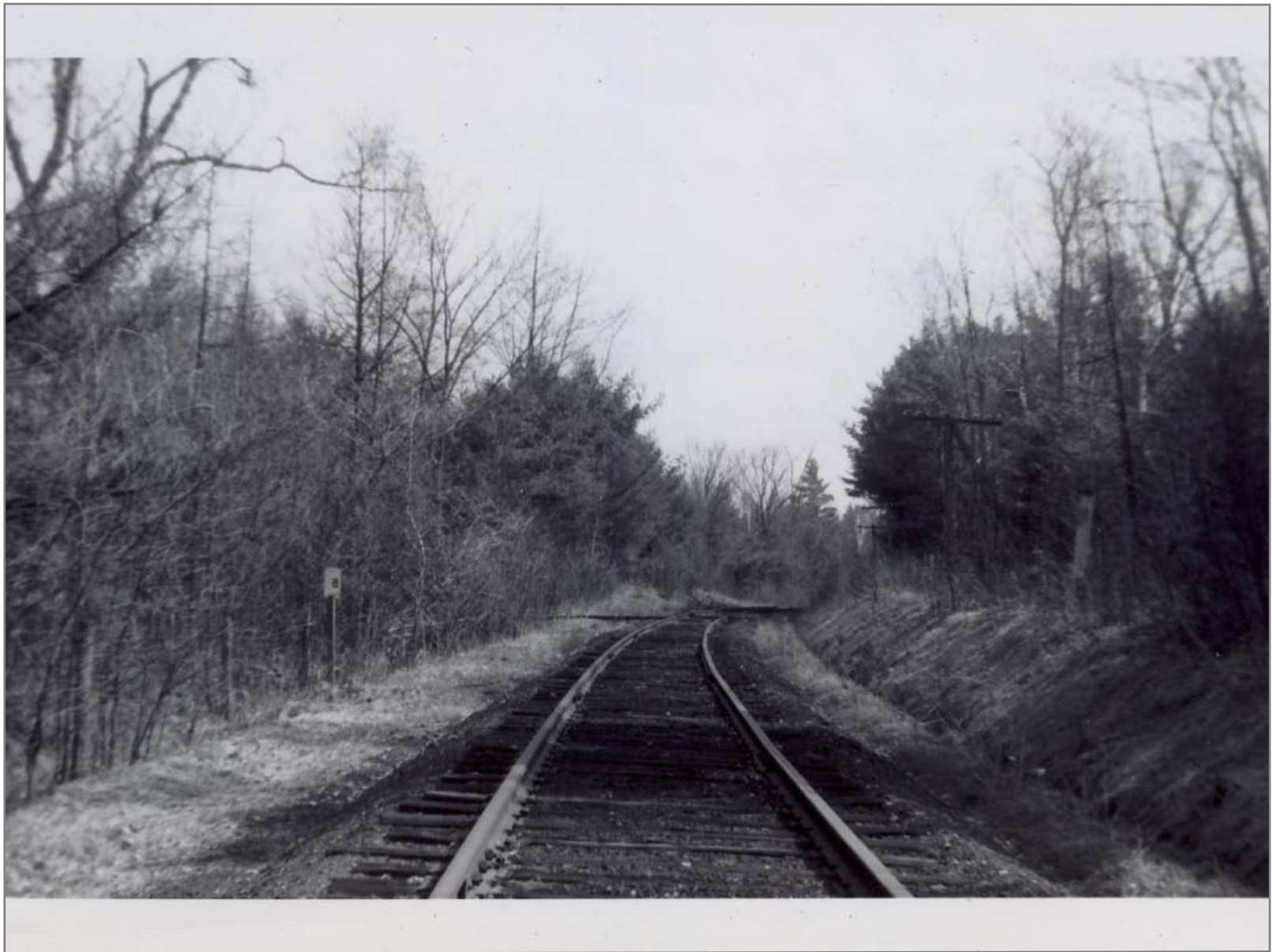
MP 8 on Left Looking Southbound 4/21/1962
