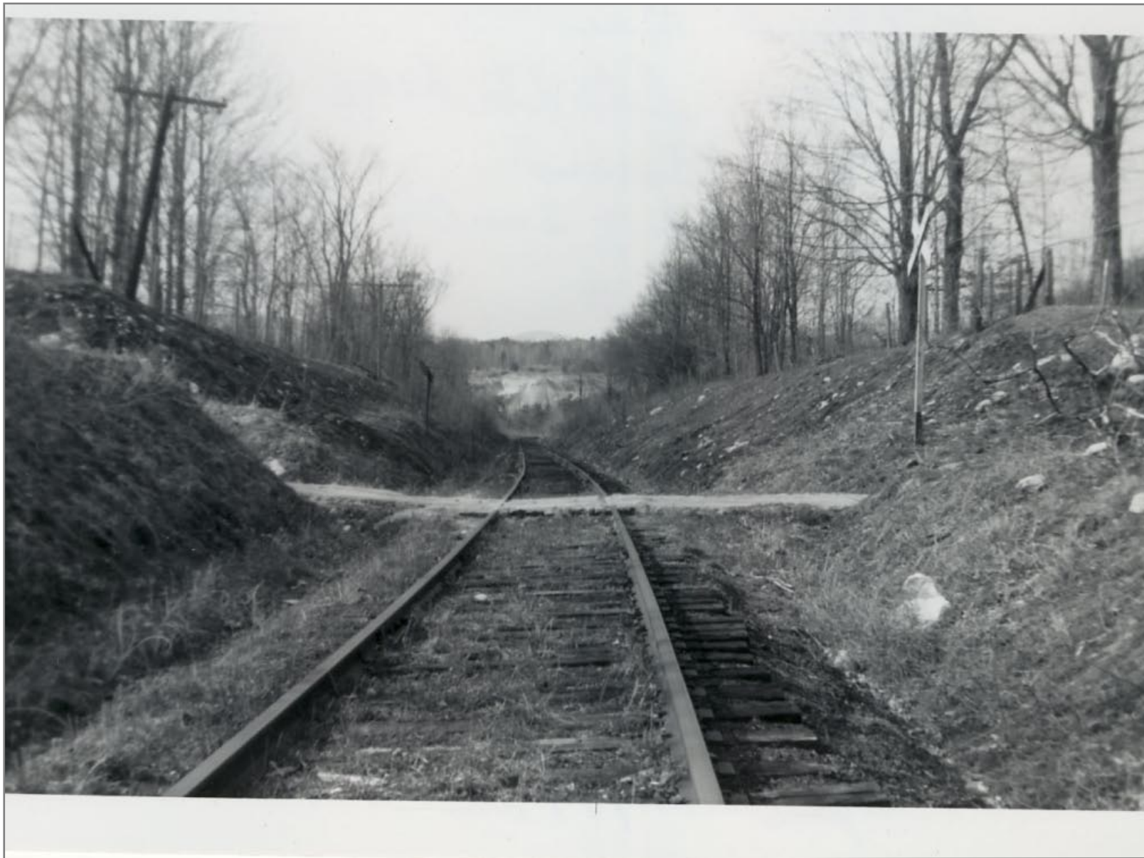
First Crossing North of So. Shaftsbury Looking North 4/21/1962
