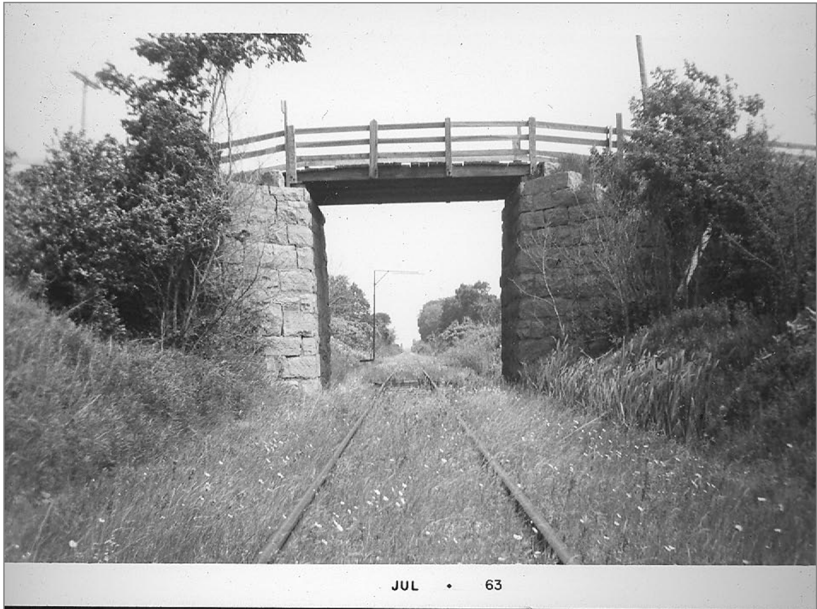
Northbound Bridge 272 South Hero
