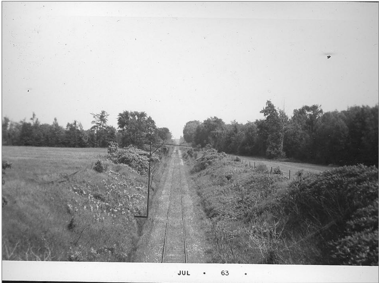
Northbound Bridge 272 South Hero
