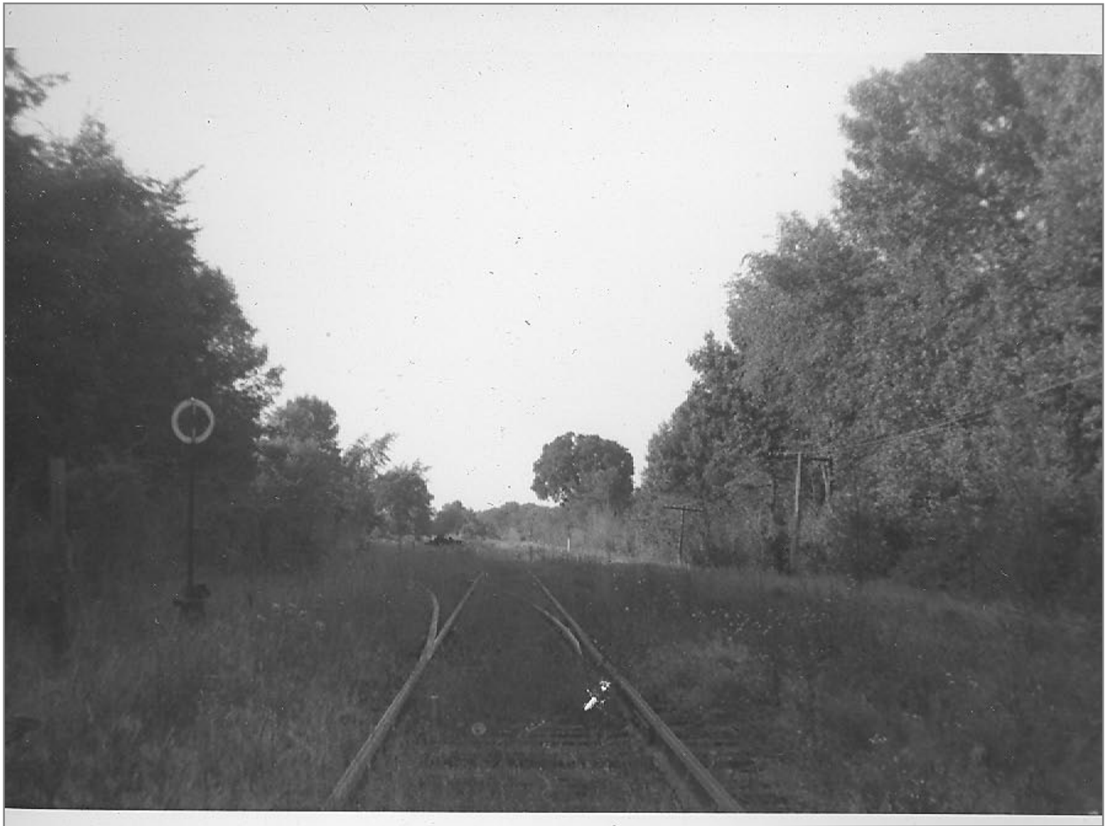
Northbound @ So. Hero Station 8/62
