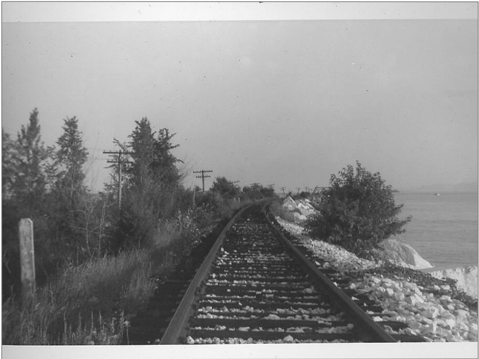
Southbound @ MP 133 Bridge 270 in Background 8/10/62
