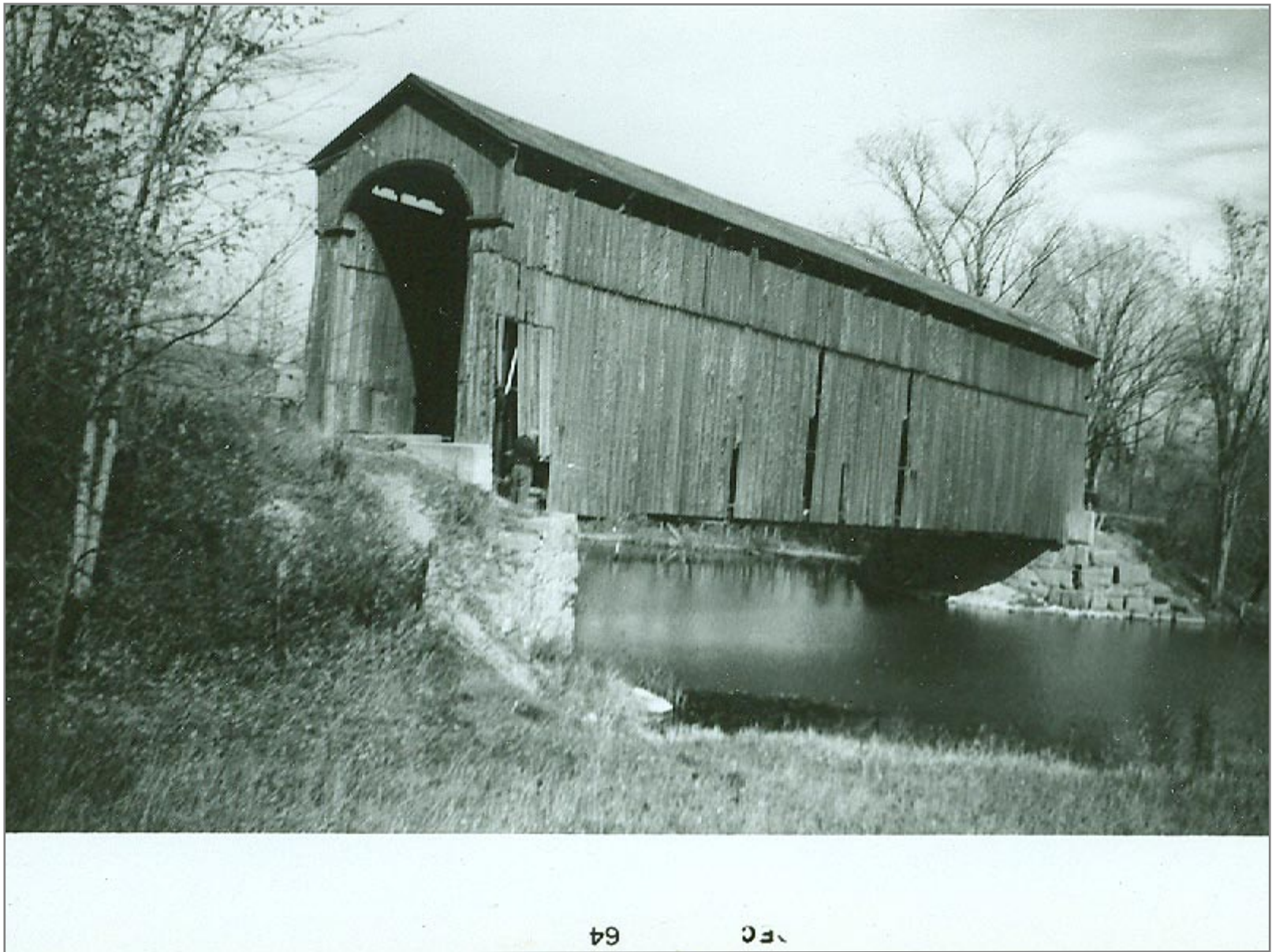
East Shoreham Covered Bridge
