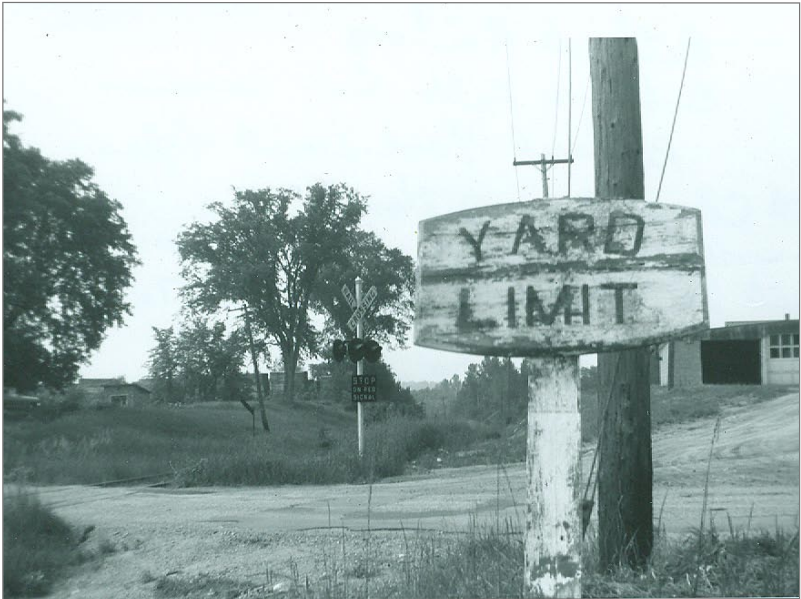
Northbound Rutalnd Yard Limit about 20 feet north of MP 51
