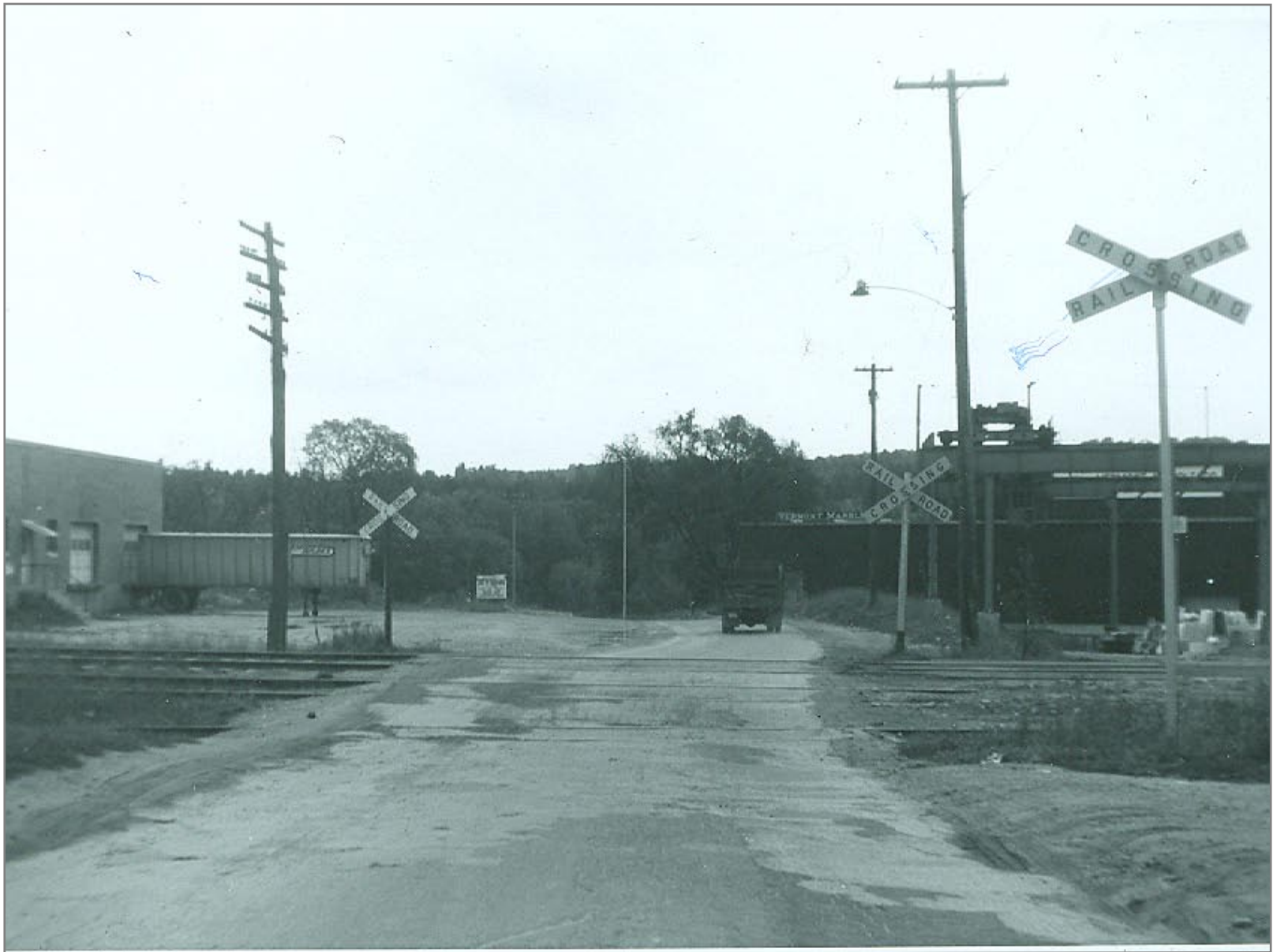
Looking west toward Vt Marble Plant on right - Ctr. Rutland to right
