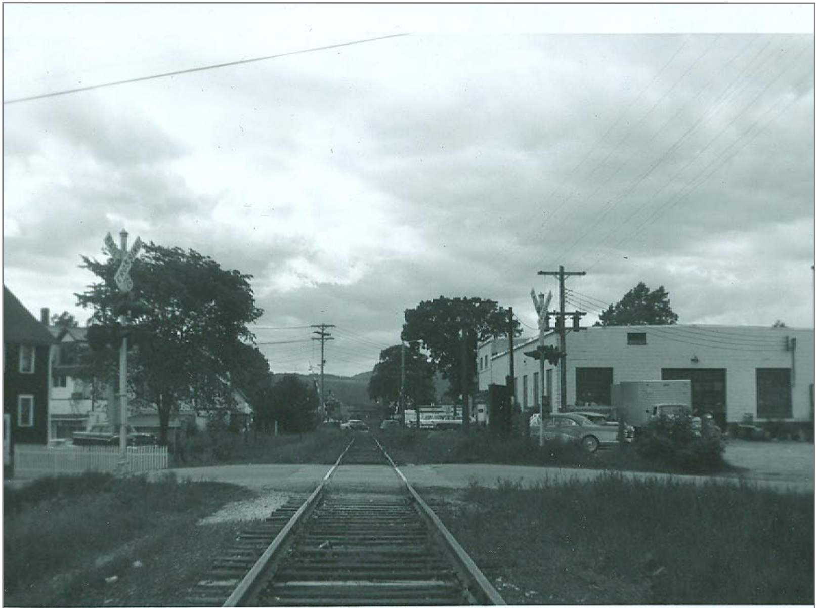
Northbound Crossing Allen Street
