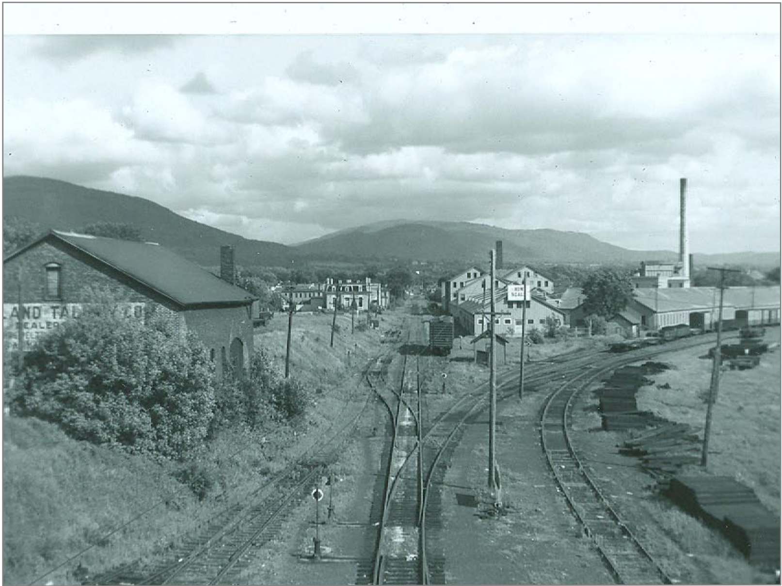
Southbound from Stong Ave. bridge
