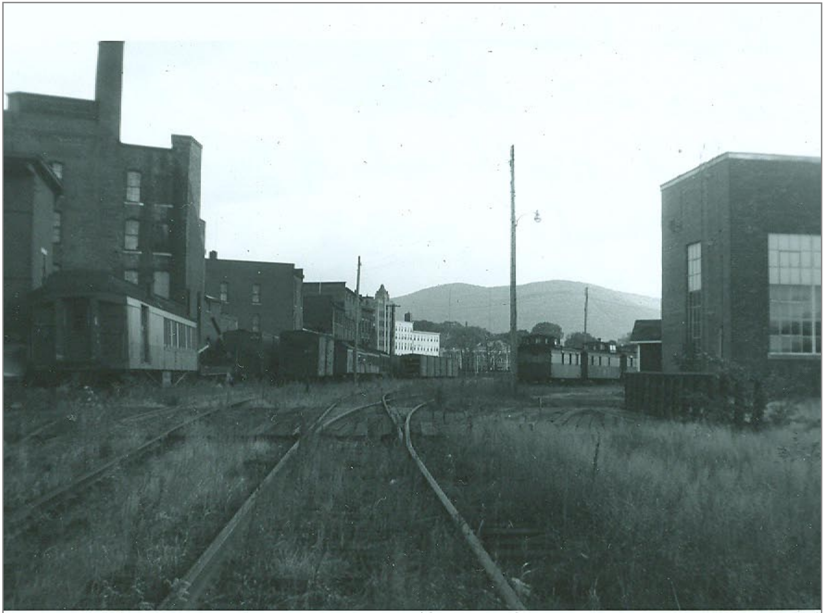
North end of Rutland Yard looking south
