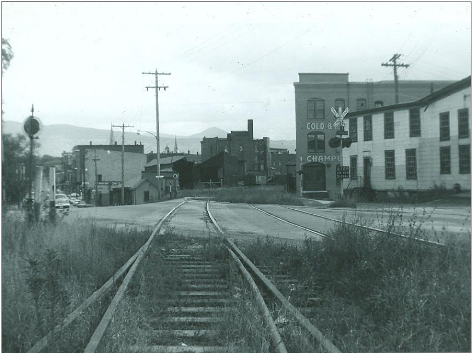
West Street Crossing looking Southbound
