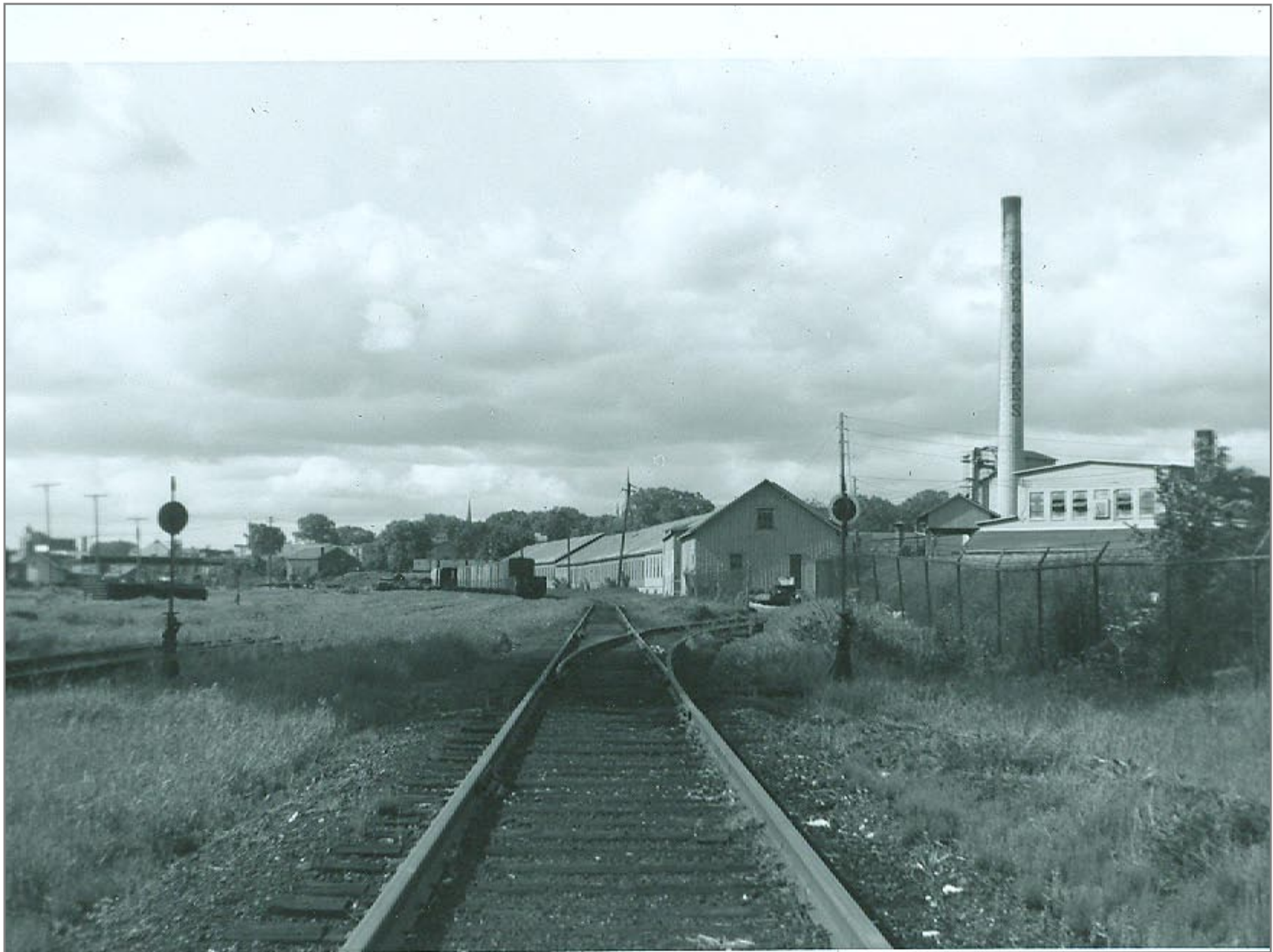
Northbound Switch into Howe Scale on right
