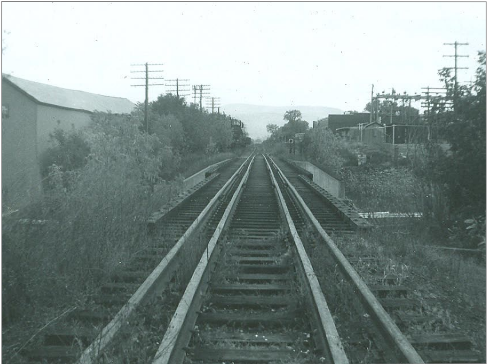
Northbound Bridge over Otter Creek
