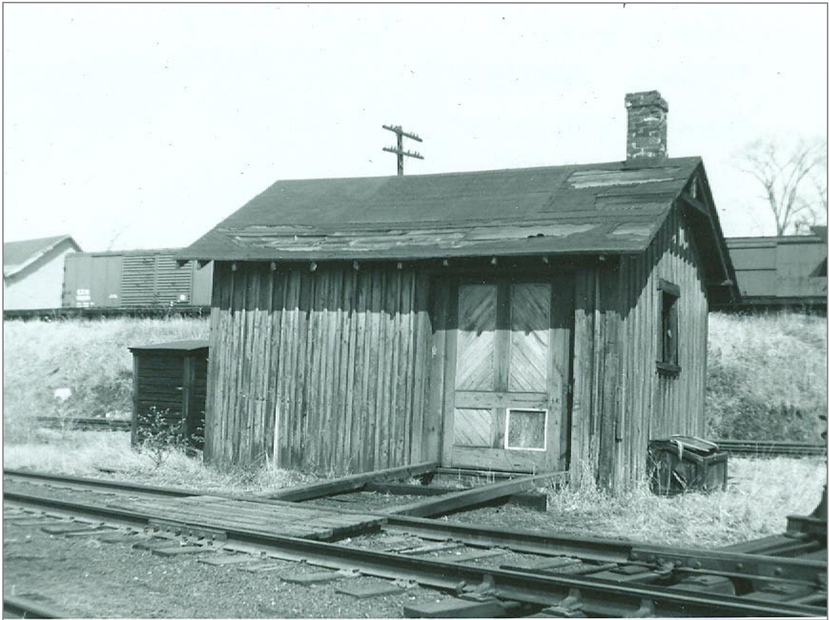
Tool House in Rutland yard
