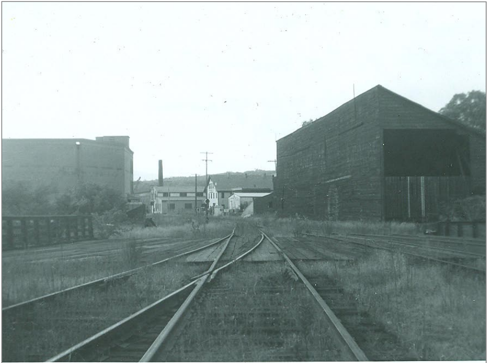
Northbound at North end of Rutland yard Bridge 210 in foreground
