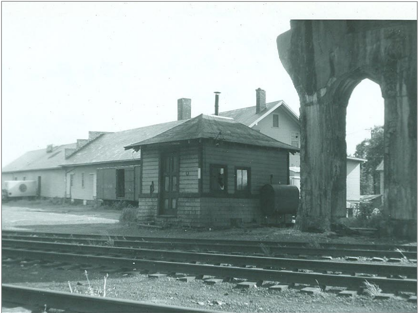
Yard office Rutland
