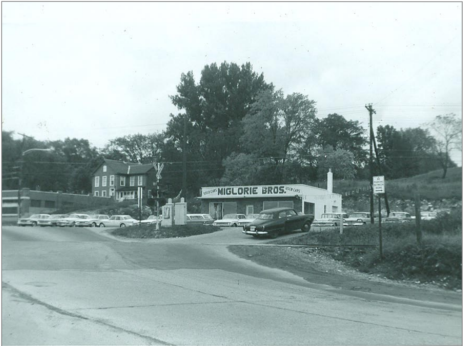
Route 4 Ahead Looking North
