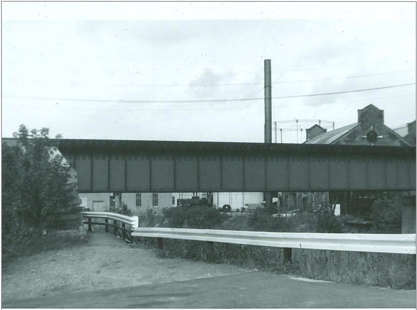
Rutland Bridge over Otter creek
