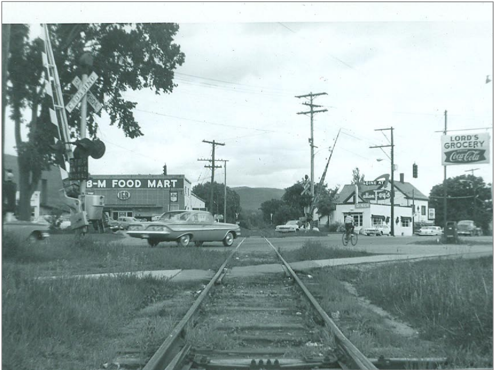
Southbound to Bellow's Falls across Route 7
