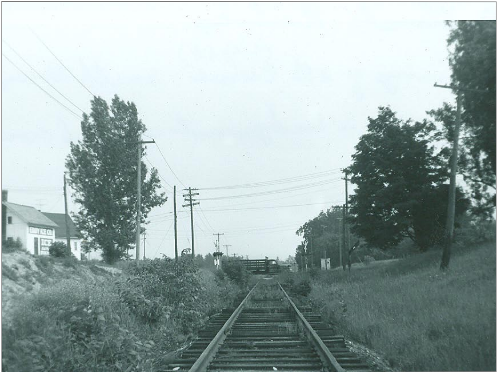
Southbound into No. Clarendon
