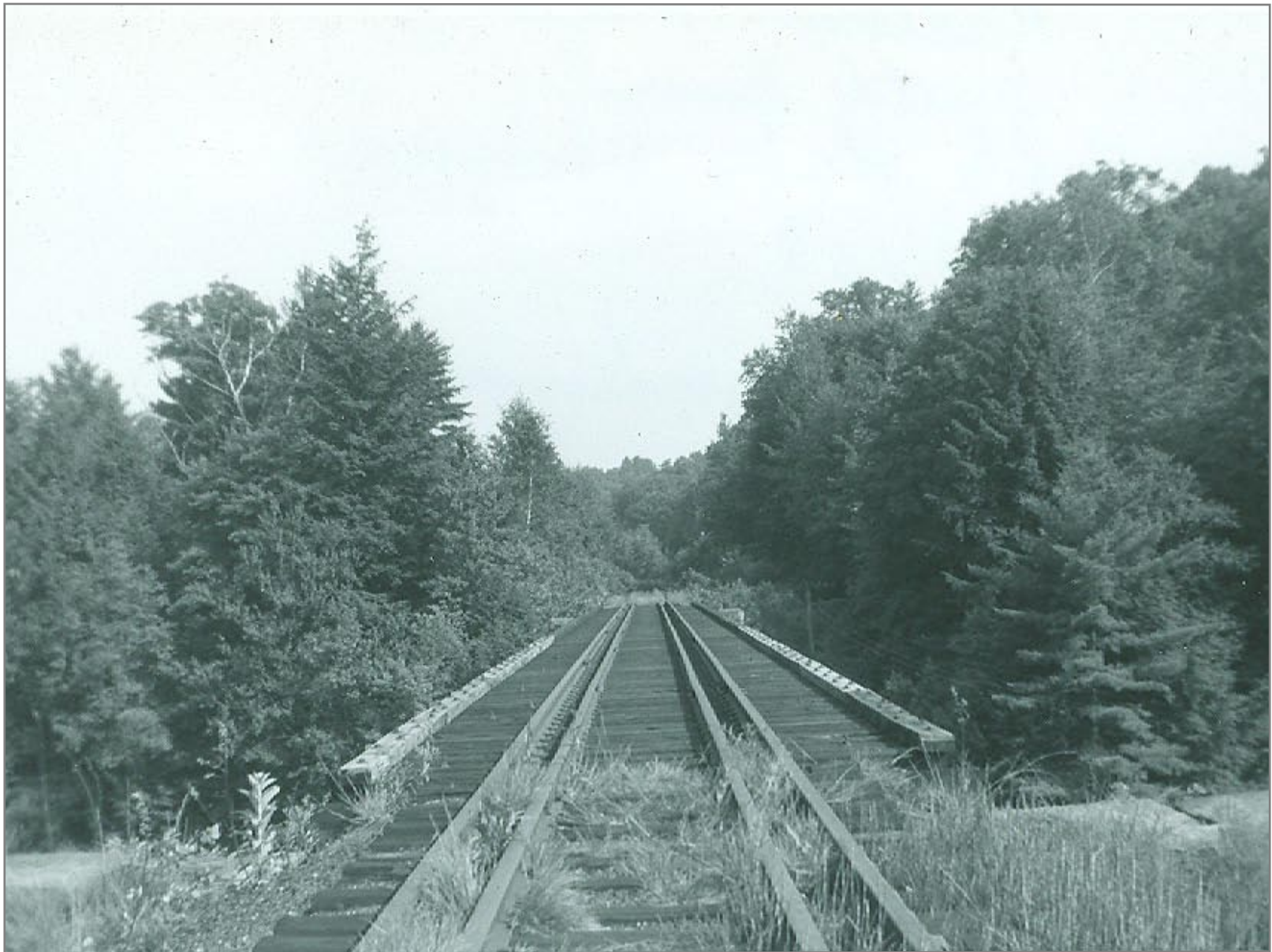
Southbound @ Rockingham Bridge 108
