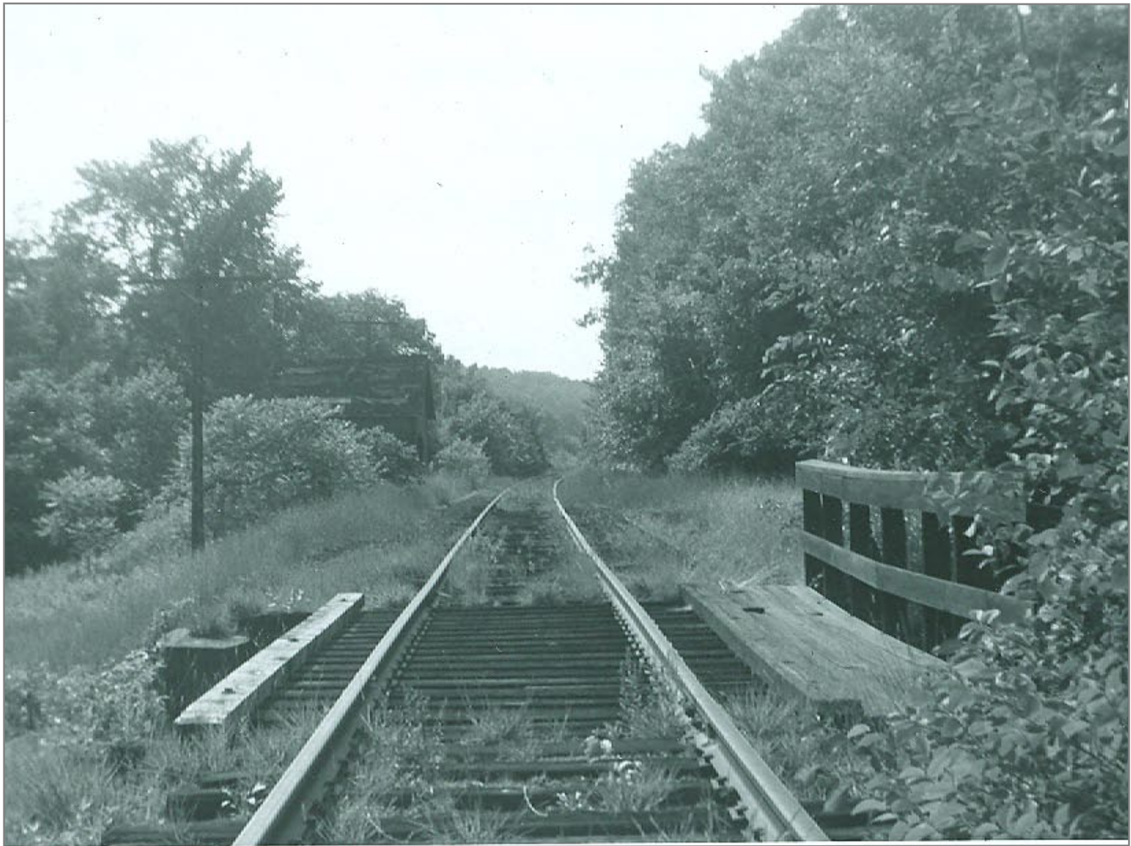
Northbound @ Rockingham Tool House on left
