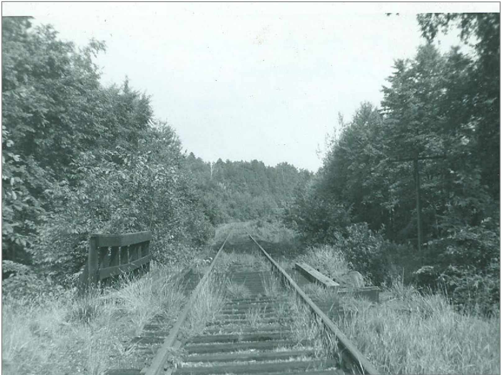
Bridge @ Rockingham Southbound
