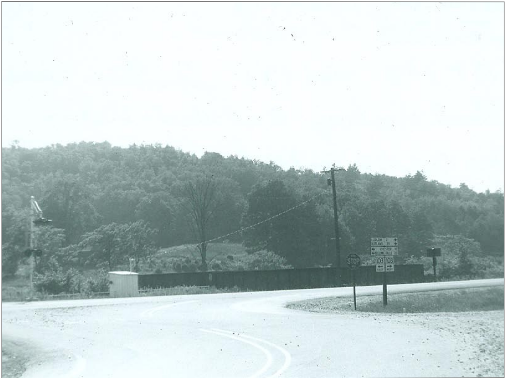
Bridge 132 in background
