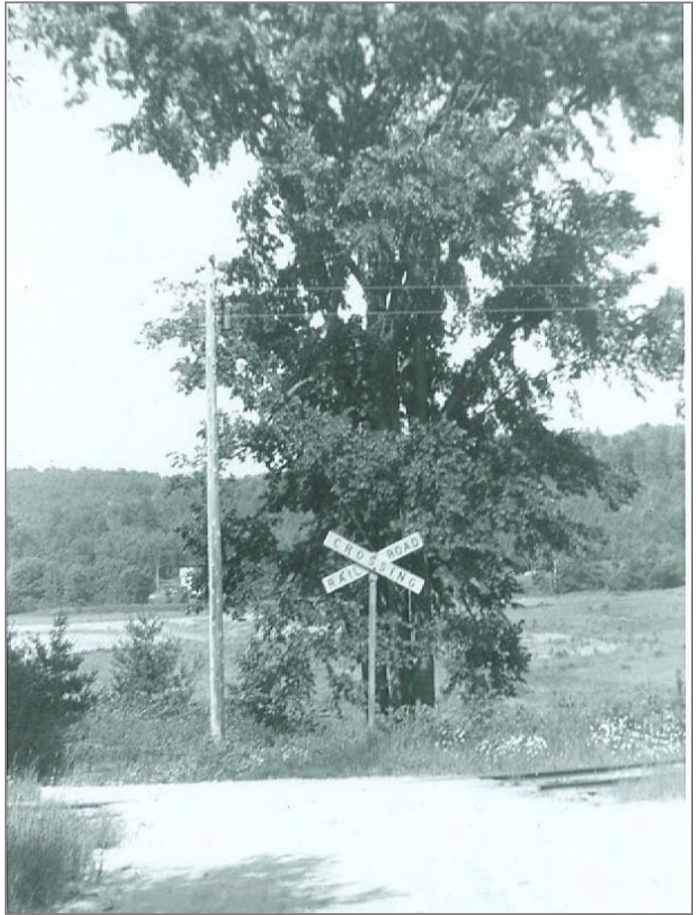
West View of East Hill Road crossing
