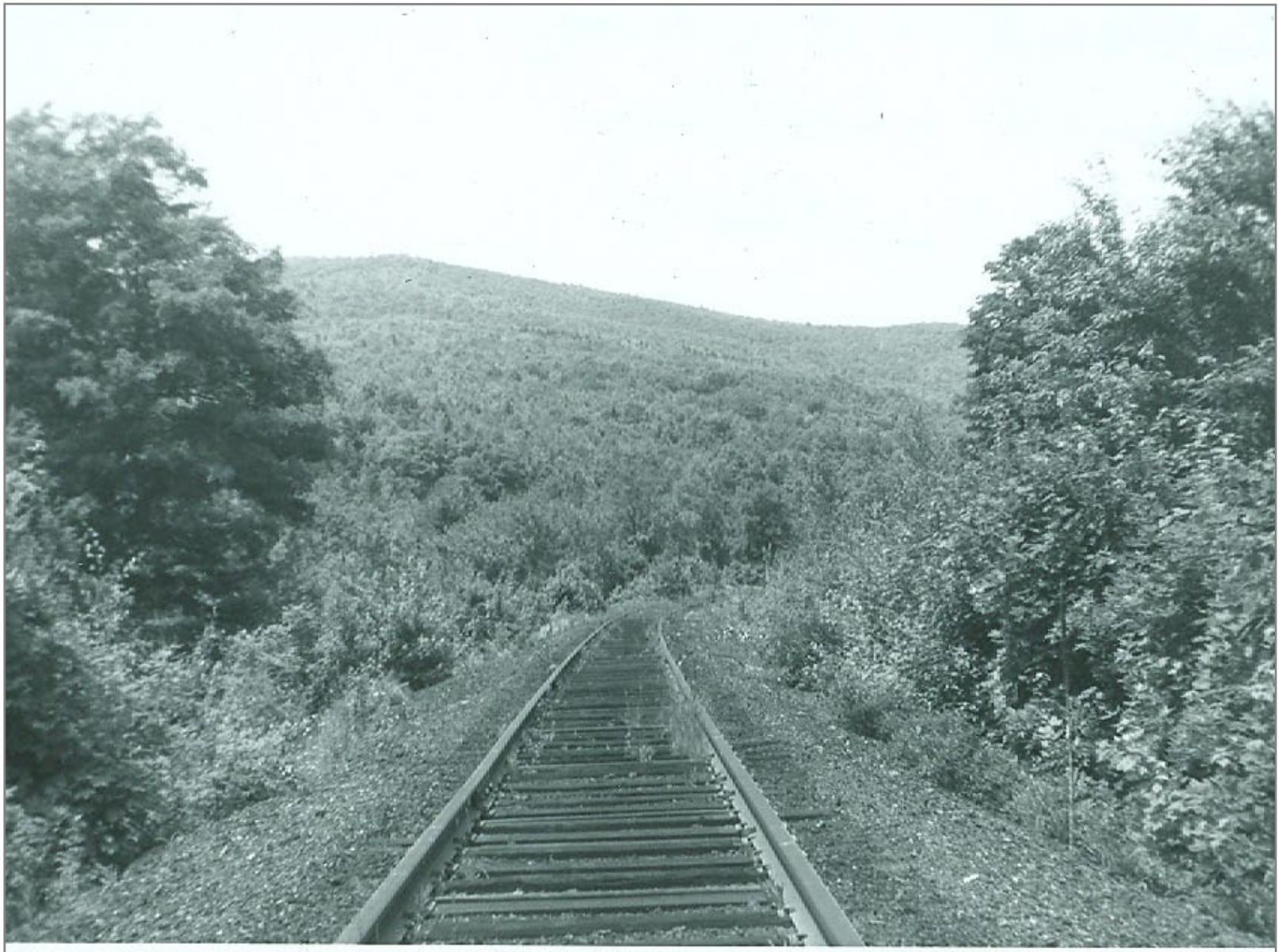
Southbound just south of Ludlow
