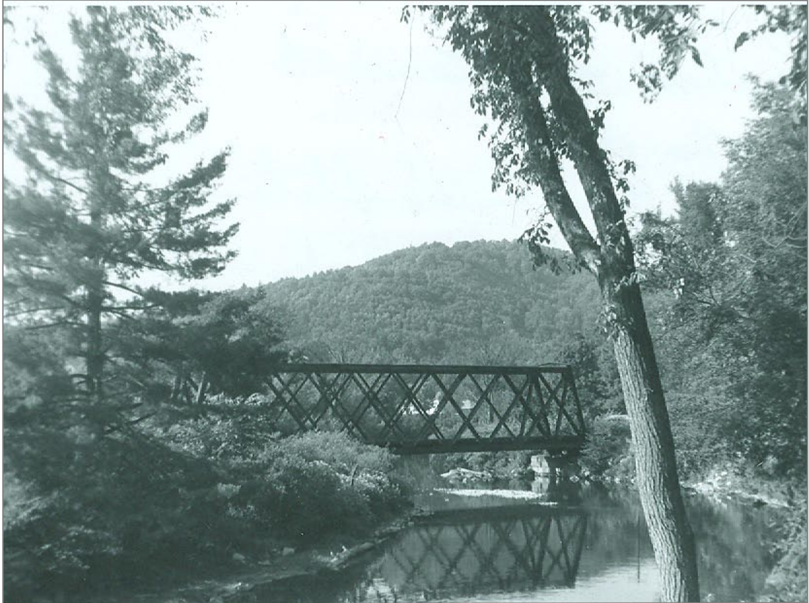
Bridge 130 south of Proctorsville Station
