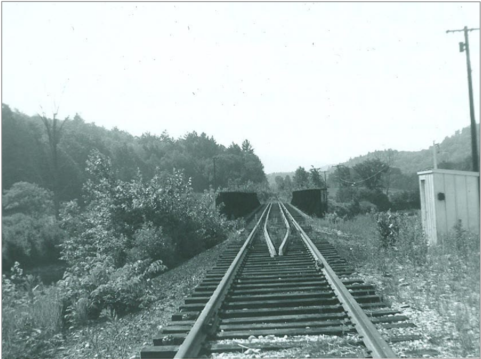
Northbound @ Bridge 132 - Shed for flashing signals at crossing on right
