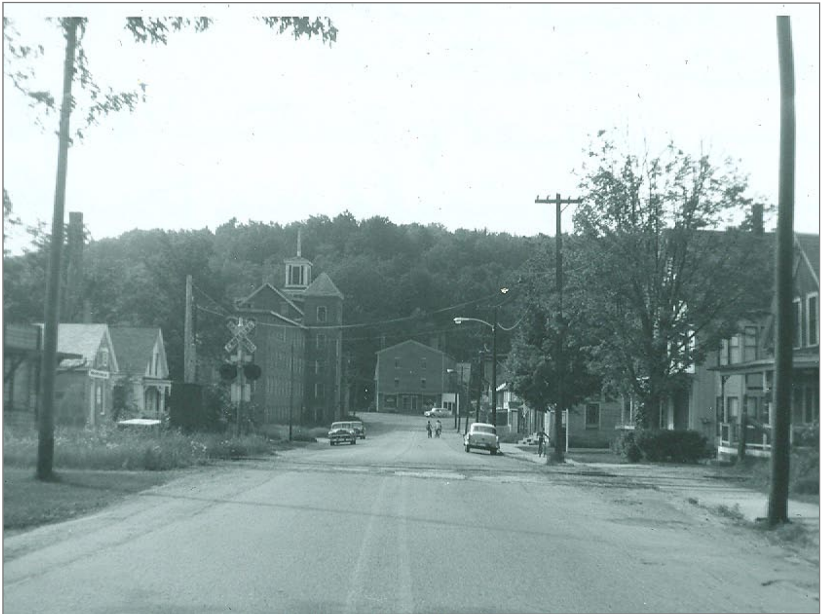
Proctorsville looking west - edge of station on left being demo'd
