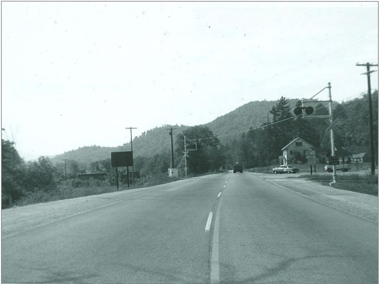
North on 103 - Bridge 132 on left
