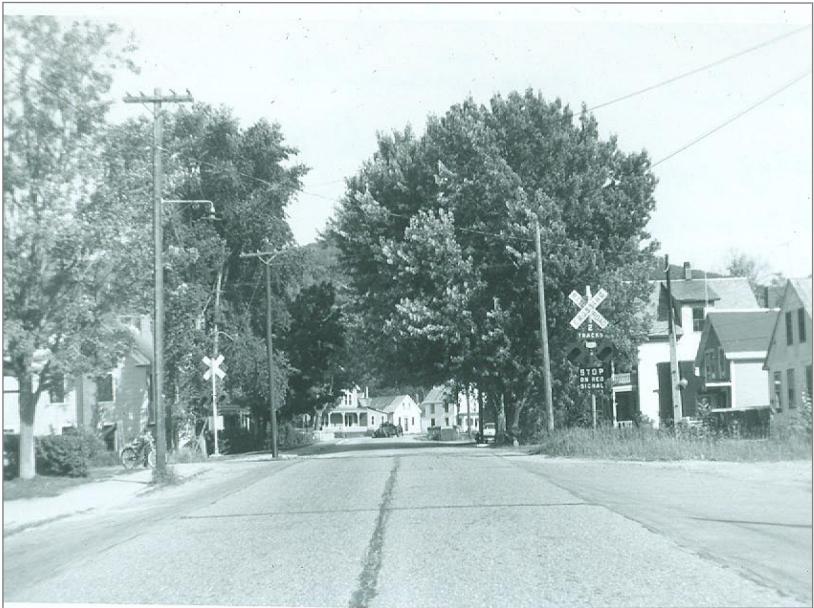
Looking East at Crossing just south of Proctorsville Station
