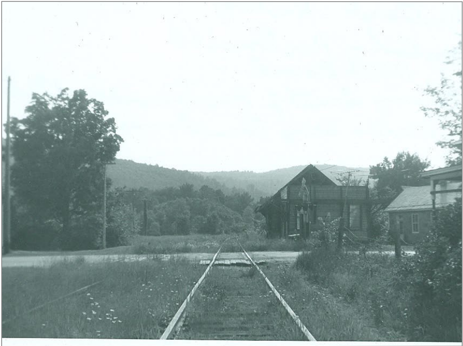
Proctorsville Station being demolished on right looking North
