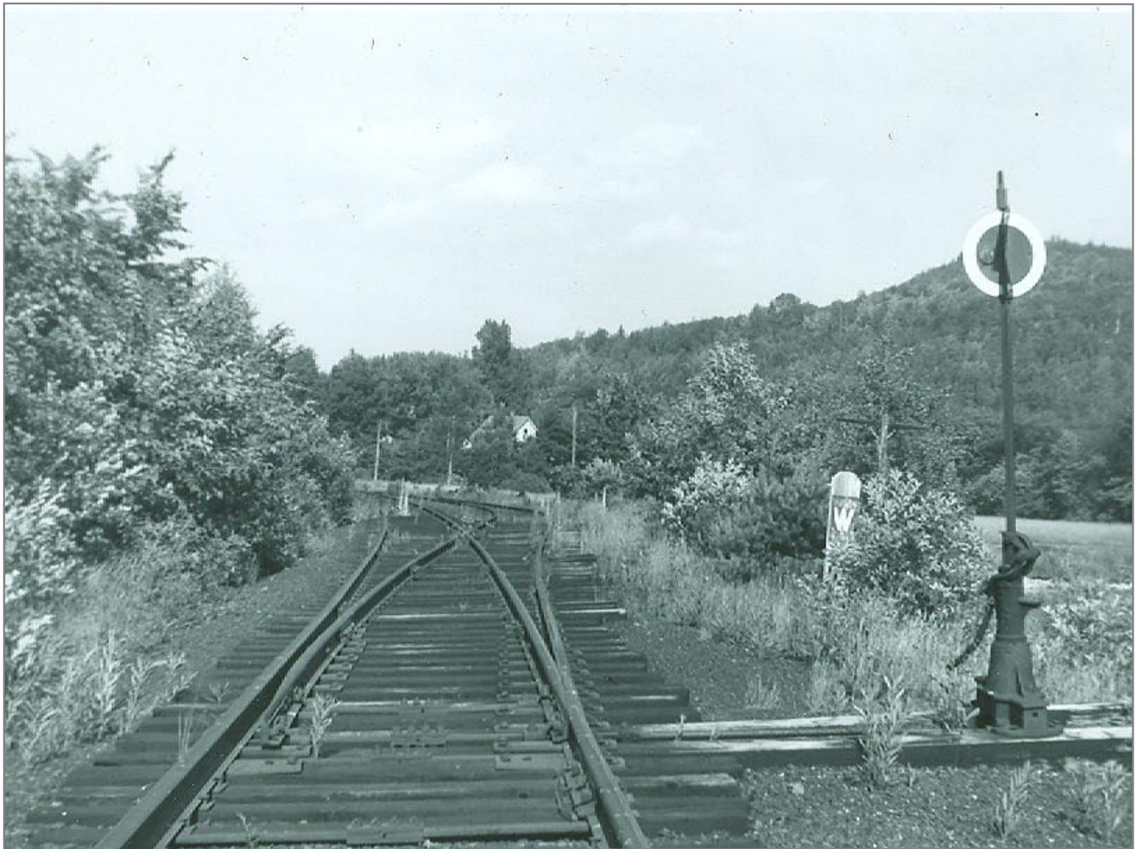
Southbound @ Siding Switch just north of Station
