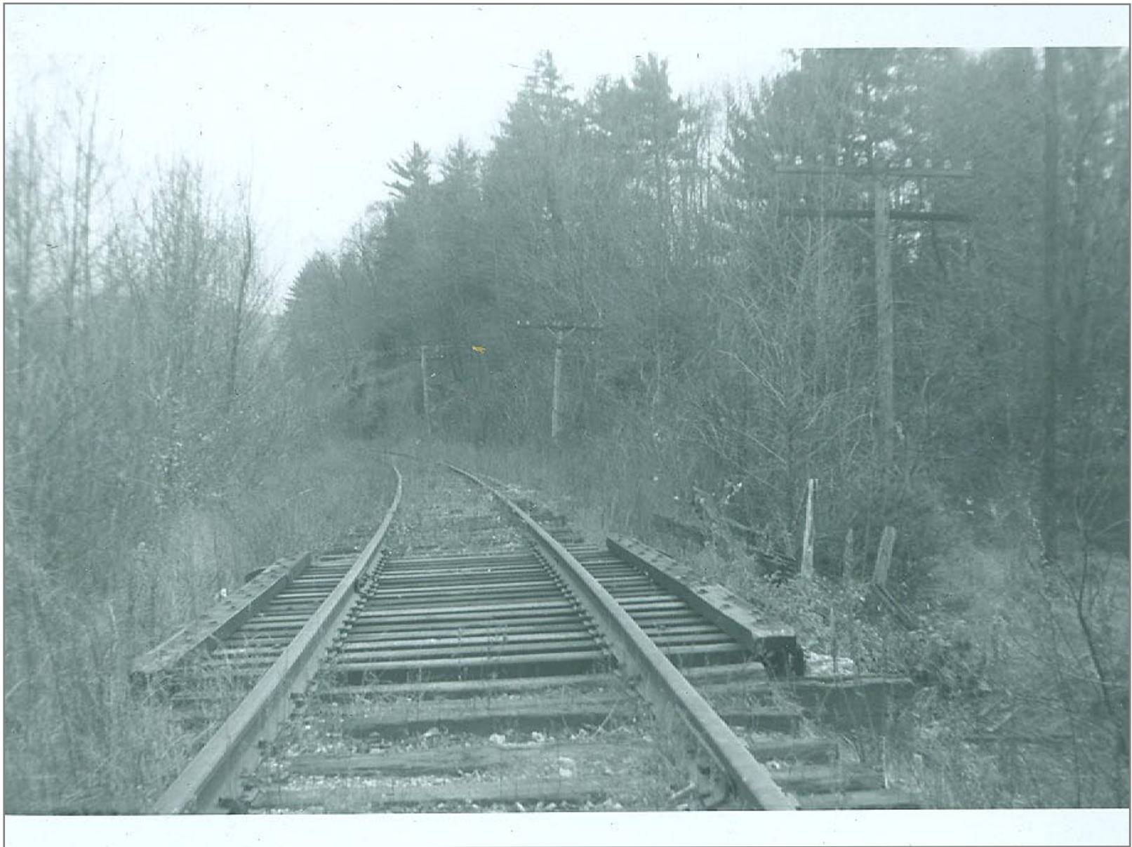
Timber bridge north of Proctor Southbound?
