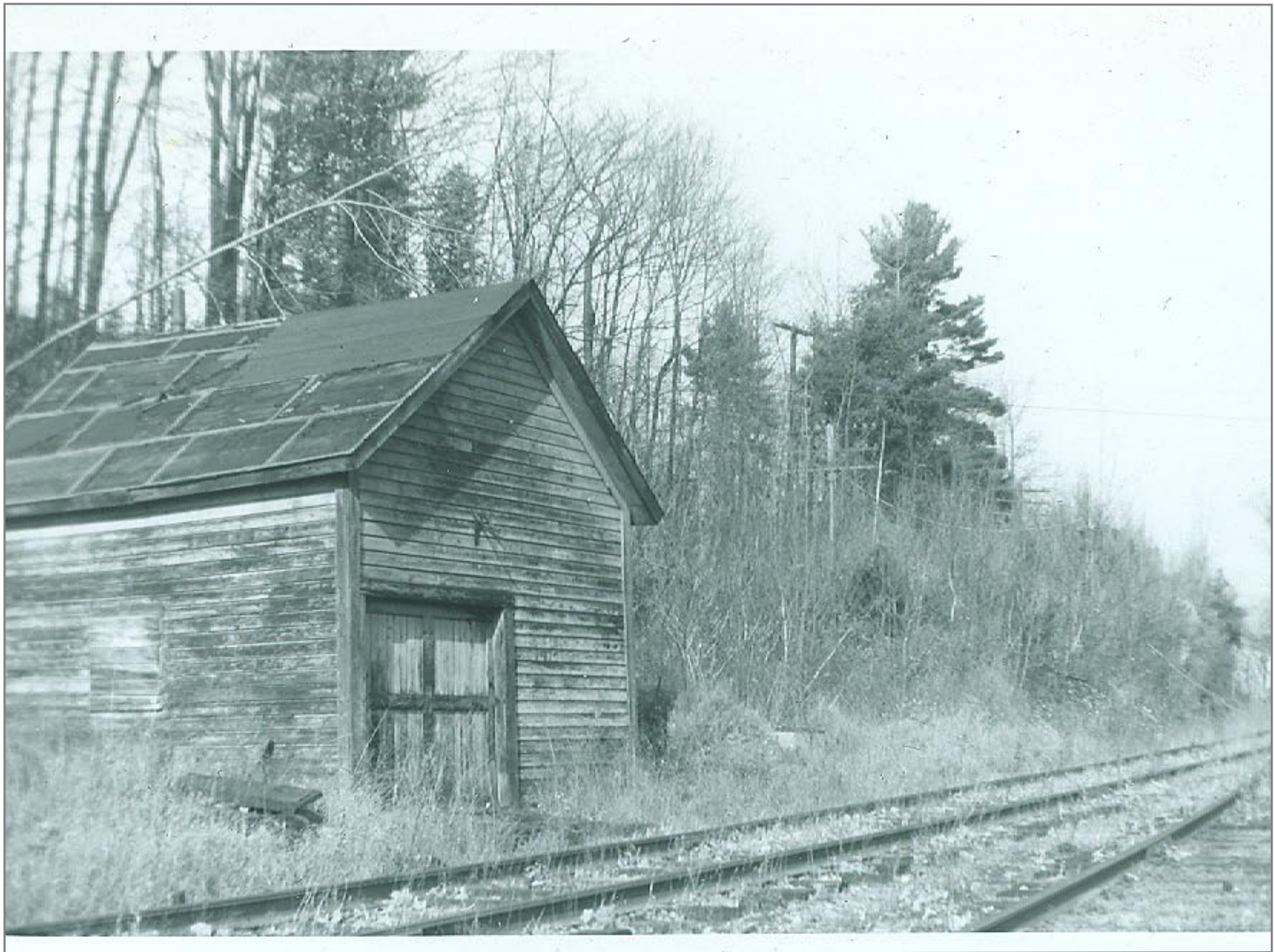
Section House on left at proctor Long Siding Northbound
