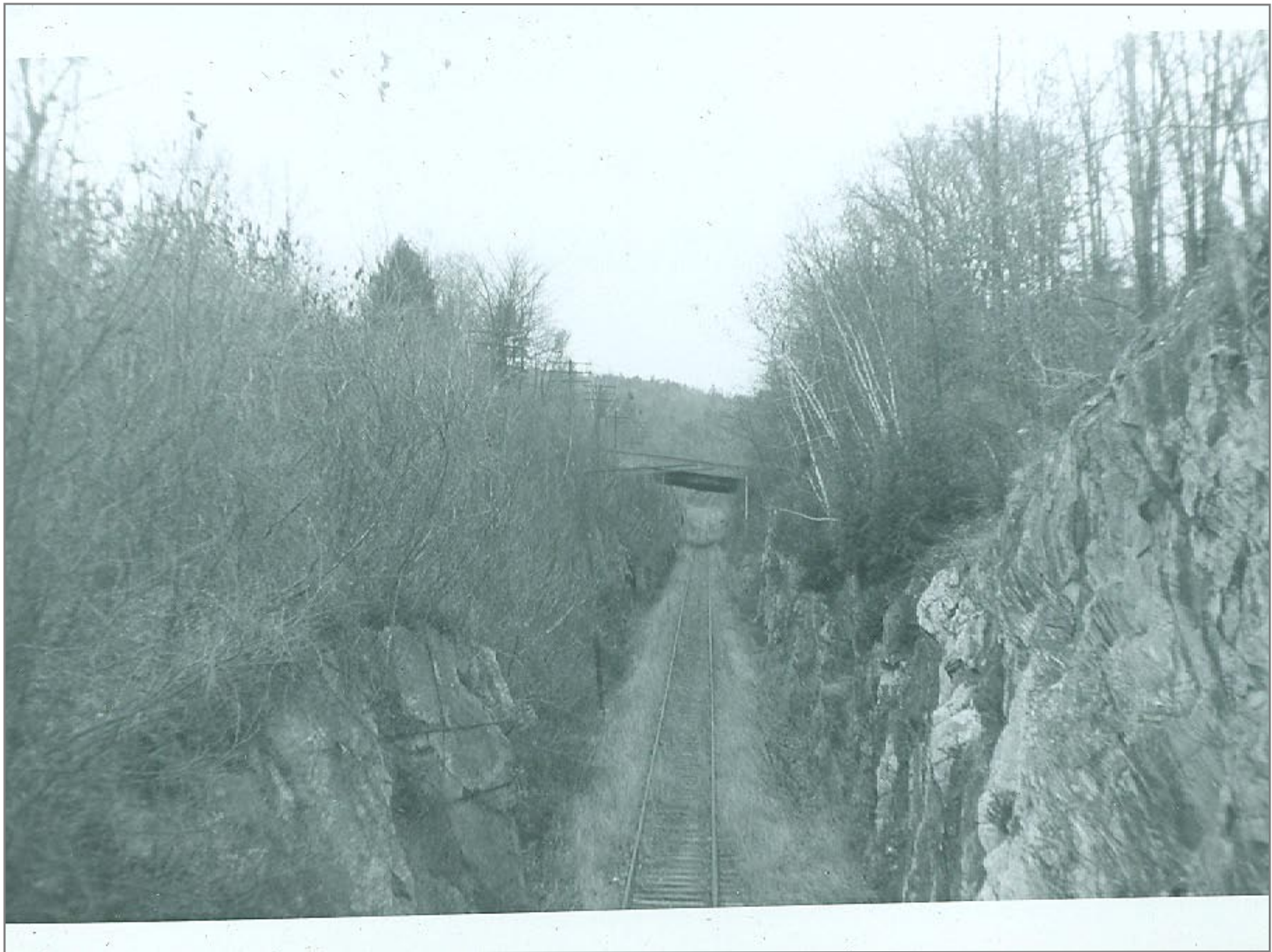
Northbound off C&P Bridge
