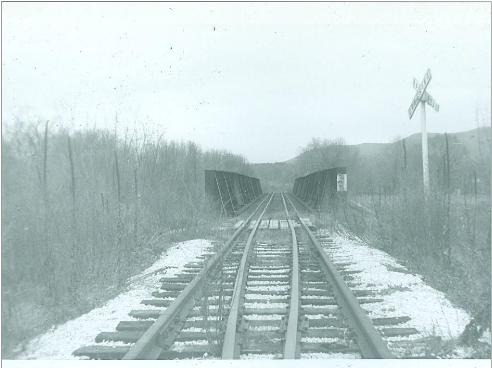
Southbound Near Pittsford Bridge 215
