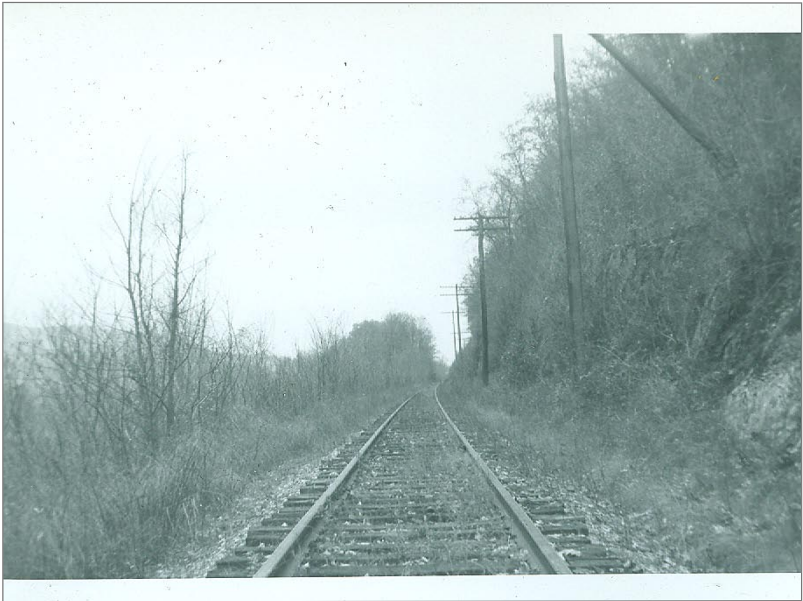
Southbound into Proctor
