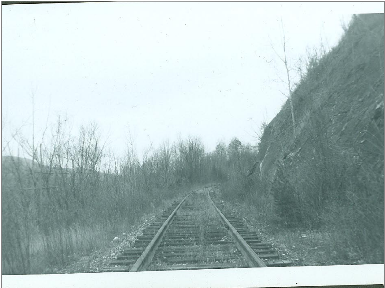
Southbound into Proctor
