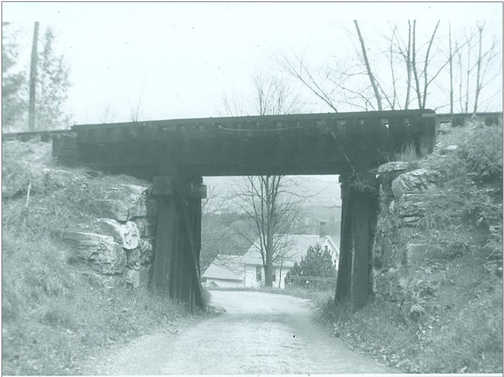
Timber Bridge North of Proctor
