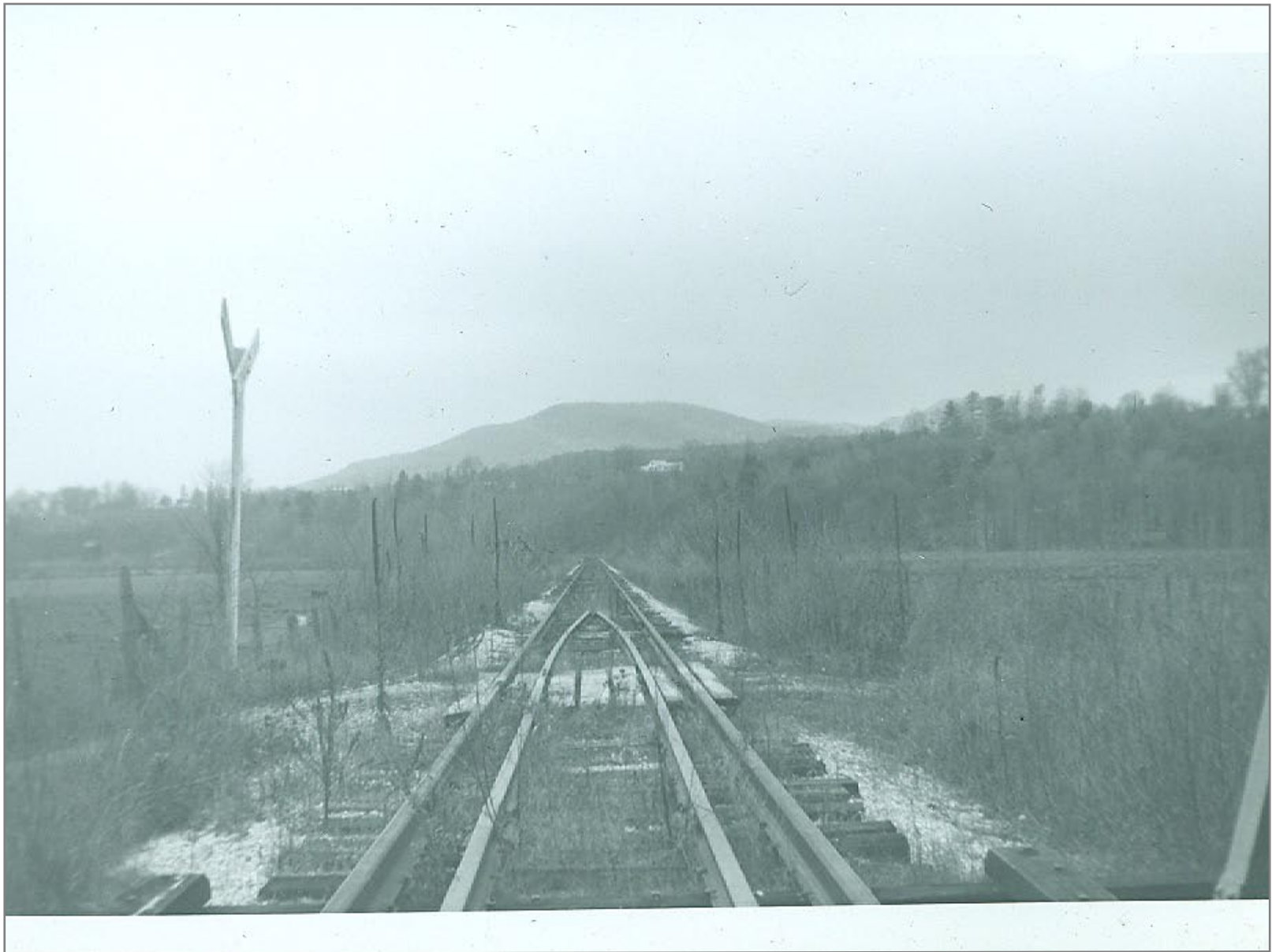
Farm Crossing Northbound into Pittsford
