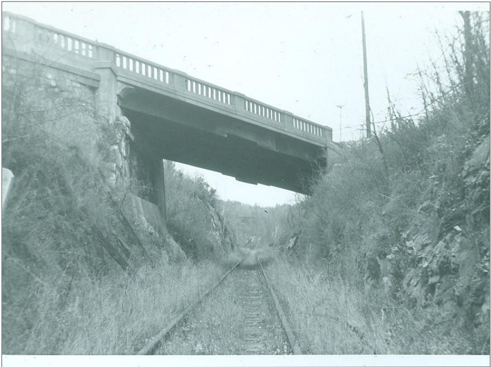
Northbound under North Street Bridge Proctor
