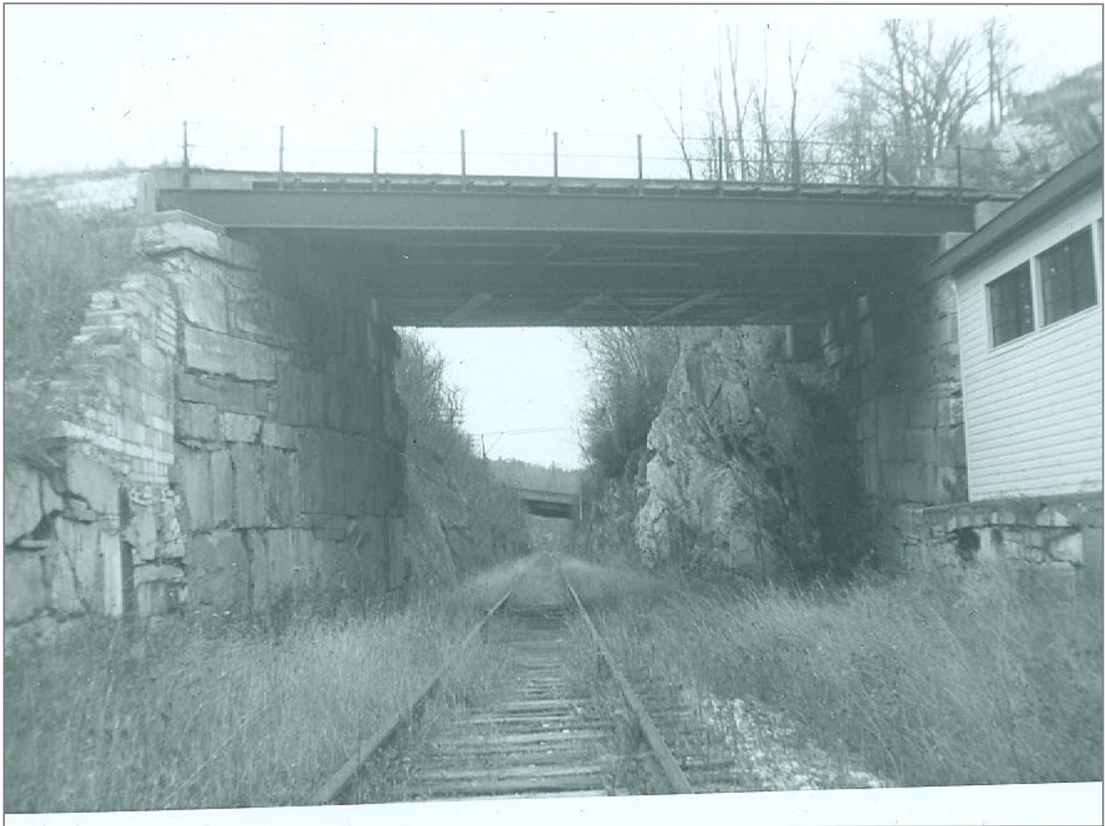
Northbound at C&P bridge in Proctor
