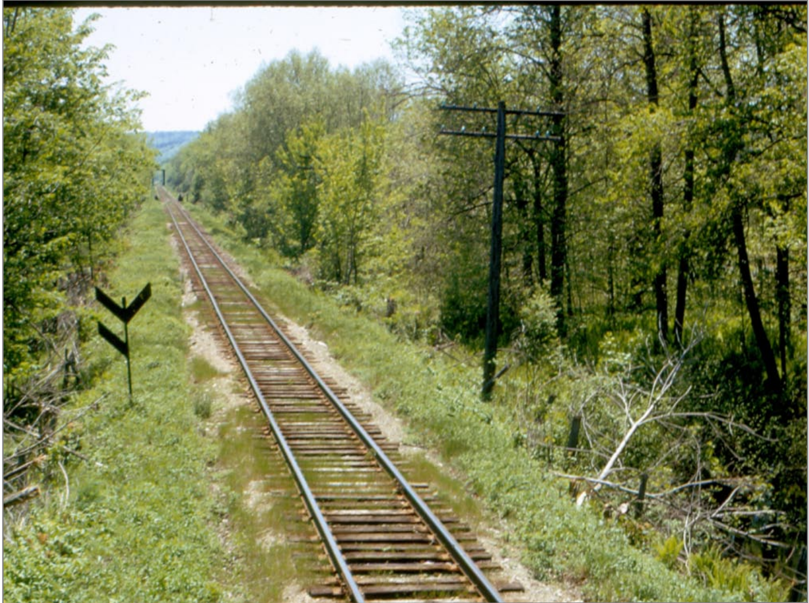
Looking South at beginning of Proctor Long Siding
