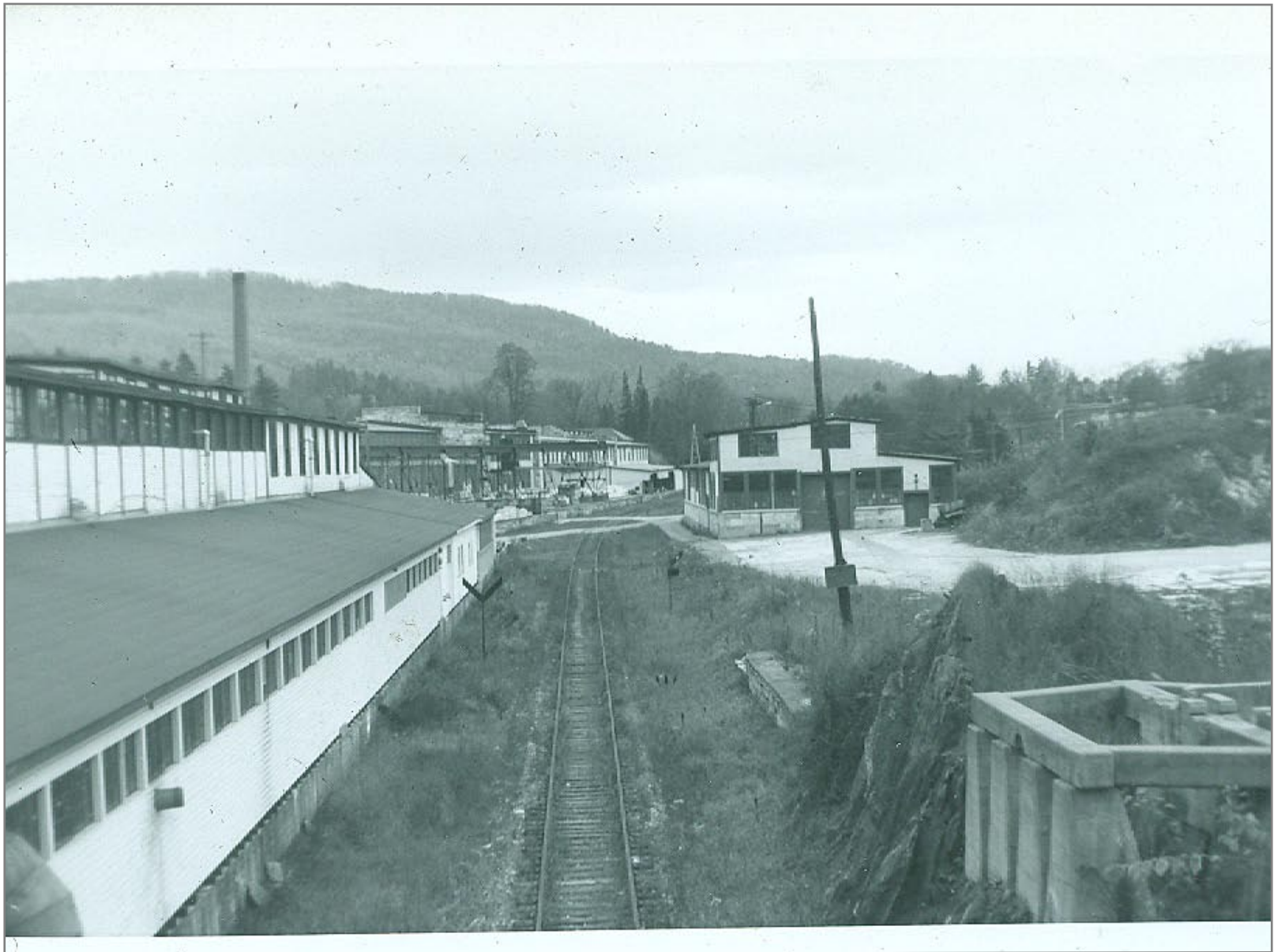
Southbound at C&P bridge, Rutland Water tank foundation on right
