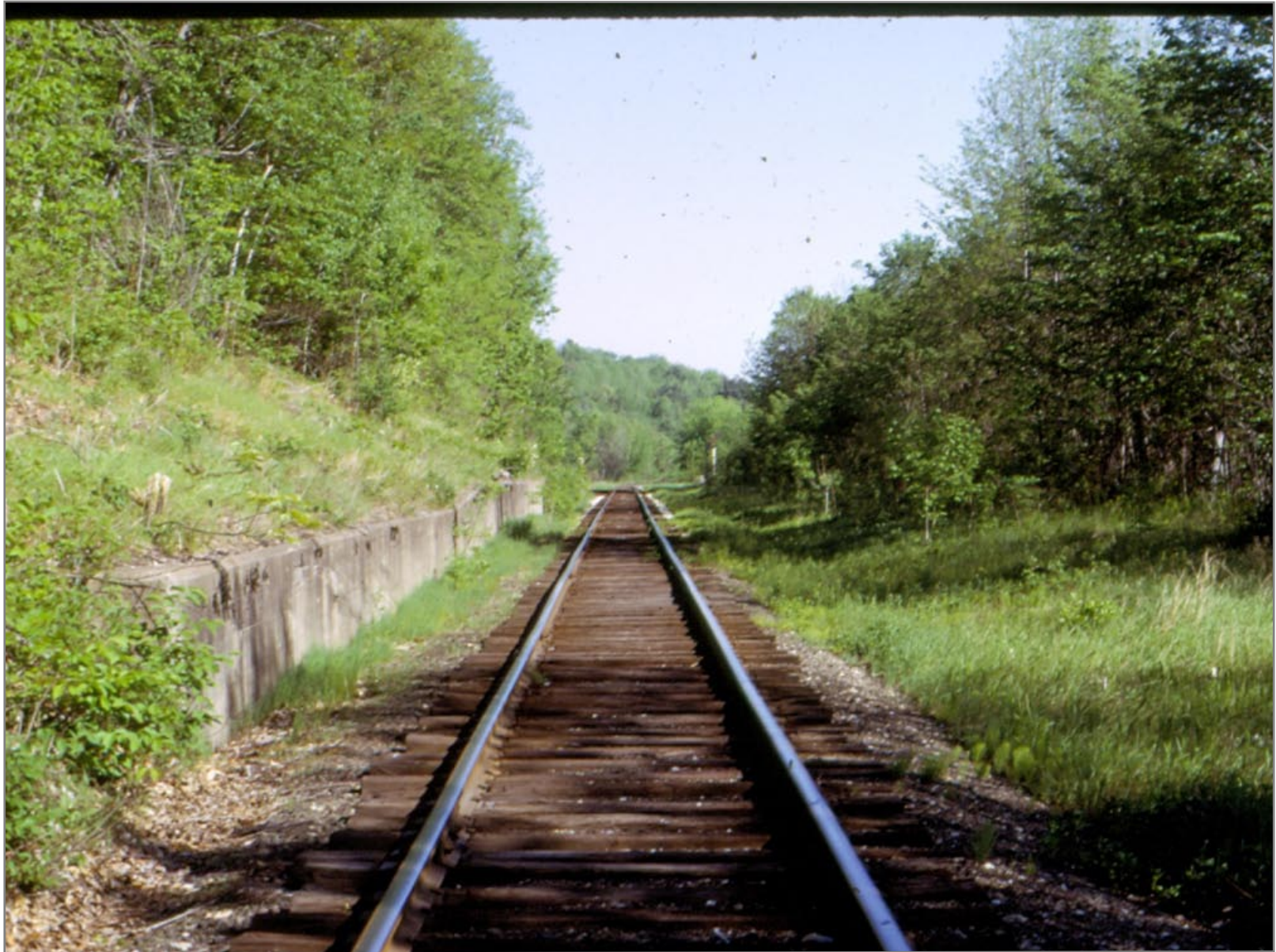
Southbound into Proctor
