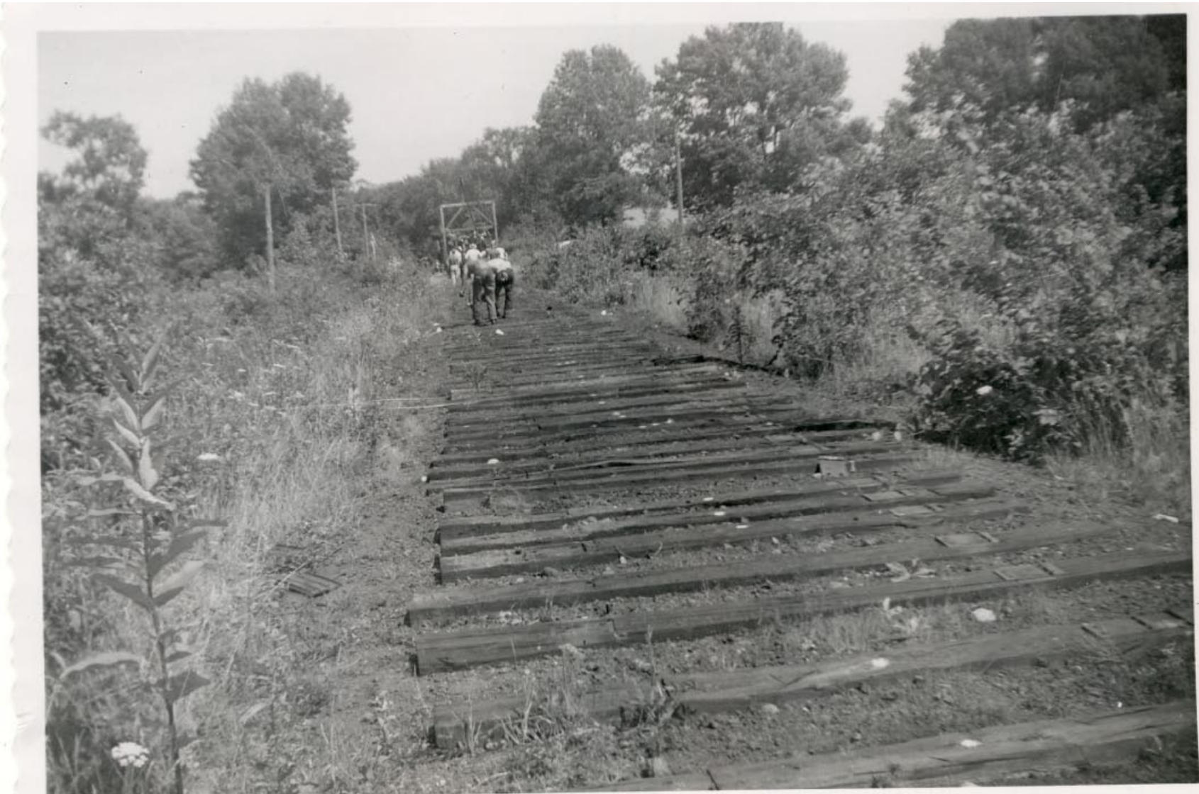
Wrecking Crew on Chatham
