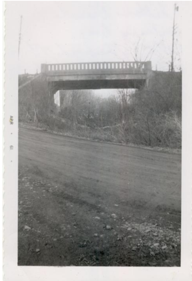
Highway Bridge over Rutland RR looking North from Petersburg Station site 4/2/1961
