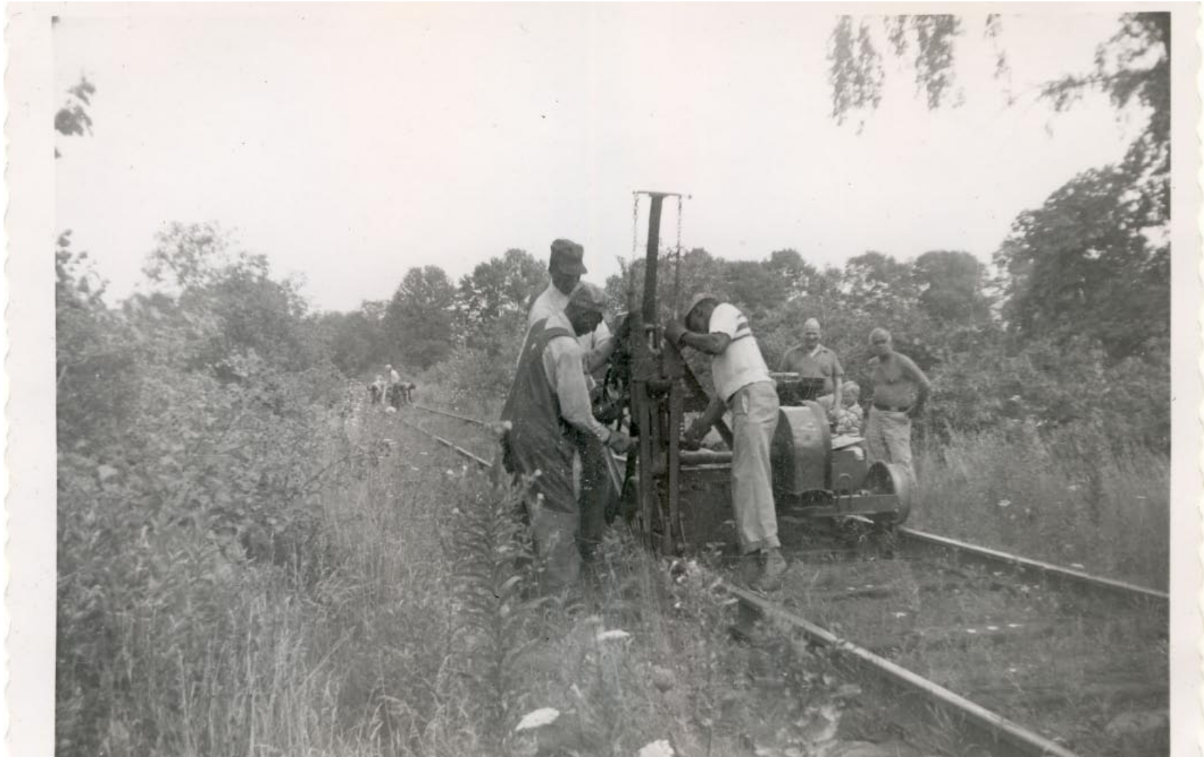
Wrecking Crew on Chatham Branch
