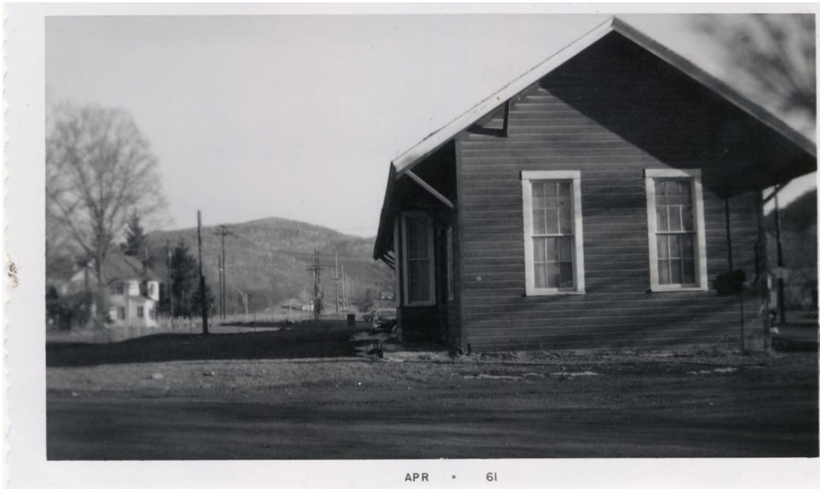
Berlin looking Southbound 4/1961
