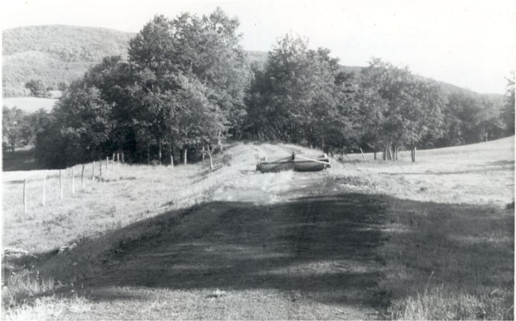
Rutland ROW Between VT/NY State Line and Route 7 1964
