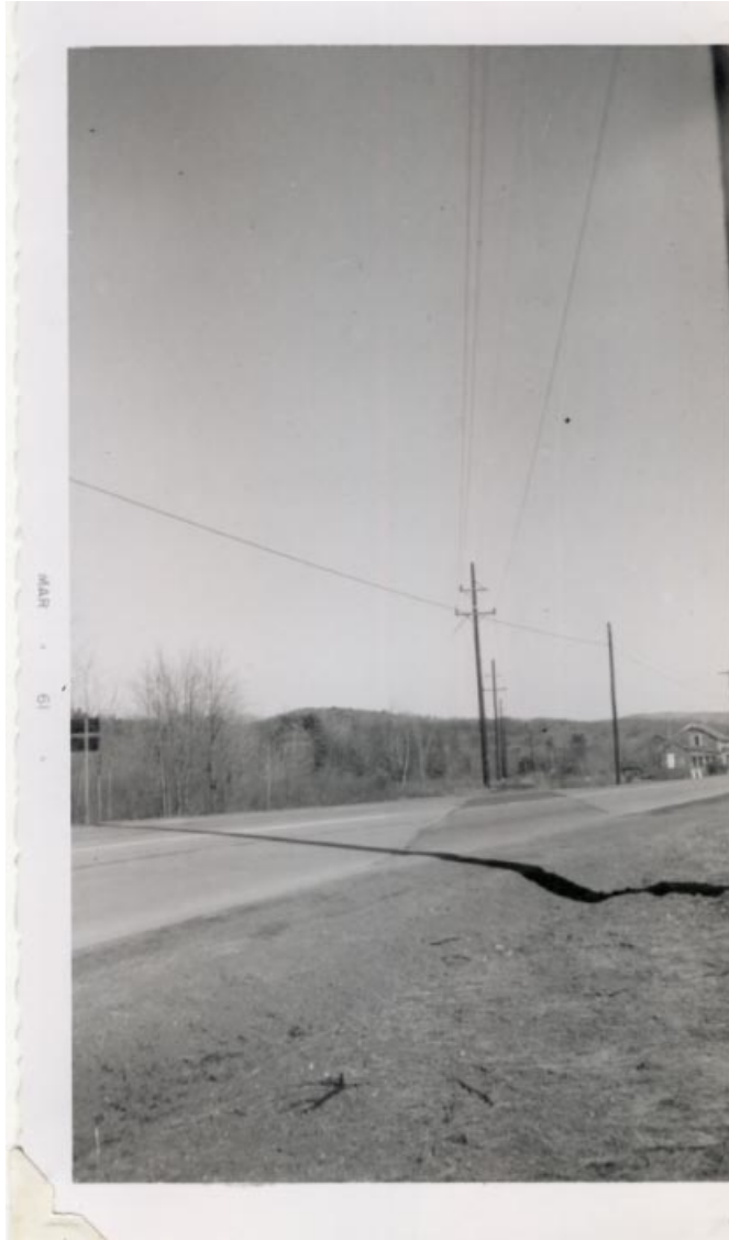
ROW crossing Route 20 Between Brainard & West Lebanon 3/26/1961
