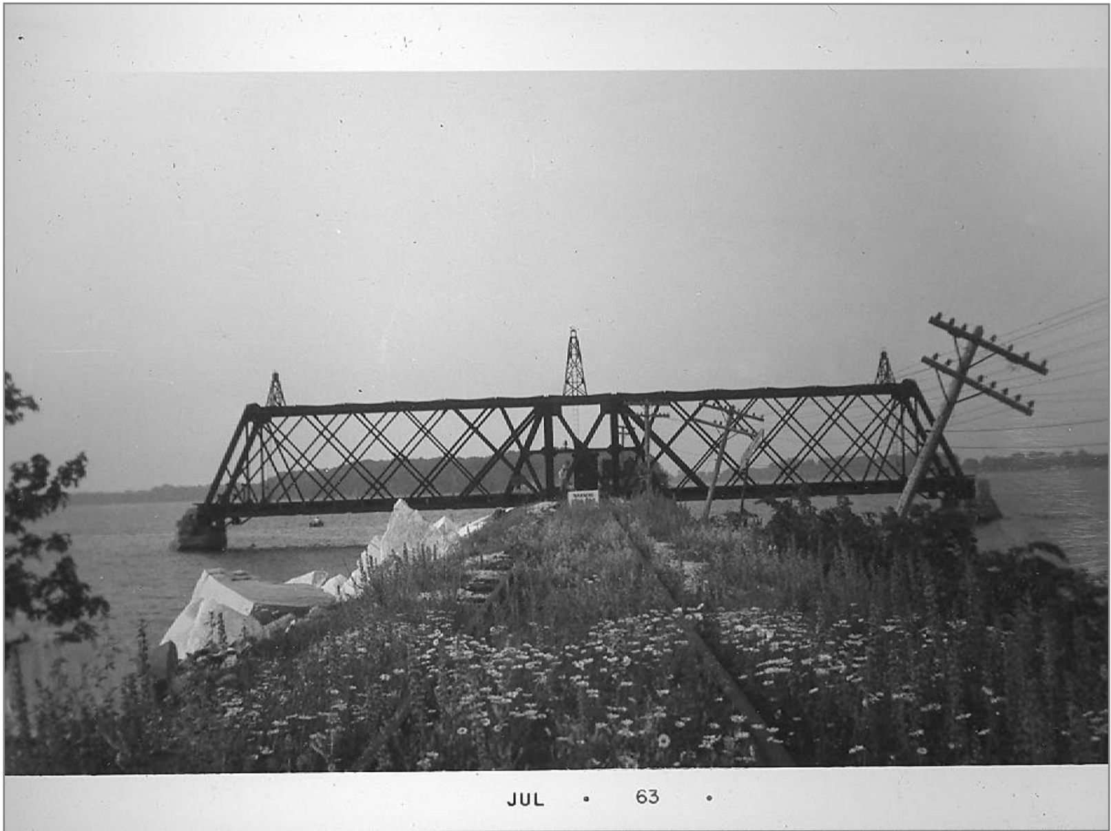
Pelot Point Northbound 6/29/63
