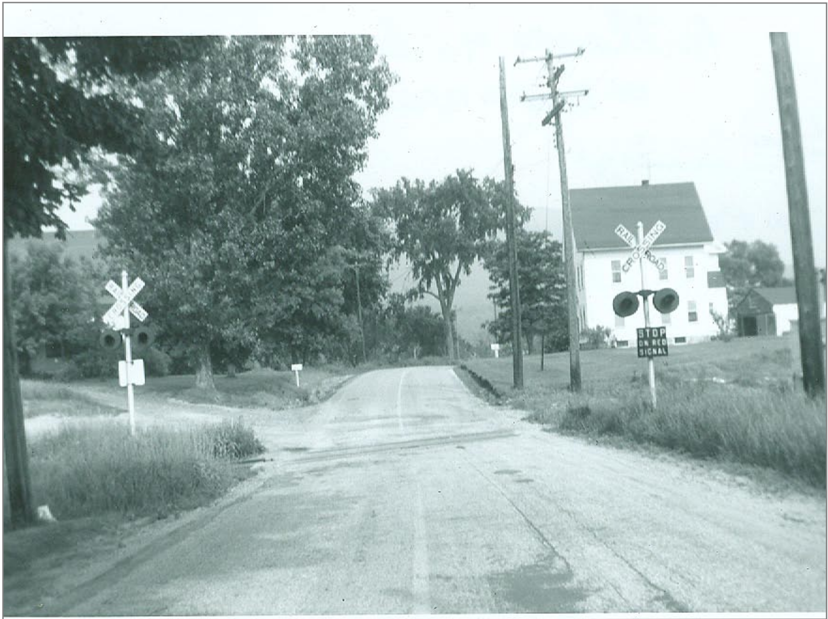
2nd crossing north of No. Clarendon - MP 51 on right
