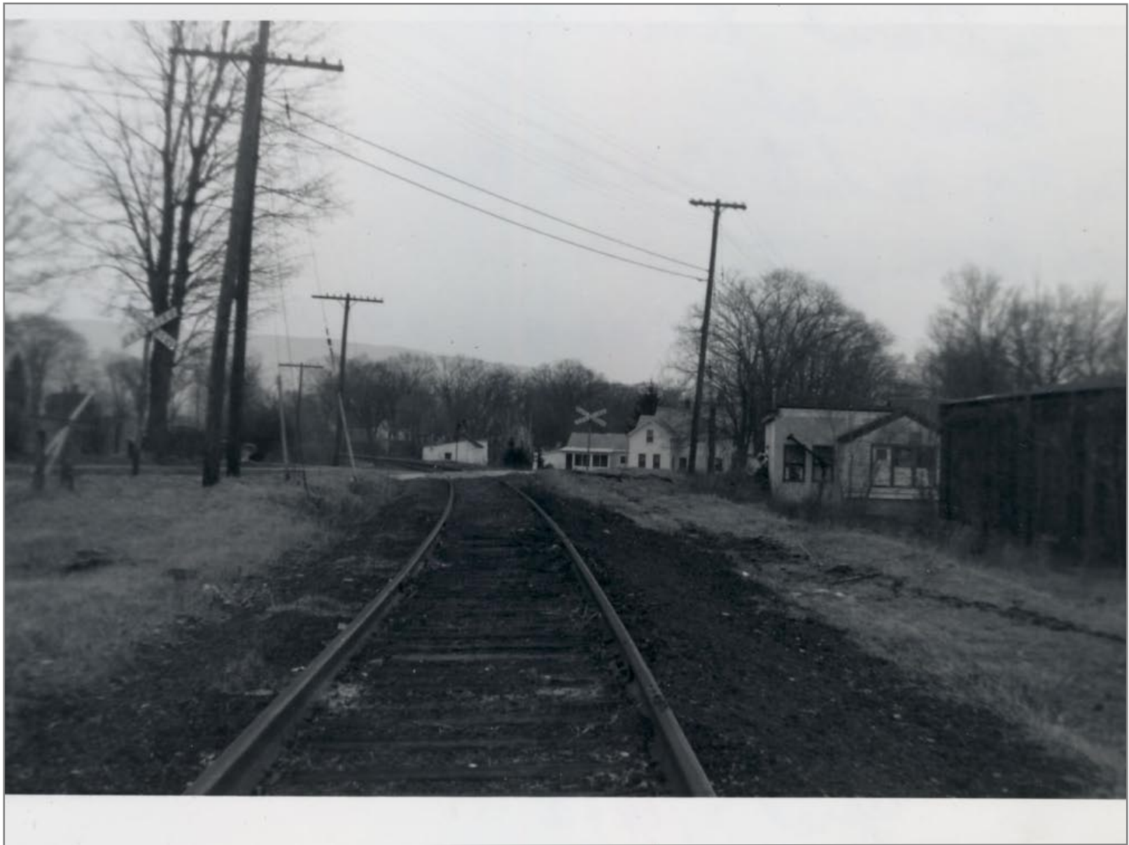
West of White Creek Road looking East Toward No. Bennington Old Trolley Barn on Right 4/8/1962
