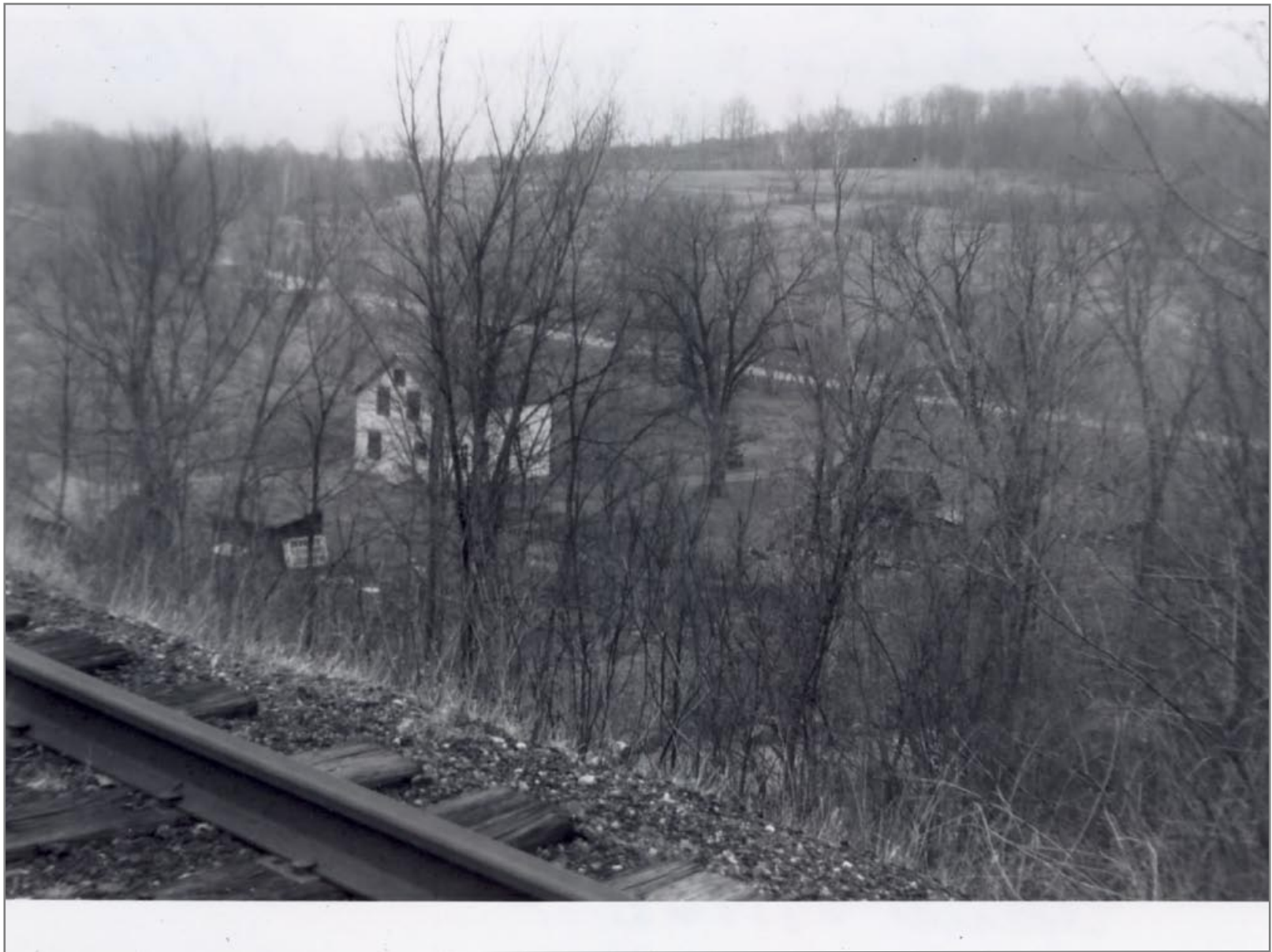
Looking South From Fill Toward Route 67 4/8/1962
