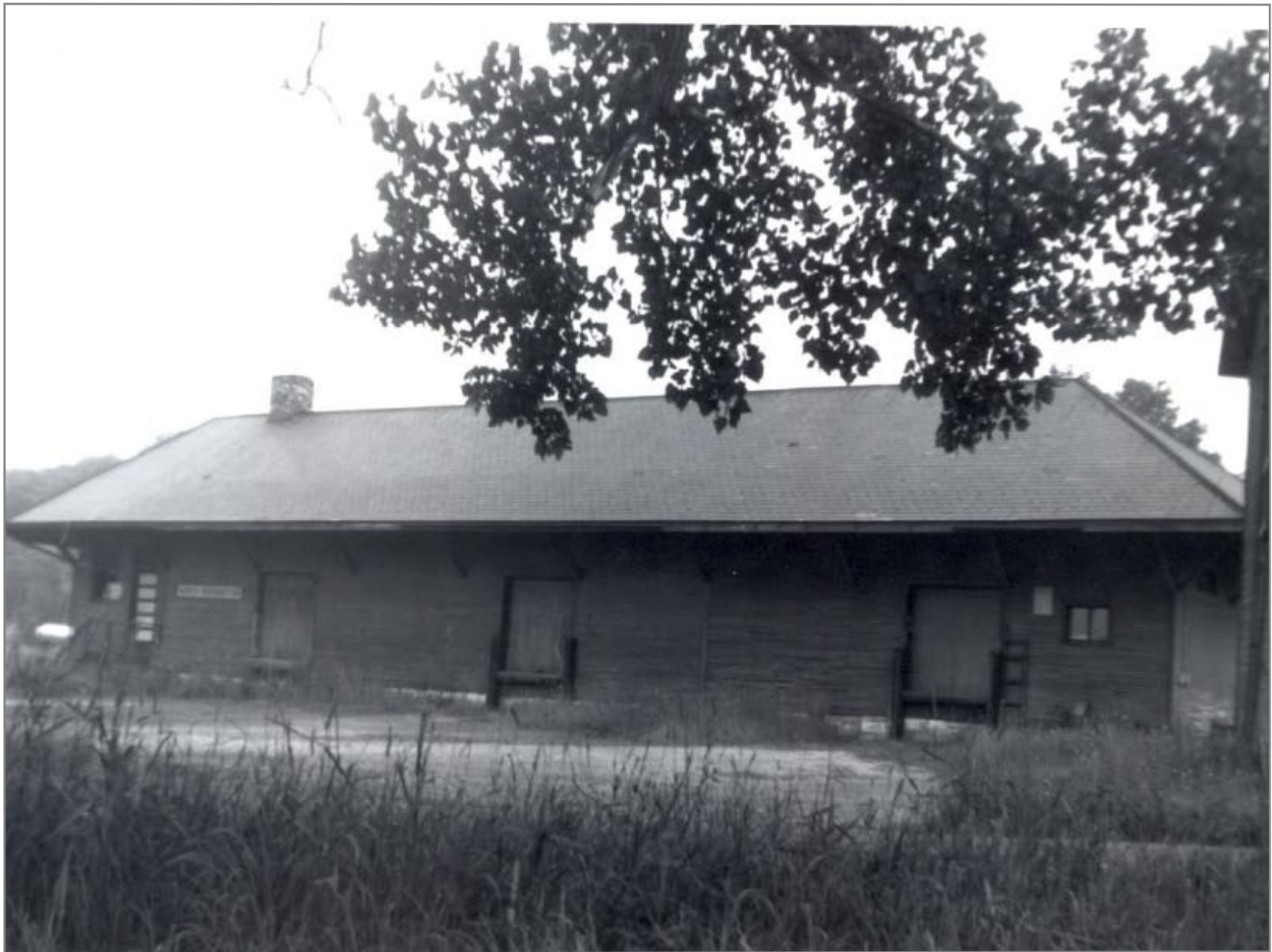
North bennington Freight House with Ice House in Right Foreground 7/1/1962
