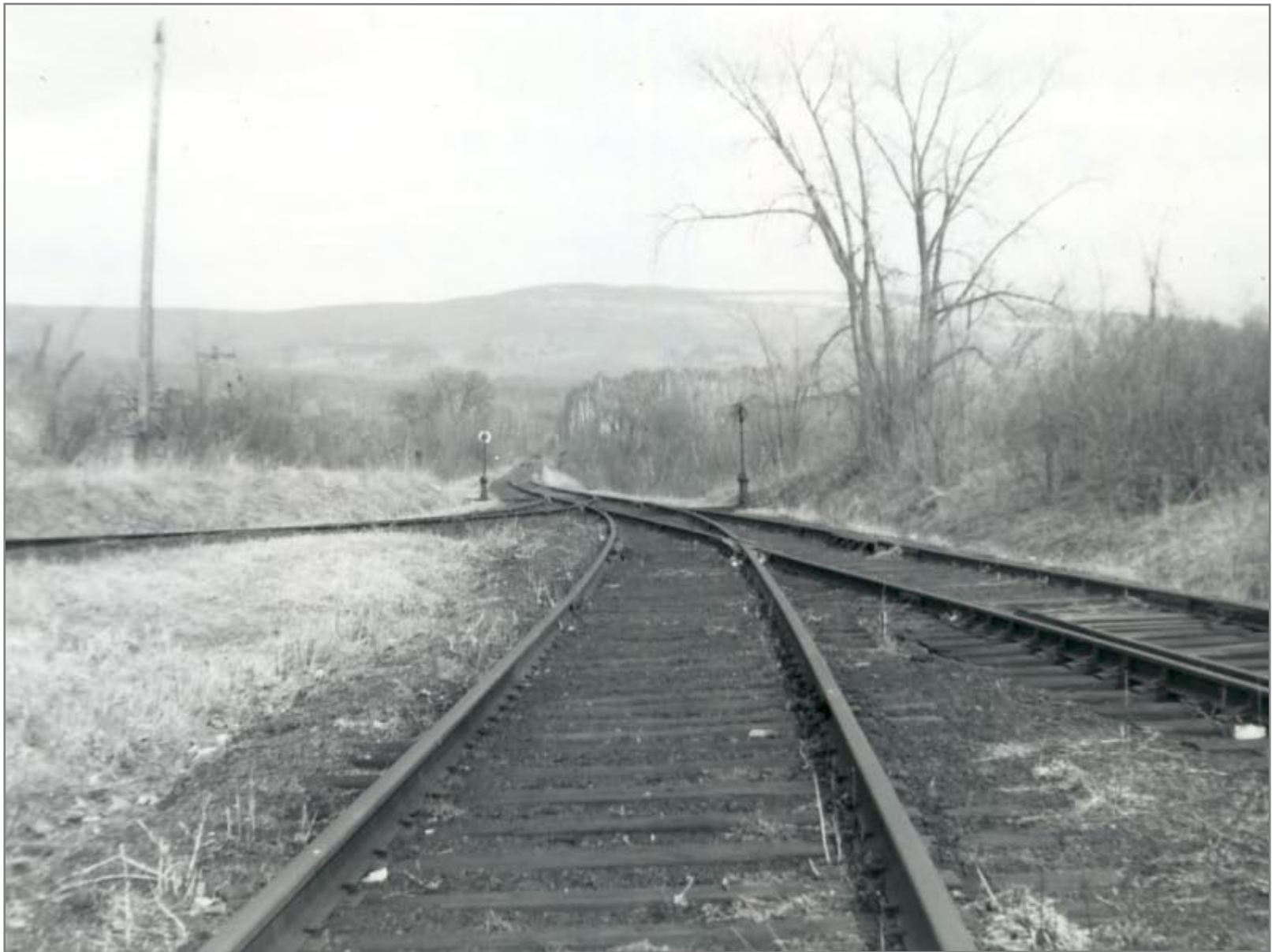
Looking South at beginning of North Bennington Wye 4/15/1962
