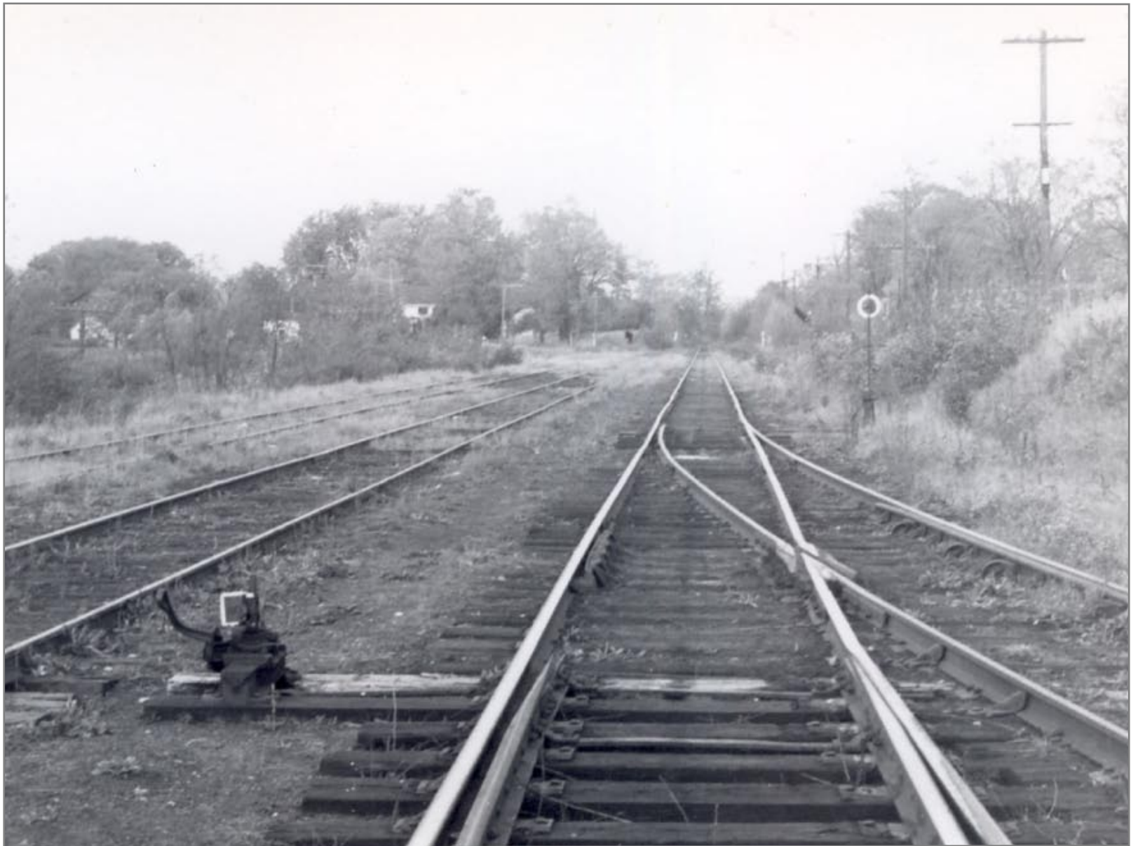
Looking North from No. Bennington toward Rutland 10/11/1964
