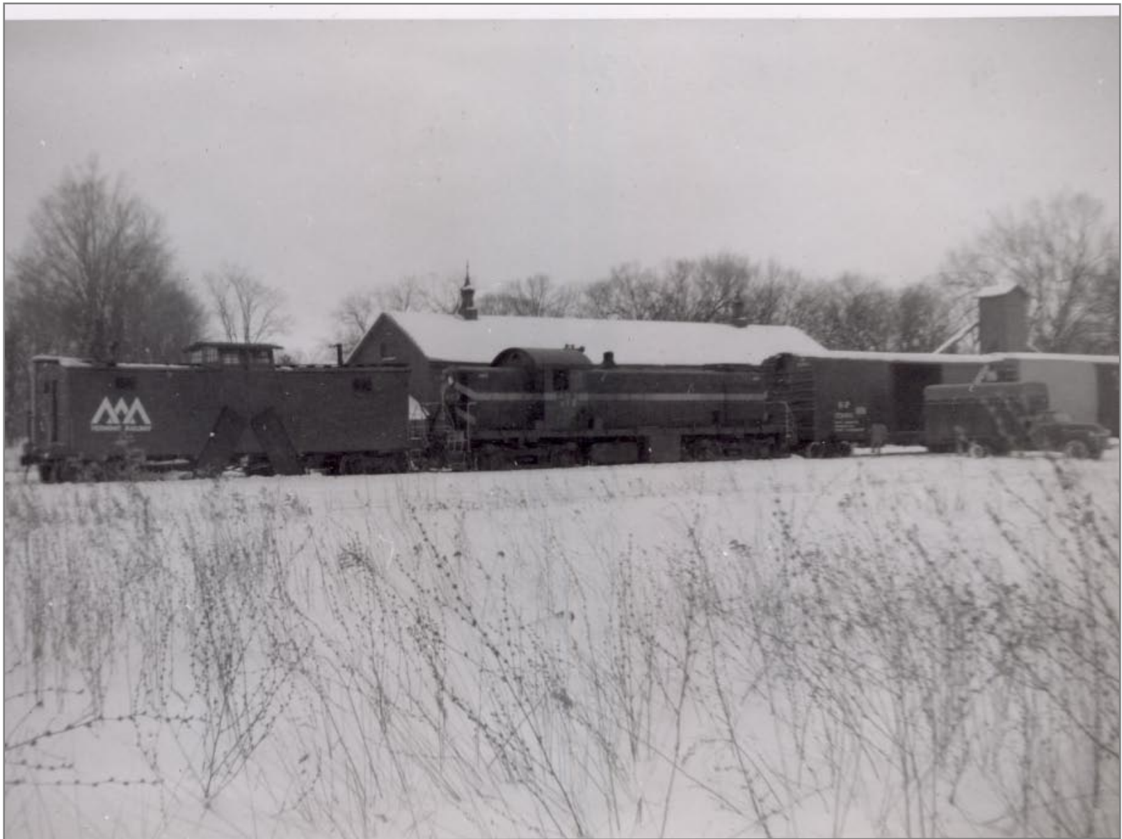
North Bennington Coal Shed & Warehouse in Background
