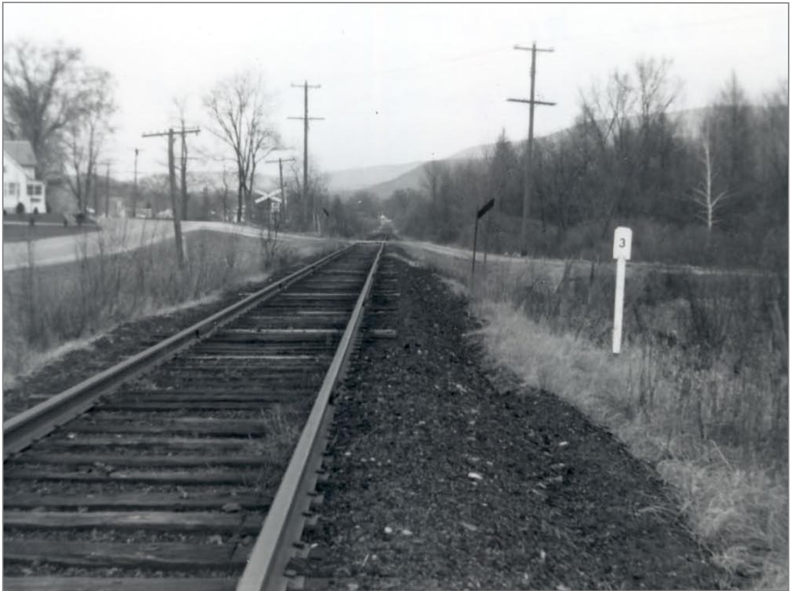
Milepost 3 on Right looking Northbound Route 67 on Left 4/21/1962
