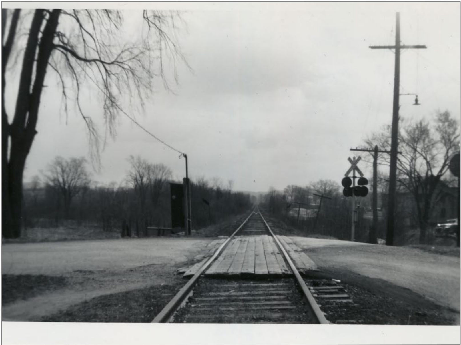
Looking Southbound Church Street Crossing 4/21/1962
