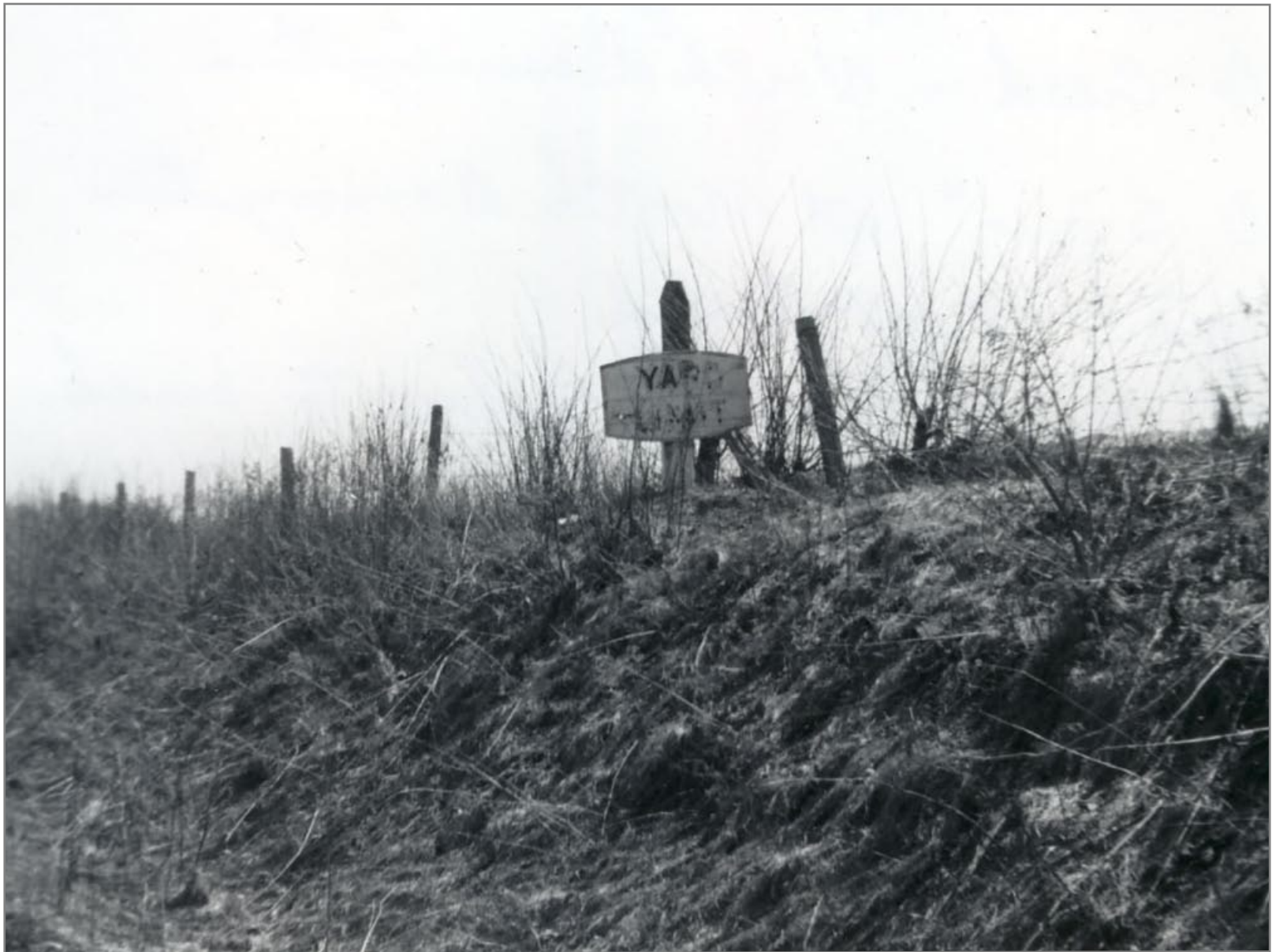
Yard Limit Sign for No. Bennington 4/21/1962
