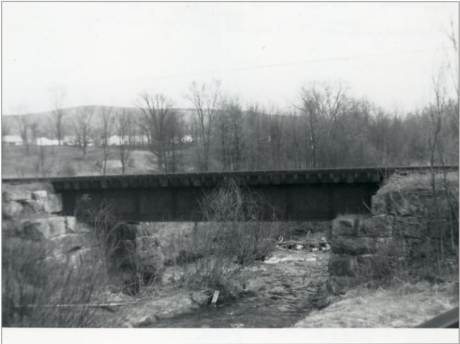
Bridge #59 Built by American Bridge Co. 1902
