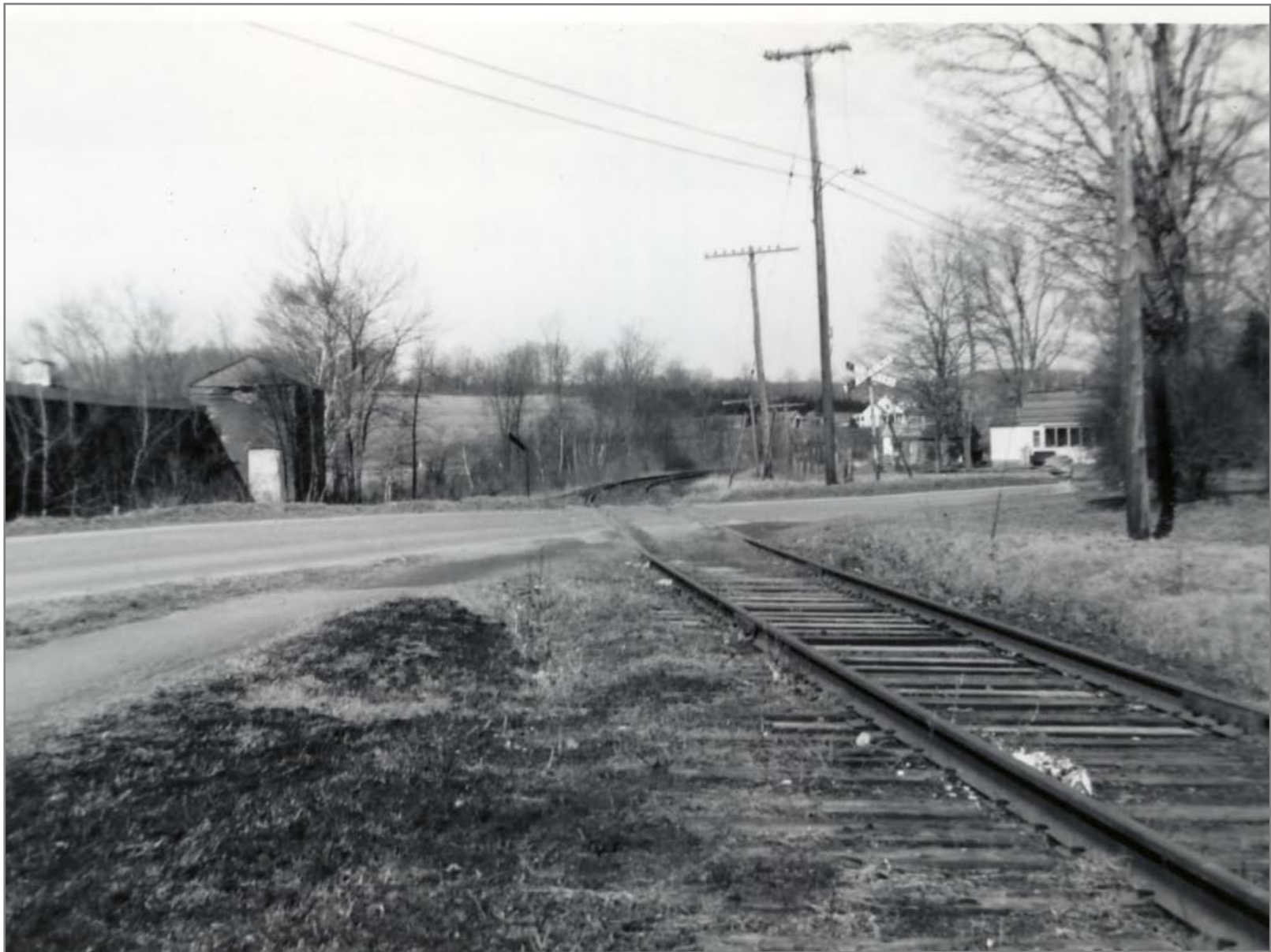
Looking West toward White Creek from North Bennington - Bennington & Hoosac Valley RR Car Barn on Left 3/22/1962
