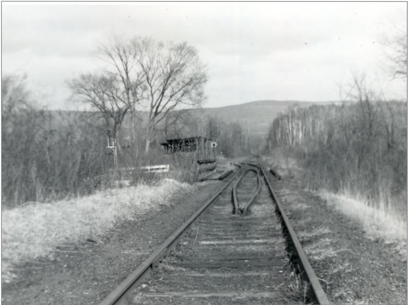
Looking South from North Bennington - Bridge is over outlet of Lake Paran, Coal Dealer on Left after Bridge 4/15/1962
