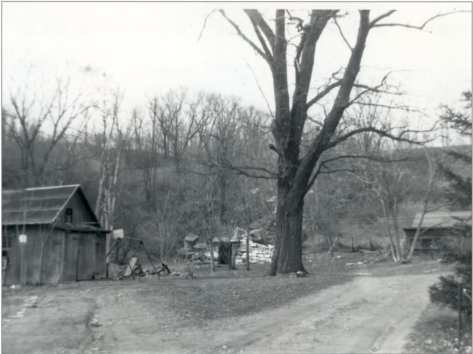
Looking North toward West End of Fill 4/15/1962
