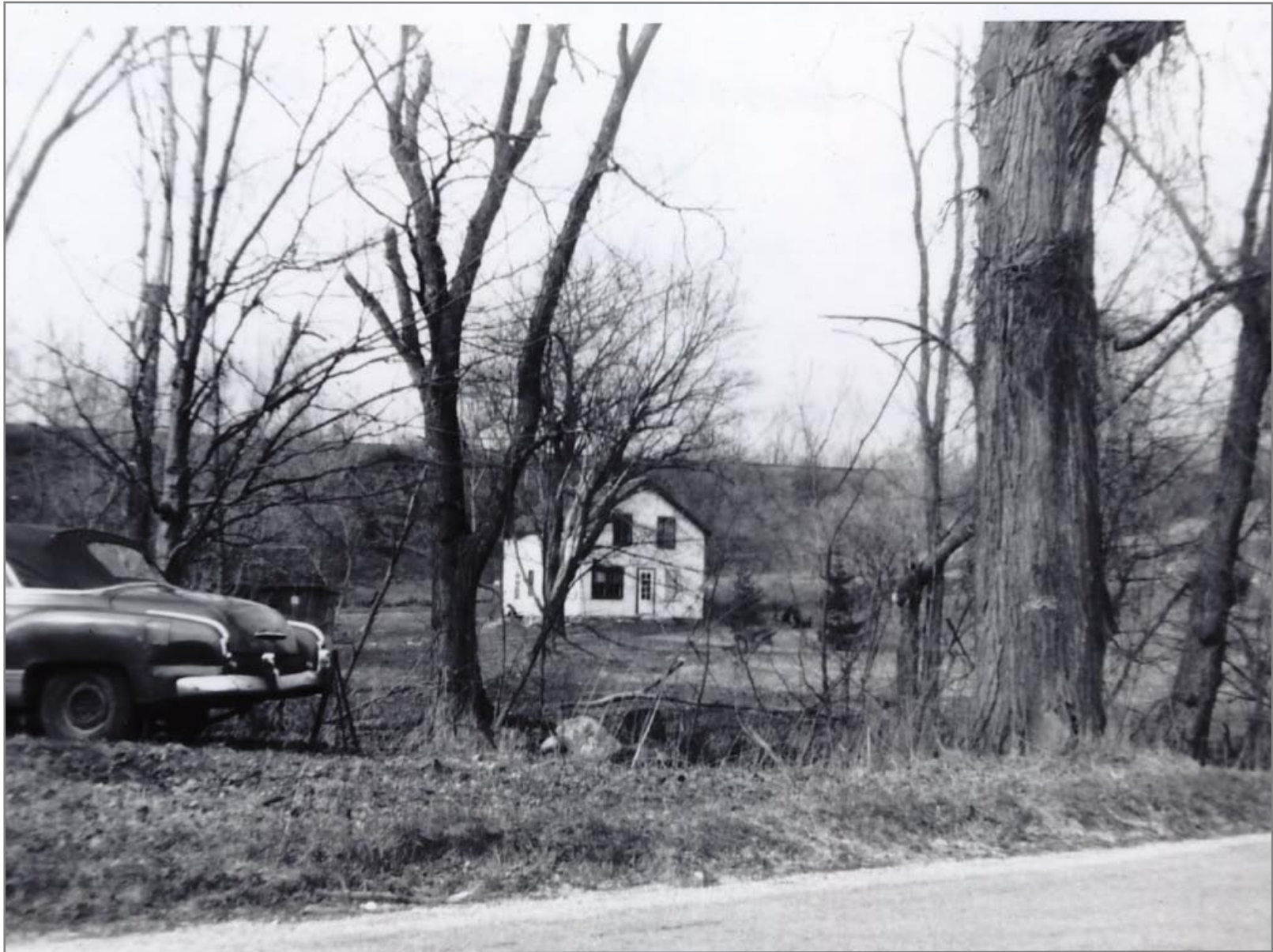
Looking North From Route 67 at High Fill Over Cold Spring Creek 4/15/1962
