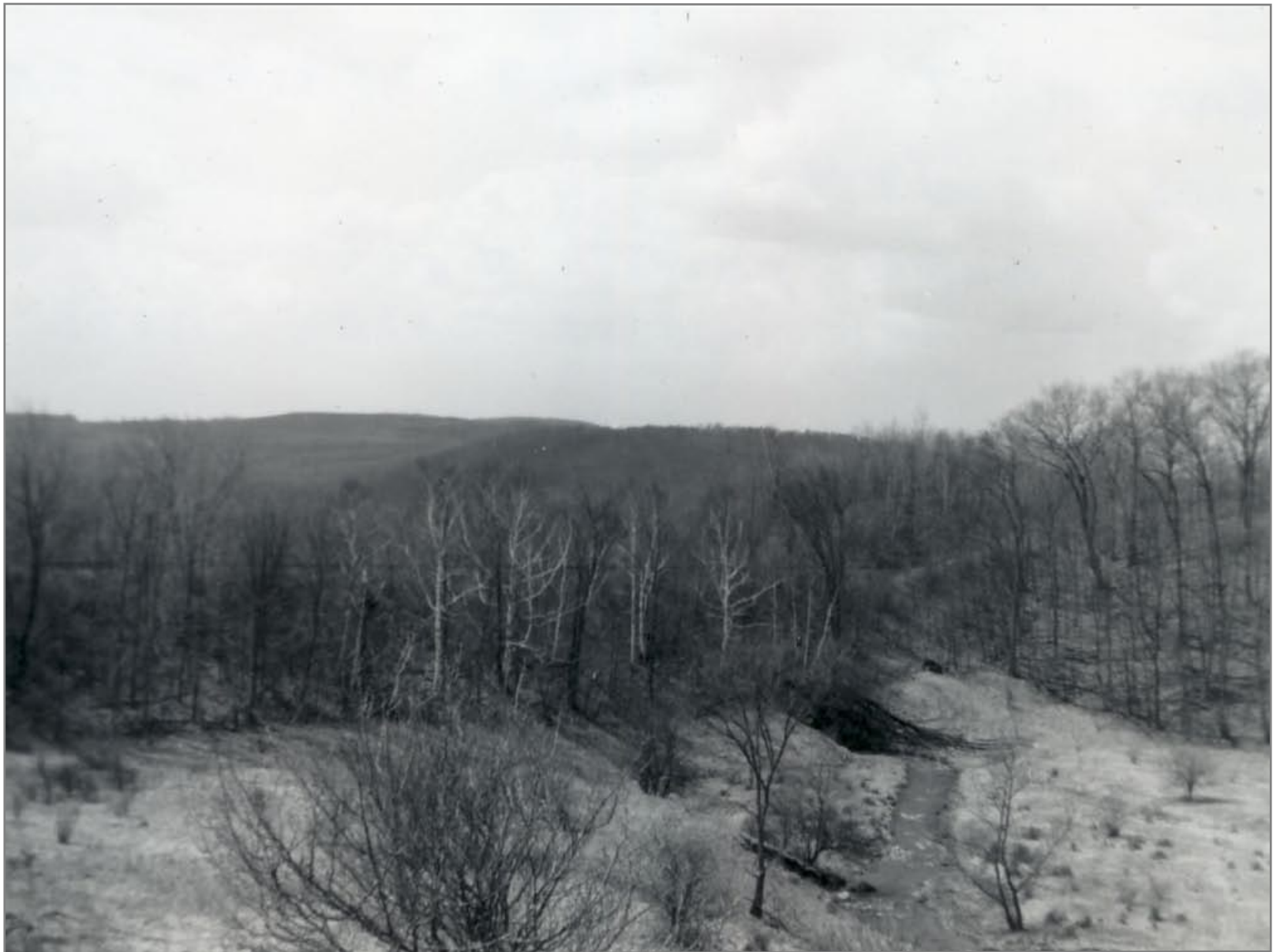
Looking South at Rutland Embankment over Cold Spring Creek 4/20/1962
