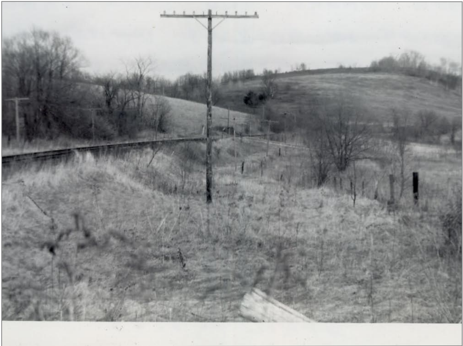
Looking East To Vermont - Old Spur on Right Heading Behind White Creek Station 4/15/1962
