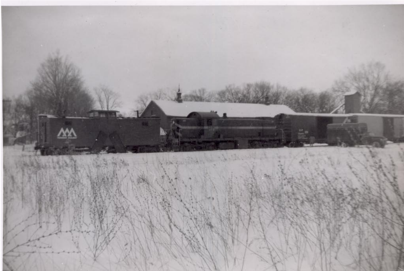
North Bennington Coal Shed & Warehouse in Background
