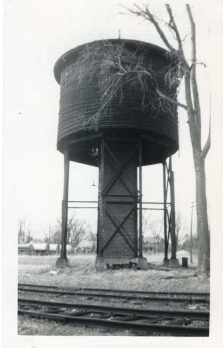
North Bennington Water Tank 1962
