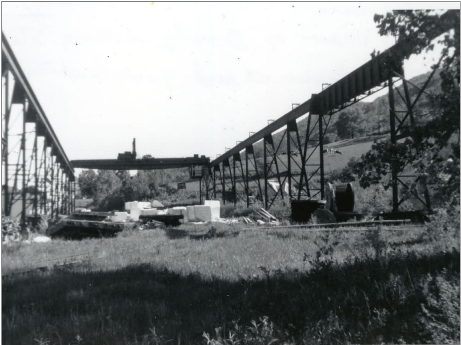
VT Marble 40 Ton Crane in Background 5/27/1962
