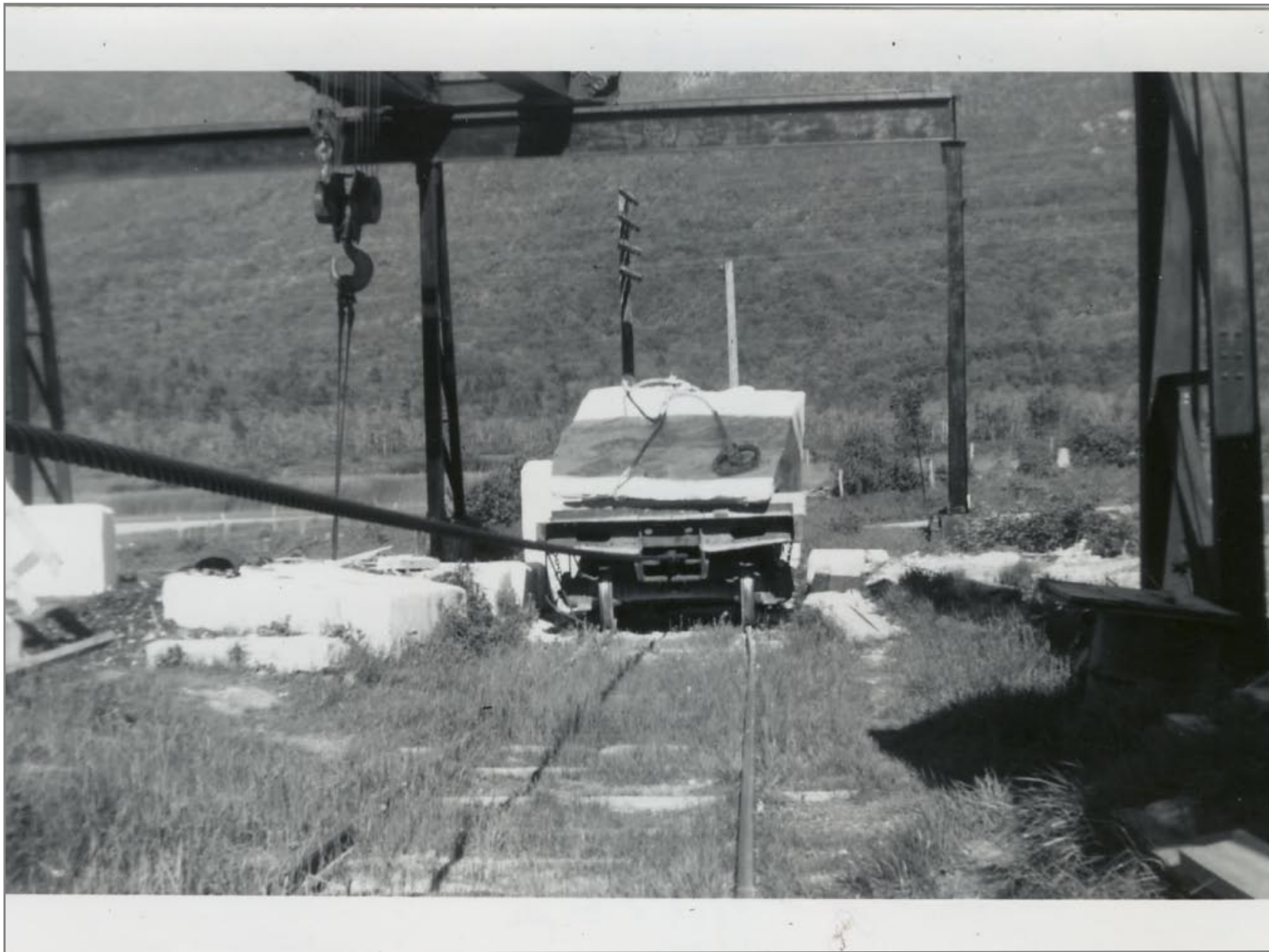
Foot of Incline to Quarry Flat Car w/ 1-12" Cable Attached 5/27/1962
