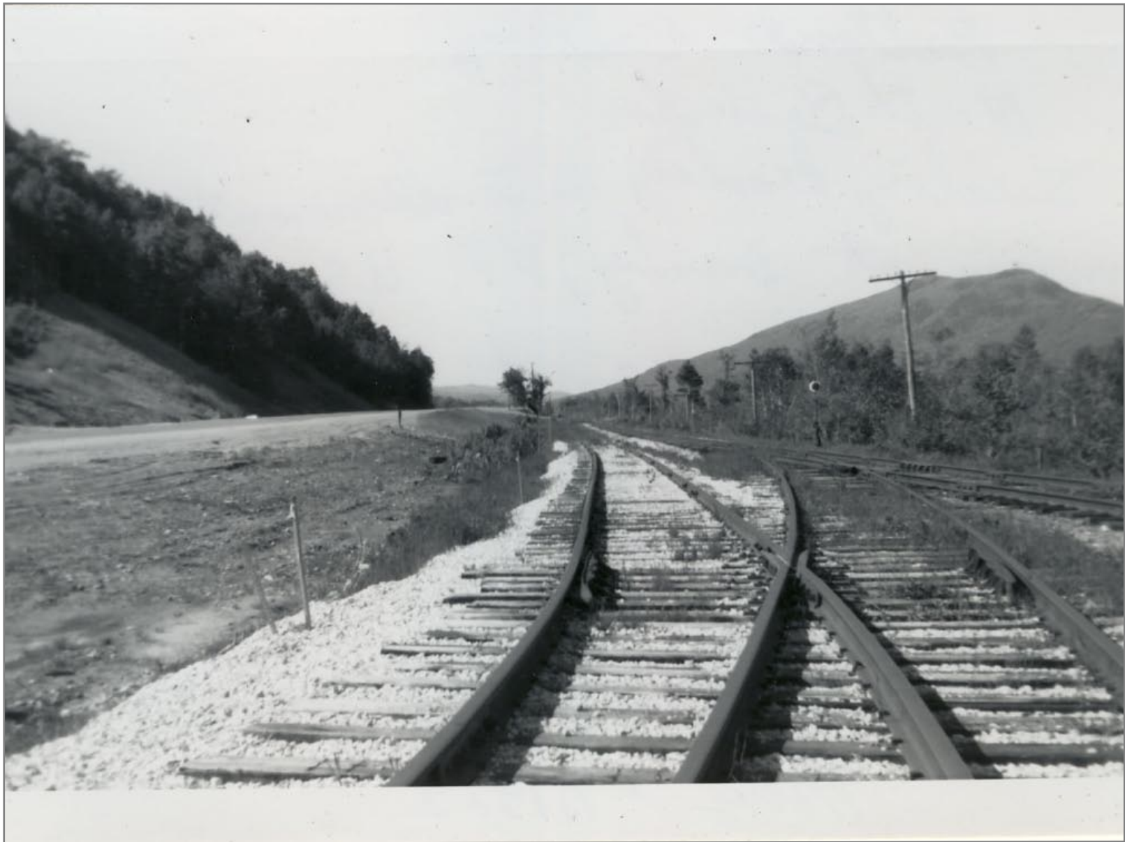
Looking Northbound Track on Left is Long Siding of VT Marble - Track on Right Rutland Main 5/27/1962
