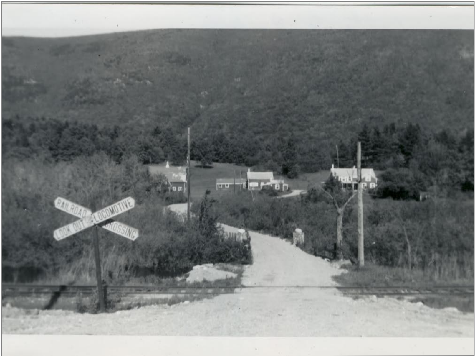
1st Crossing South of Danby Looking East 5/27/1962
