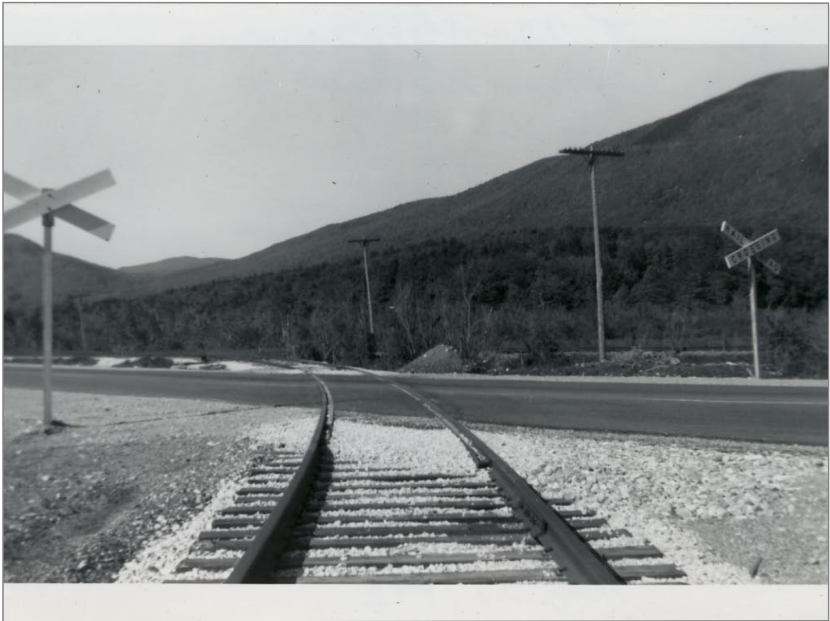
Siding to Vermont Marble Company looking back to Main 5/27/1962
