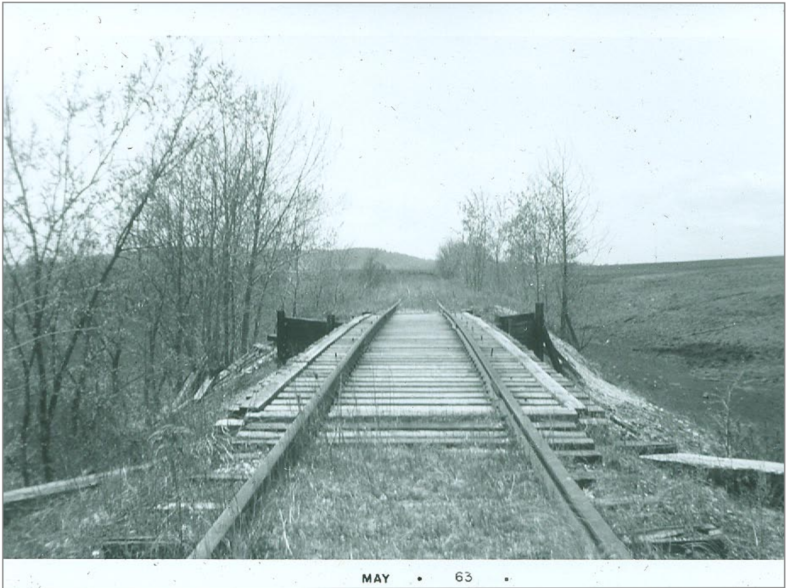
West over trestle back toward Rutland main
