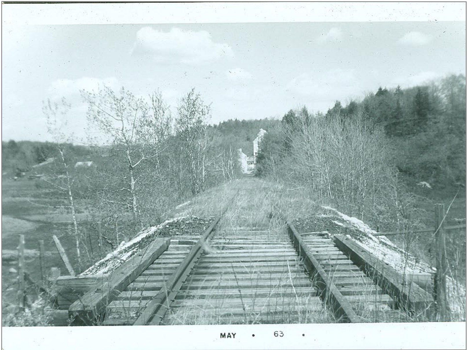
East over trestle into Vt. Lime
