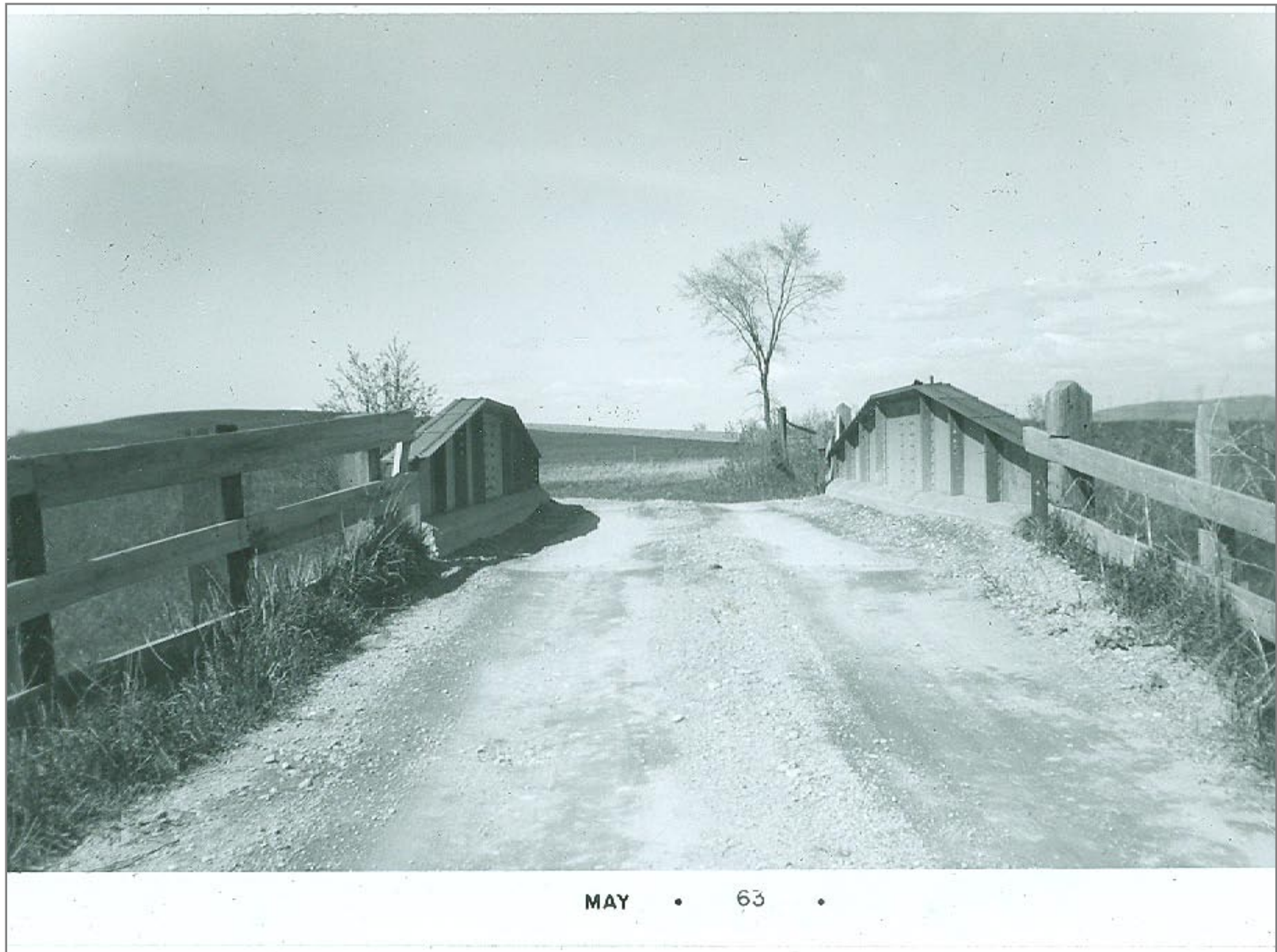
Looking East on Bridge 248
