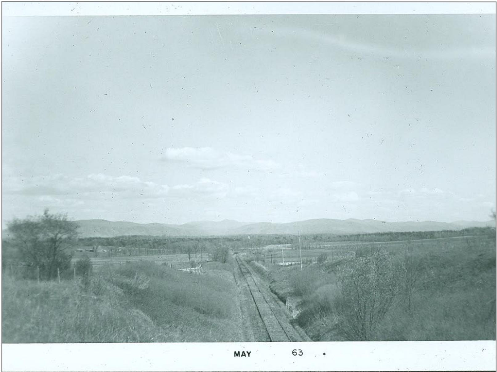
View from Bridge 248 South
