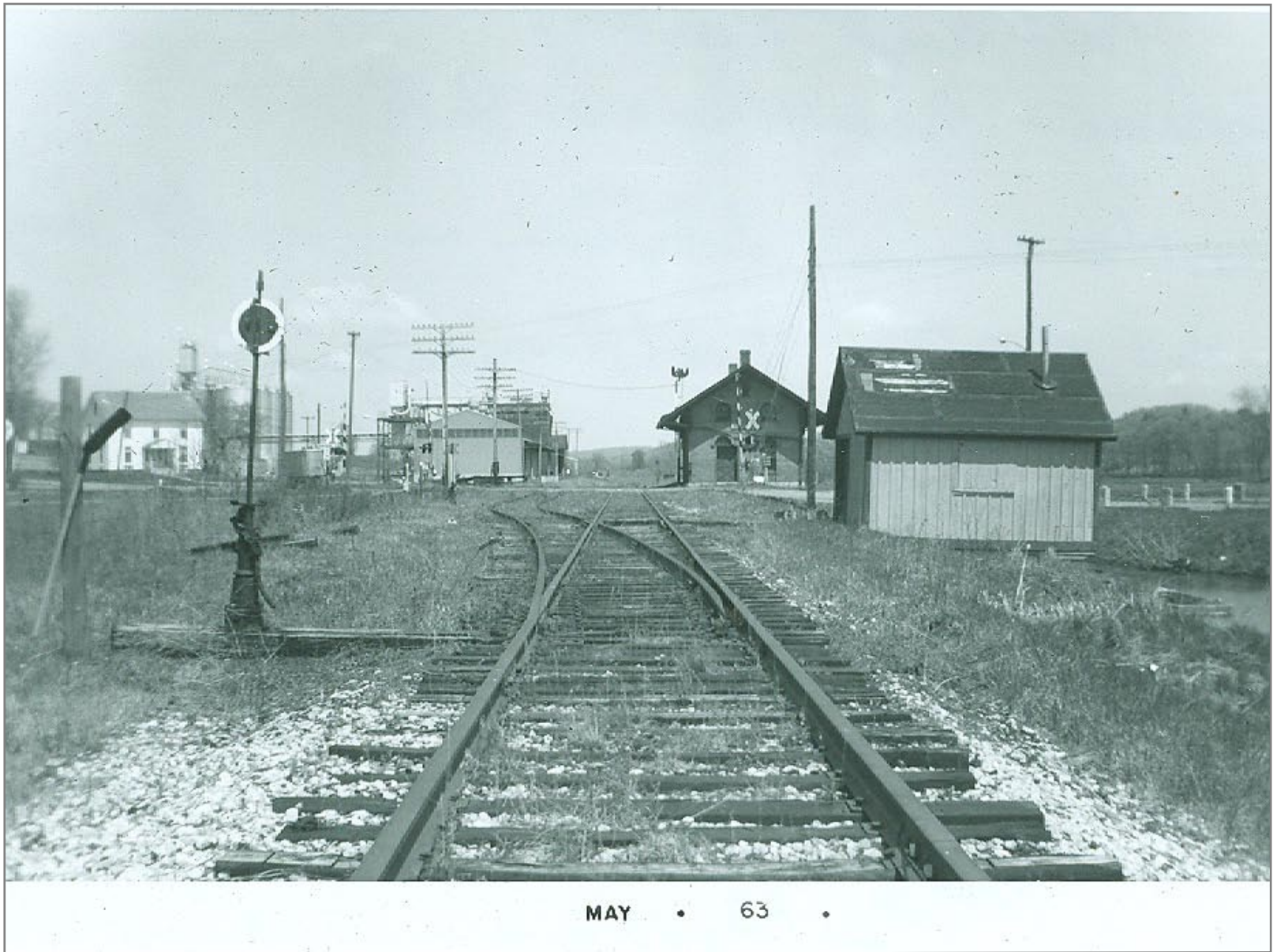
Northbound into New Haven
