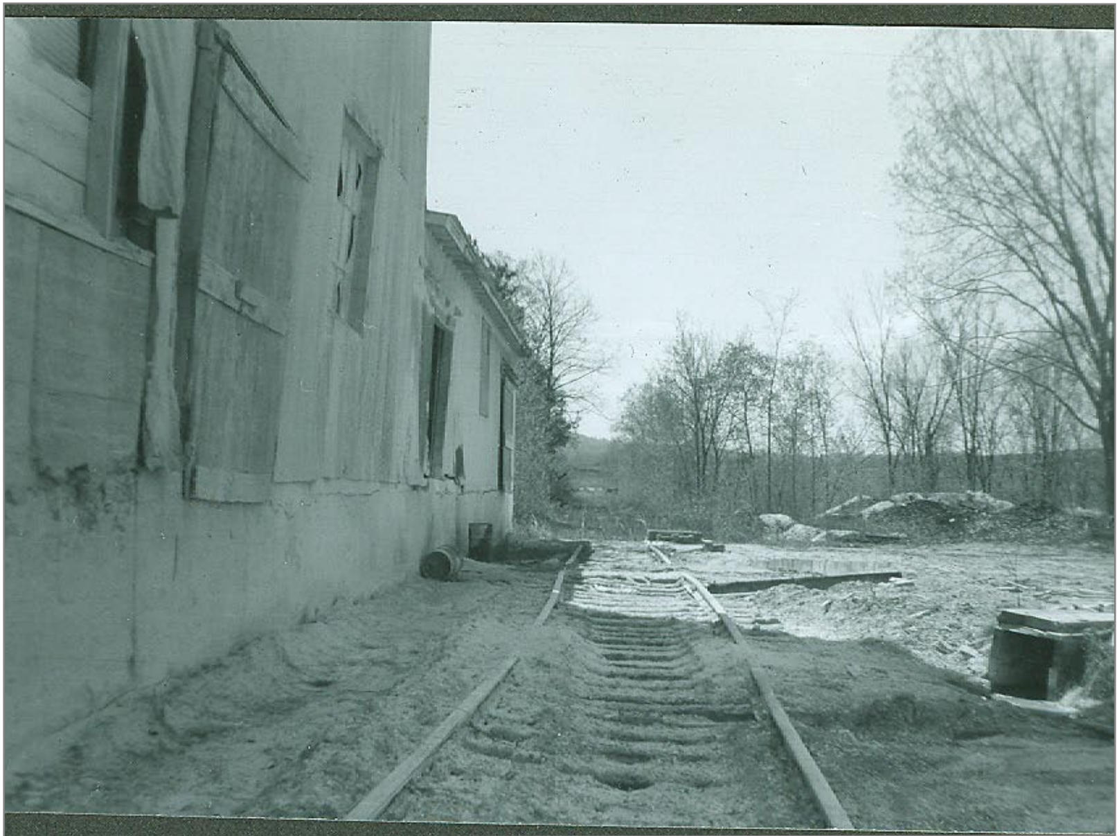
Vermont Lime looking west to Rutland main
