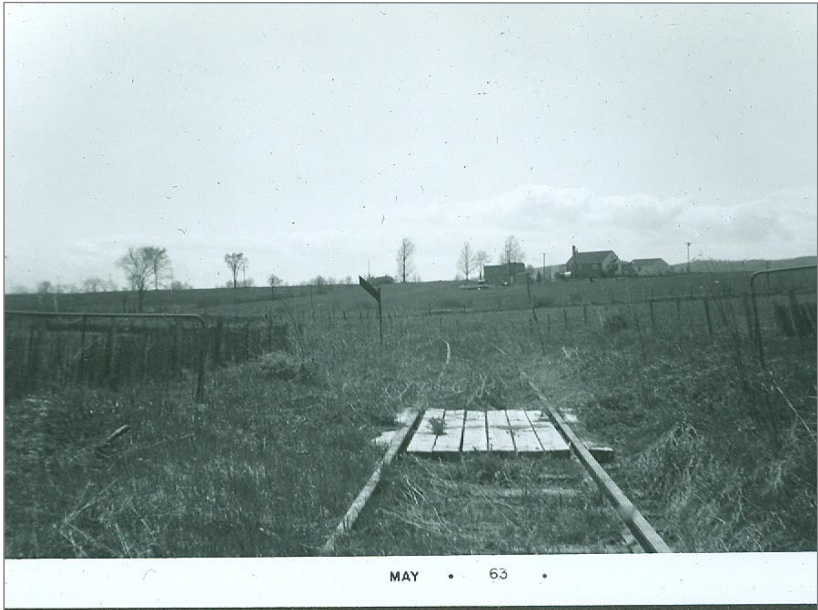
Crossing on Peck's Siding looking West
