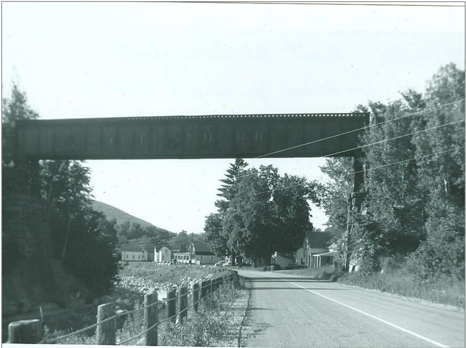
Bridge 146 East View - American Bridge Company 1902
