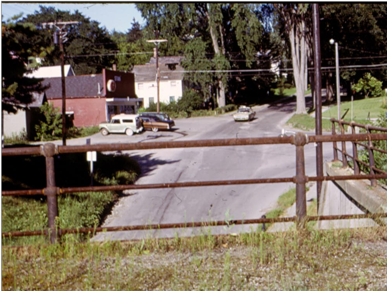
Looking East on bridge 241a
