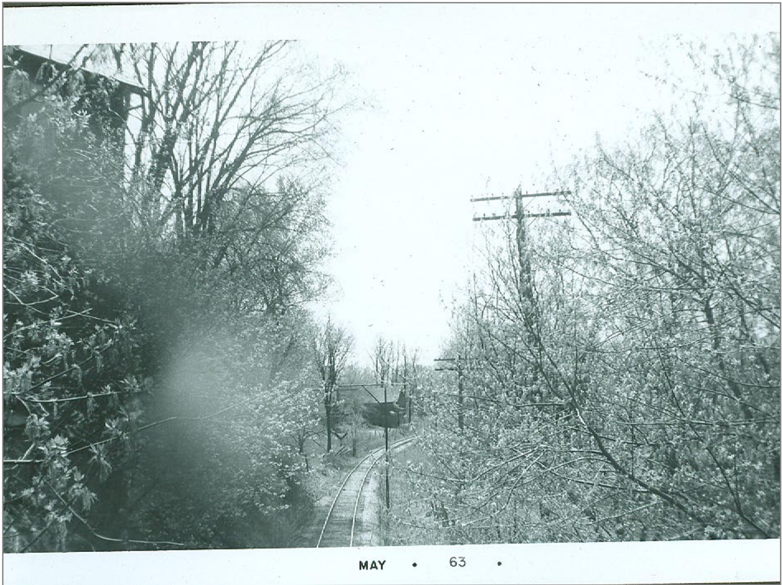
Standing on bridge 240 Southbound
