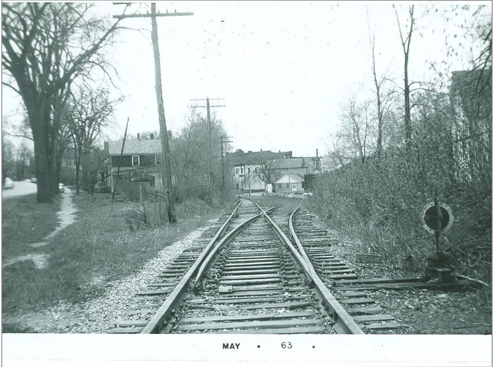
Southbound near Middlebury Depot
