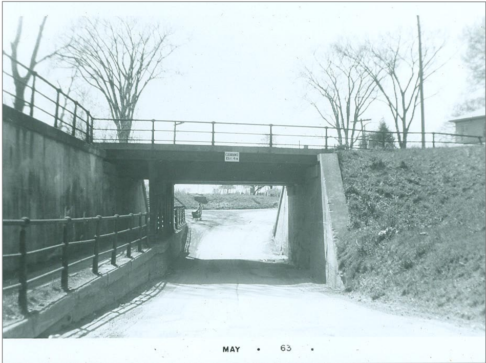
Bridge 241a just north of Station
