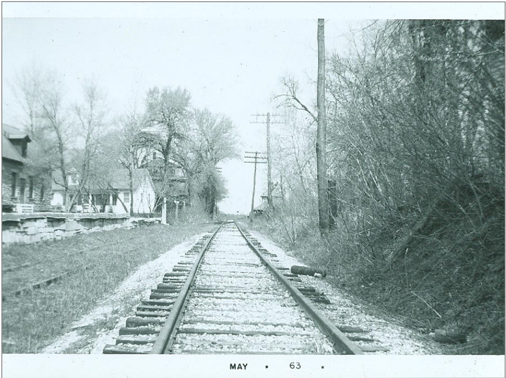
Northbound with station on right
