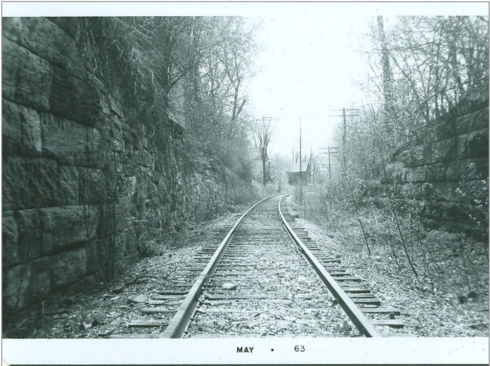
Under bridge 240 Southbound
