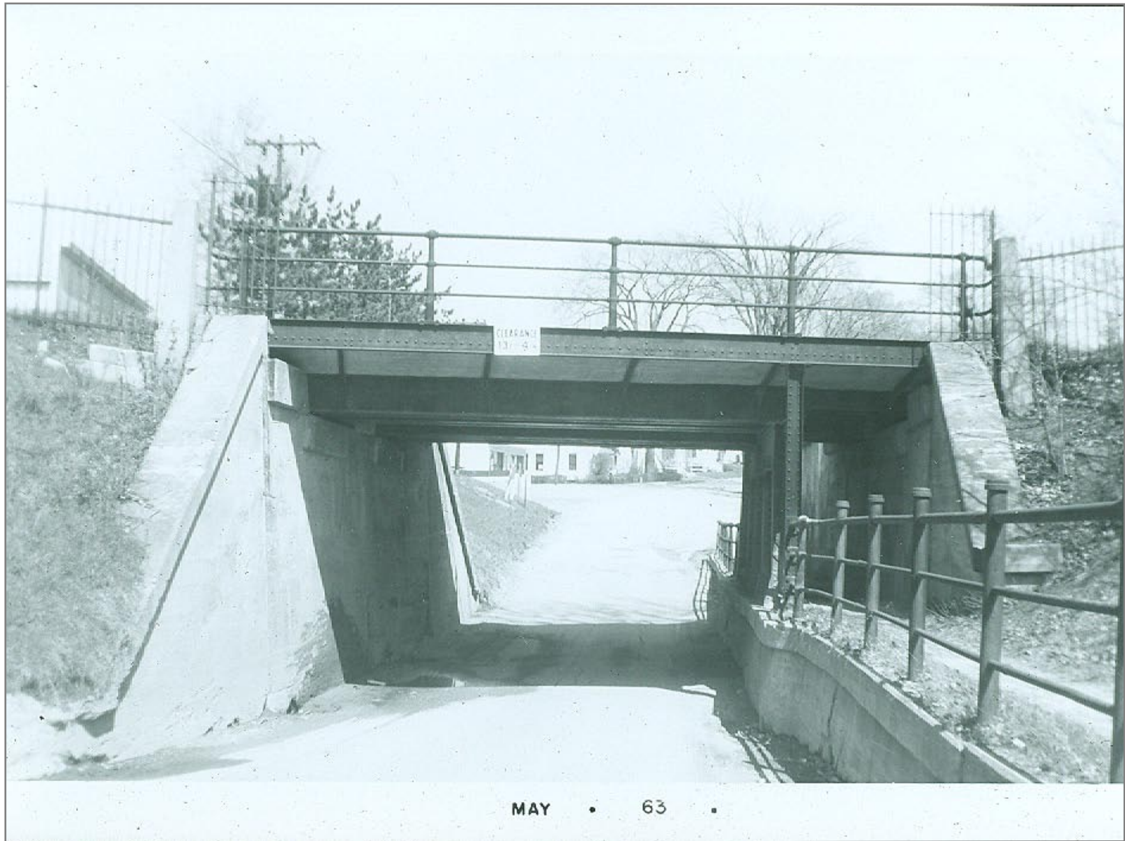
Bridge 241A looking east
