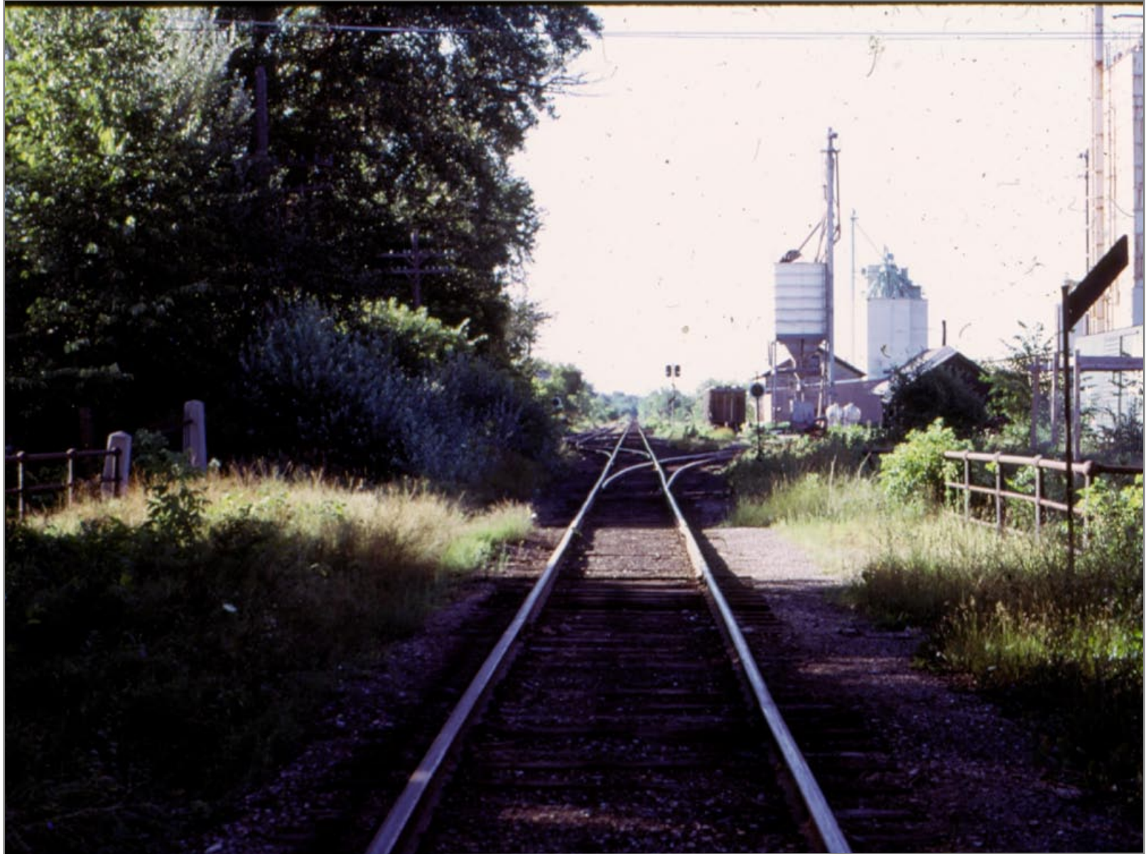
Northbound over bridge 242
