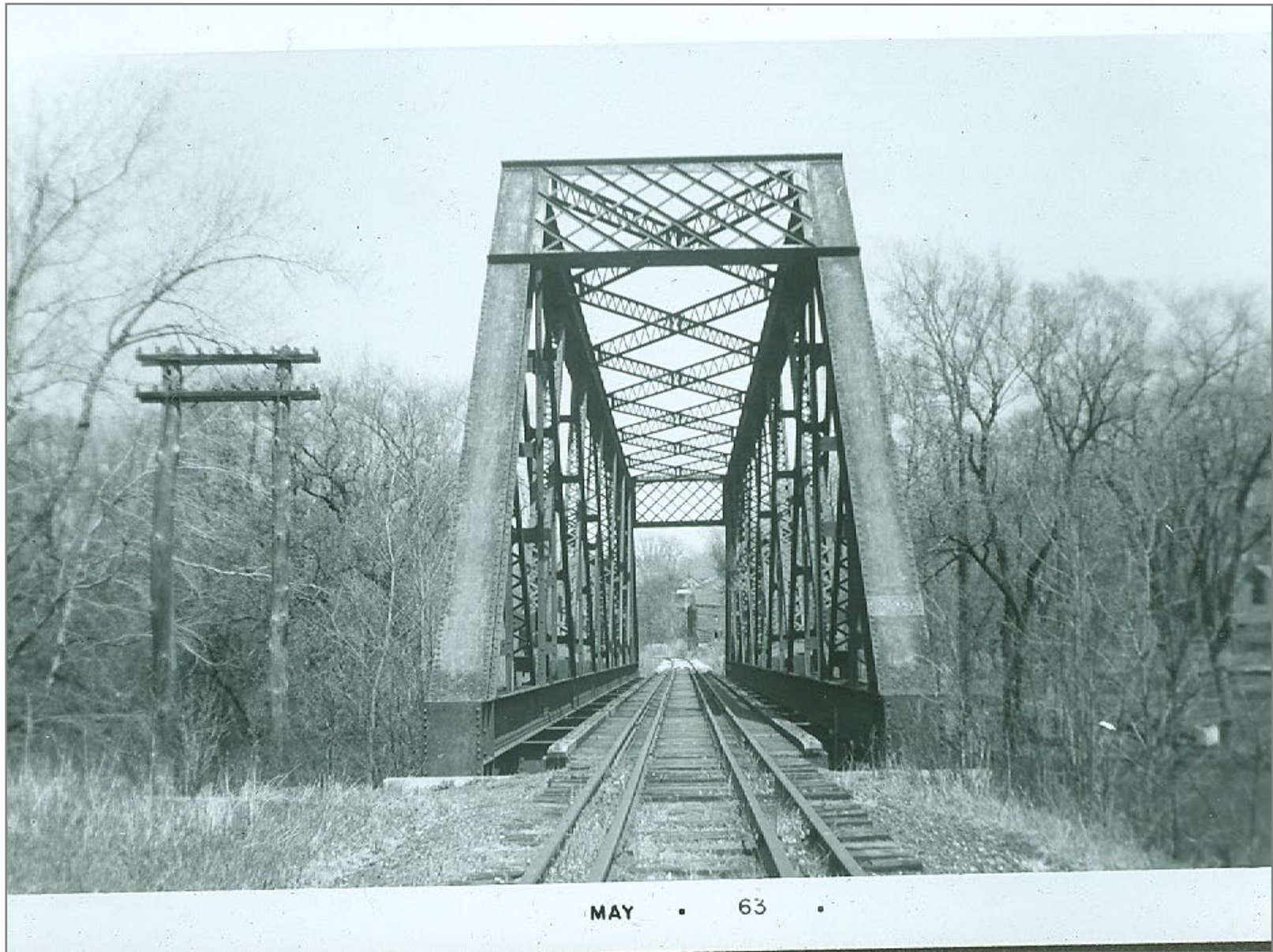
Bridge 239 Northbound into Middlebury
