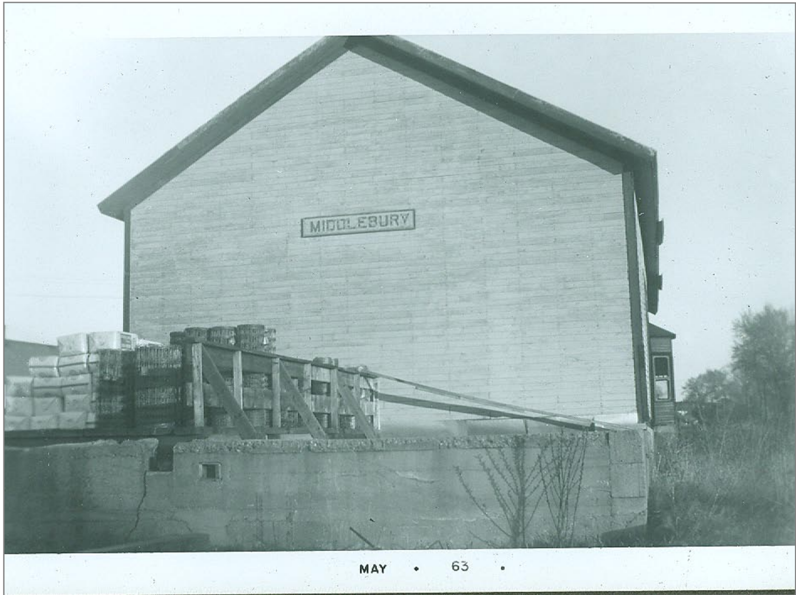
Southbound at Middlebury Freight House
