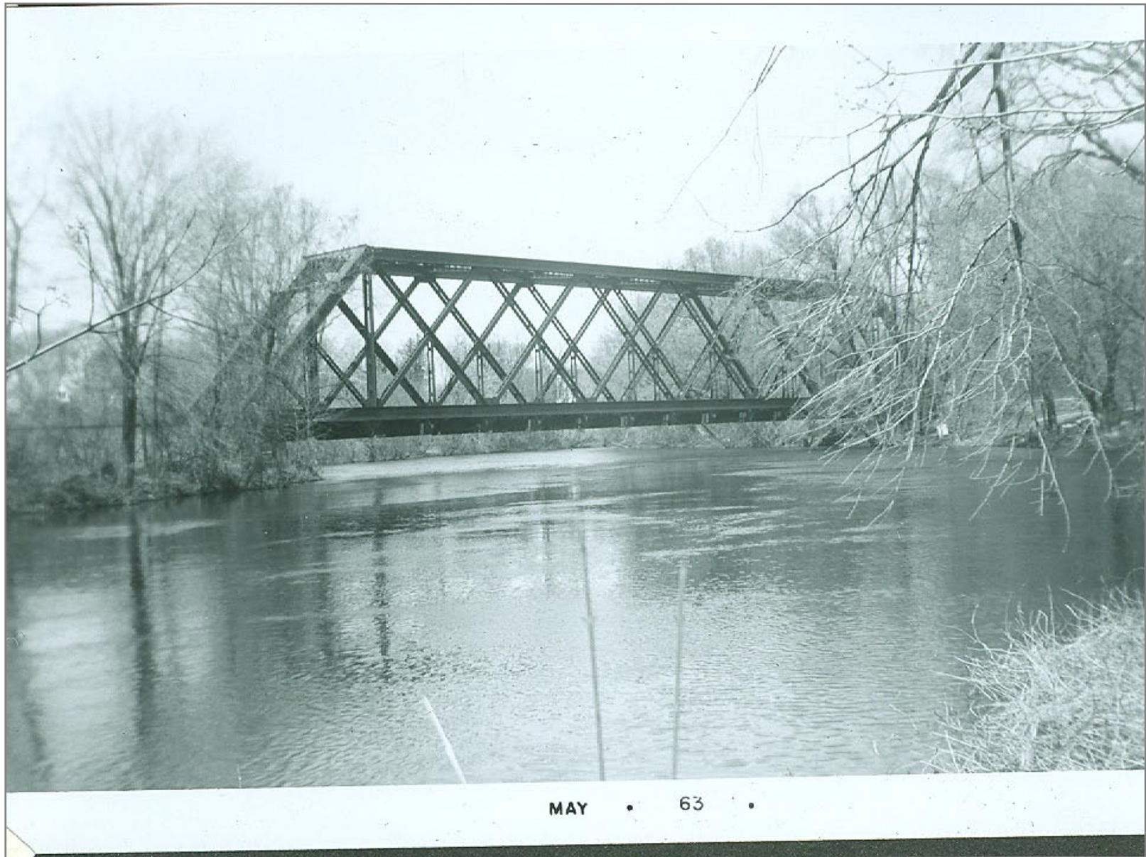
Bridge 239 just south of Middlebury
