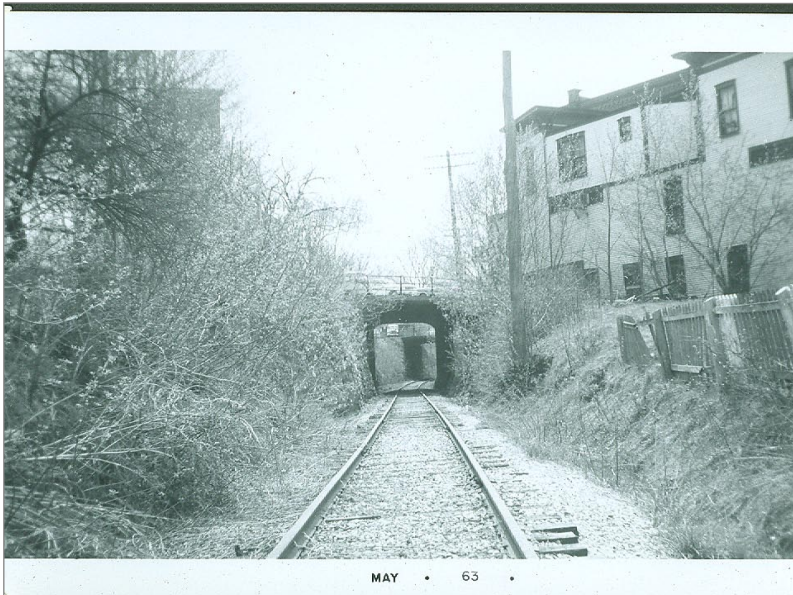
Bridge 240 Northbound - Bourdon Insurance Building on right
