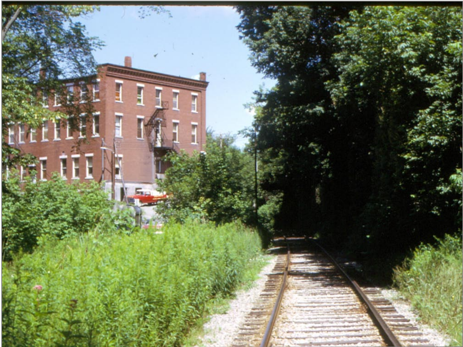
Northbound into Bridge/Tunnel 240 - Battell Block on left
