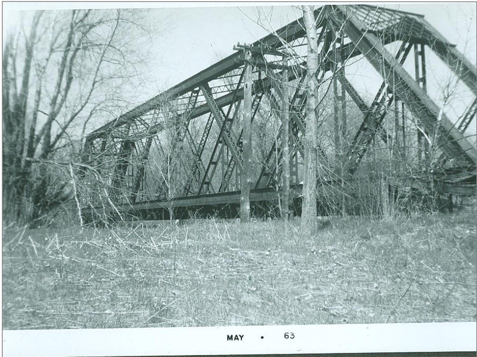
Bridge 239 just south of Middlebury
