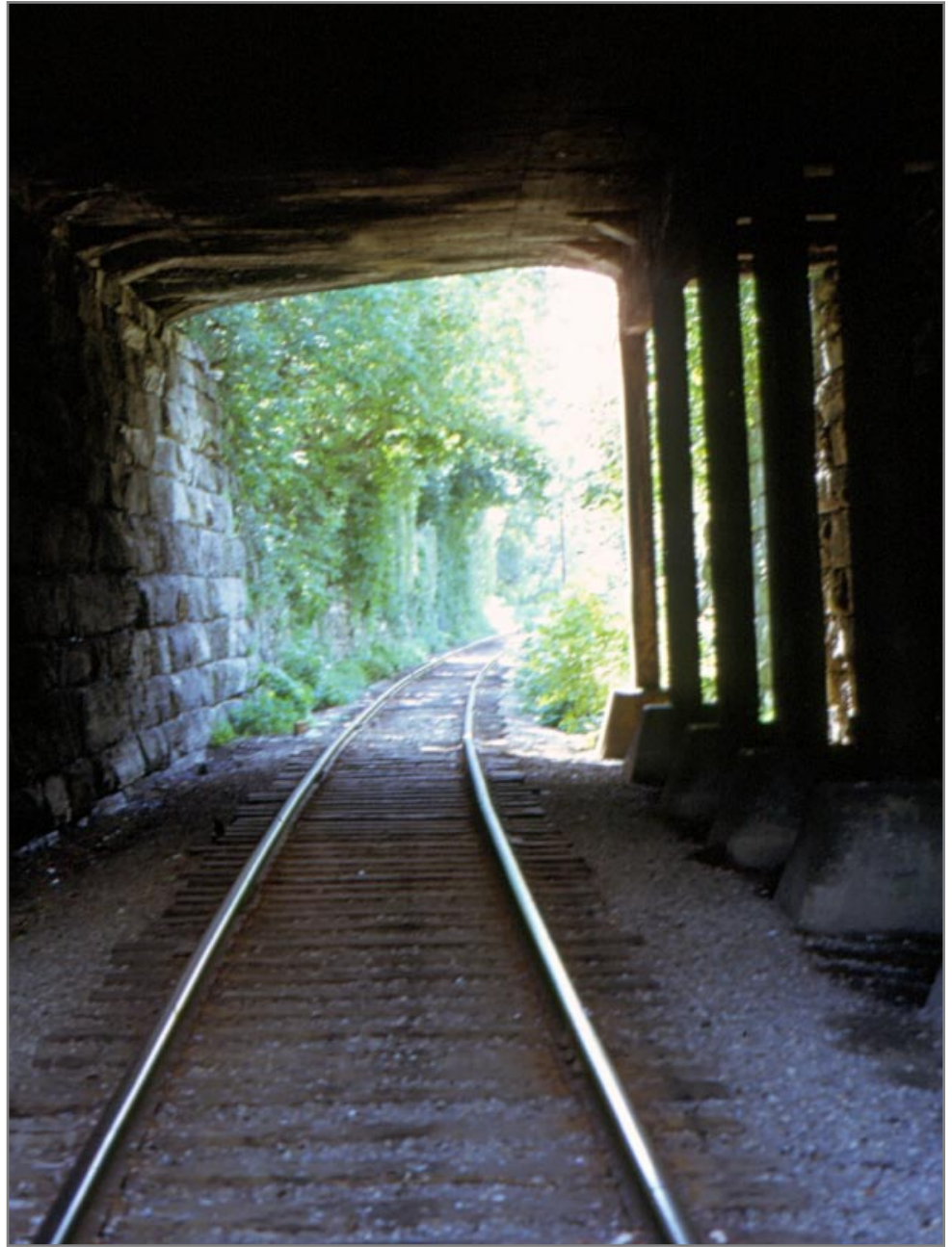
Under Bridge/Tunnel 240 Southbound
