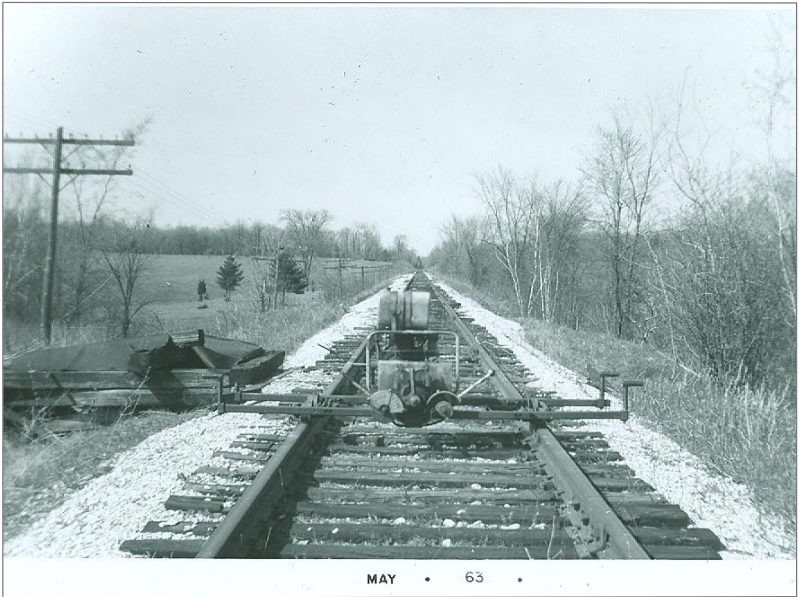
Northbound out of Middlebury - rail grinding machine
