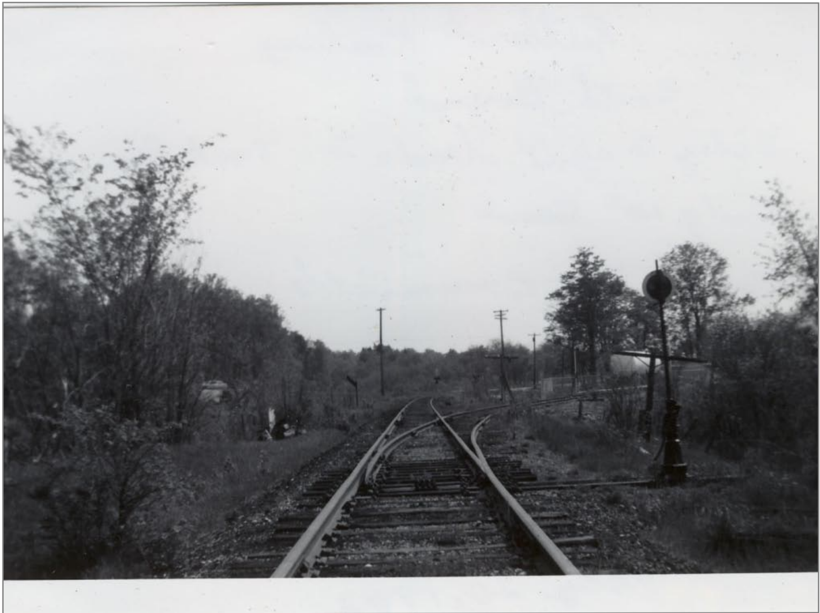
Switch to Pyrofax on Right Looking Southbound Toward Manchester 5/20/1962
