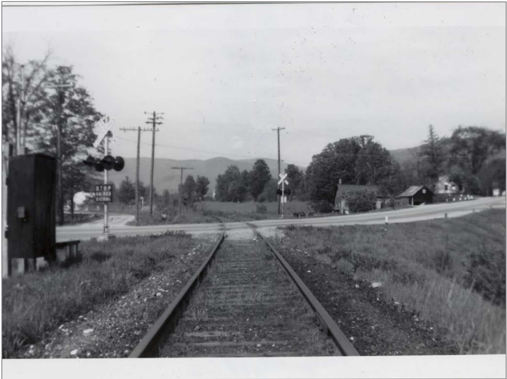
Crossing Just North of Bridge 71 Manchester 5/20/1962
