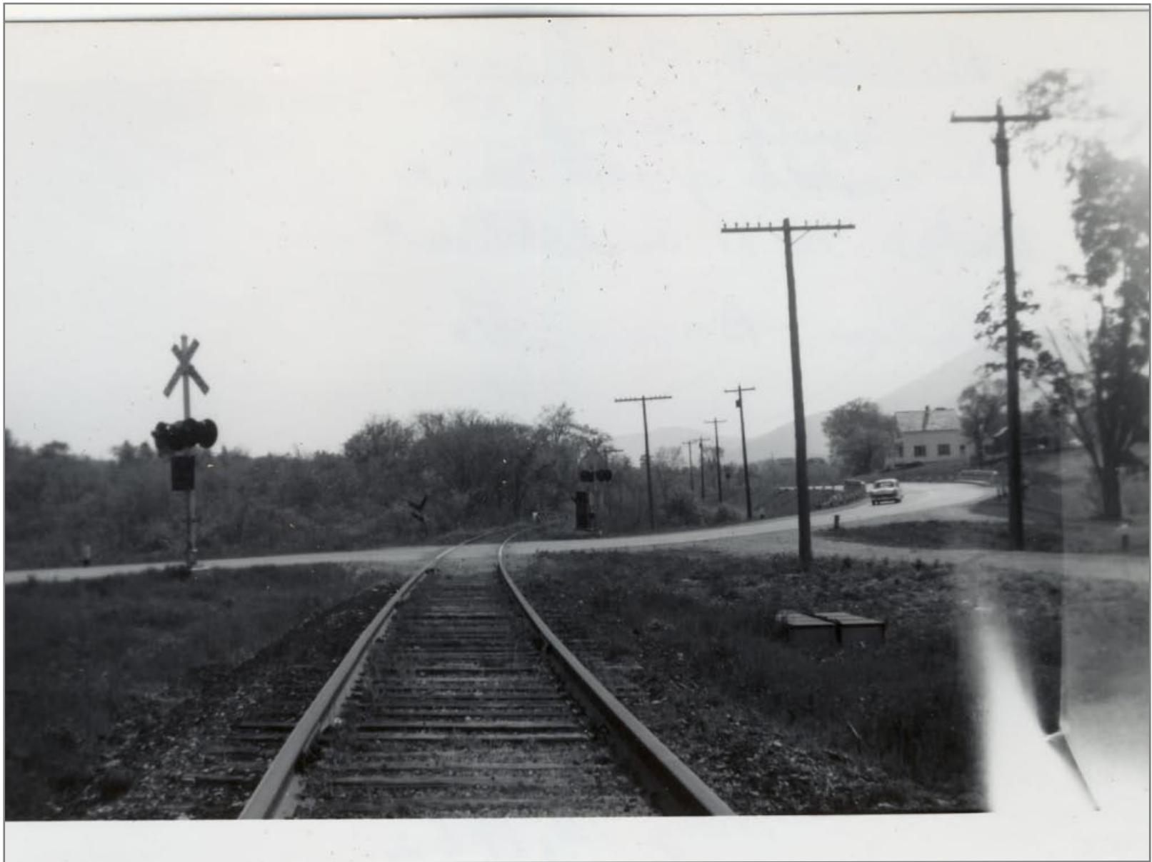
Southbound Bridge 71 in Distance 5/20/1962
