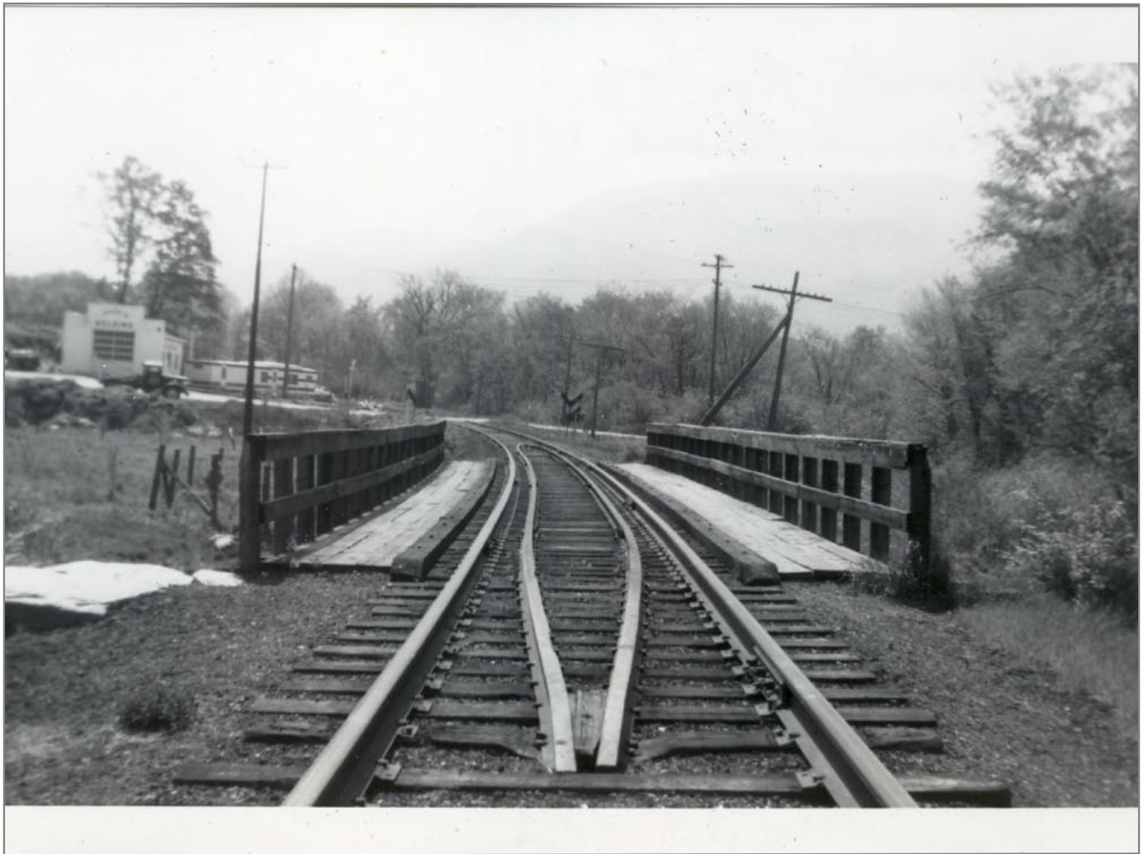
Southbound thru Bridge 70 5/20/192
