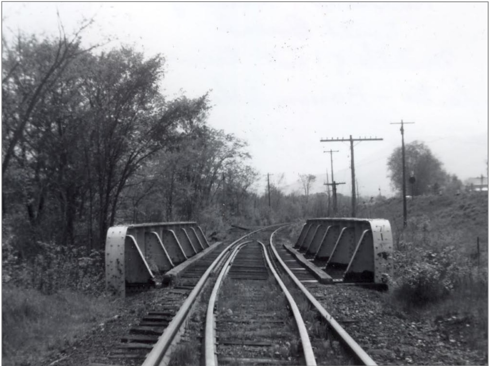
Bridge 71 Southbound Built by American Bridge Company 1903 5/20/1962
