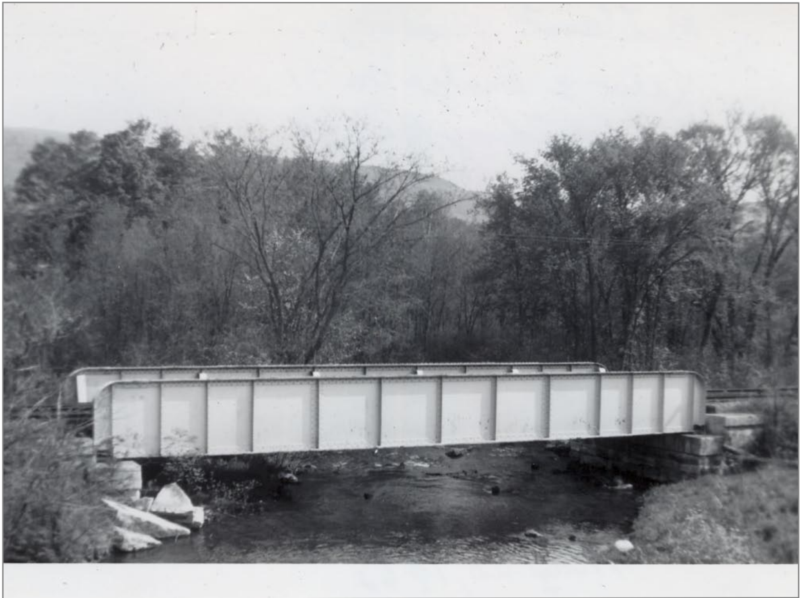
Bridge 71 Painted Aluminum 5/20/1962
