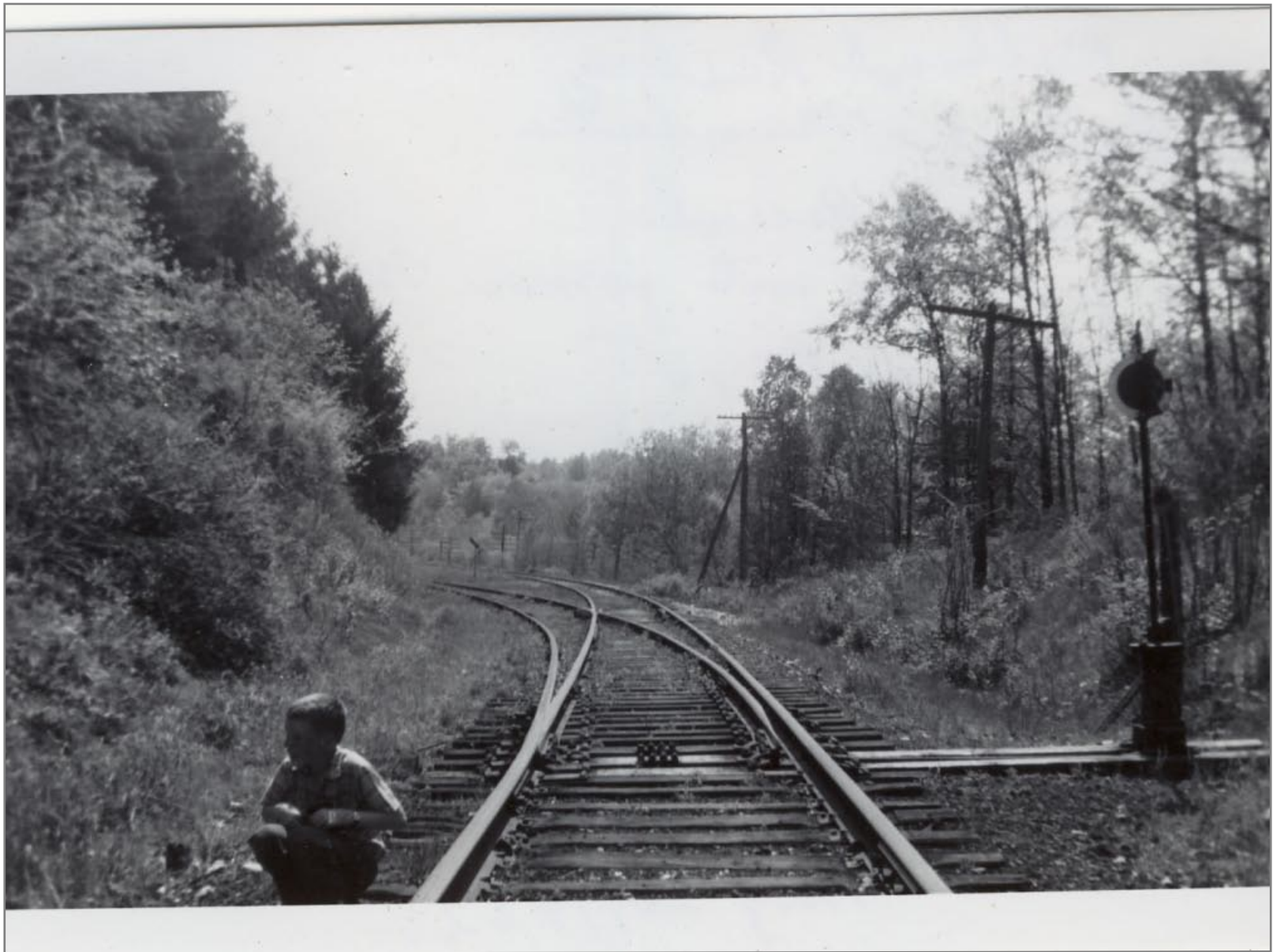
Southbound Switch into Milk Plant 5/20/1962
