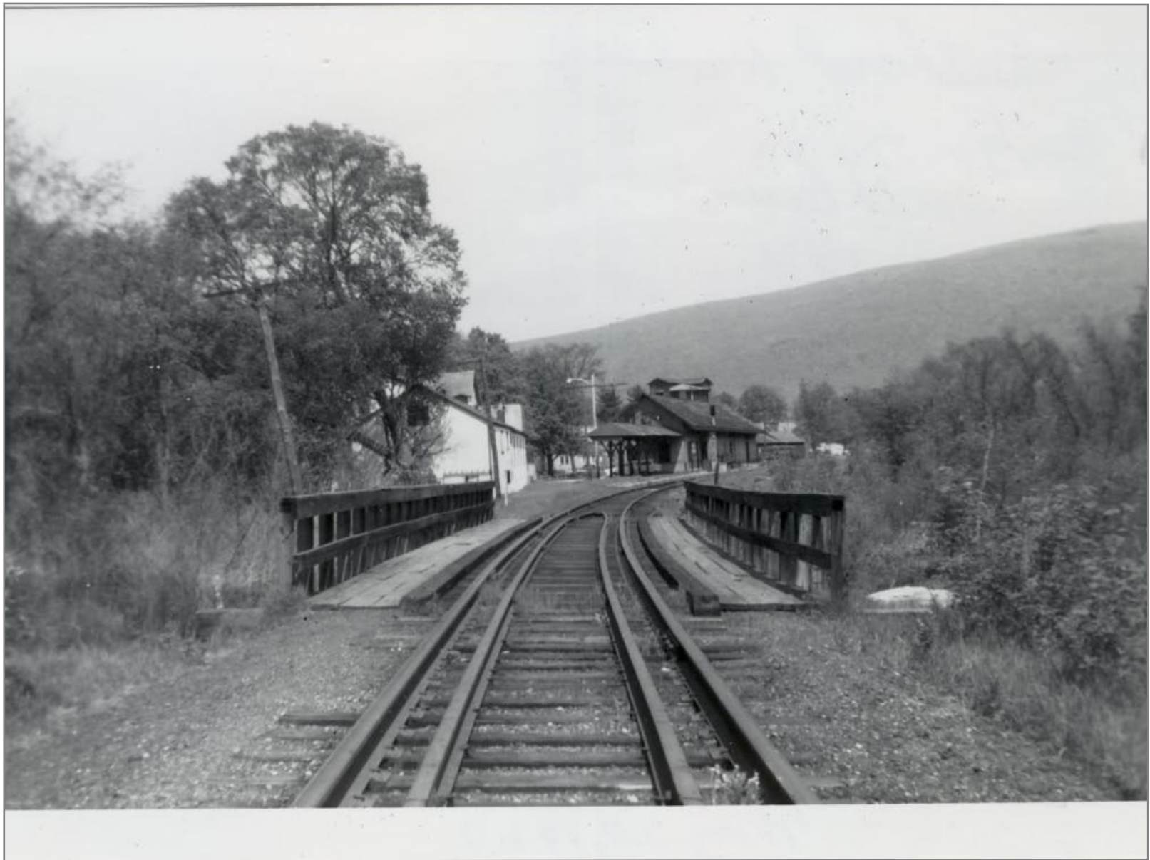
Northbound at Bridge 70 5/20/1962
