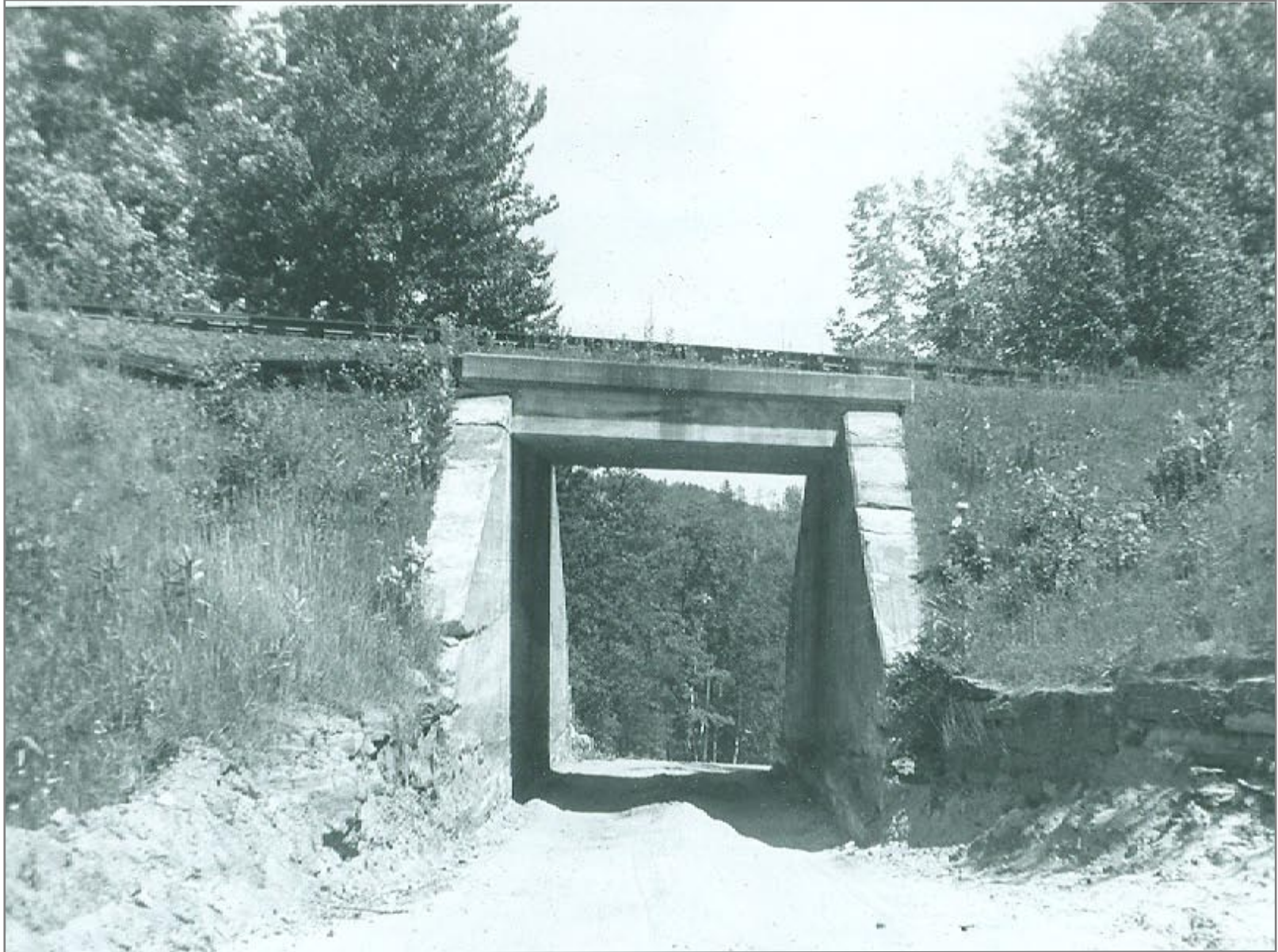
Bridge 137 North of Ludlow 7/4/62
