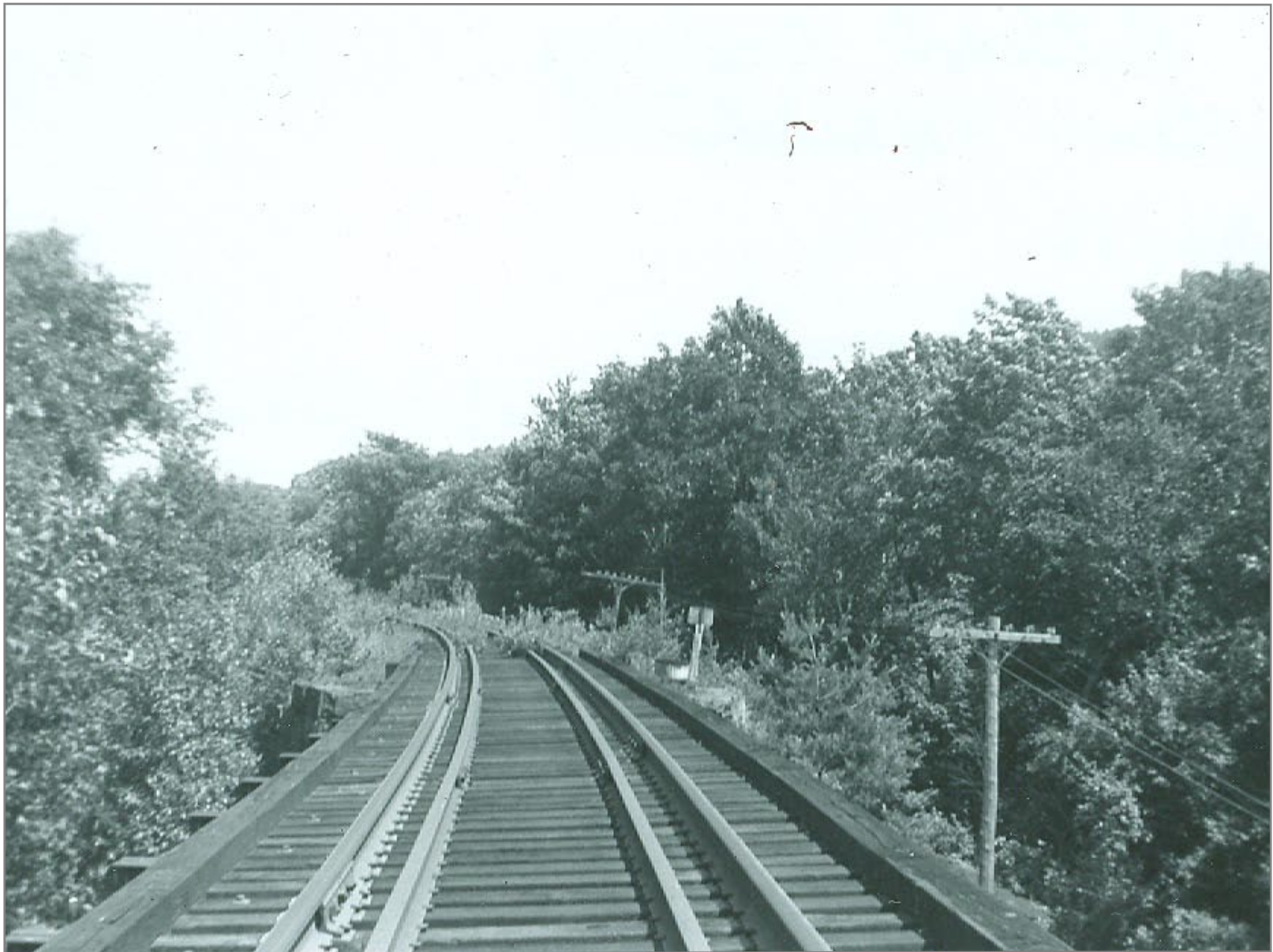
Southbound @ Bridge 136 Ludlow
