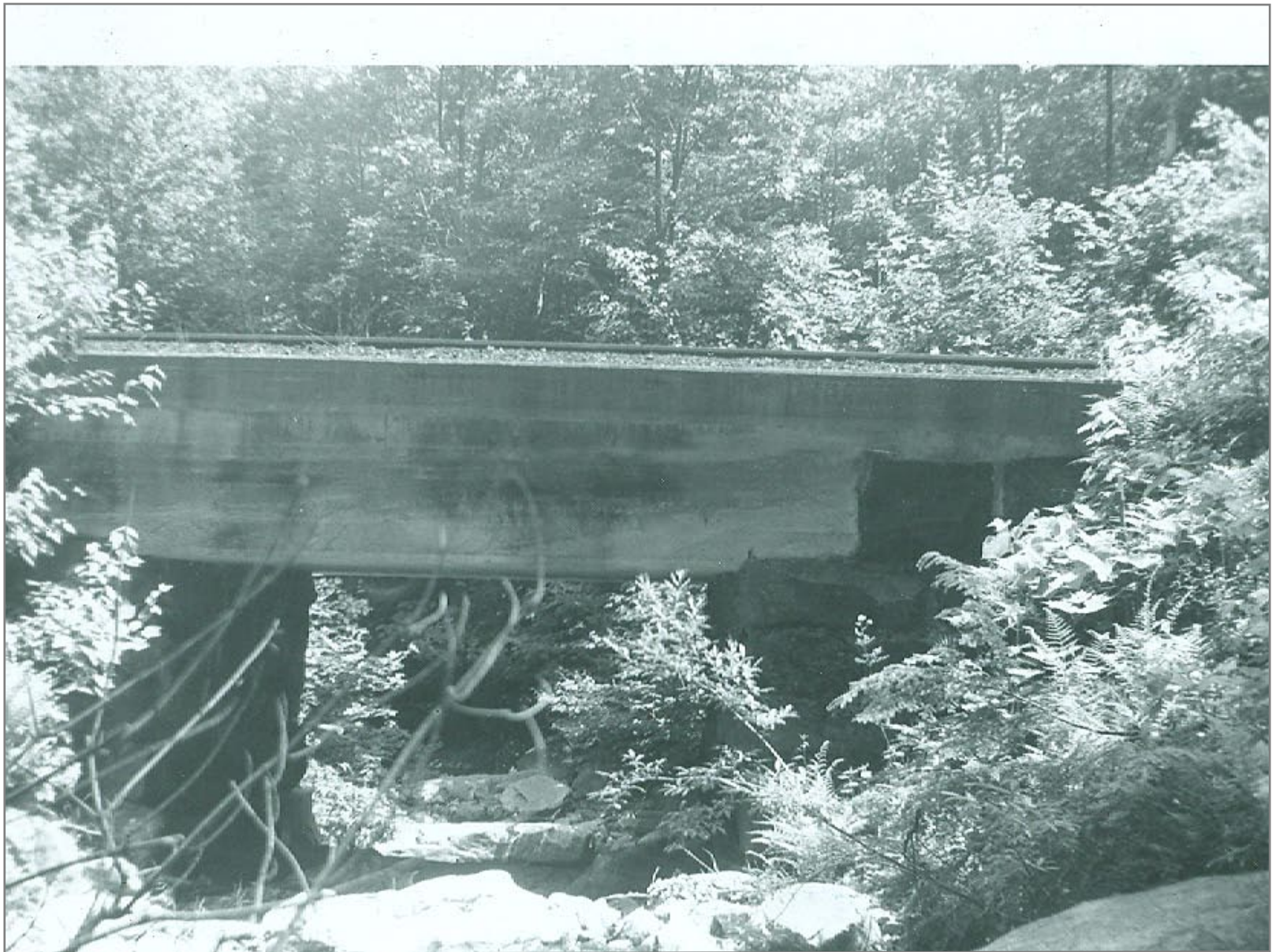
Bridge 139 north of Ludlow
