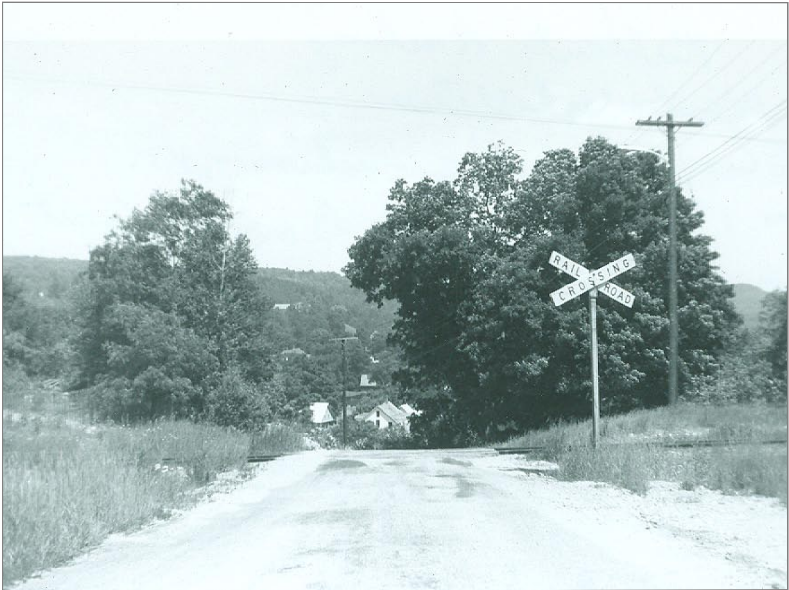
1st Crossing North of Ludlow Station
