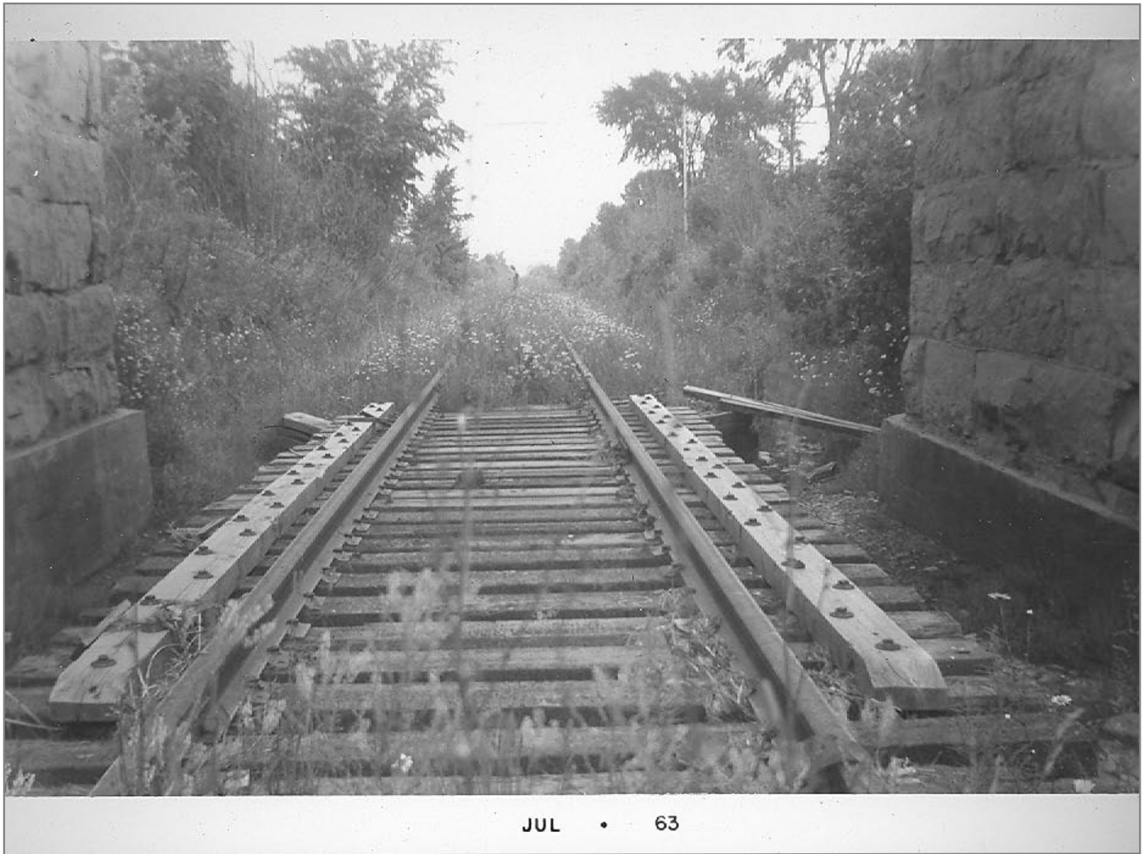
Grand Isle Northbound Bridge 274 6/29/63
