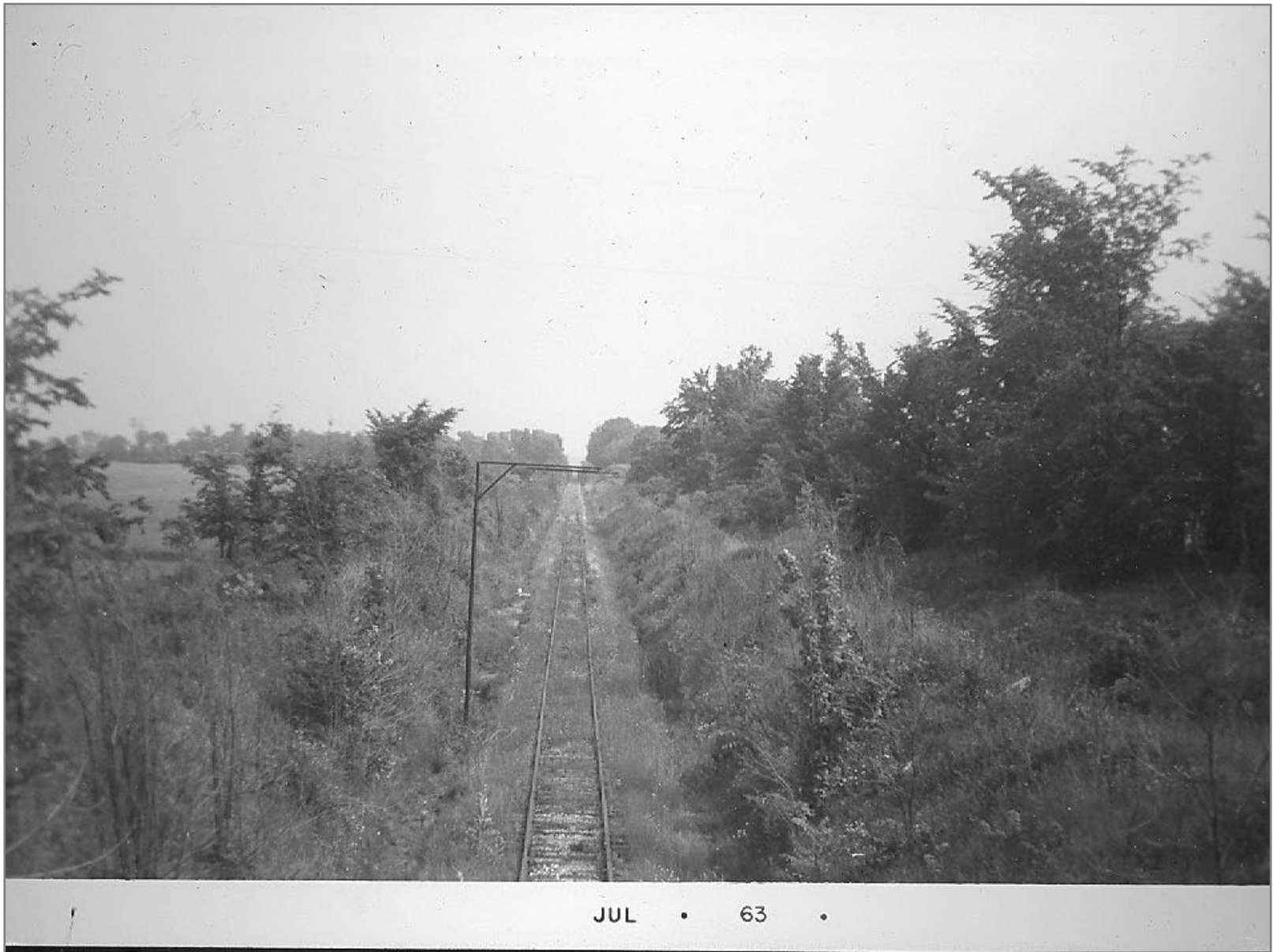
Northbound Bridge 273 Grand Isle 6/29/63
