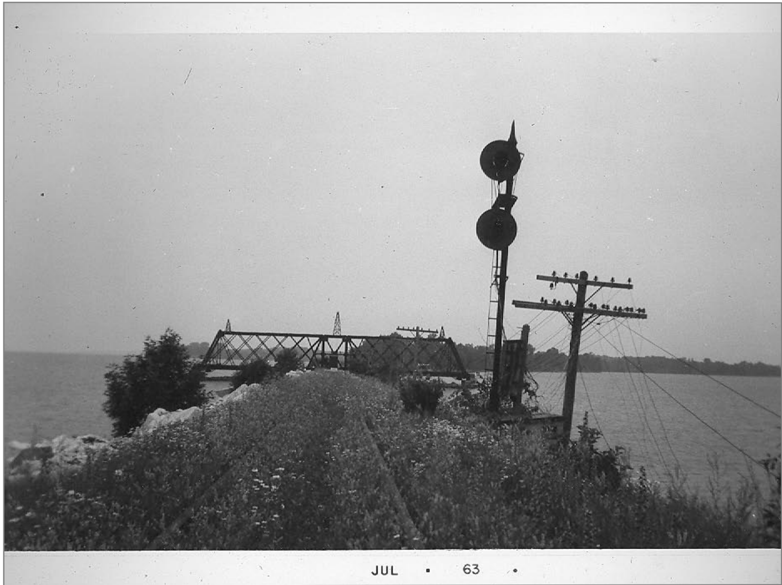
Bow Arrow Draw Bridge Northbound 3.5 miles north of Grand Isle 6/29/63
