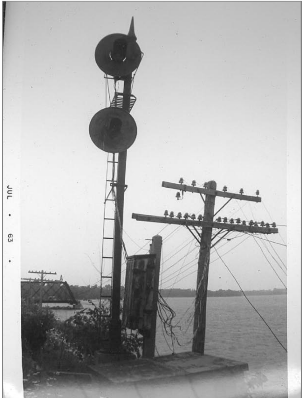
Northbound Bridge 275 in background
