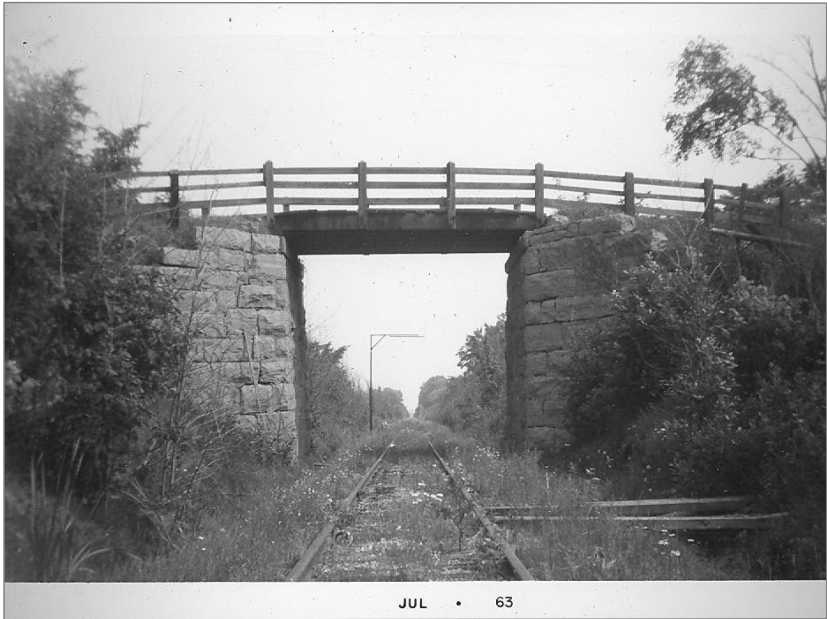
Northbound Bridge 273 1.5 miles north of Grand isle station 6/29/63
