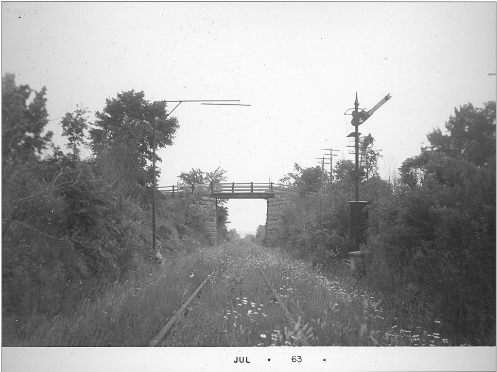
Northbound @ Signal 141.7 Approach Signal to Bow Arrow Draw Bridge - Bridge 274 2.5 miles north of Grand Isle 6/29/63
