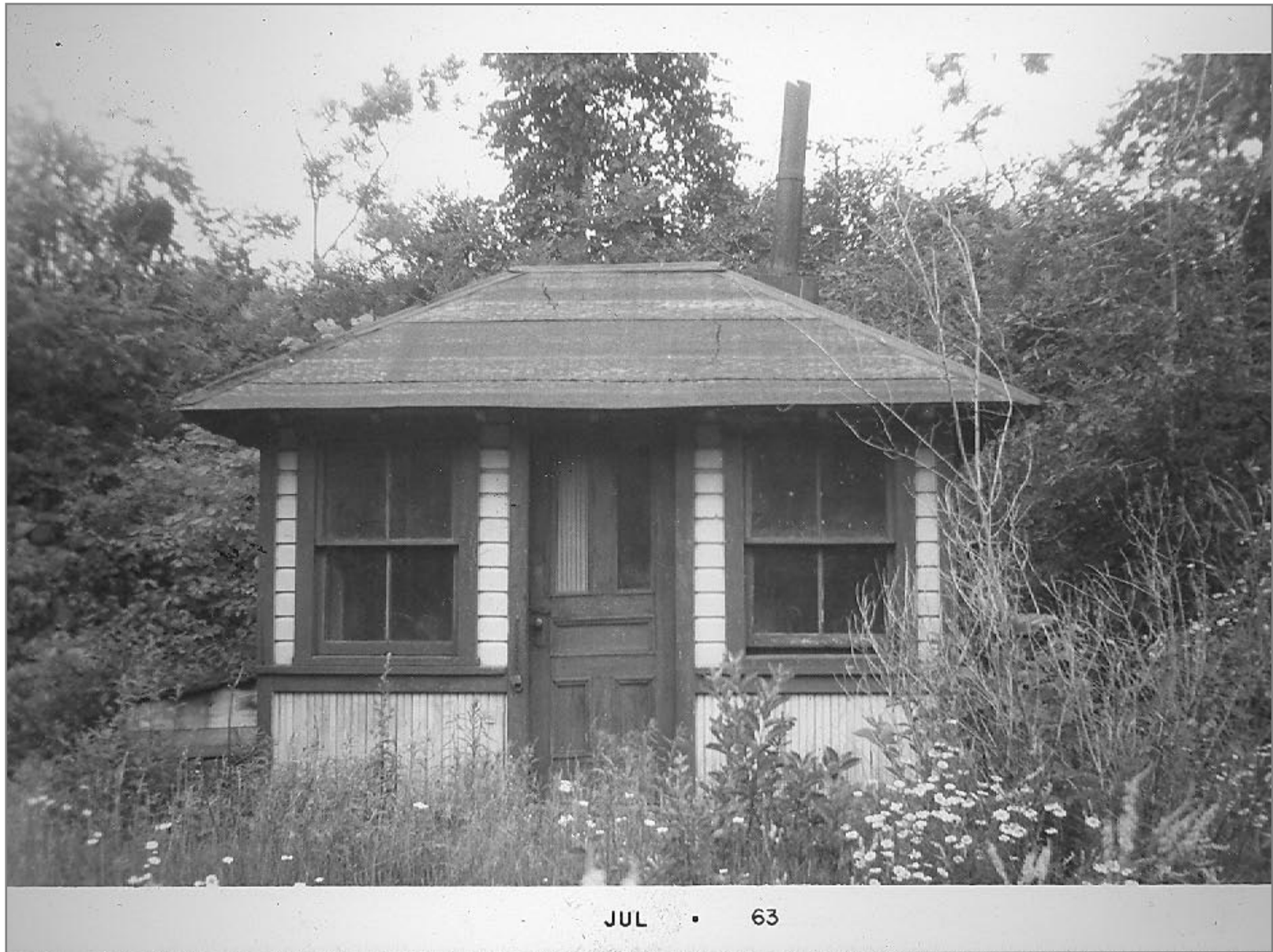
Section House left is north between bridges 273 and 274
