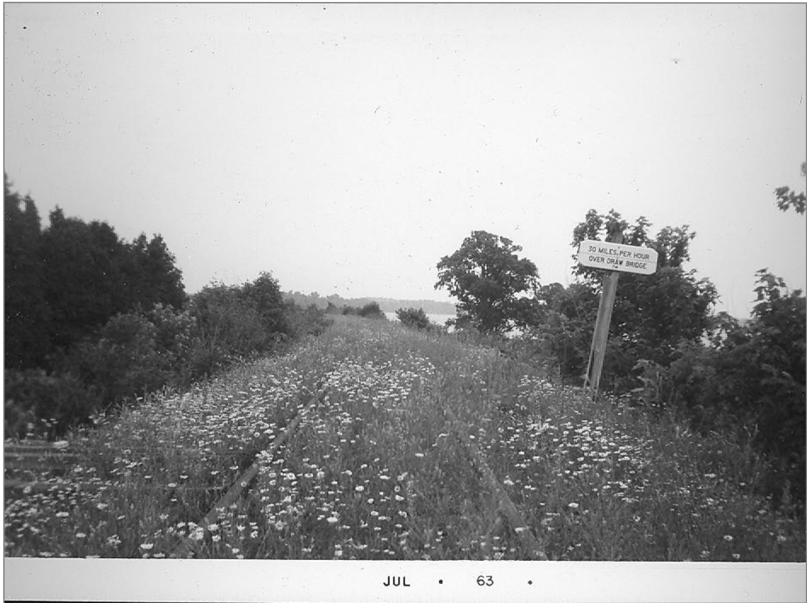
Northbound approaching Bow Arrow Draw Bridge 6/29/63
