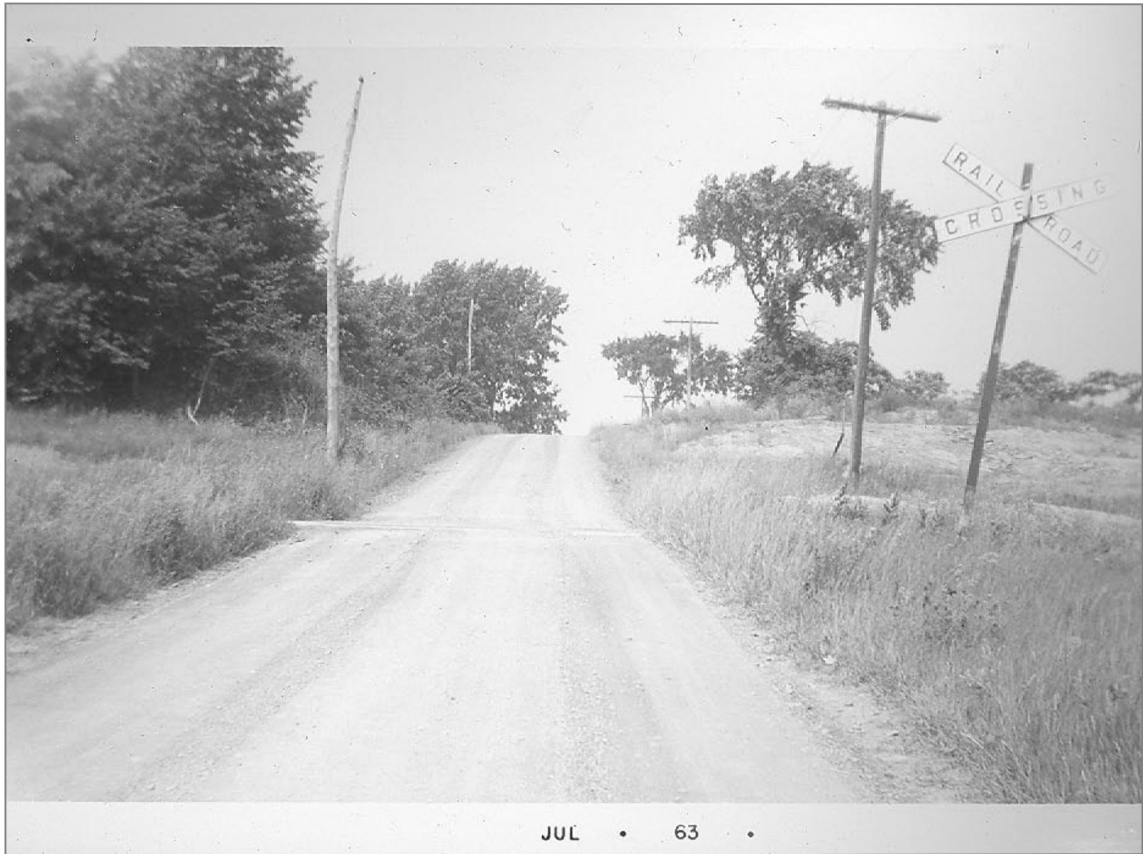
Road Crossing near Bow Arrow Draw bridge
