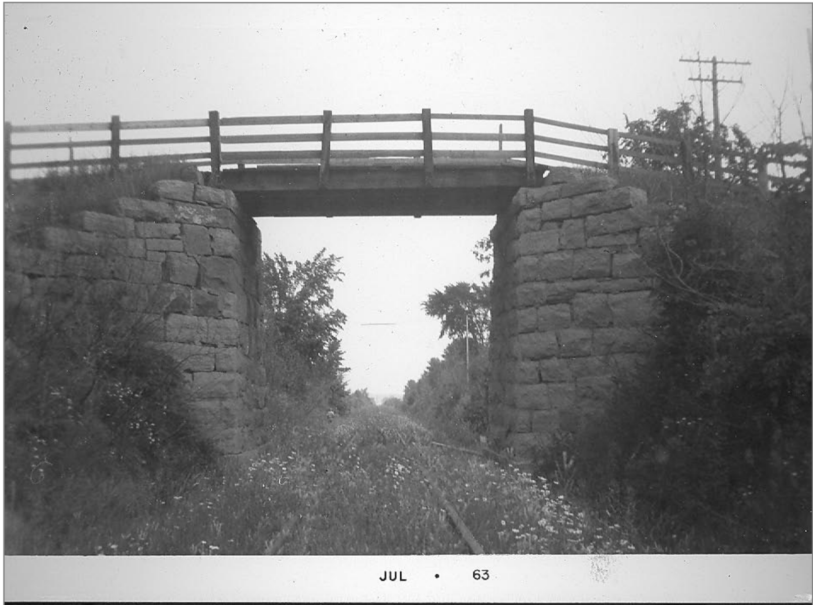
Grand Isle Northbound Bridge 274 6/29/63
