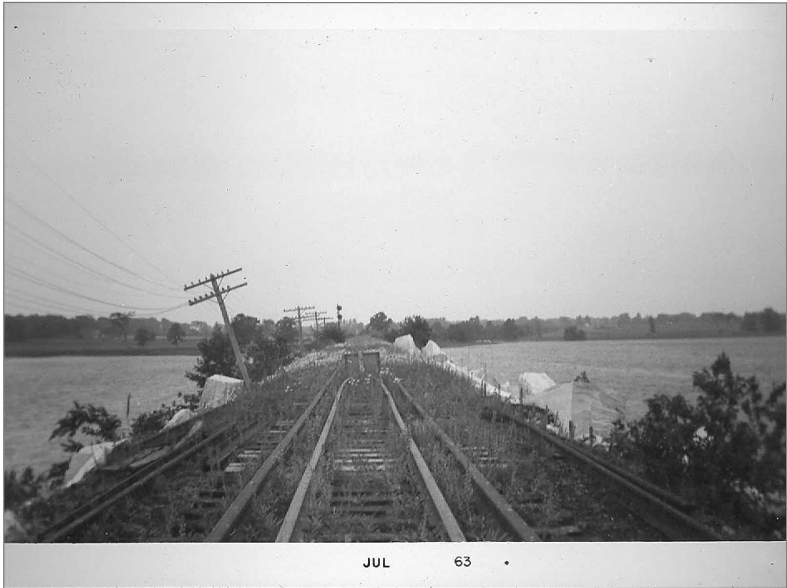
Southbound at Bow Arrow Bridge 6/30/63
