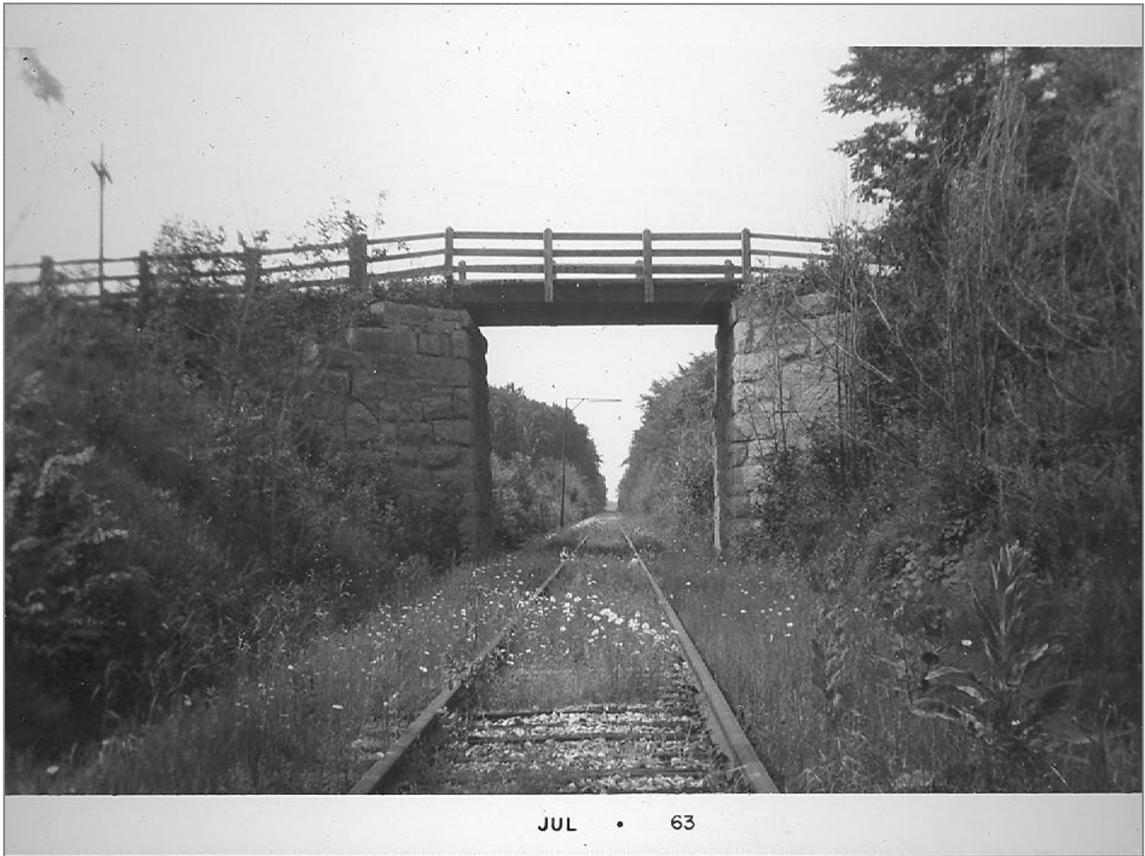
Grand Isle Bridge 273 Southbound
