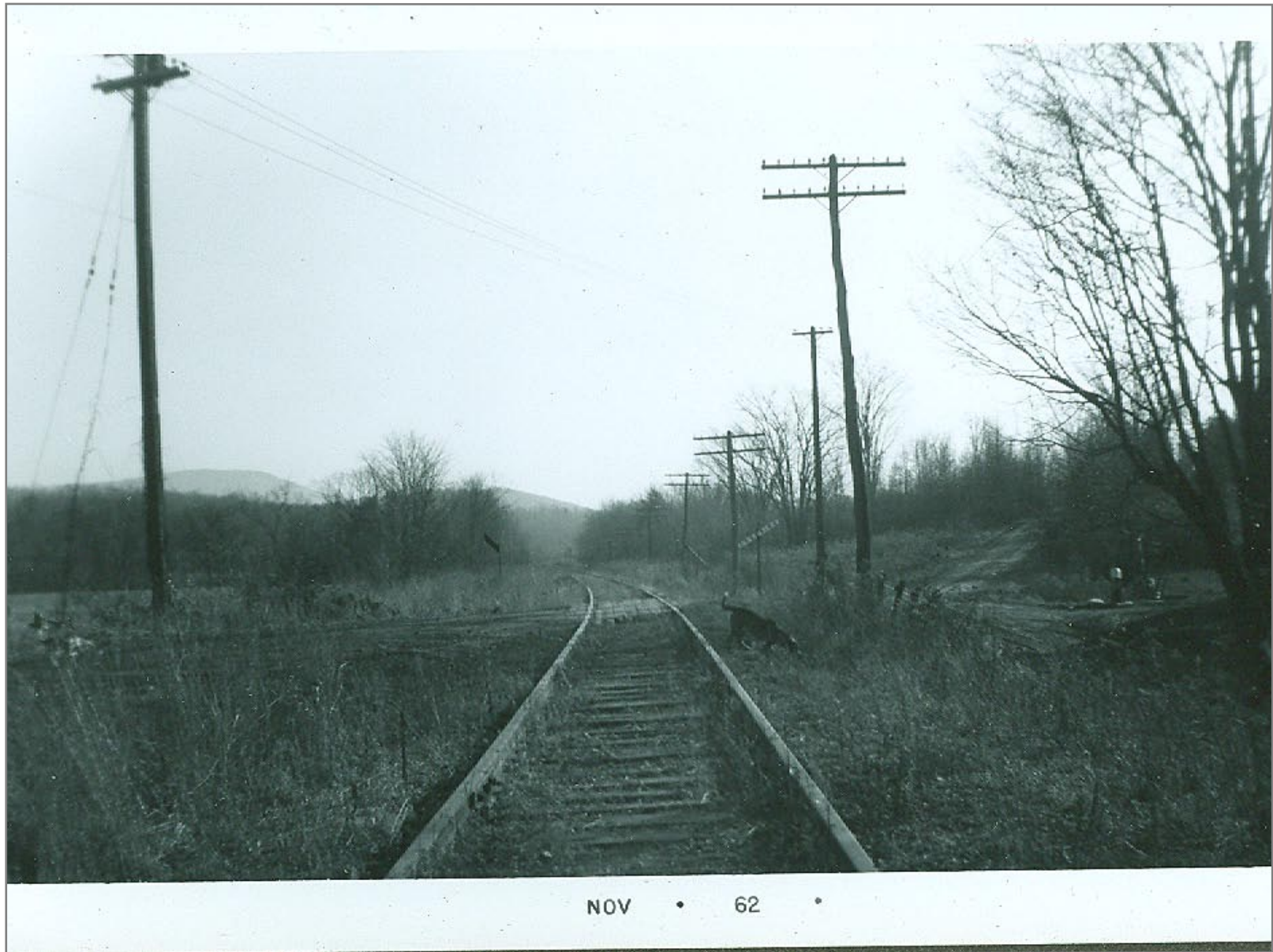
Southbound south of Brandon
