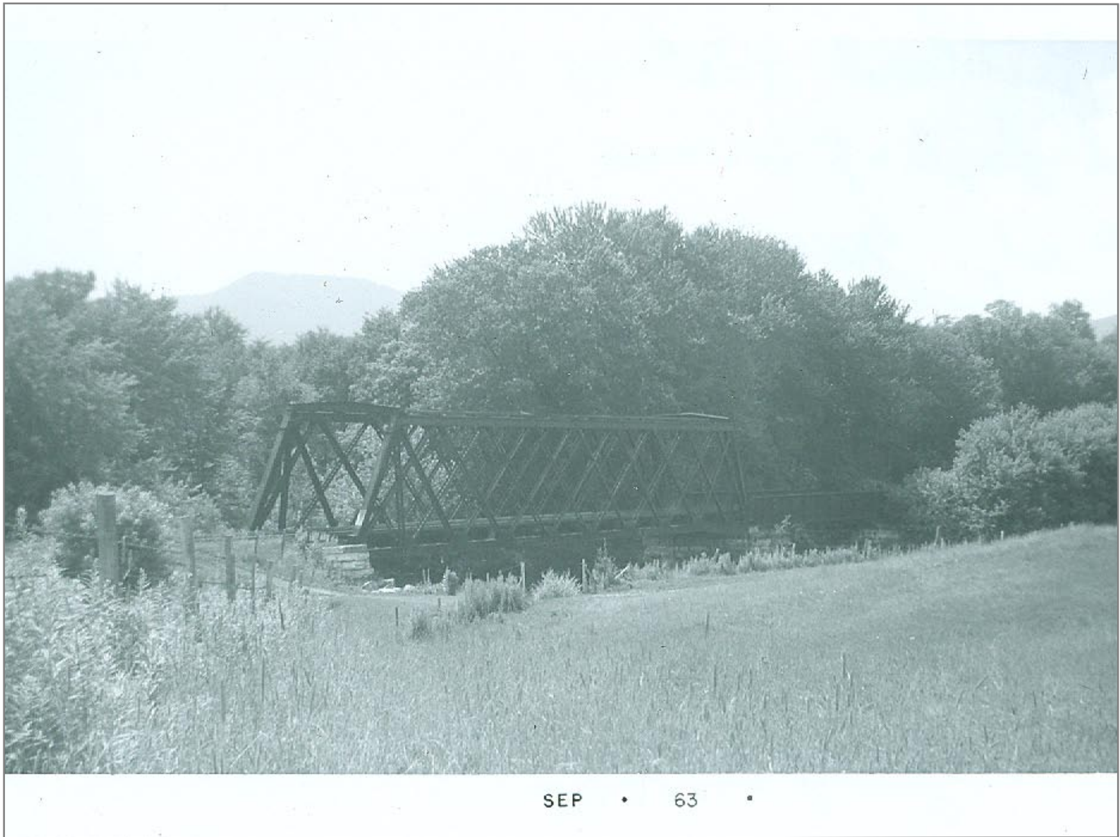
Looking West @ Bridge 219
