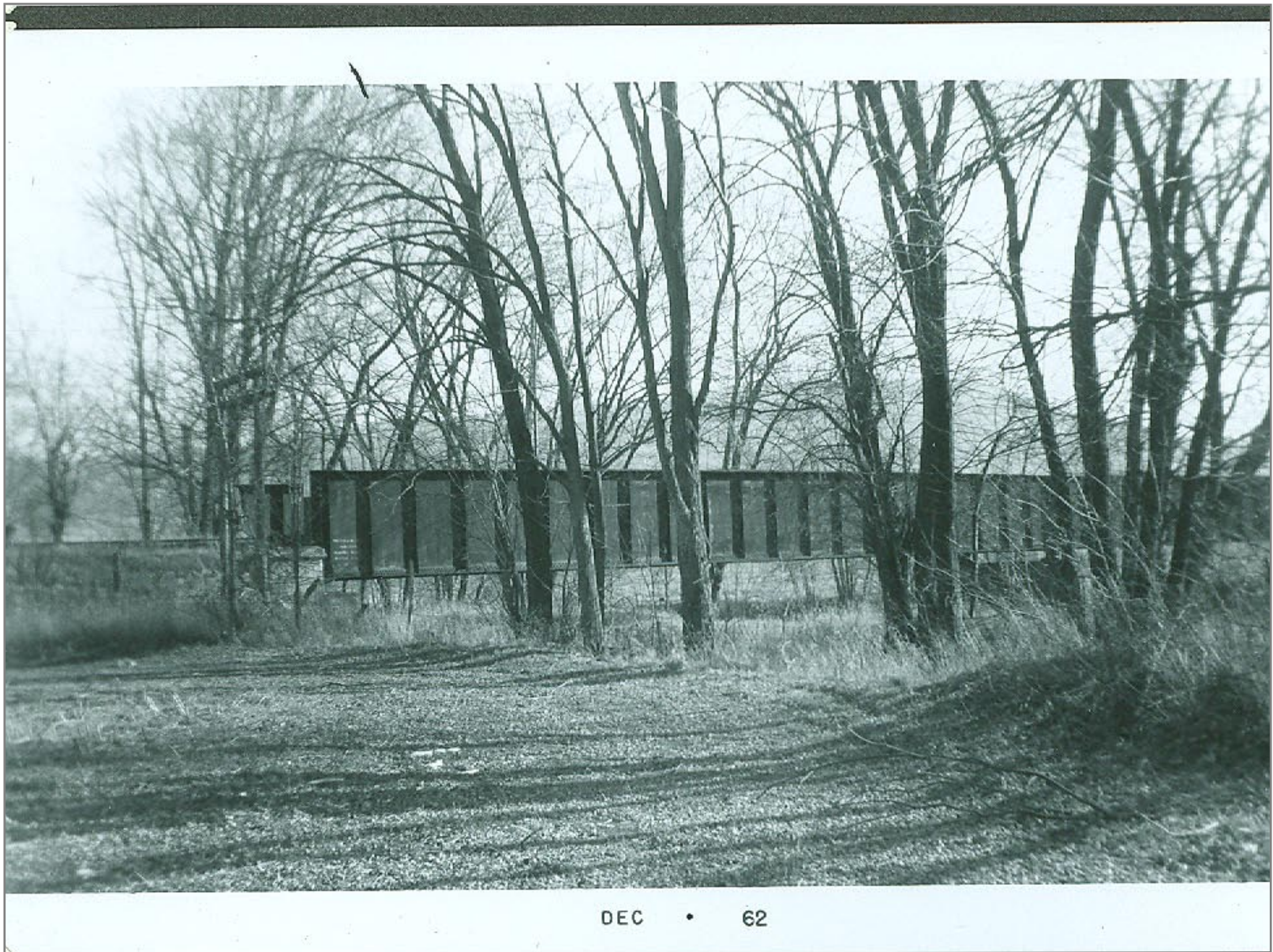
Bridge 220 Between Brandon and Florence
