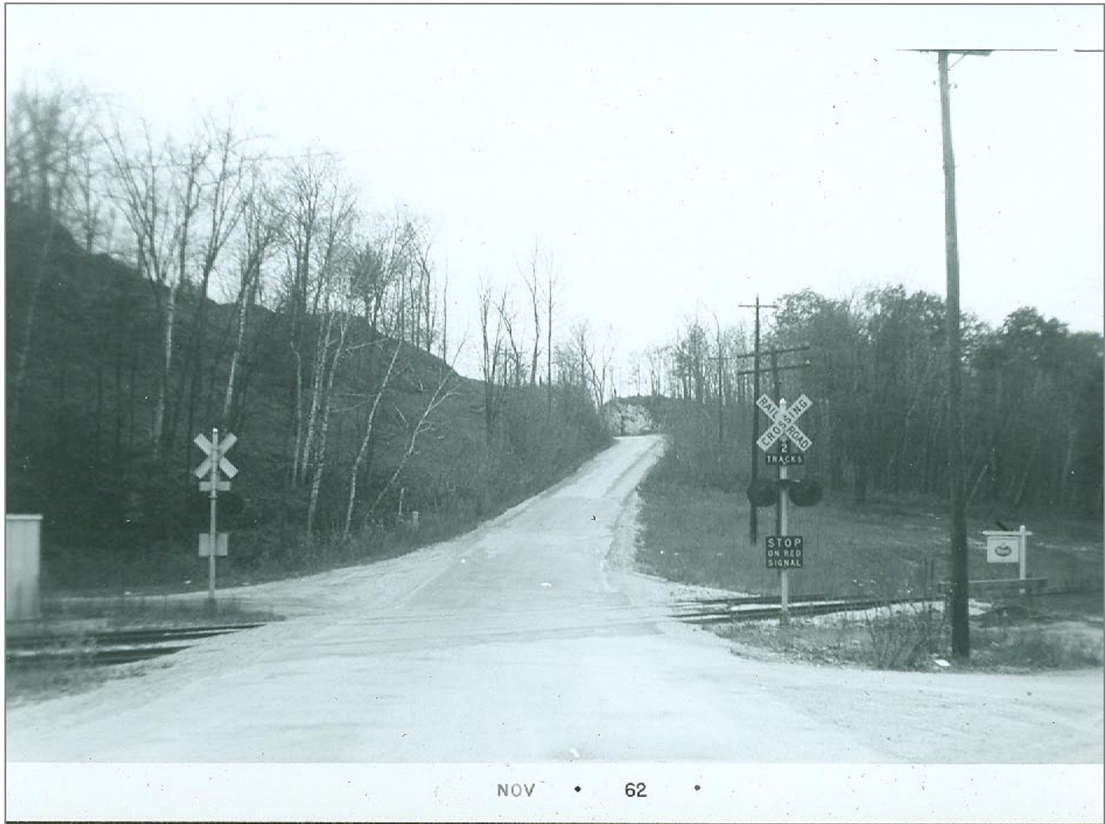
Florence looking west
