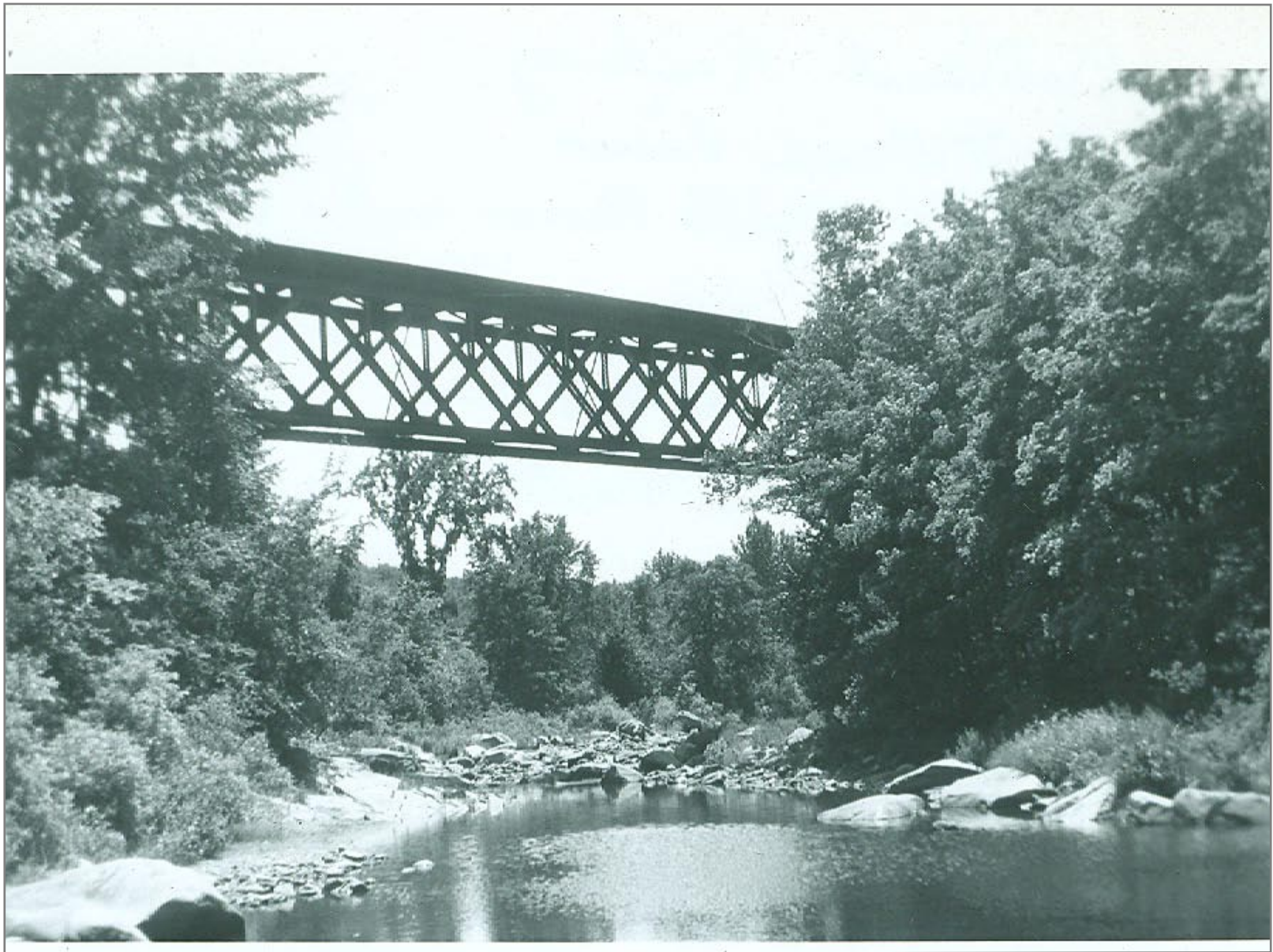
Bridge 145 Looking South
