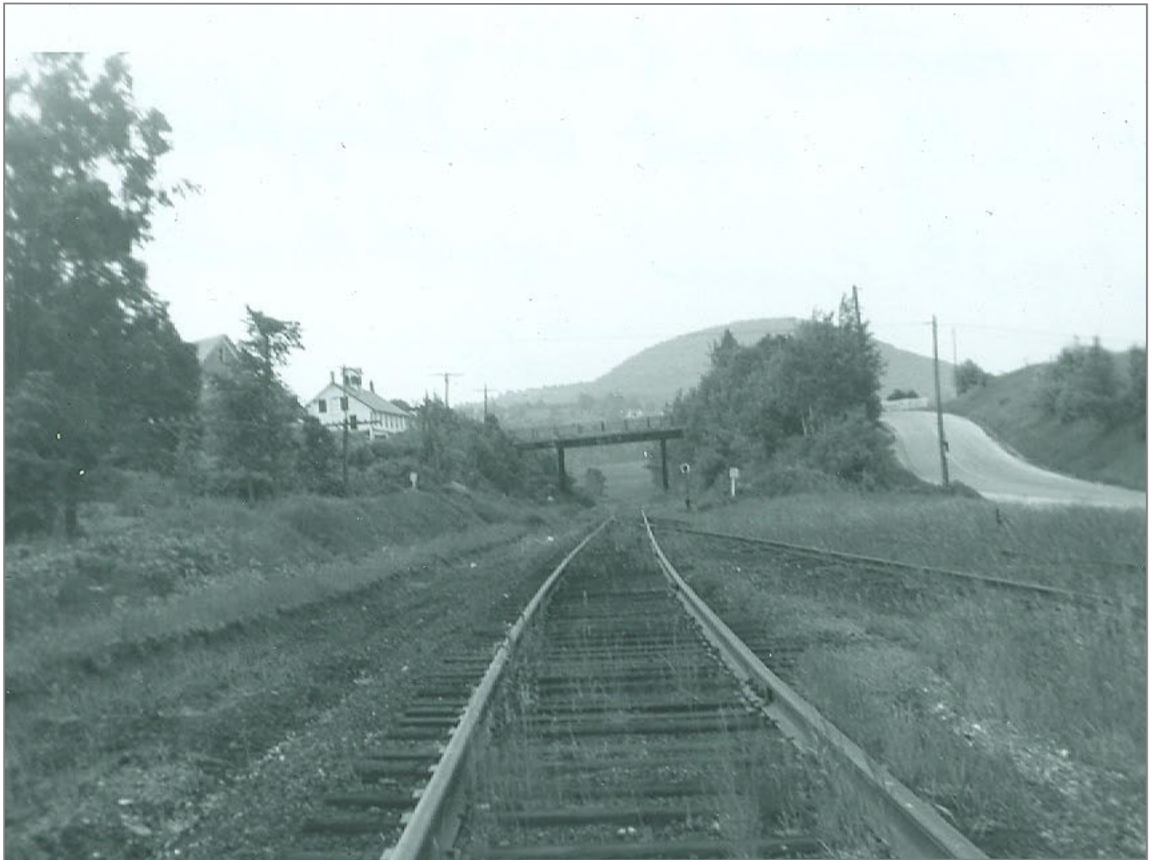
Northbound at East Wallingford - Station site on left
