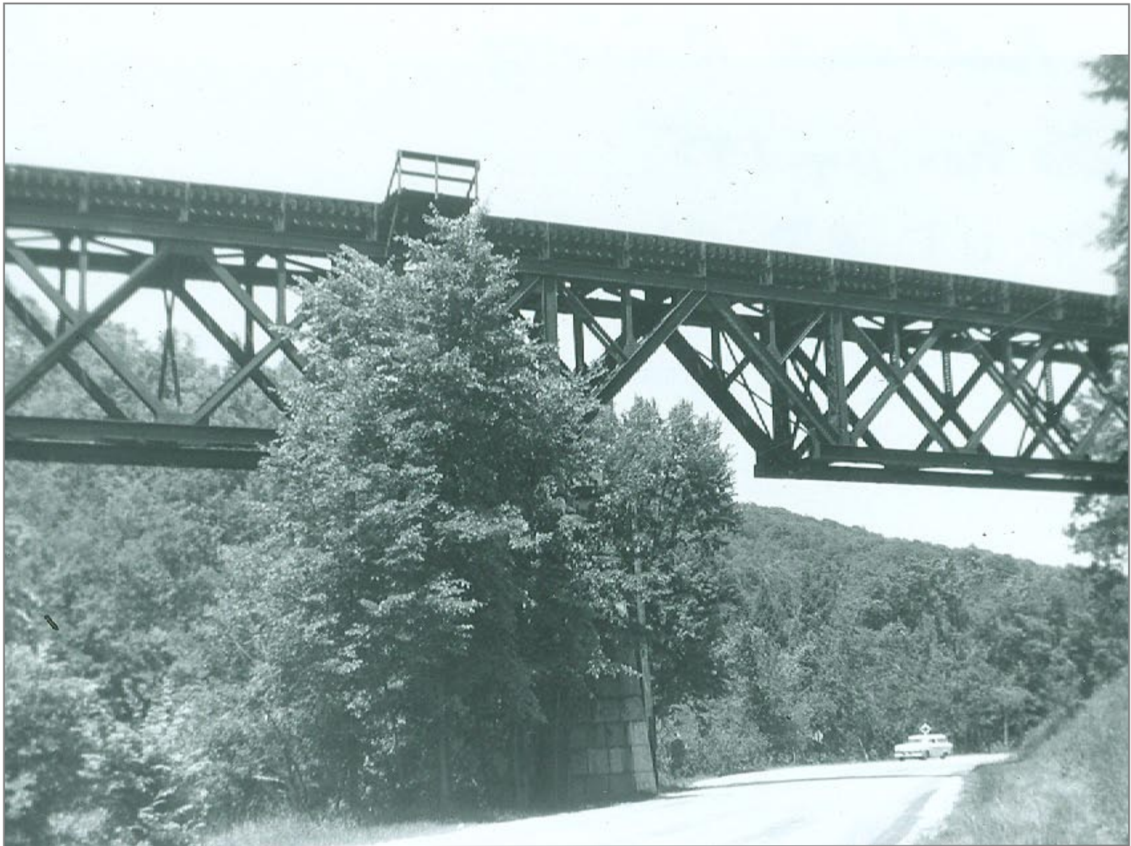
West View at bridge 145
