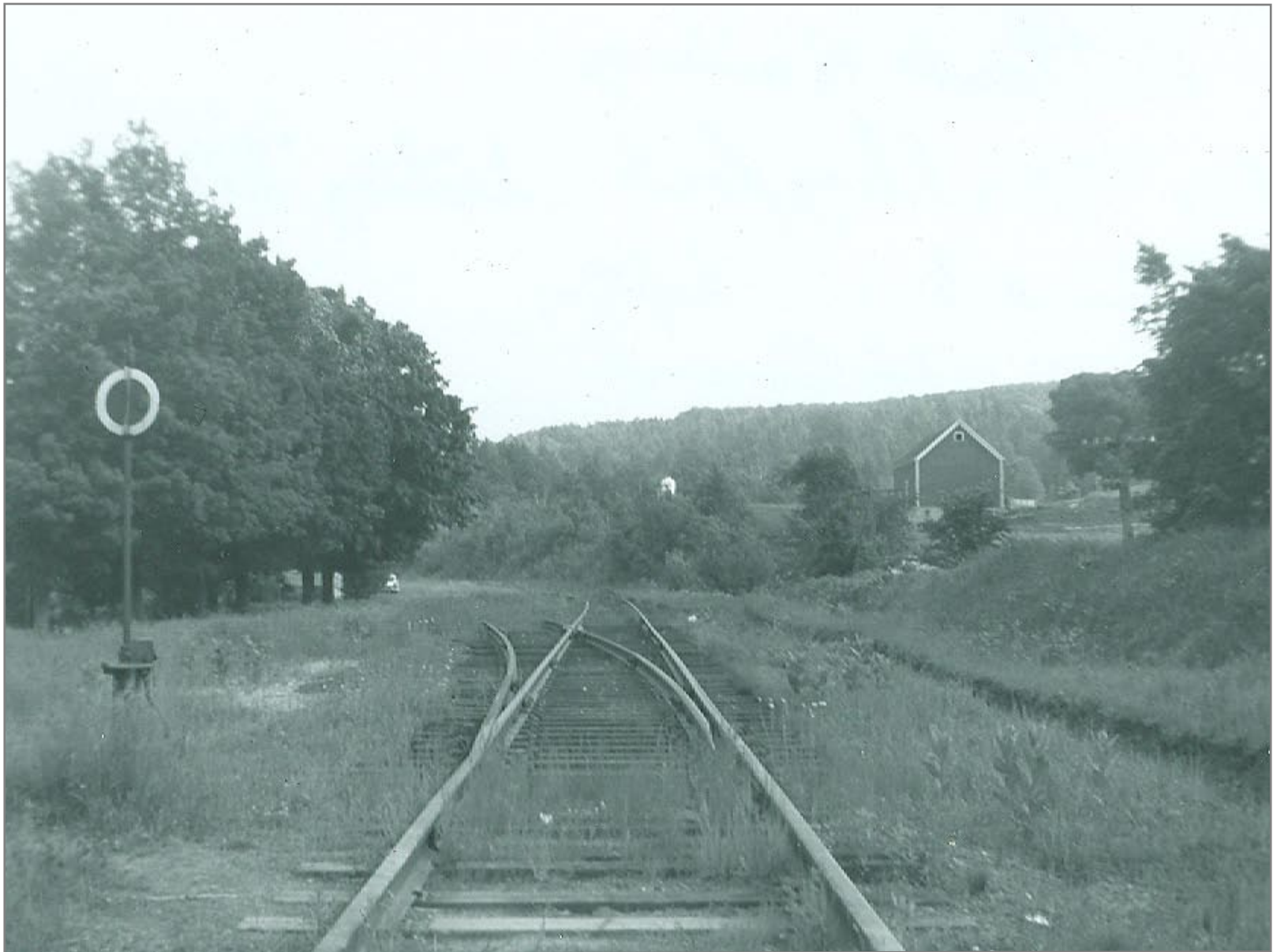
Southbound at East Wallingford - Station site on left
