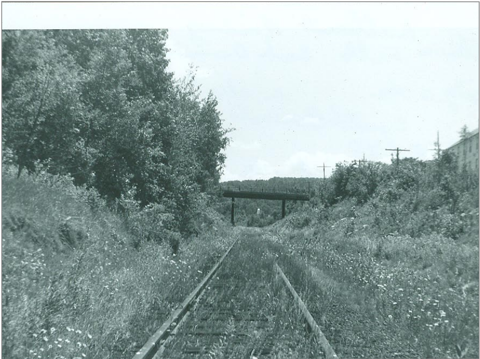
Southbound @ East Wallingford - Route 140 Bridge in distance
