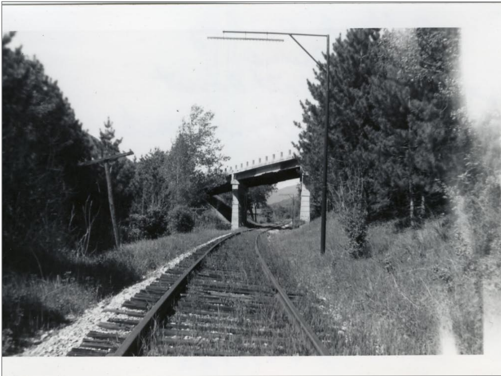
Route 7 Bridge Northbound 2nd Bridge North of East Dorset 5/26/1962
