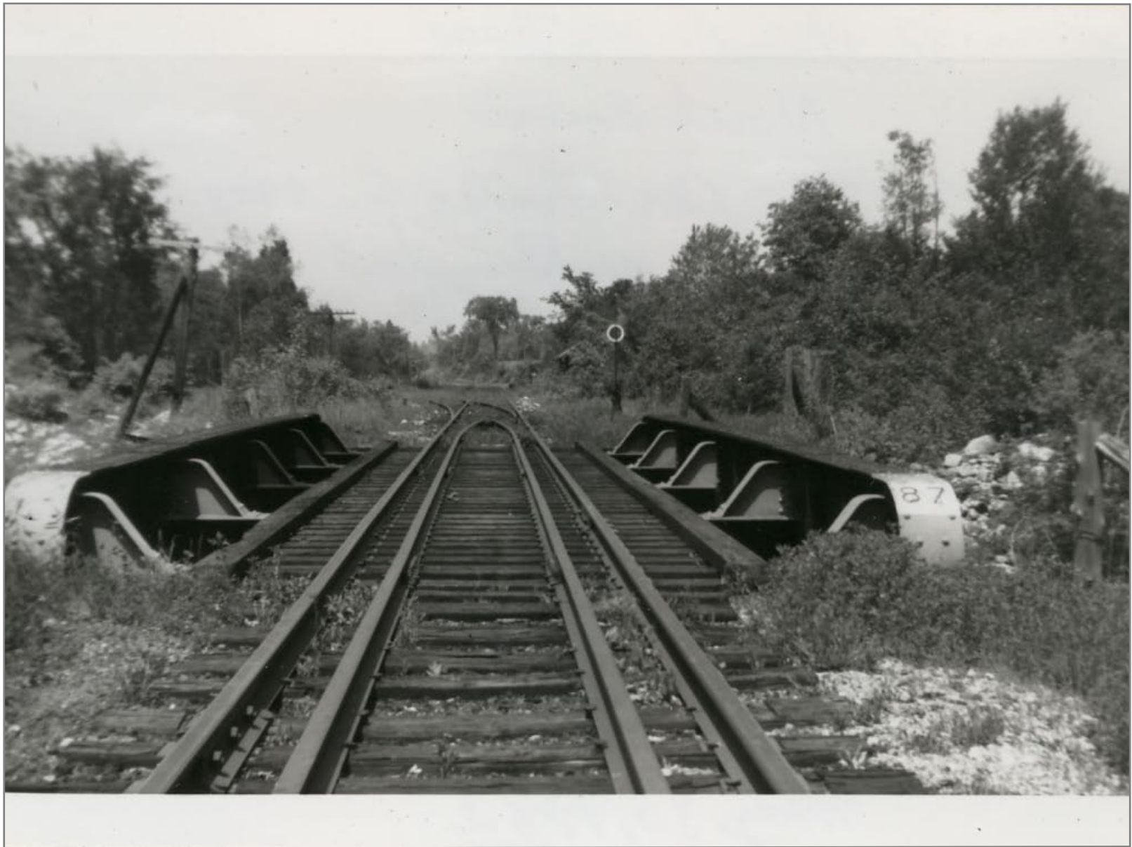
Bridge 87 Northbound American Bridge Co. 1903 5/30/1962
