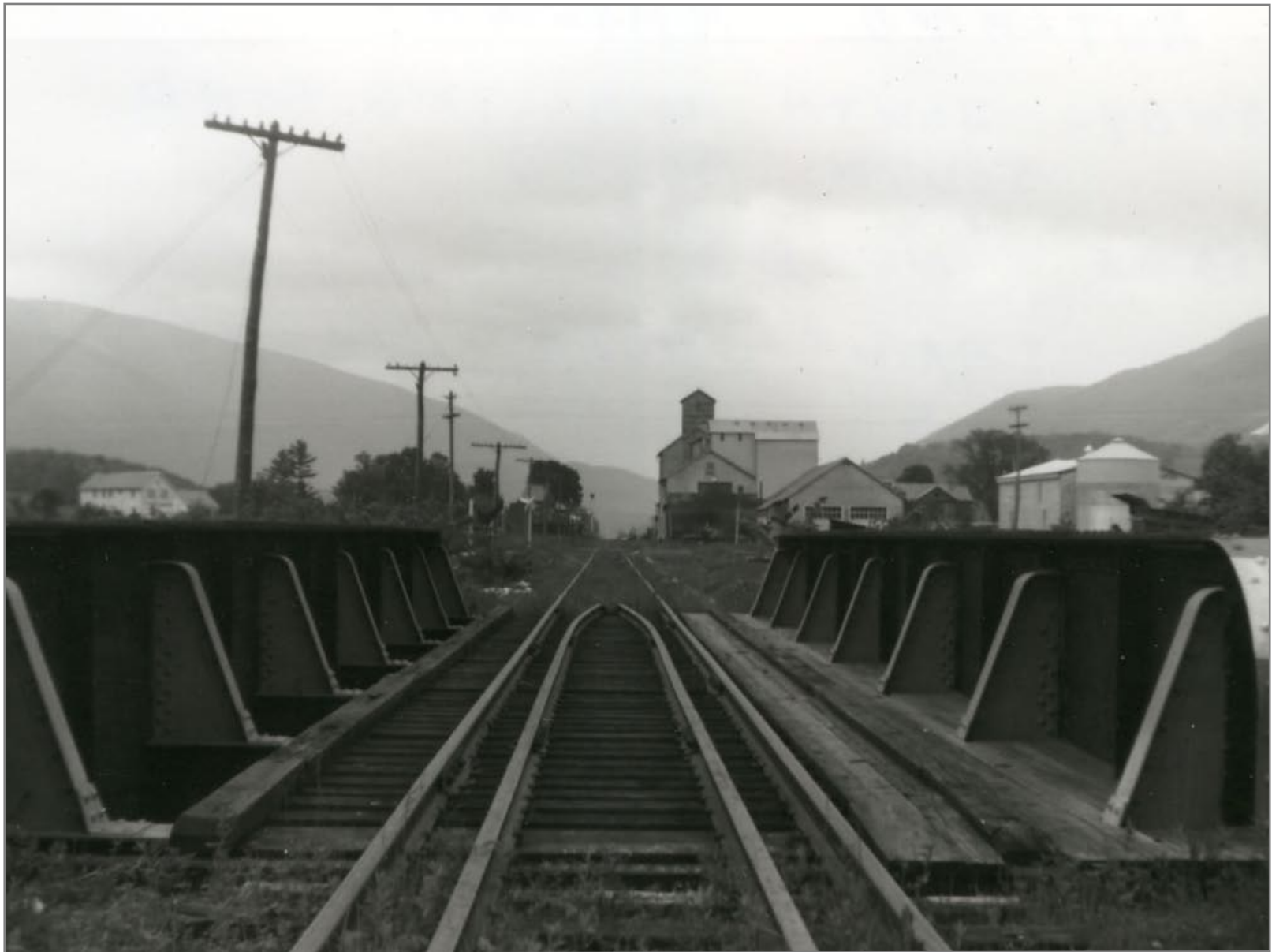
Soouthbound Thru Bridge No. 83
