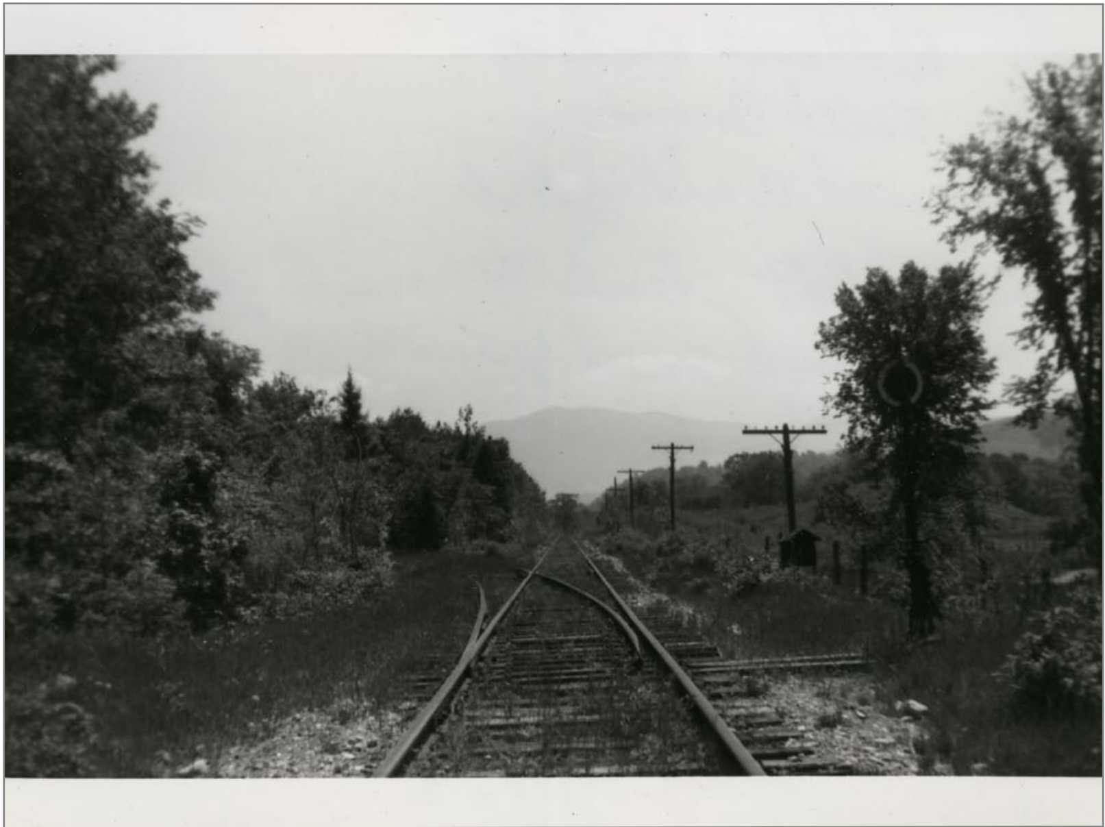
Southbound - Siding to Left Leads to Gravel Pit South of South Wallingford 5/30/1962
