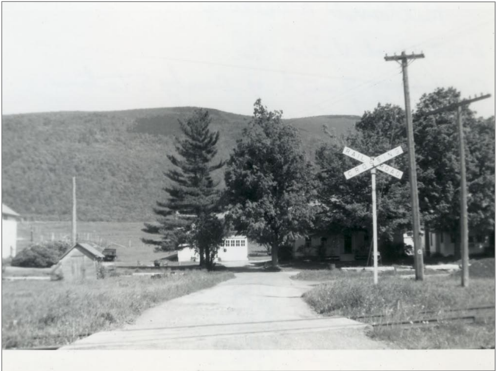
East View of Crossing Just South of Danby Station 5/27/1962
