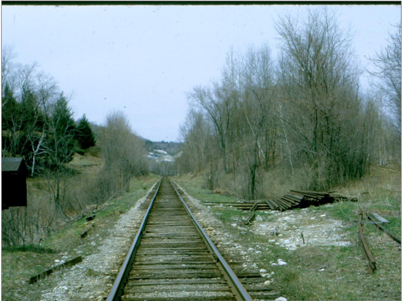
Former Siding into Stafford Pit
