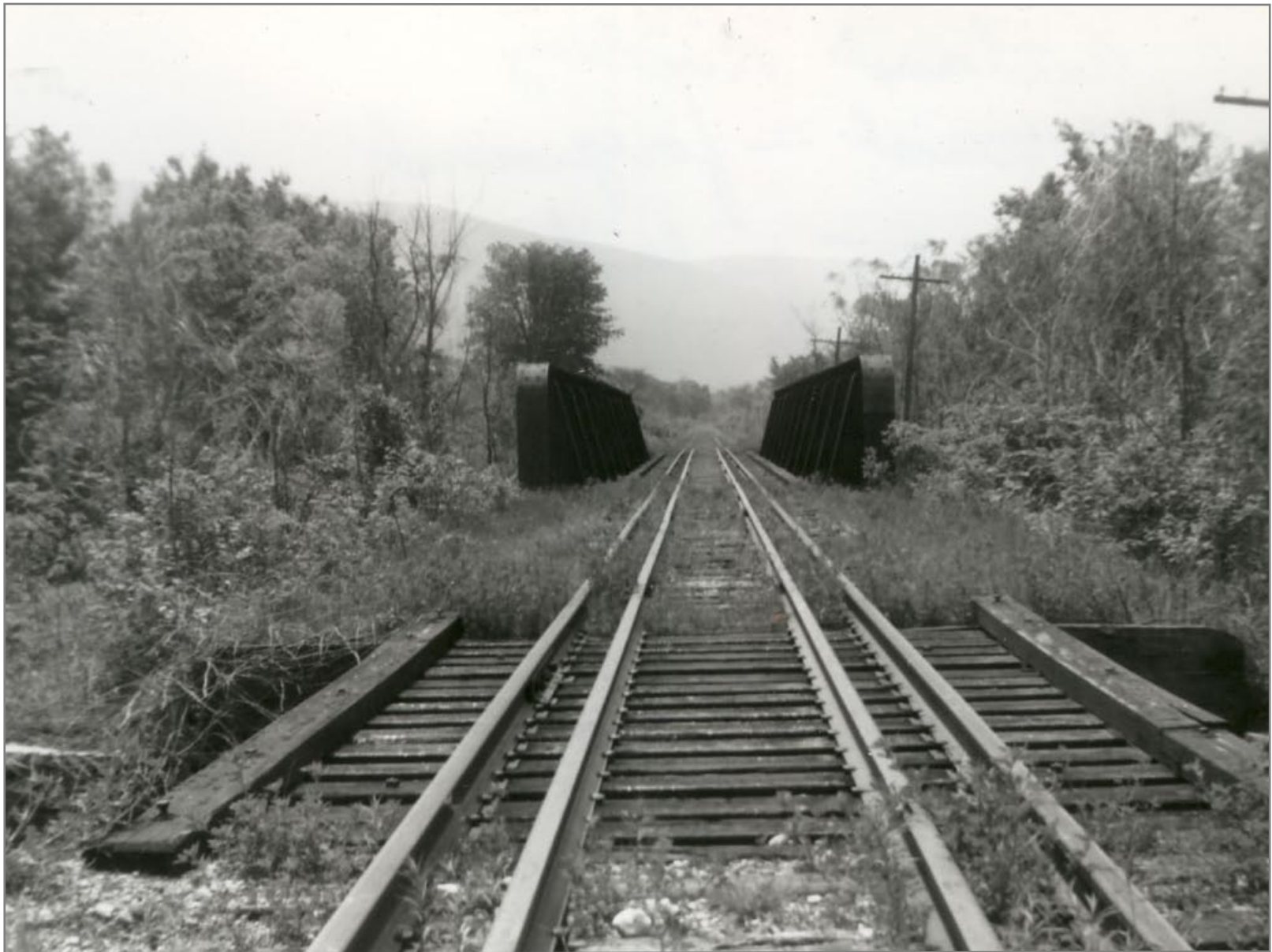
Southbound @ Bridge 85 5/30/1962 Bridge 86 in foreground
