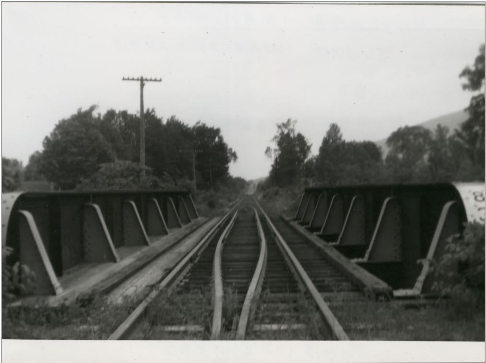
Norhtbound thru Bridge #83 5/26/1962
