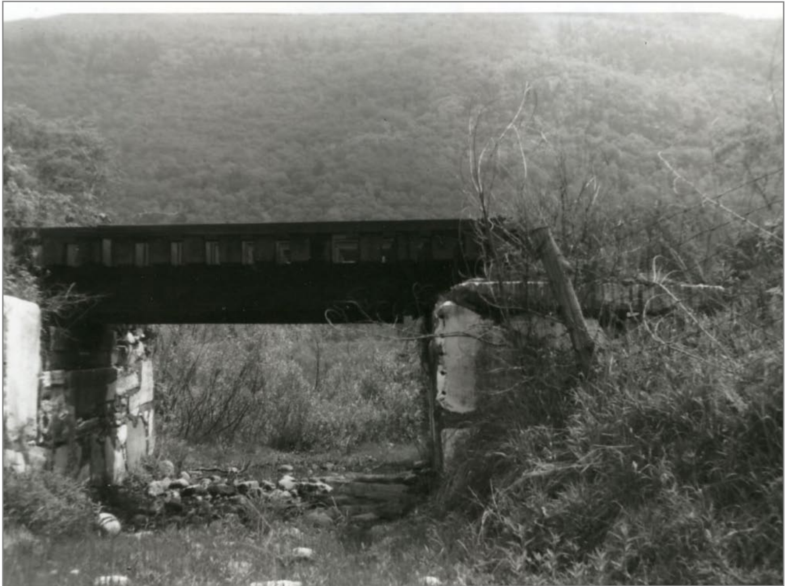
Cattle Underpass Bridge 86
