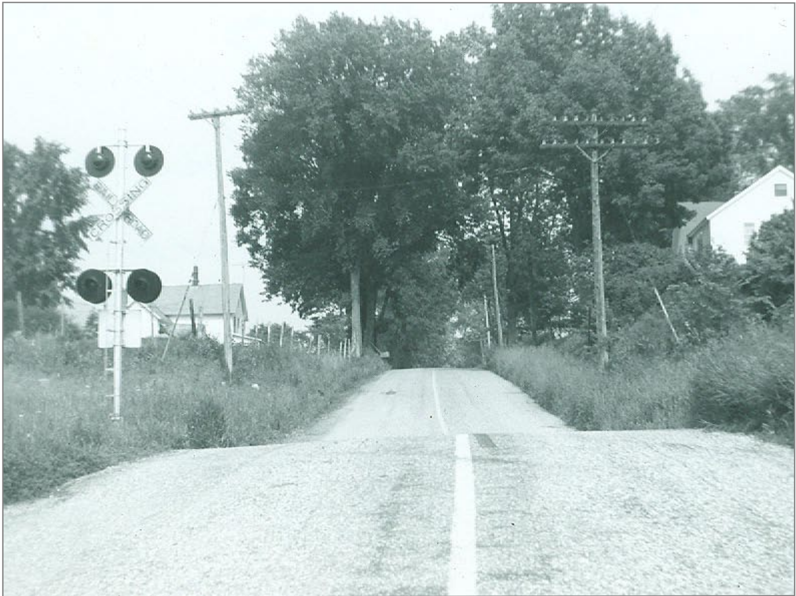
Road Crossing south of Horth Clarendon Station
