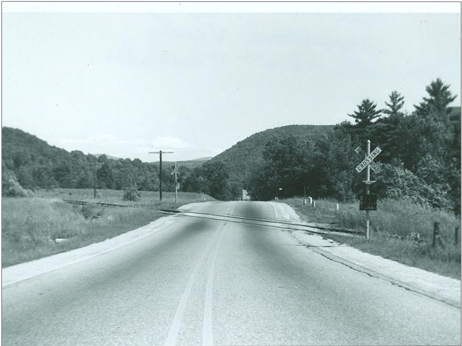
Route 103 Crossing-East View
