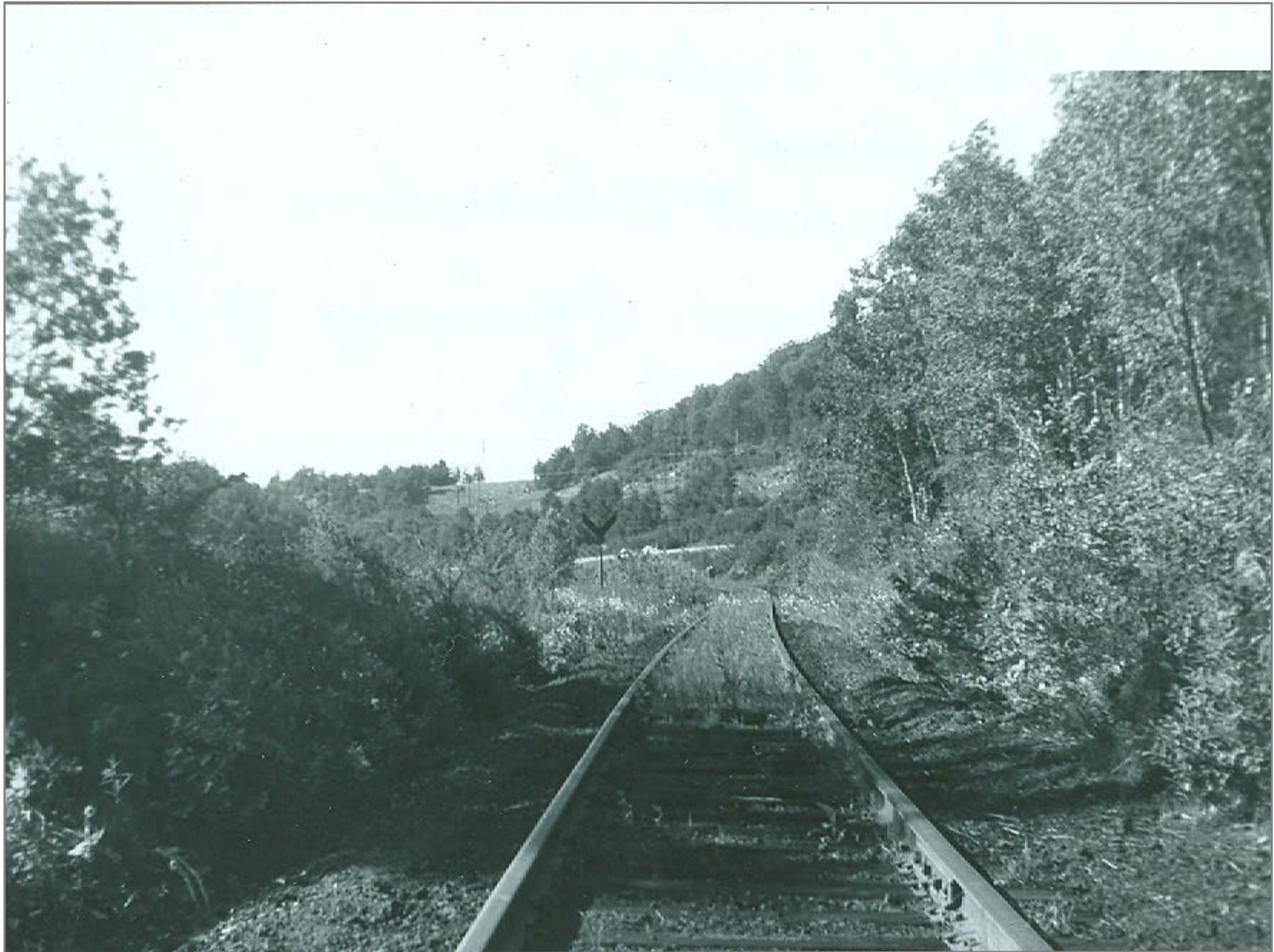
Northbound - Route 103 in distance
