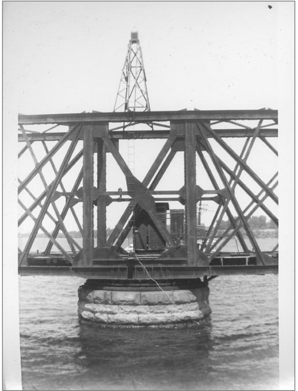
Bridge 270 Northbound BLT American Bridge Co. 1906
