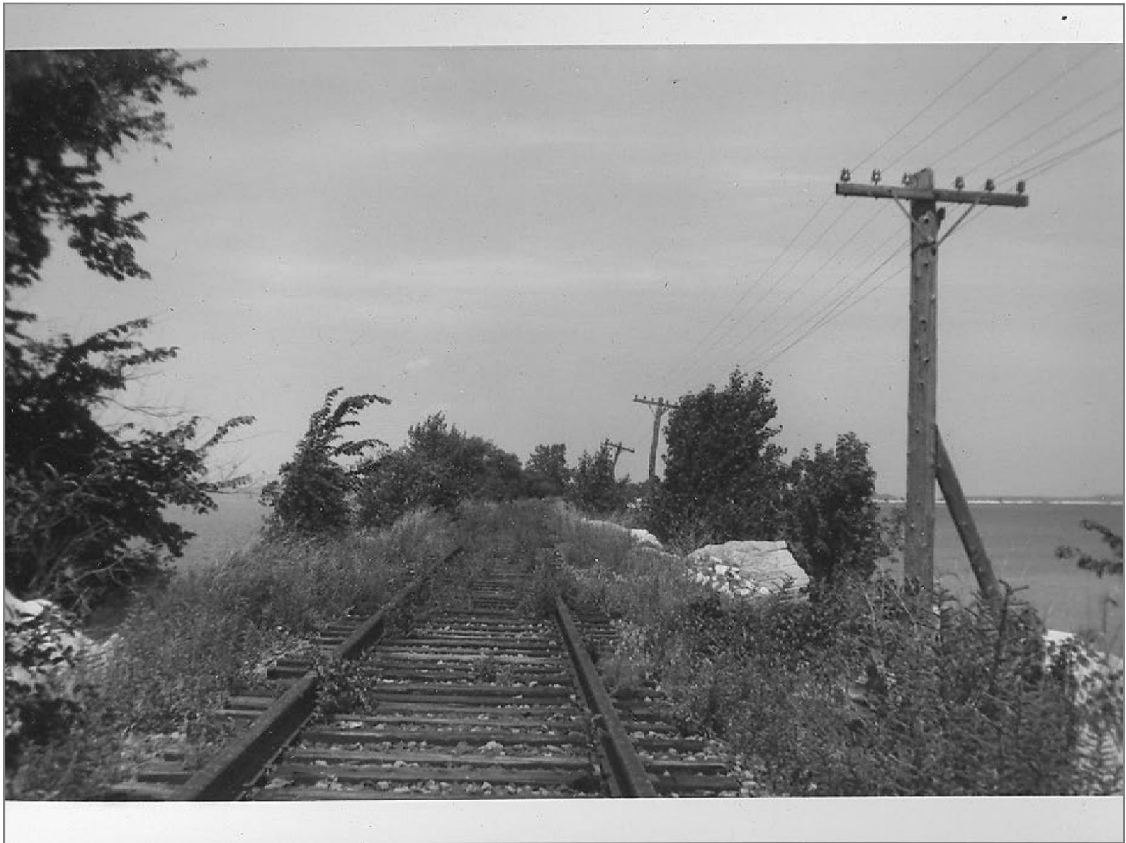
Northbound on Colchester Fill 8/10/62
