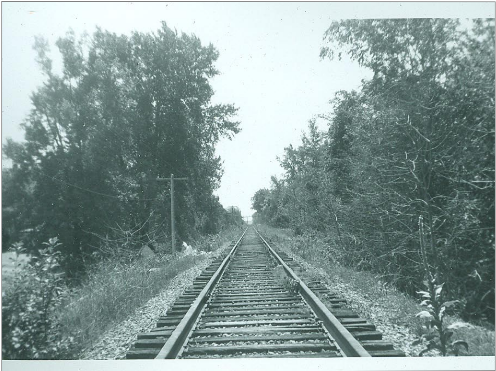
Southbound Bridge 268 in Distance 8/10/62
