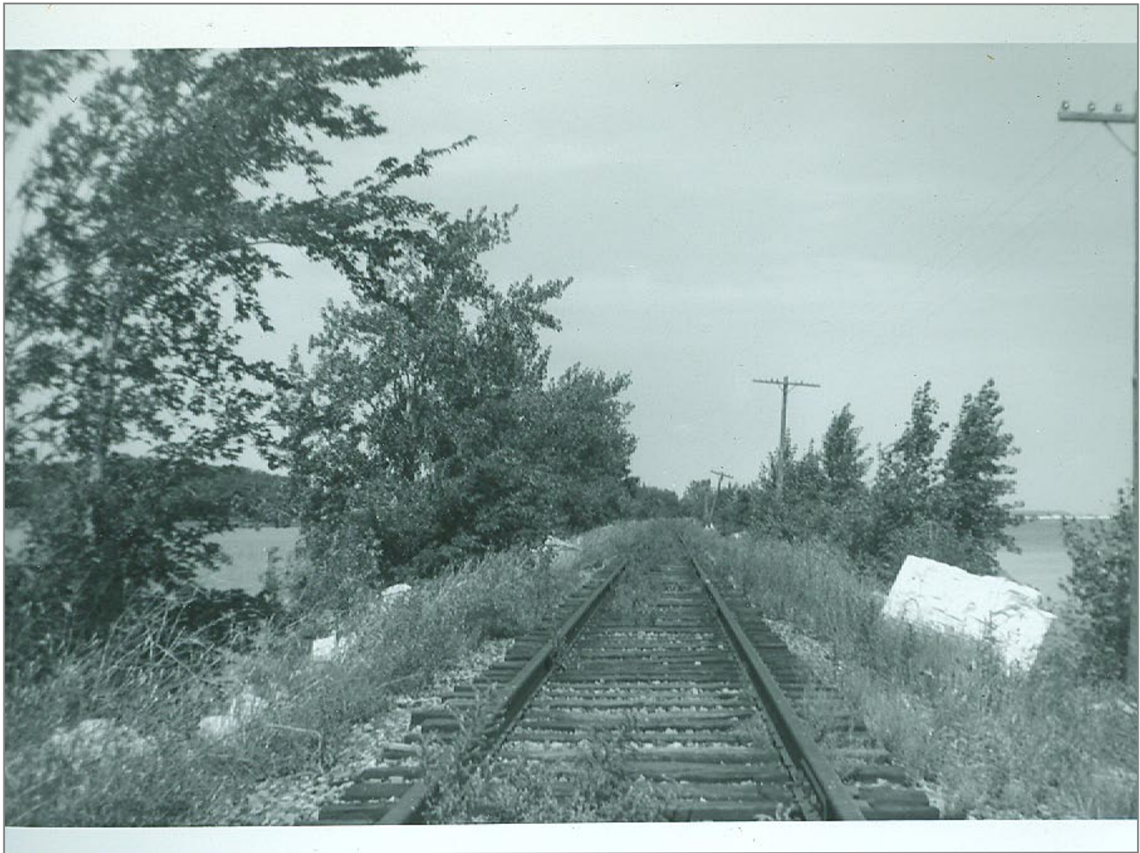
Northbound onto Colchester Causeway 8/10/62
