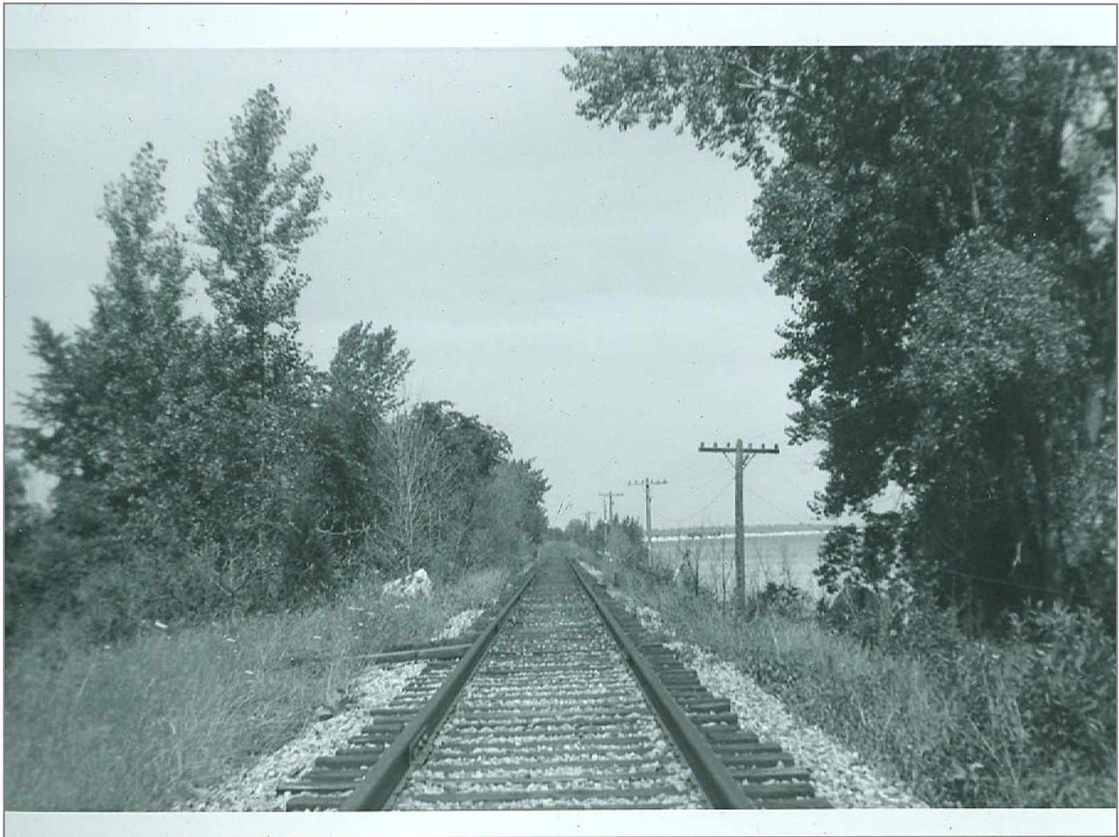
Northbound onto Colchester Causeway 8/10/62
