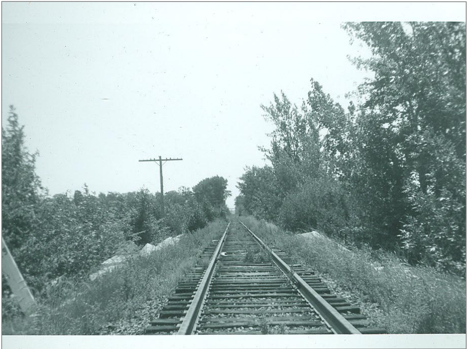
Colchester Point Southbound Bridge 268 in Background 8/10/62
