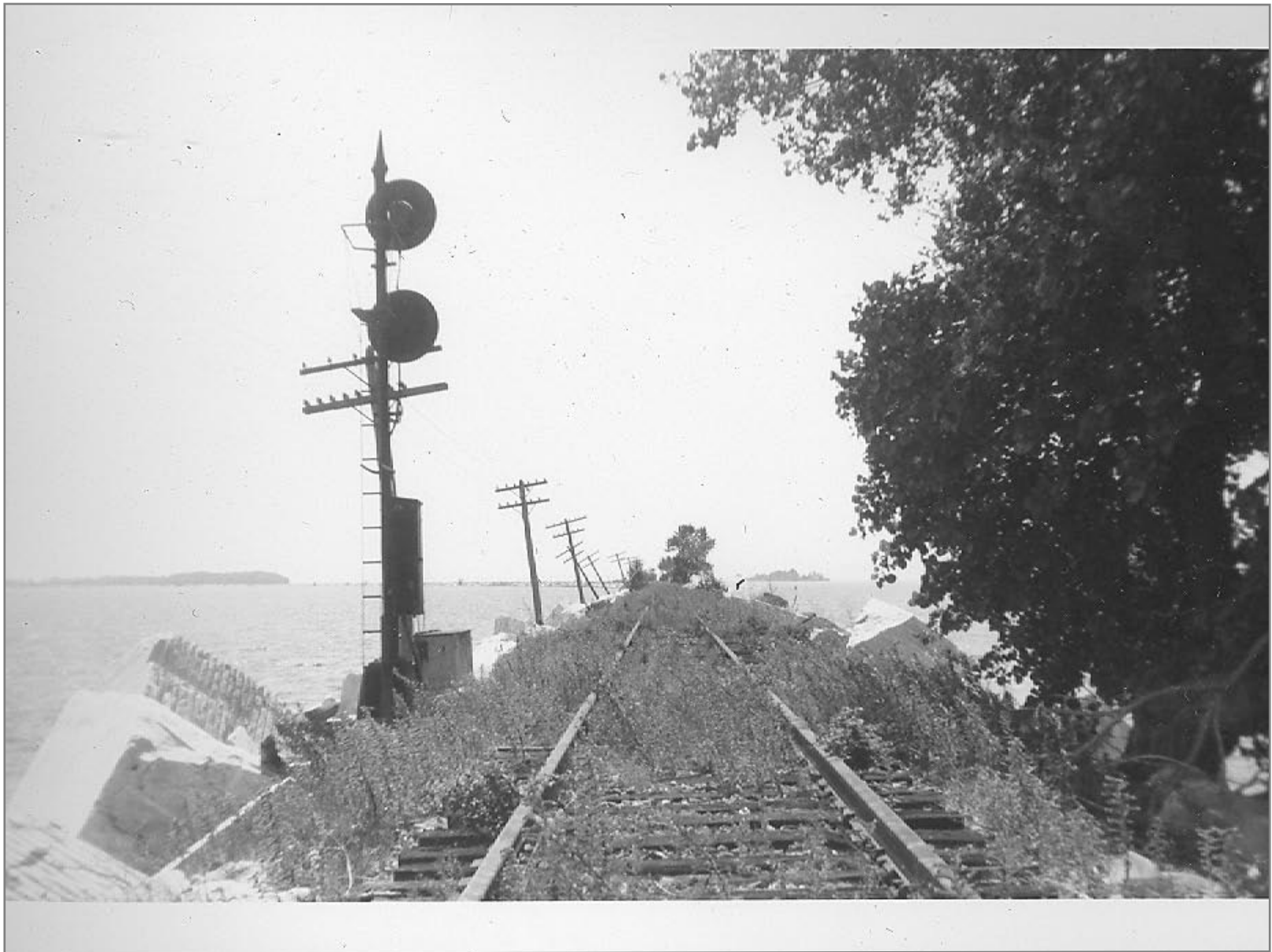
Stop signals at South End of drawbridge Southbound 8/10/62
