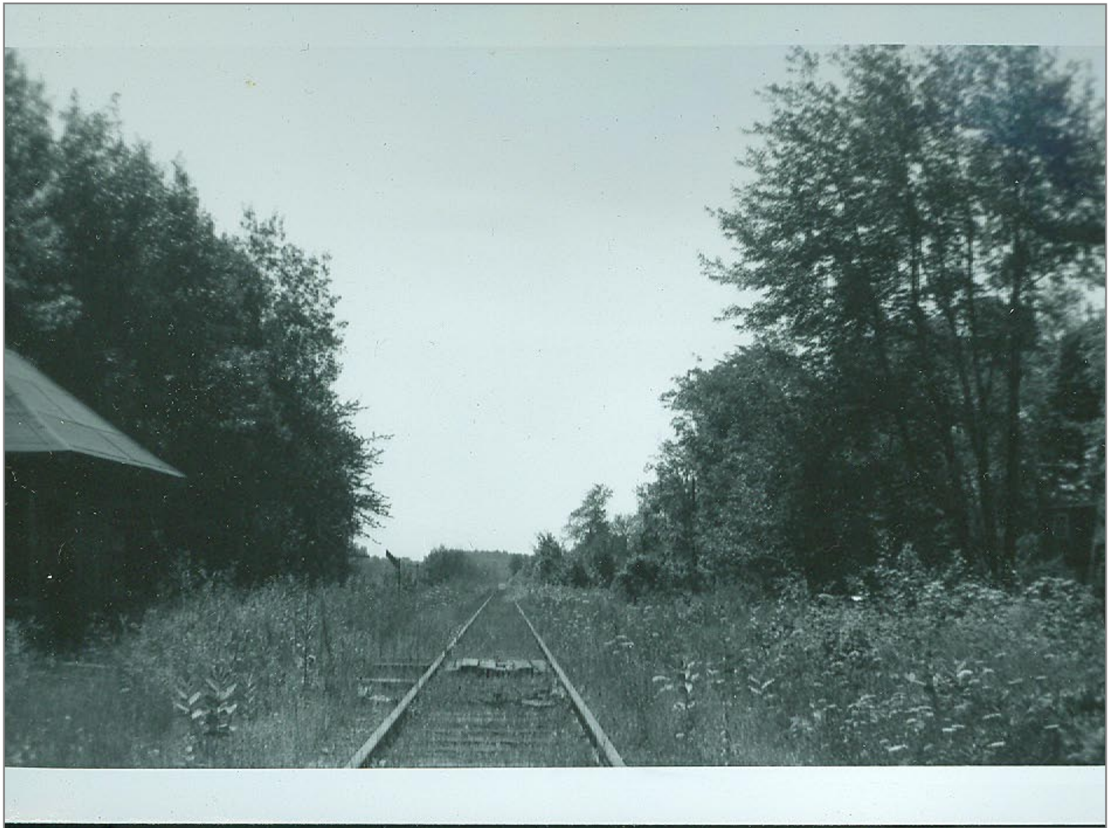
Section House @ Colchester Point Southbound 8/10/62
