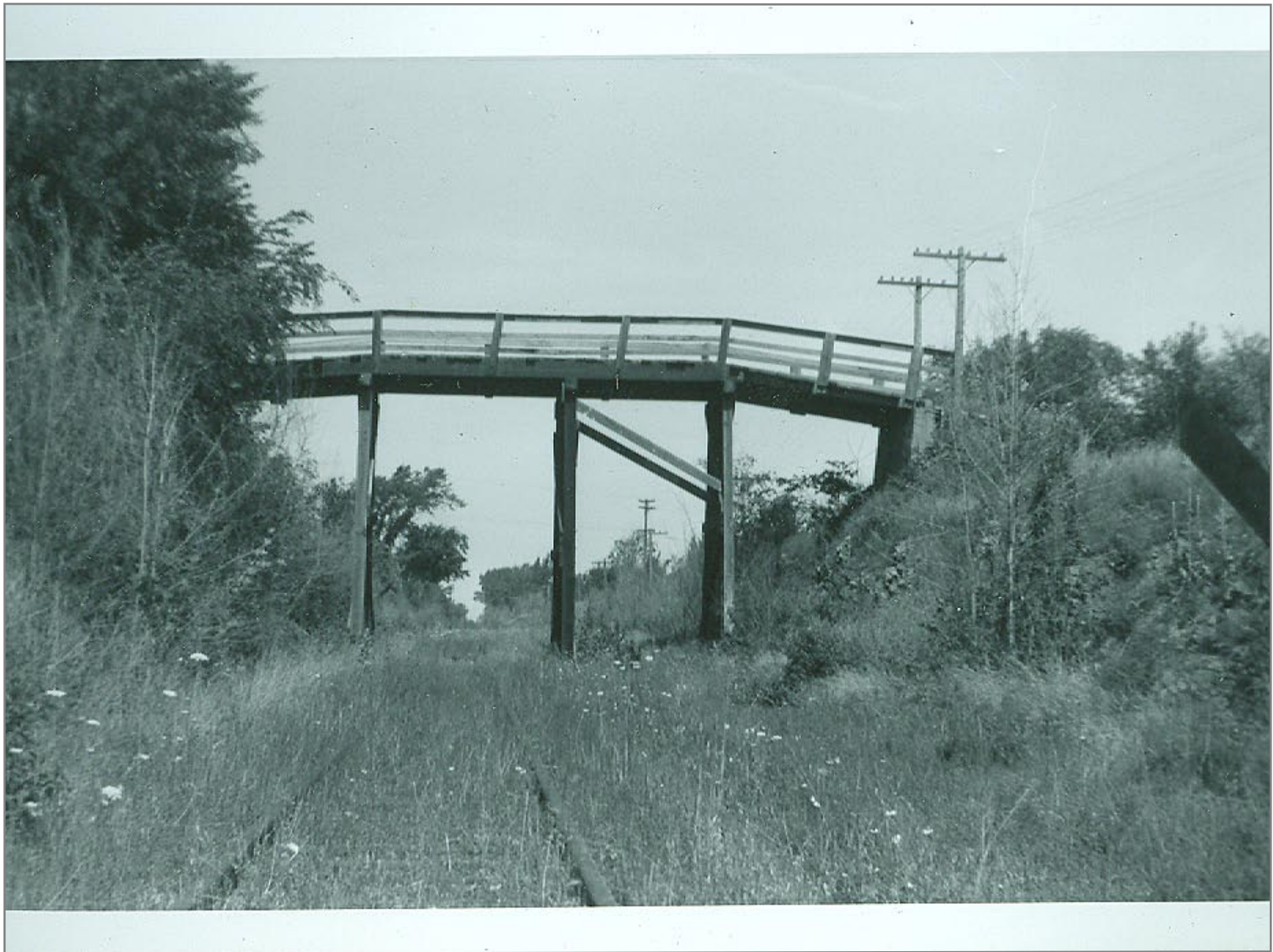
Highway Overpass at Colchester Station Northbound 8/10/62
