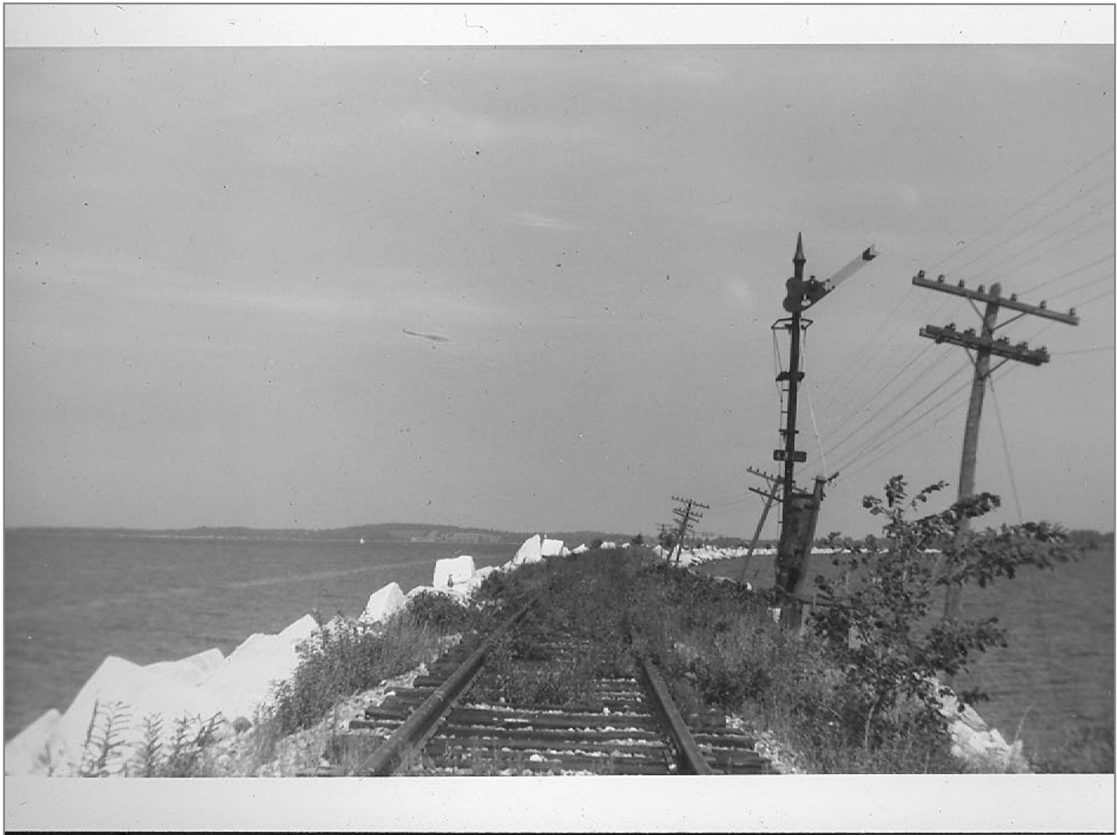
Northbound on Colchester Fill 8/10/62 Signal controls drawbridge
