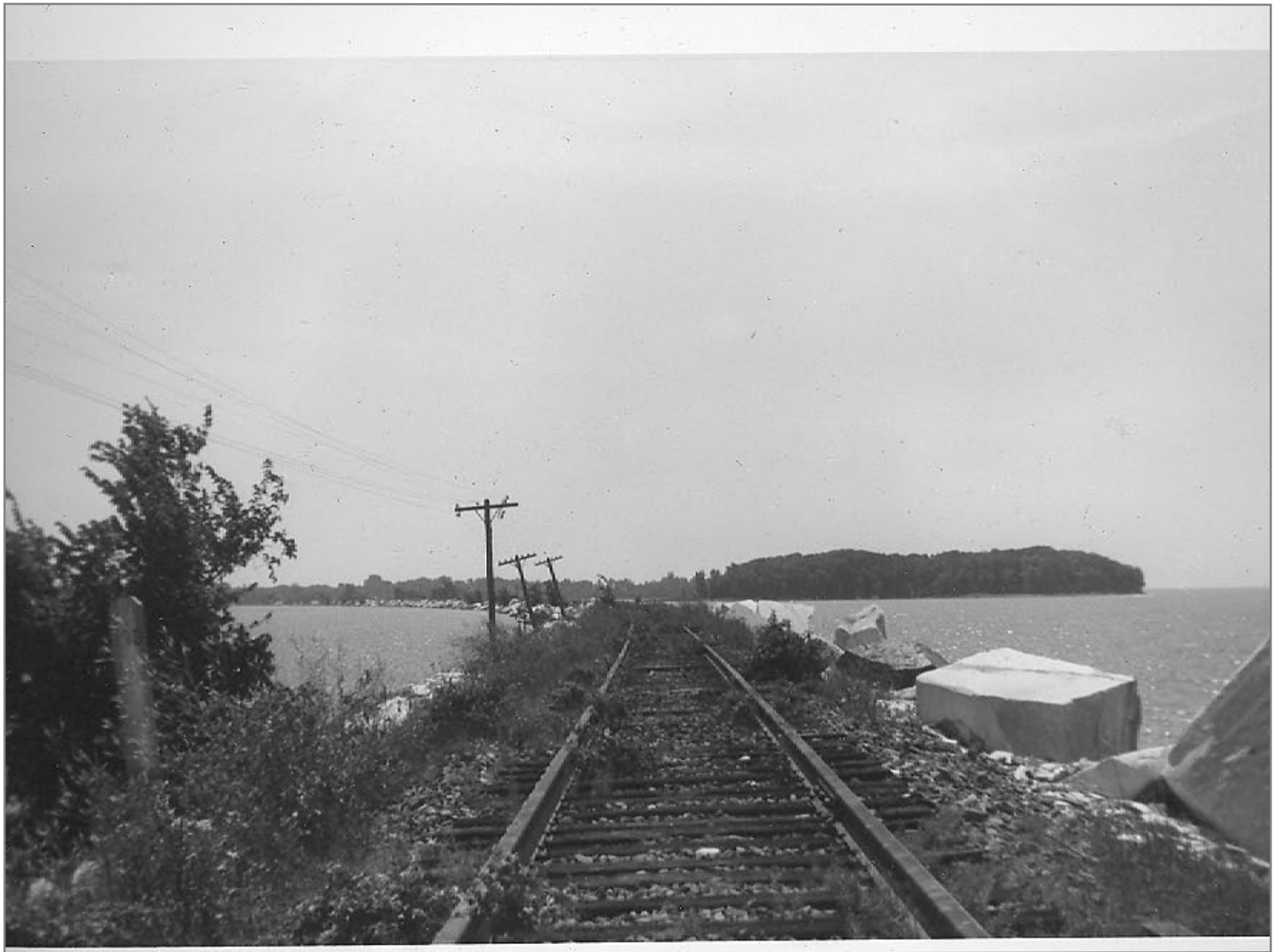
Southbound @ MP 130 on Colchester Fill 8/10/62
