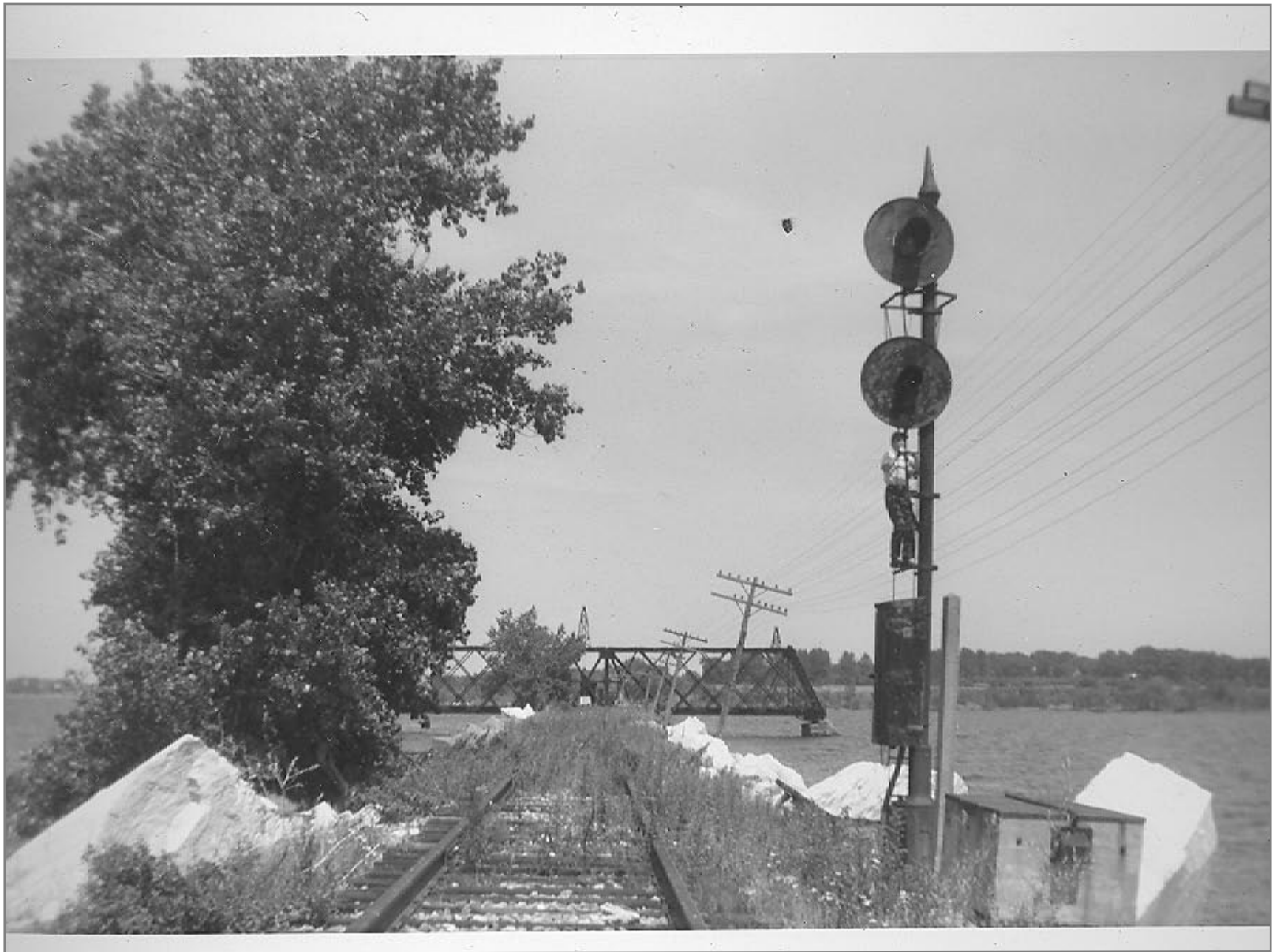
Northbound Bridged 270 in Background 8/10/62
