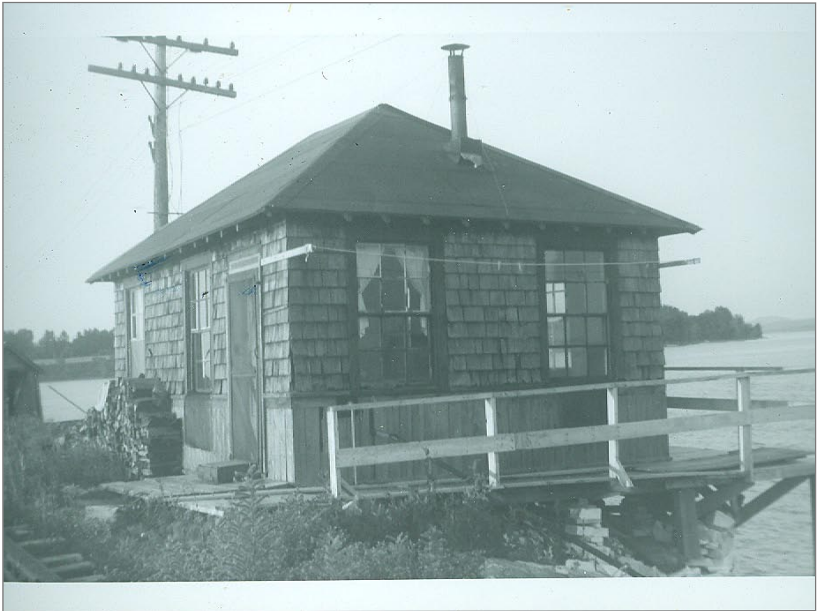
Bridge Tender House 8/10/62 North side of Bridge 8/10/62
