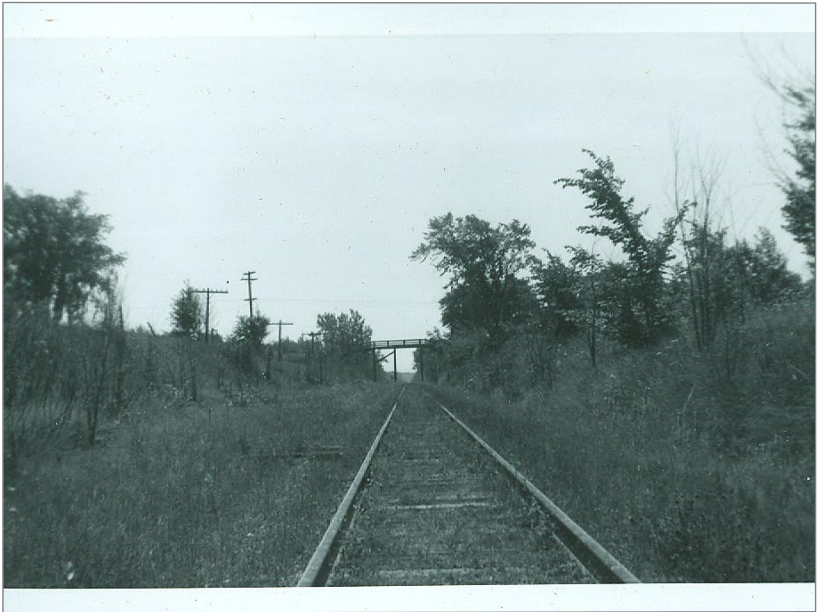
Southbound - Bridge 268 in Distance 8/10/62
