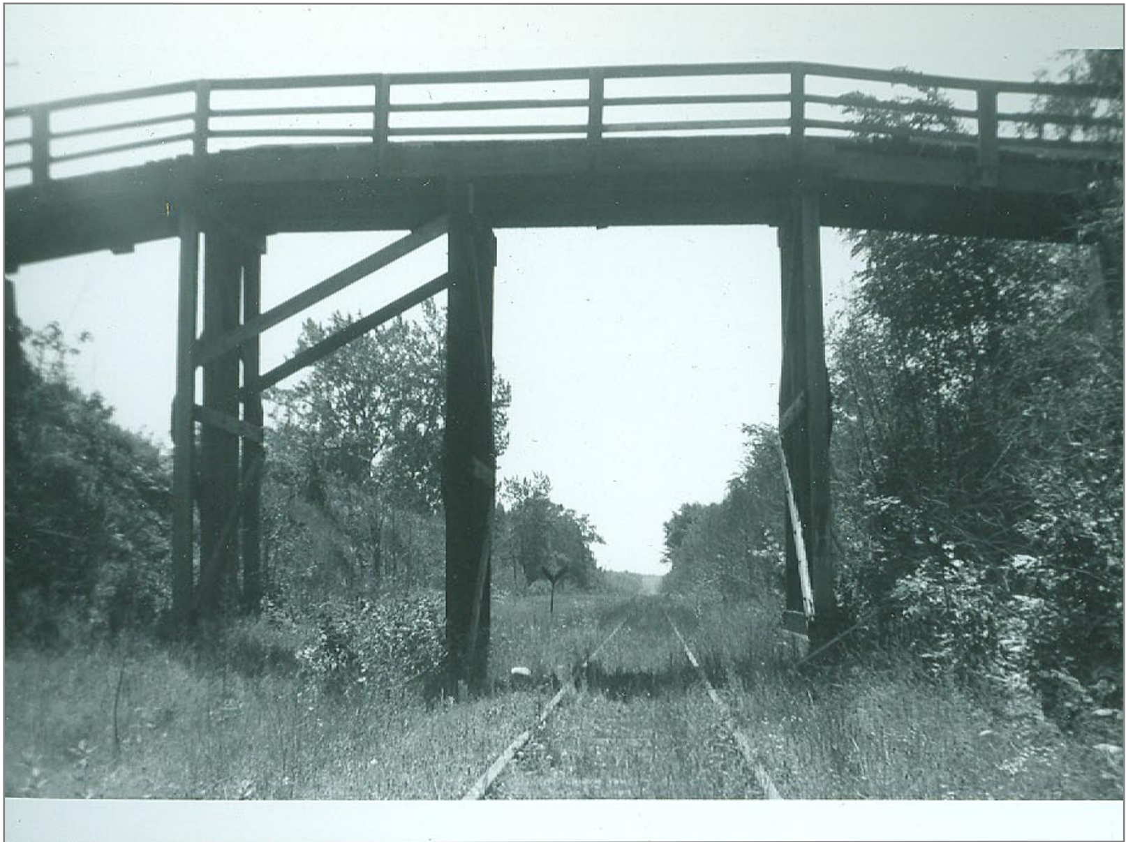
Highway Overpass North of Colchester Station Southbound 8/10/62
