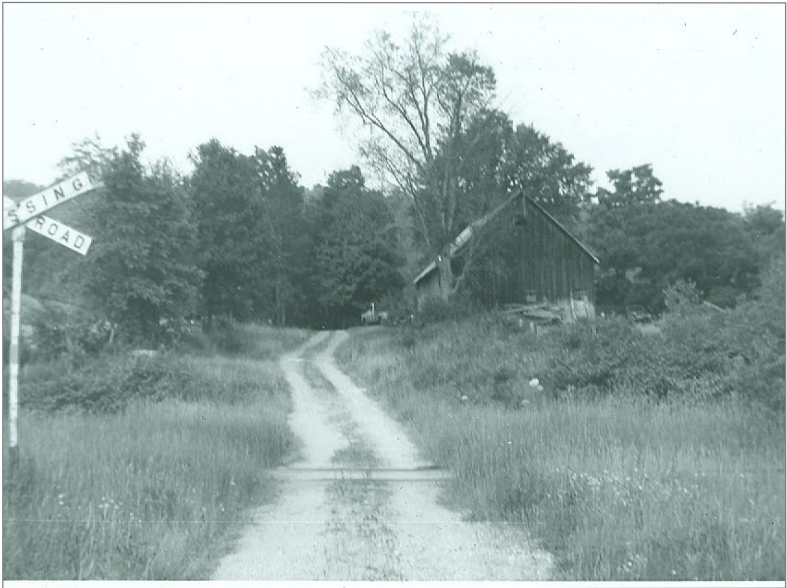
3rd Crossing south of Gassetts looking east
