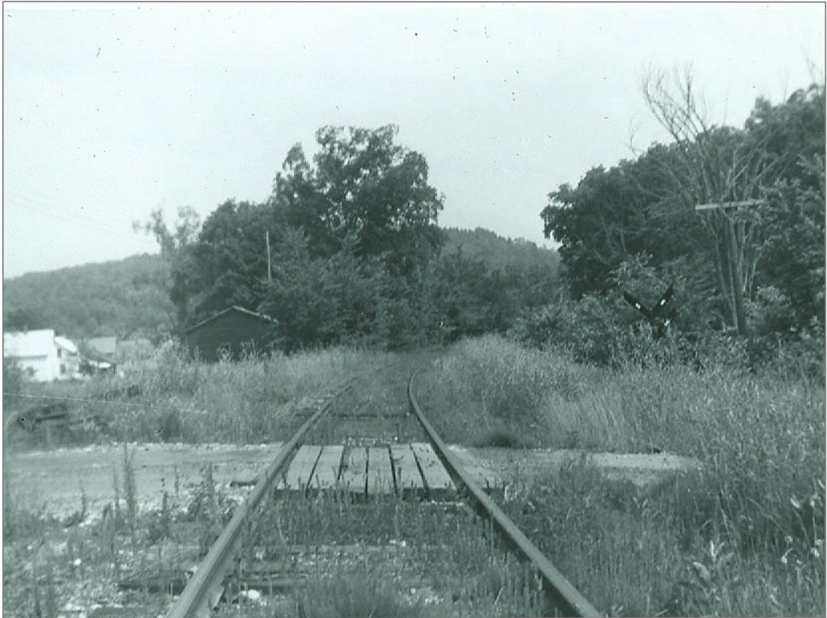
Southbound at bridge 123 on curve in distance
