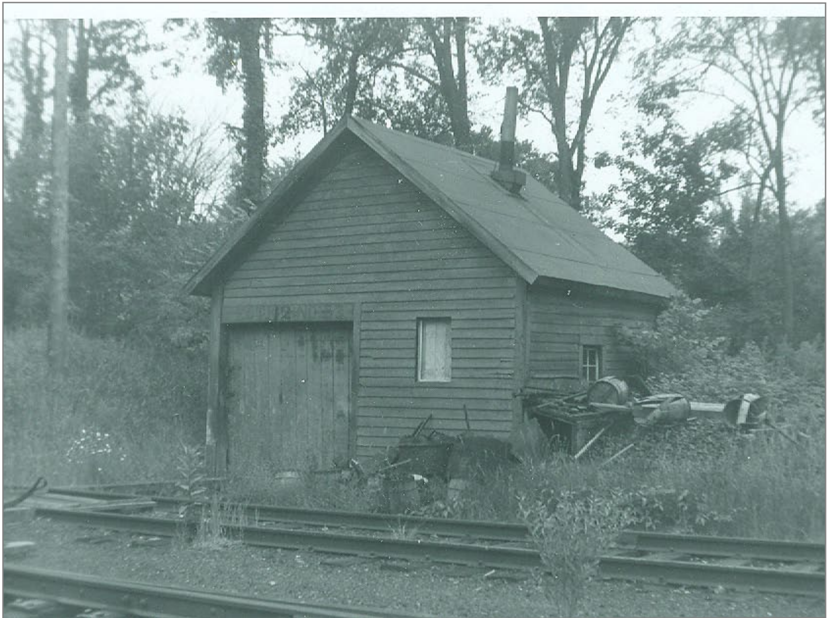
Section House south of Chester Station 7/15/62
