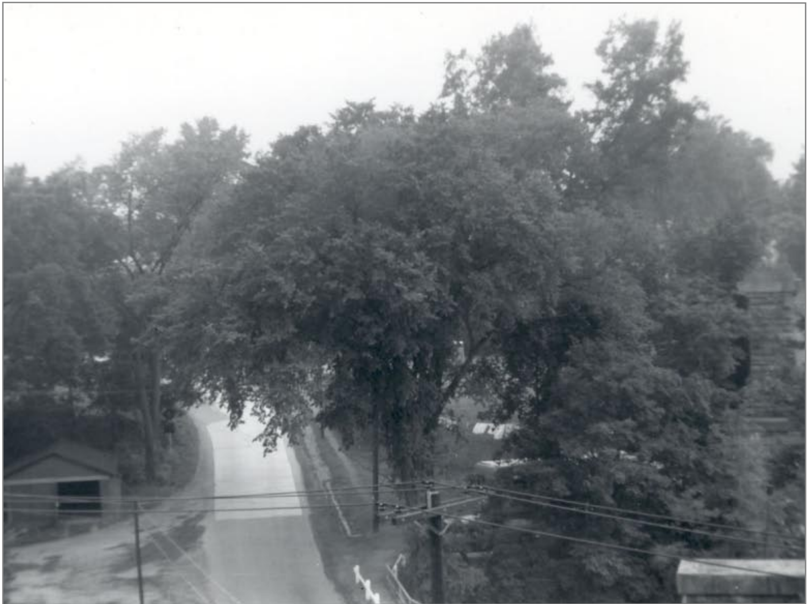
Another View of Chatham High Bridge Location
