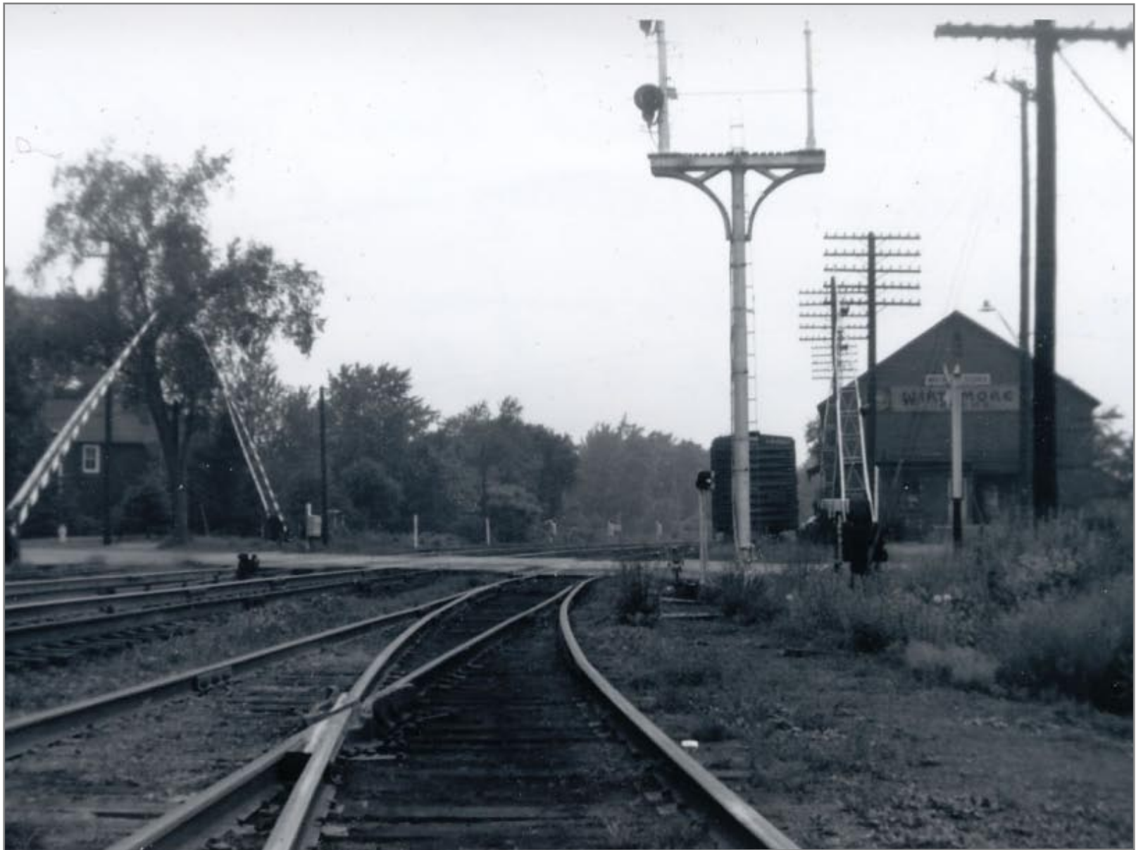
Looking South- Switch to Rutland Yard Right -Tower 66 Out of View to Left 6/28/1962
