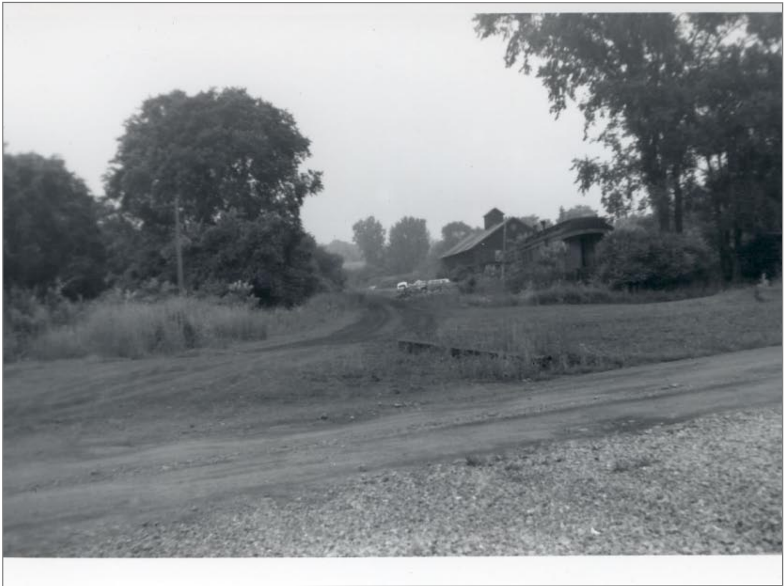
North of High Bridge Looking North into Rutland Yard
