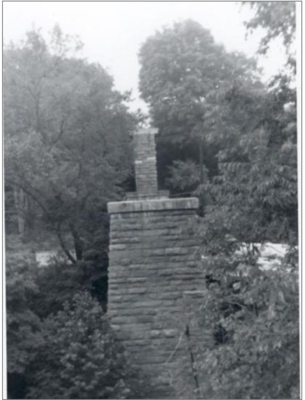
Northbound View of Center Pier Chatham High Bridge 6/24/1962
