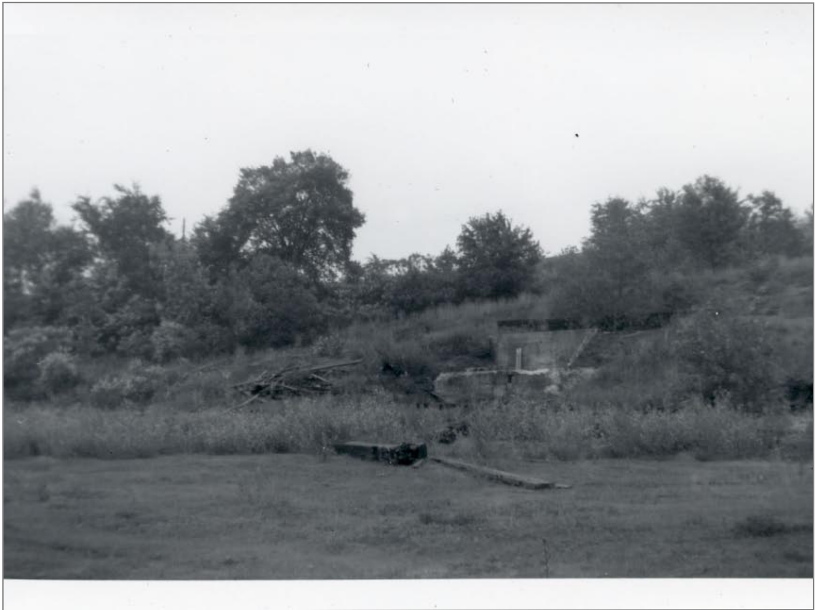
Rutland RR Chatham NY Coaling Tower Foundation
