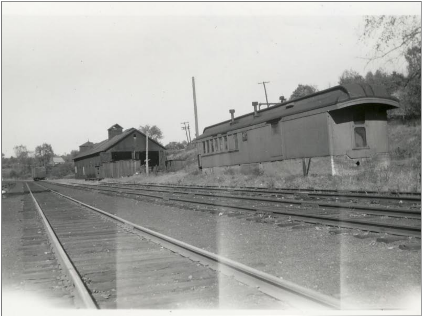
Rutland RR Chatham Yard Office & Enginehouse Looking North 5/1/1953
