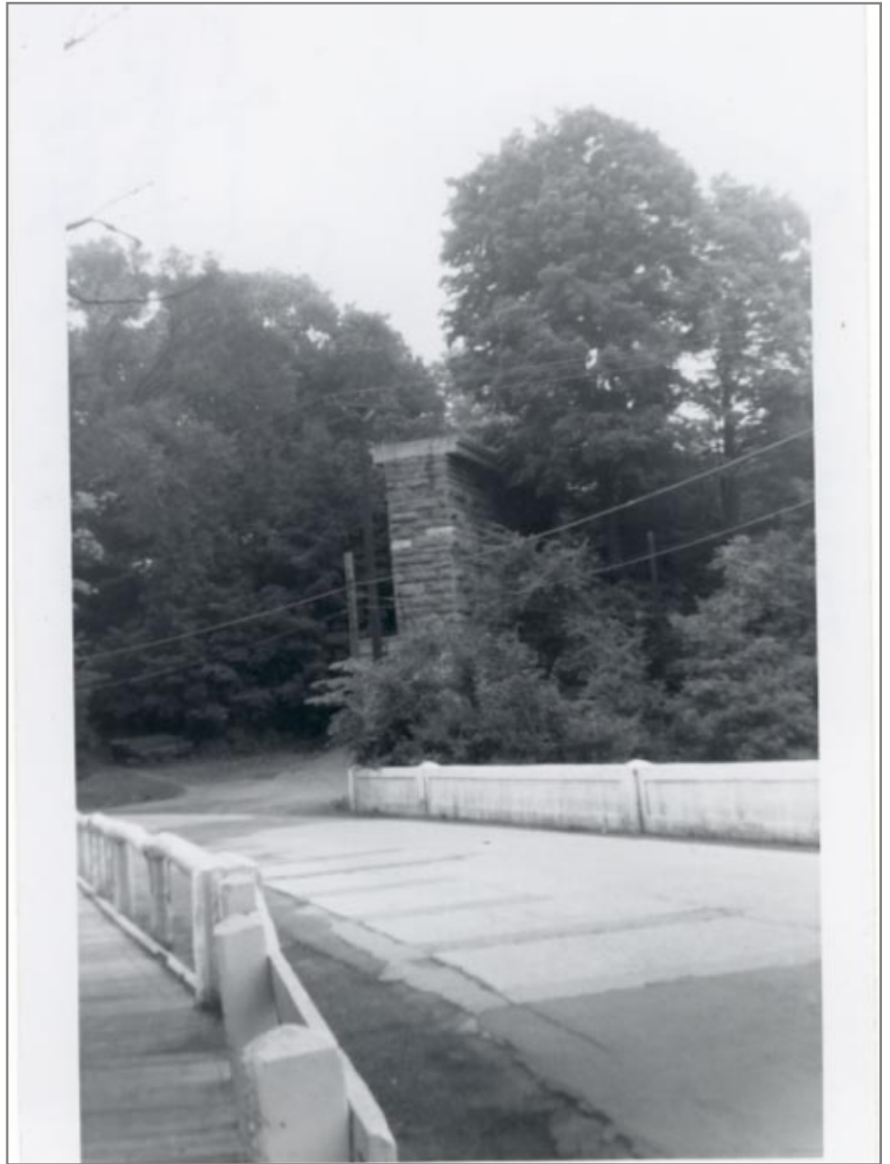
View of North Pier Chatham High Bridge From NY RT 66 6/23/1962
