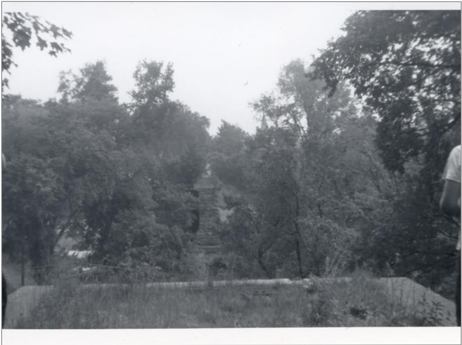
Looking South - High Bridge From North Abutment- 6/23/1962
