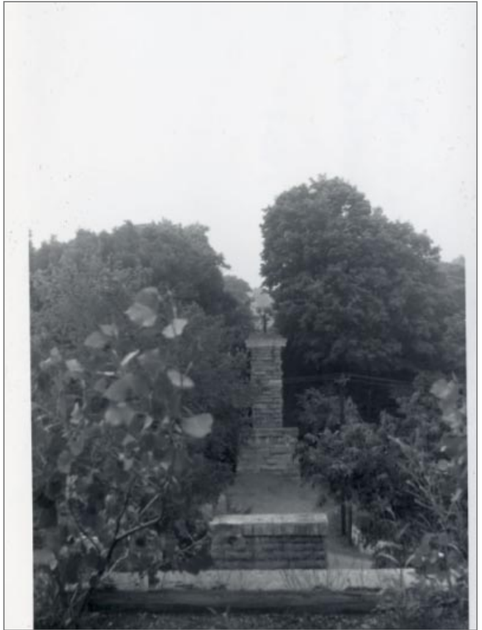
View From South Pier of High Bridge Over NY RTE 66 Looking North 6/23/1962
