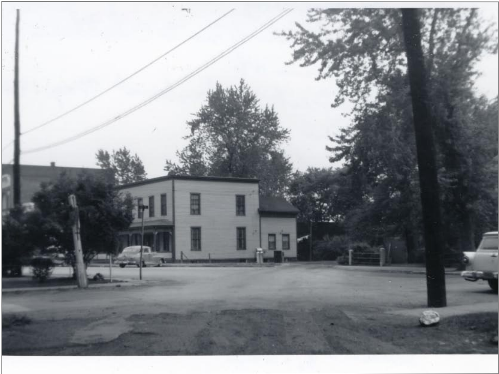
Looking South Rutland ROW into Chatham @ Park Street 6/24/1962
