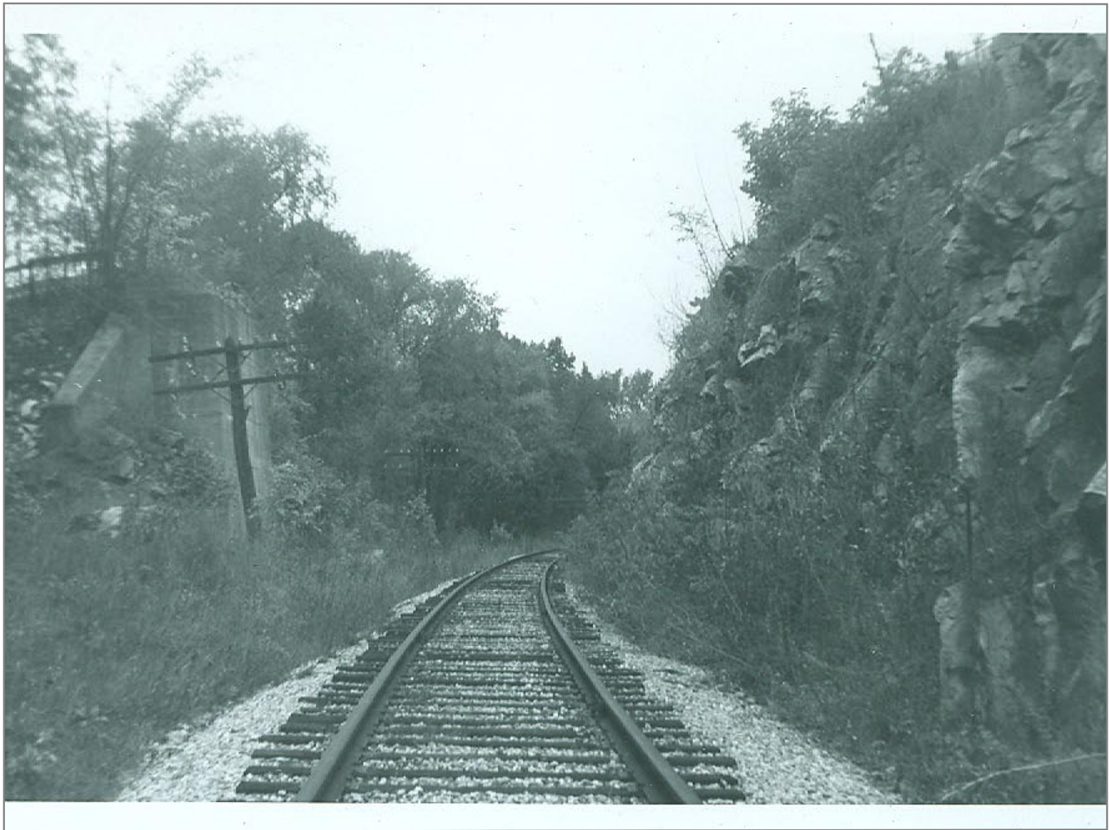
Northbound - Pier of overhead bridge on left
