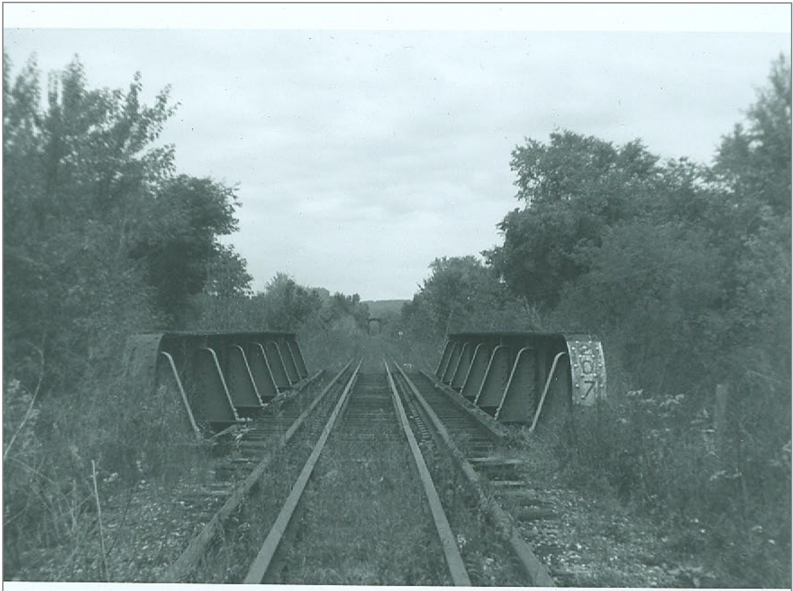
Northbound Bridge 207 American Bridge Co. 1902
