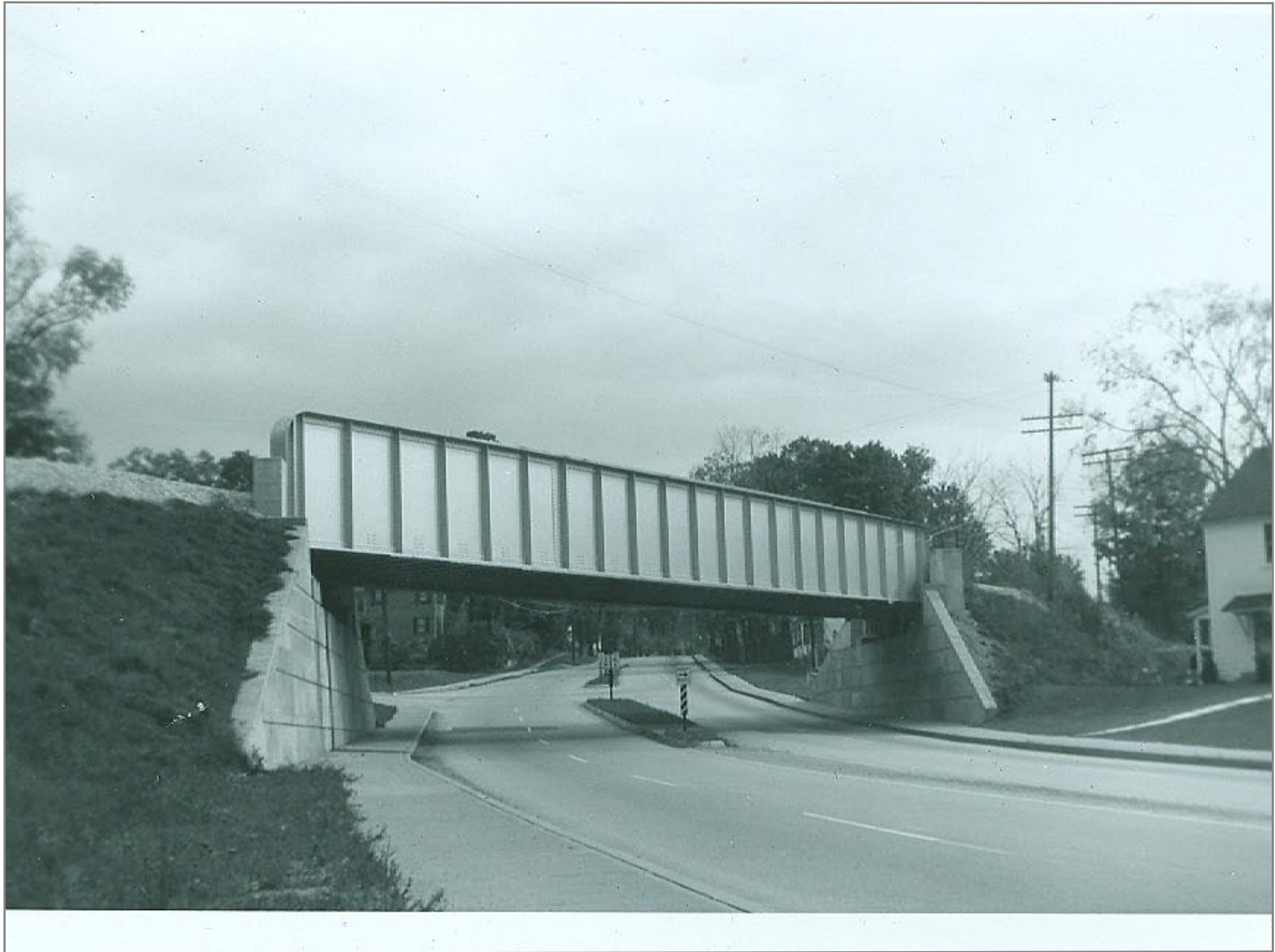
Bridge over rte 4 ctr. rutland
