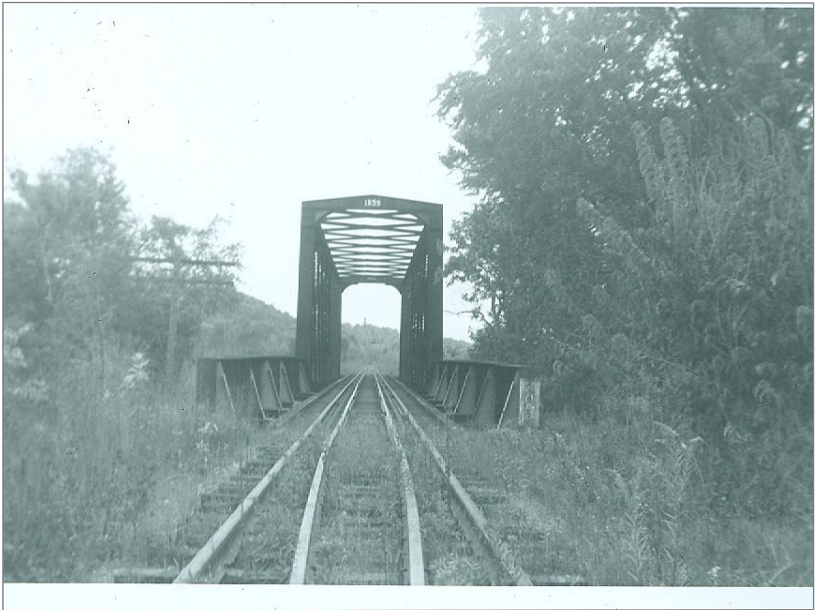
Bridge 205 Northbound Built 1899
