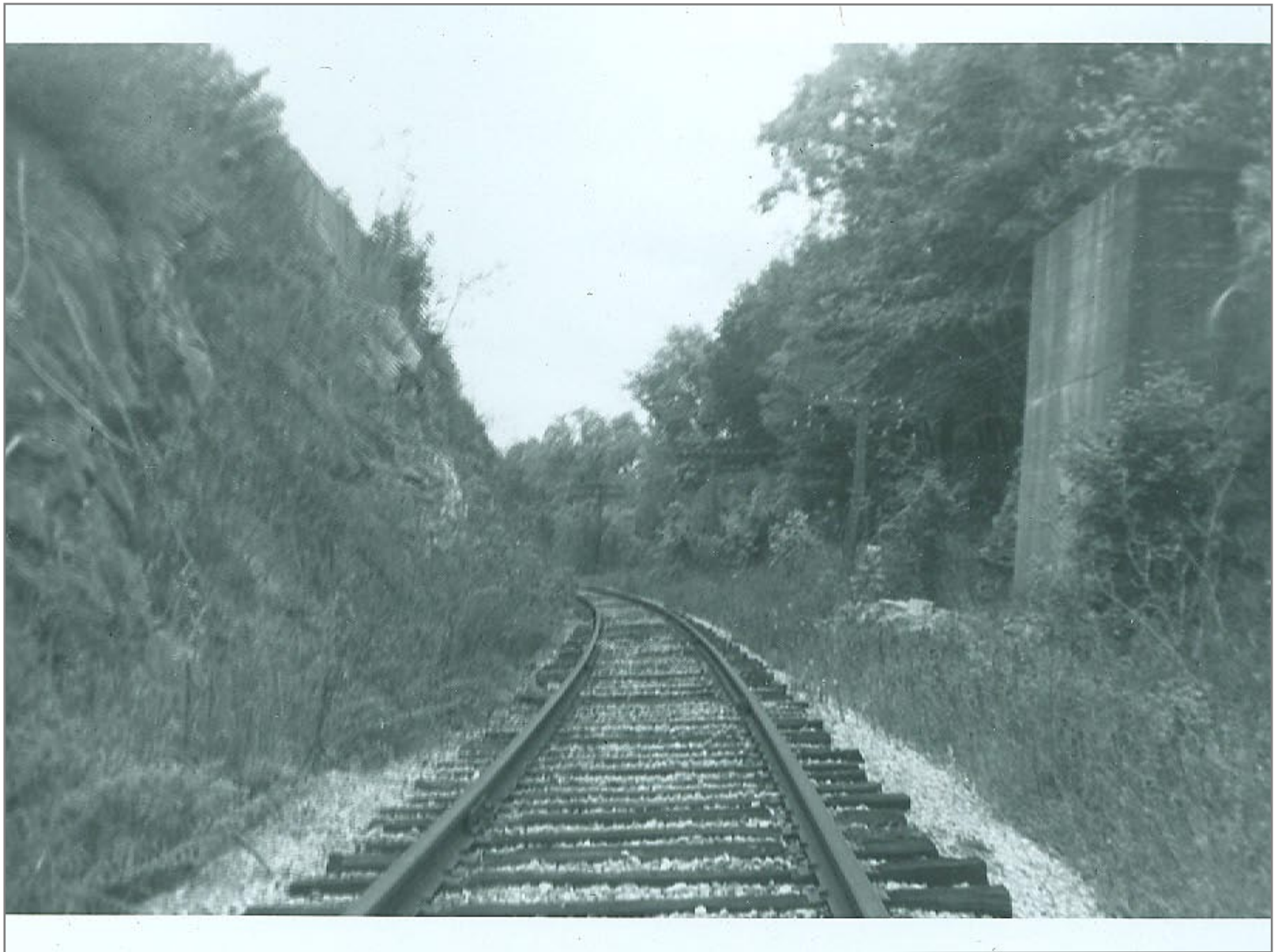
Southbound - Former overhead bridge abutment on right
