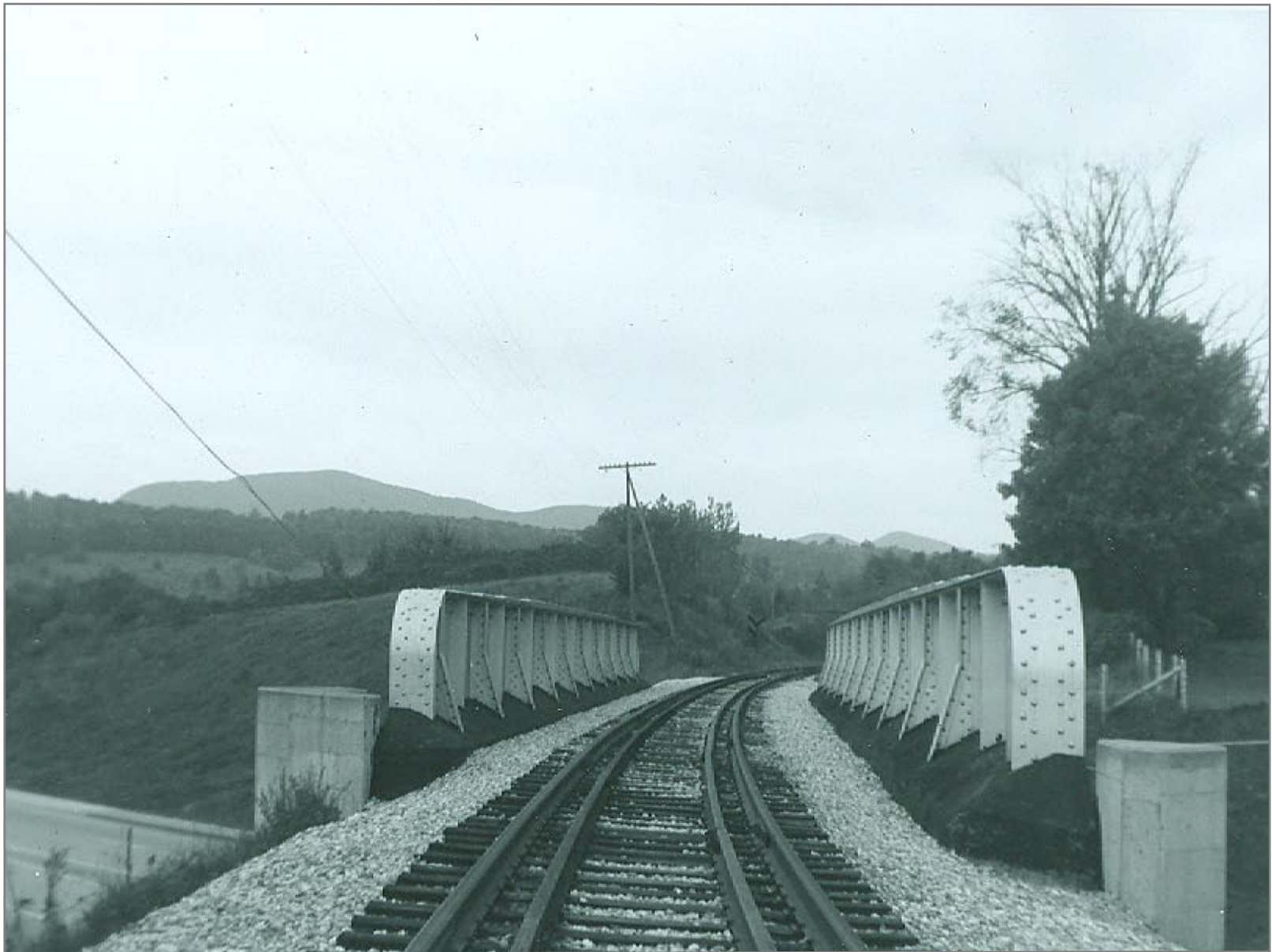
Bridge over Route 4 Northbound
