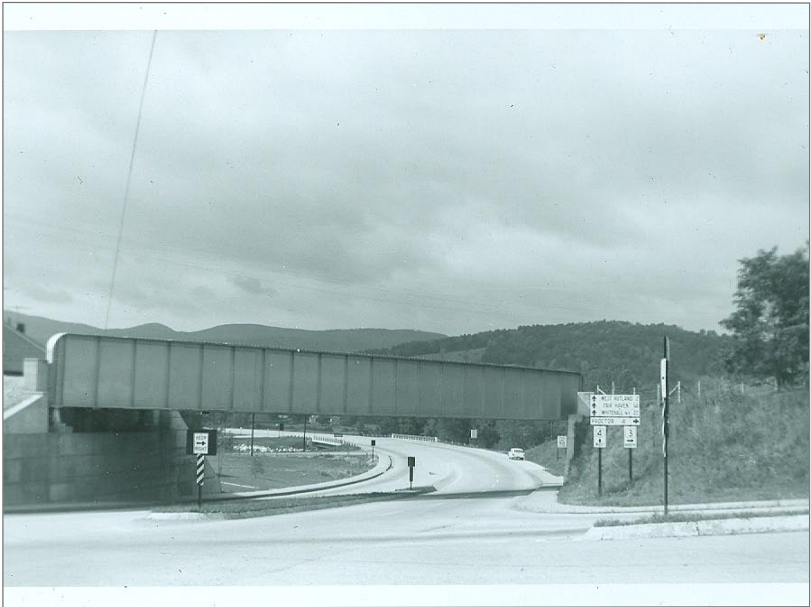
Bridge over Rte. 4 just north of ctr rutland
