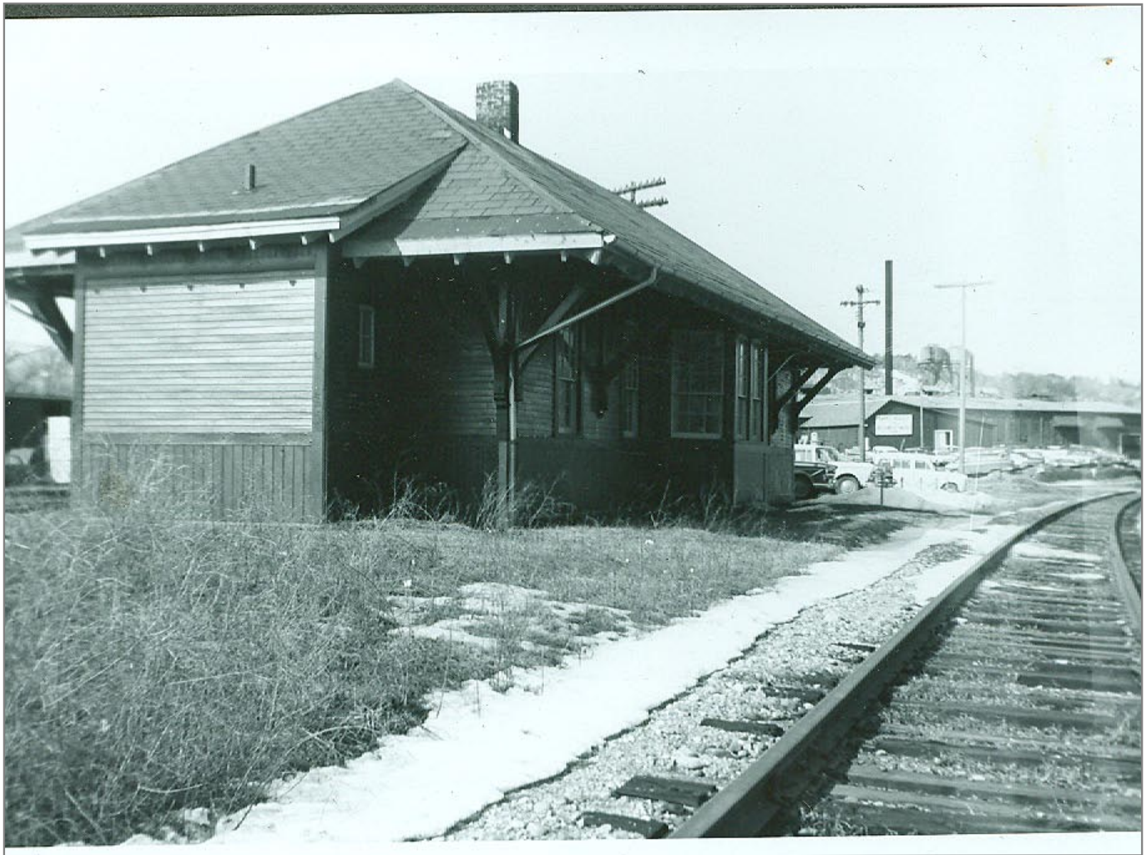
Center Rutland Station looking northbound
