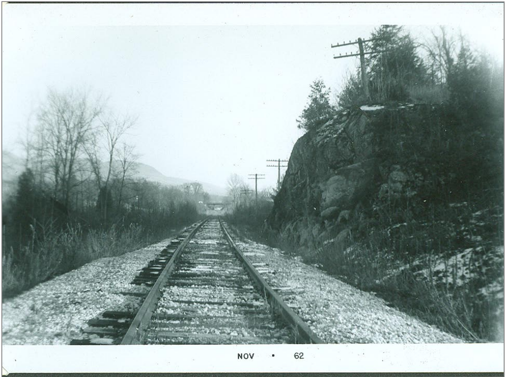
Southbound into Brandon
