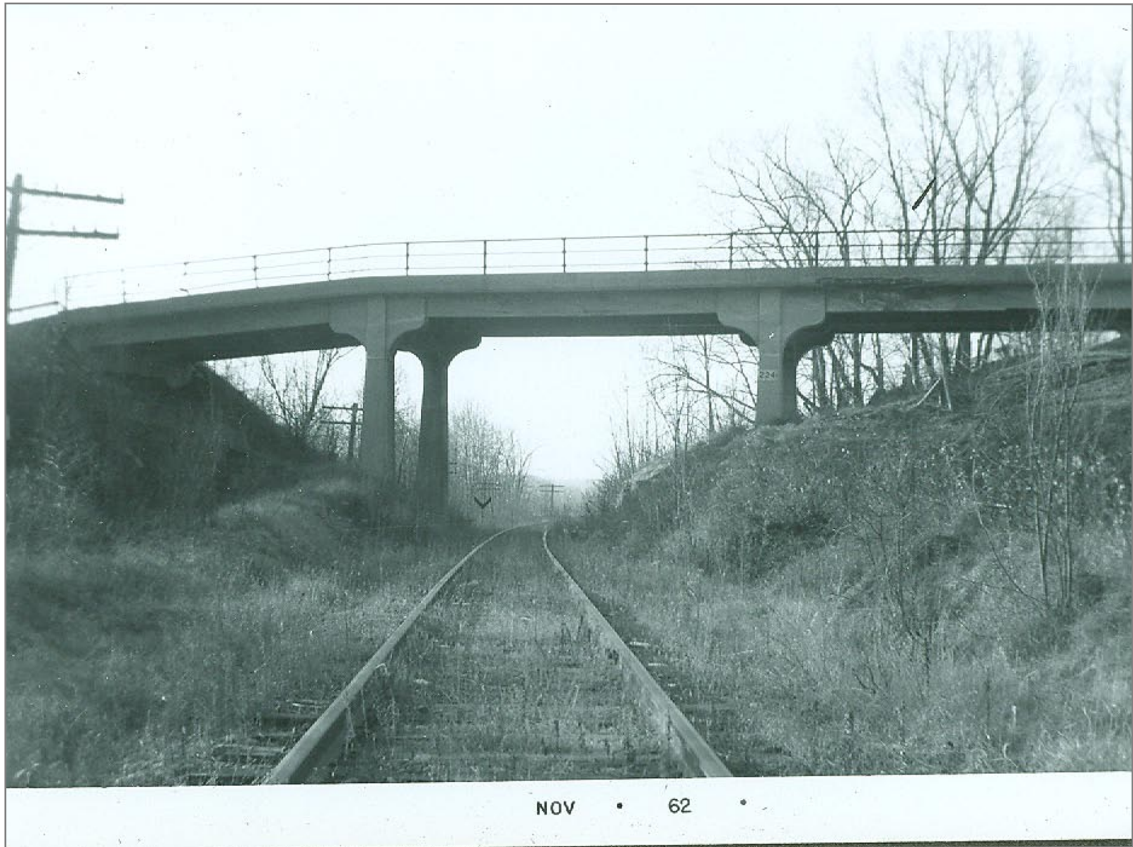
Route 73 Bridge Northbound
