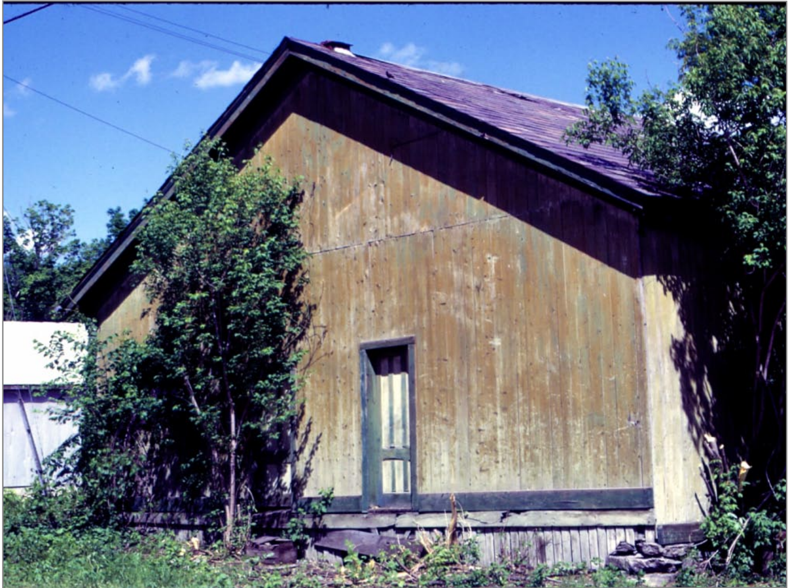
North end of Brandon freight house
