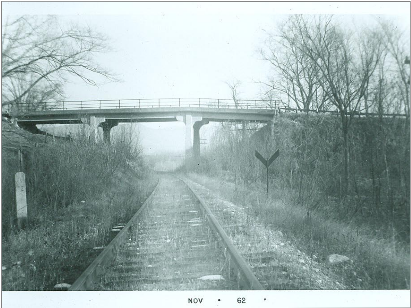
Bridge carrying Route 73 Southbound
