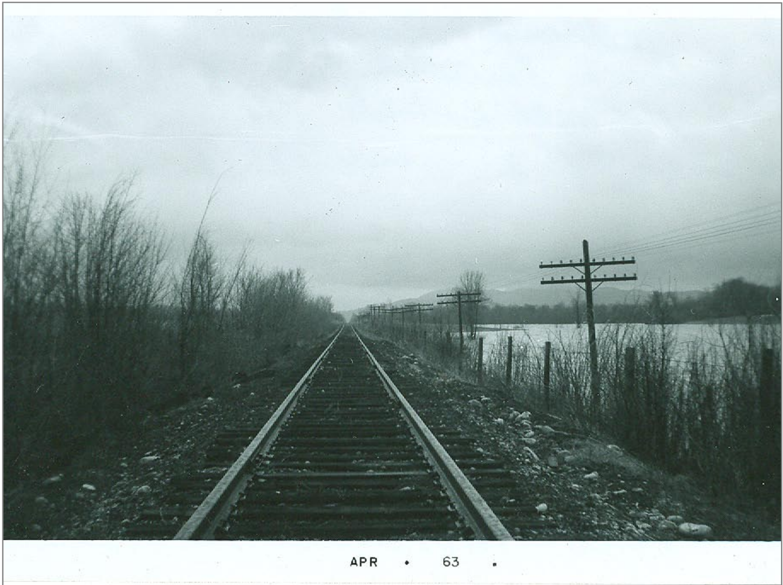
Southbound Floodwaters from Otter creek on right just south of Leicester
