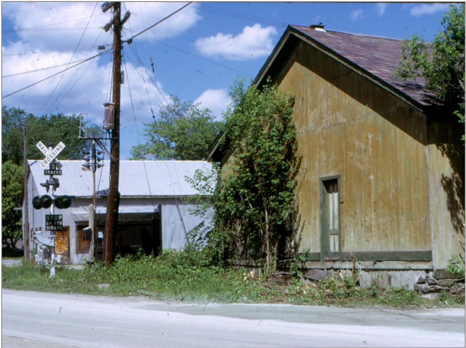
North end of Brandon freight House
