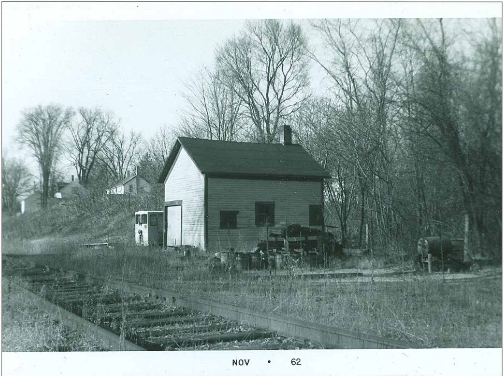
Brandon Section House Looking North
