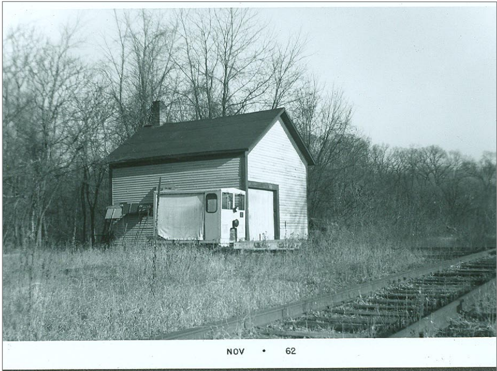
Brandon Section House Looking South
