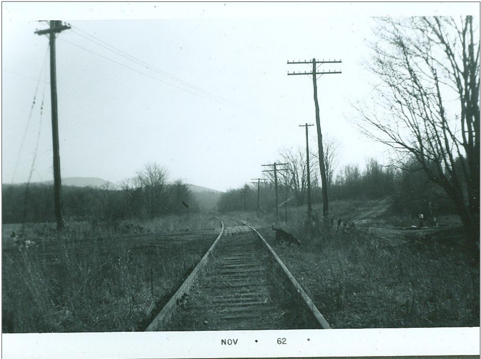
Southbound south of Brandon
