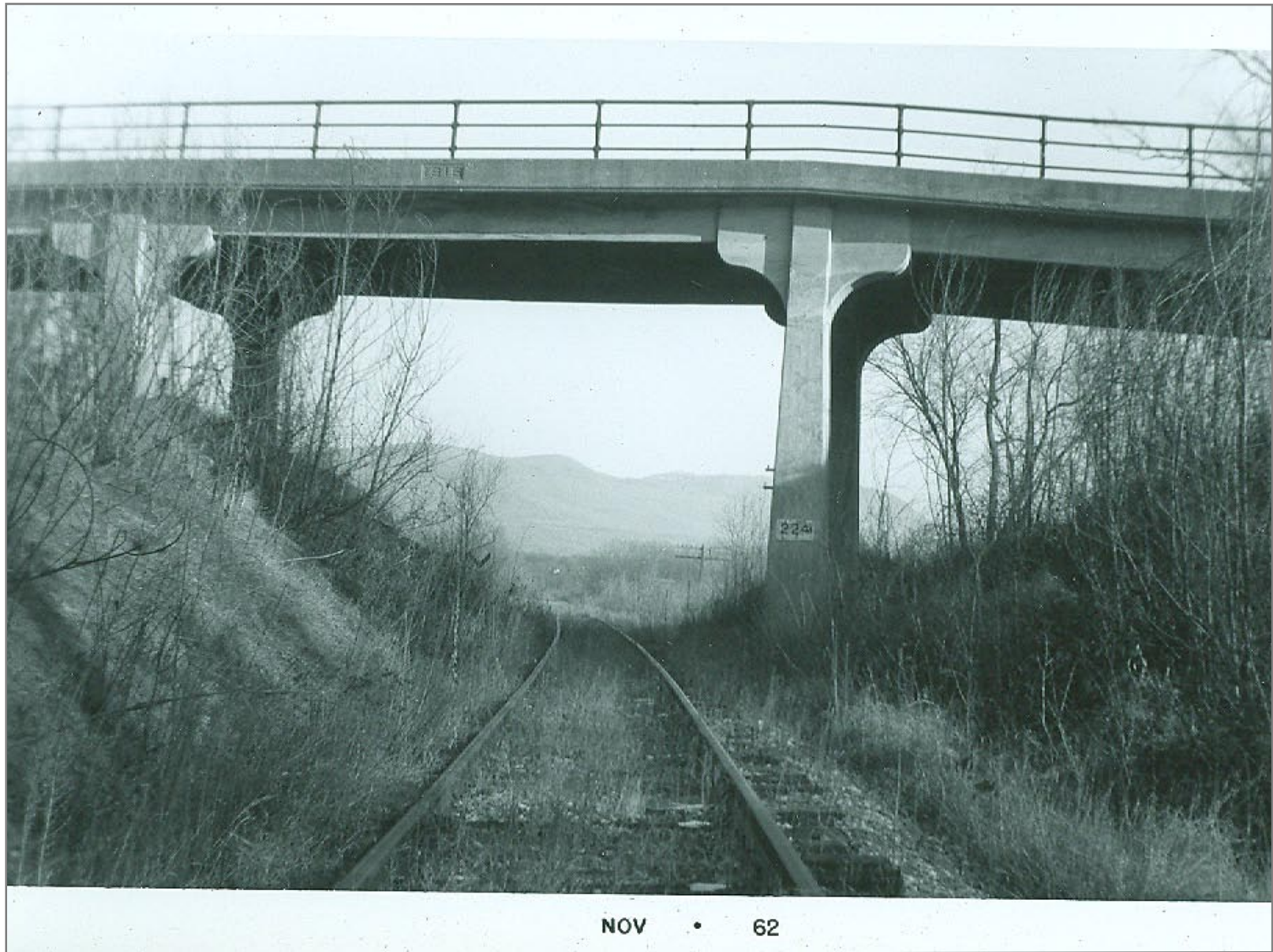
Southbound under bridge 224a built 1916 carrying VT Rte. 73
