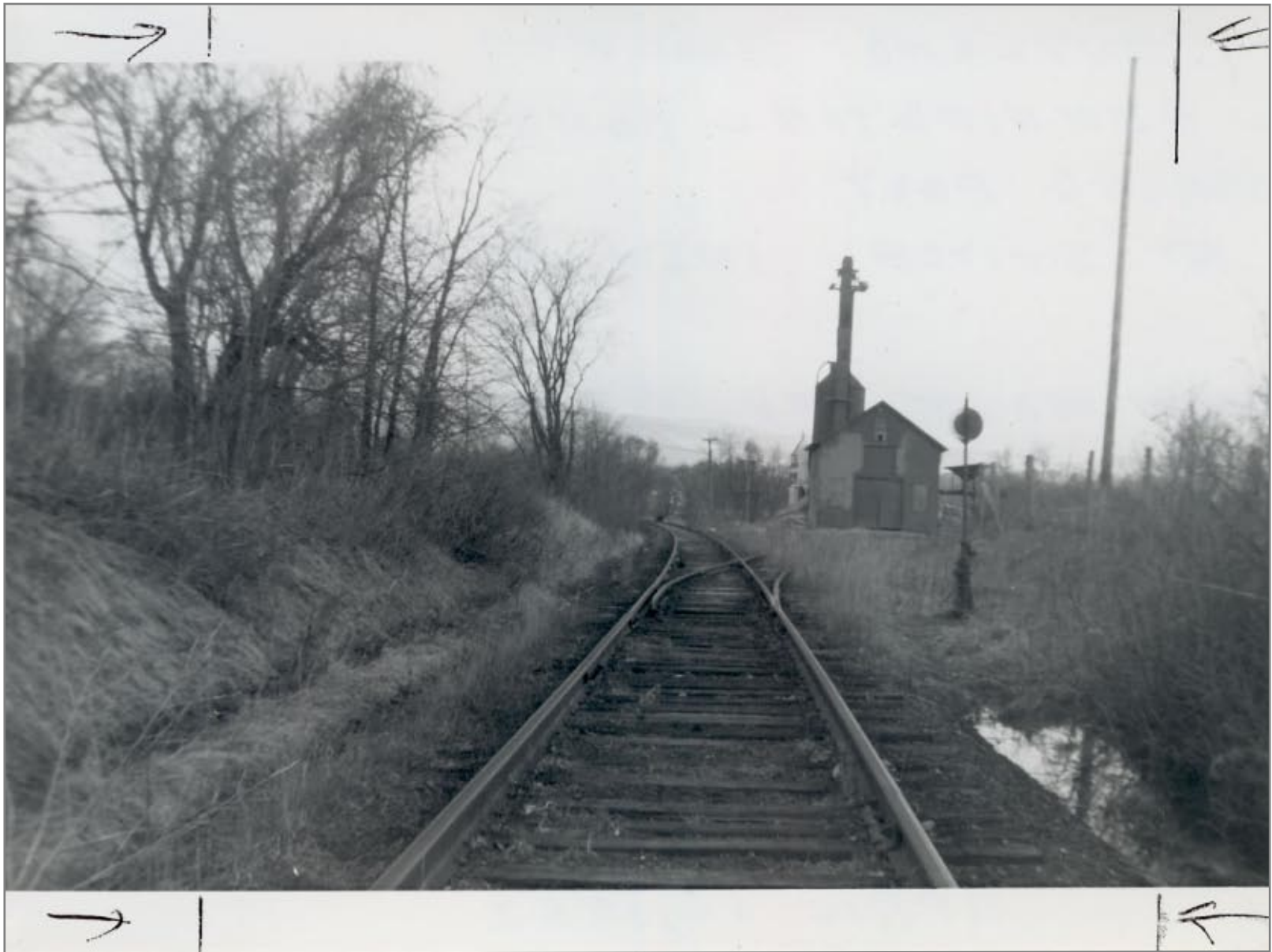
Looking South at Switch into Morse Block 4/15/1962
