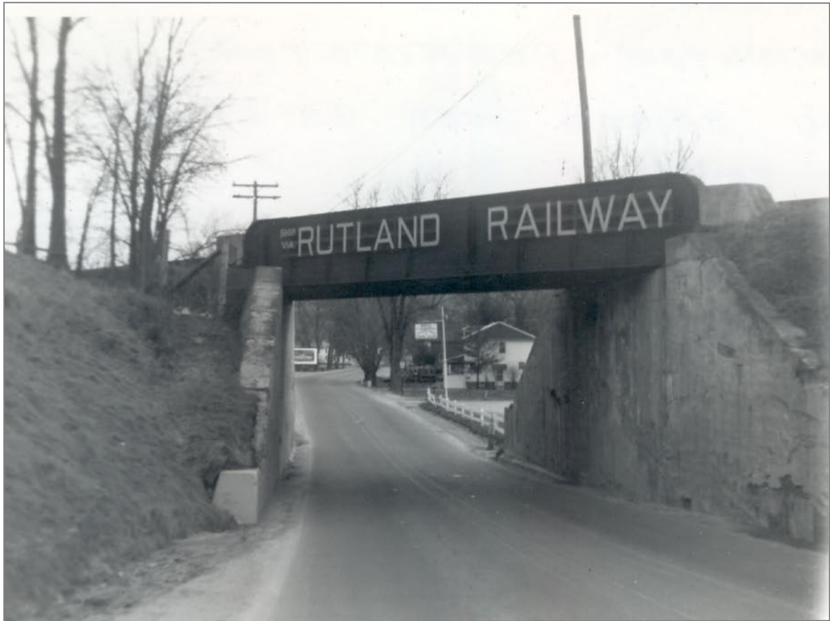
Bridge over Route 7 Built 1914 4/15/1962
