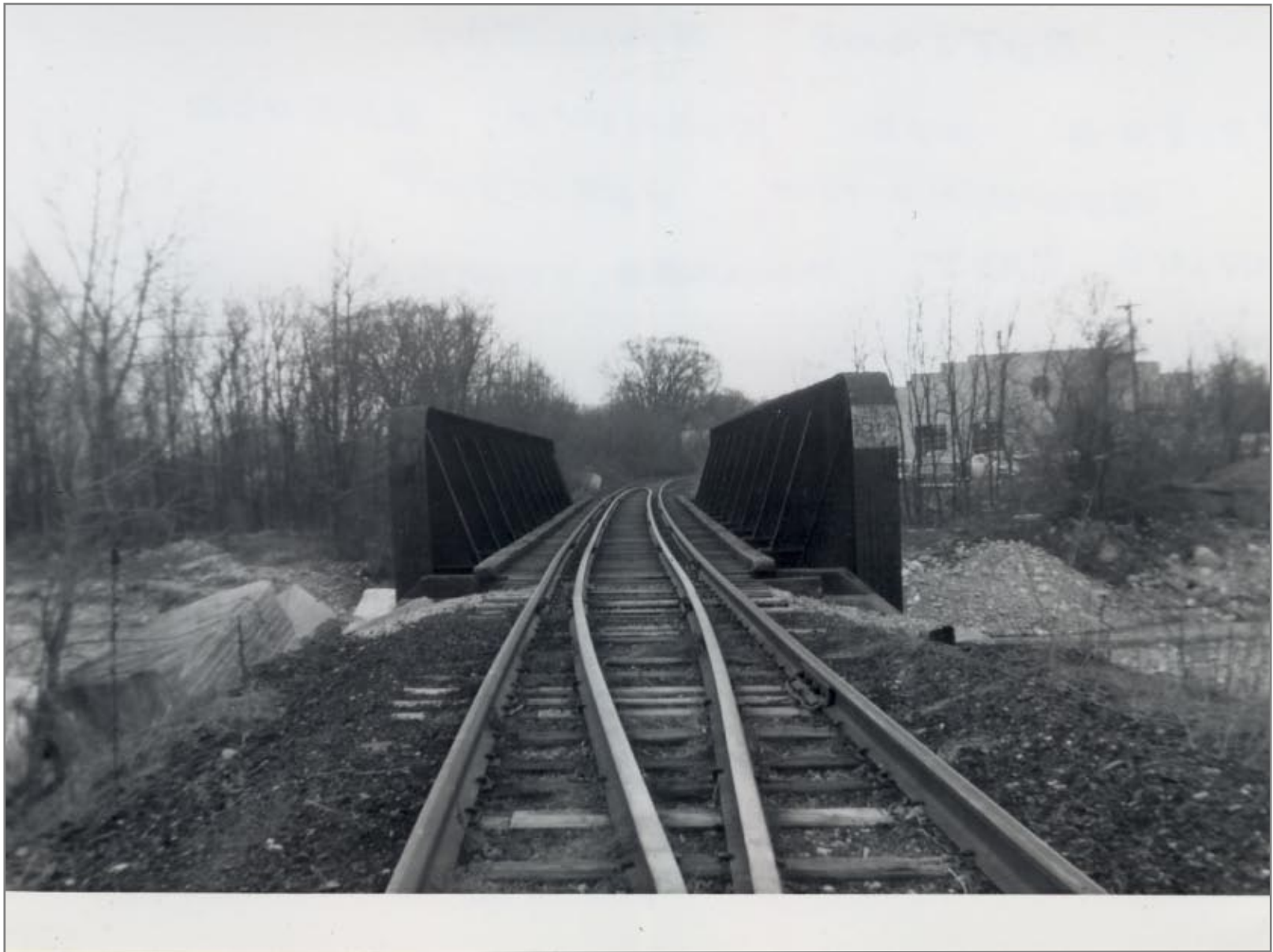
Bridge #55 Looking South 4/20/1962
