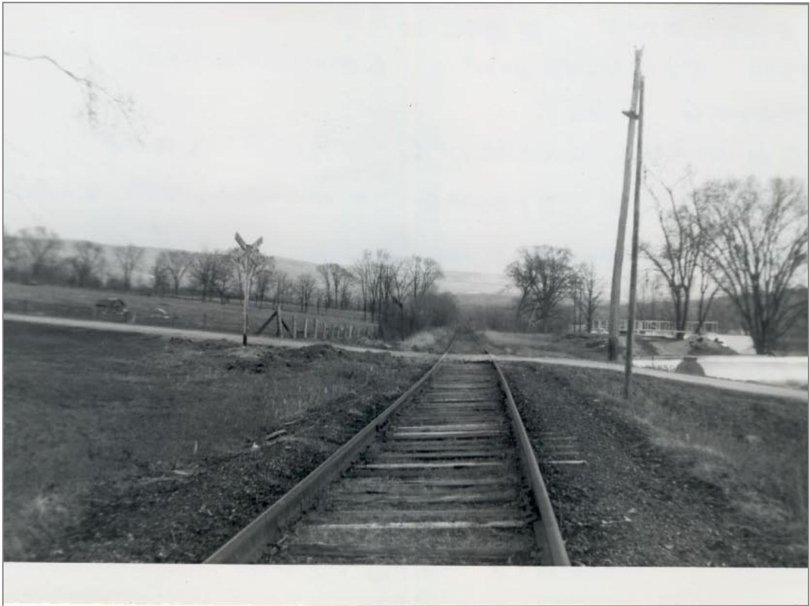
Looking South at Rice Lane Abandoned Siding on Right Beyond Crossing to Johnson & Dix Oil ( Shell ) 4/15/1962
