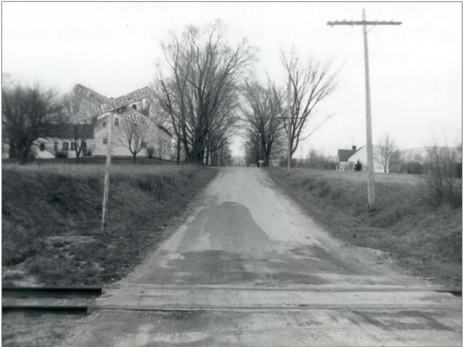
Overlee Road Crossing Looking Northeast 4/15/1962
