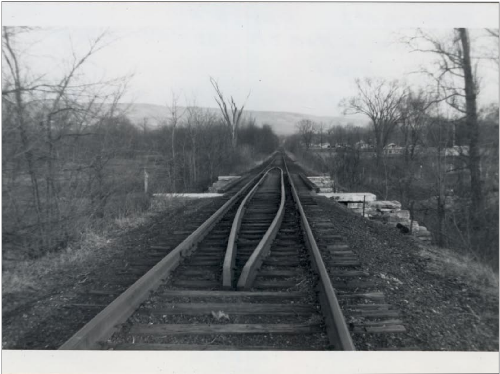
Looking South at Bridge over Oakers Stream 4/15/1962
