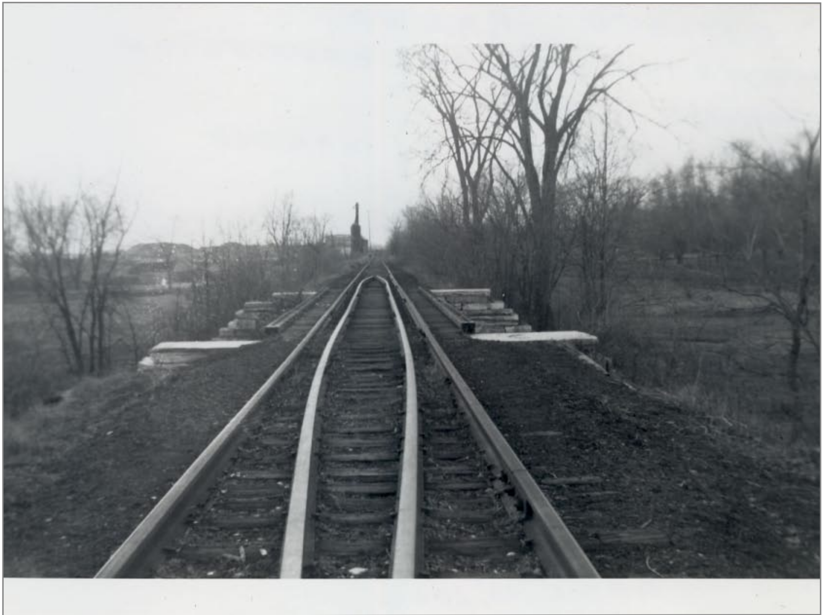
Looking North - Bridge over Oakers Stream Morse Block in Distance 4/15/1962
