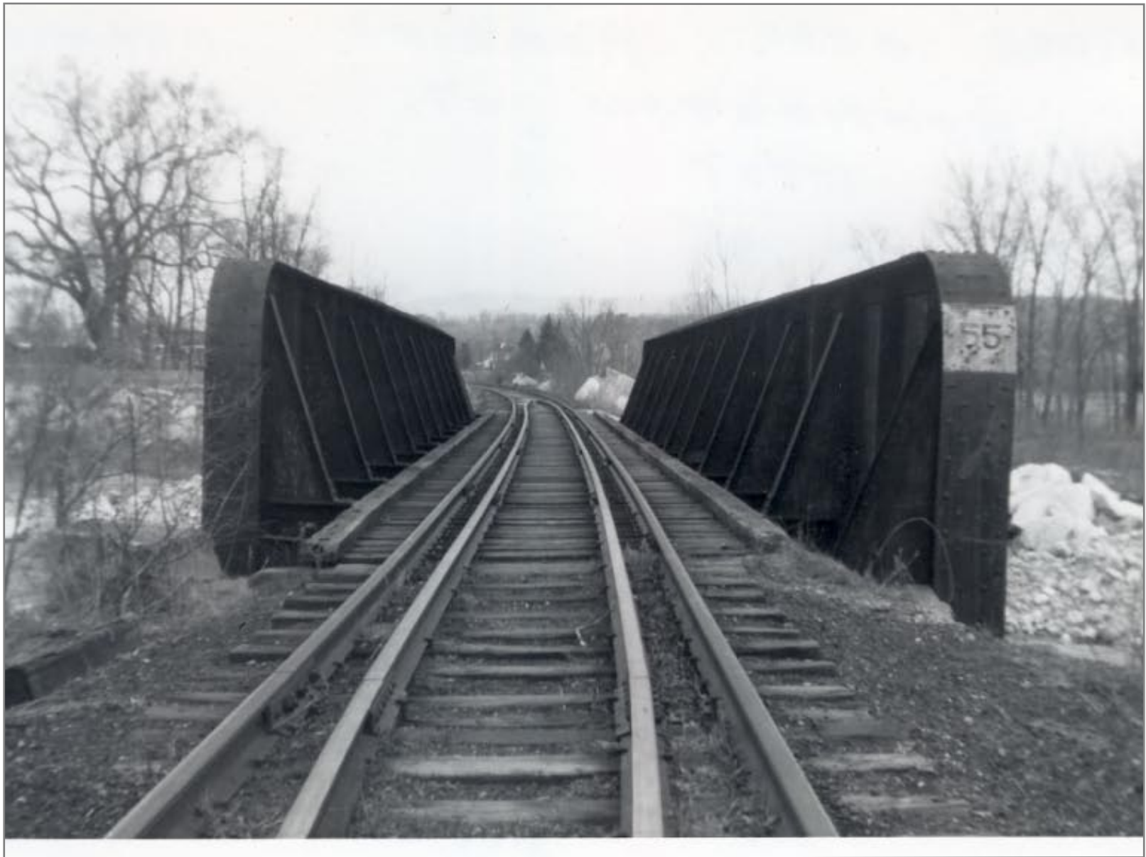
Bridge #55 Looking North 4/20/1962
