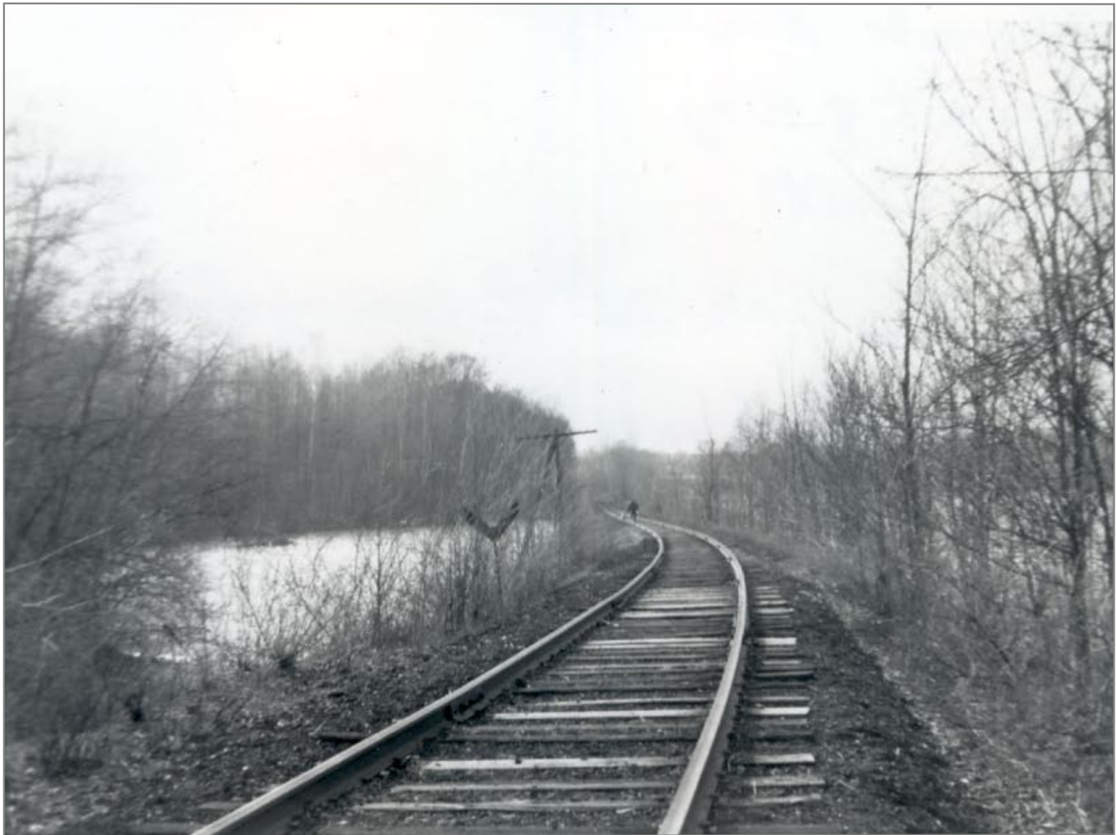
Looking North at Embankment thru Lake Paran 4/15/1962
