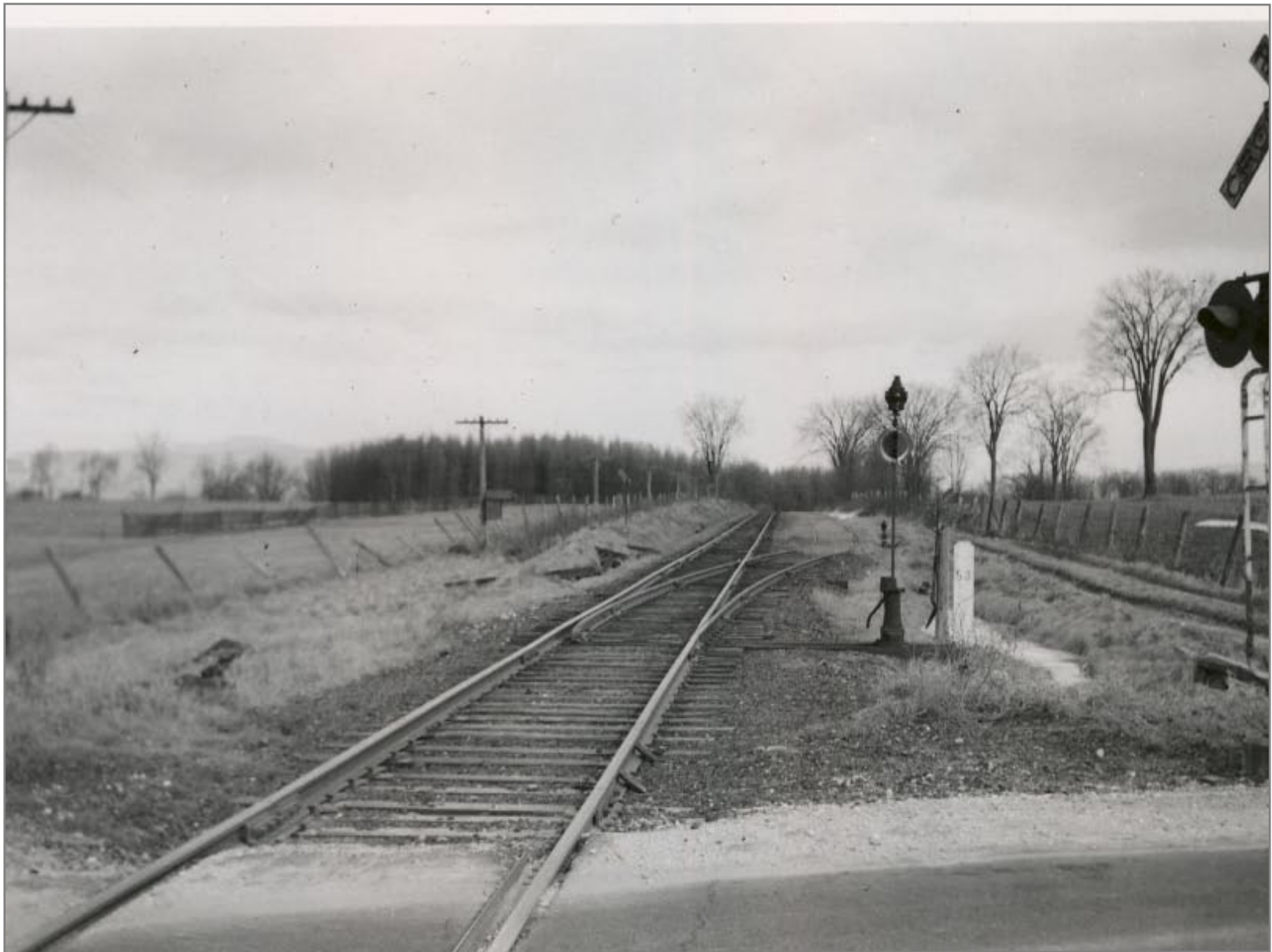
Anthony Siding before Bennington 1951
