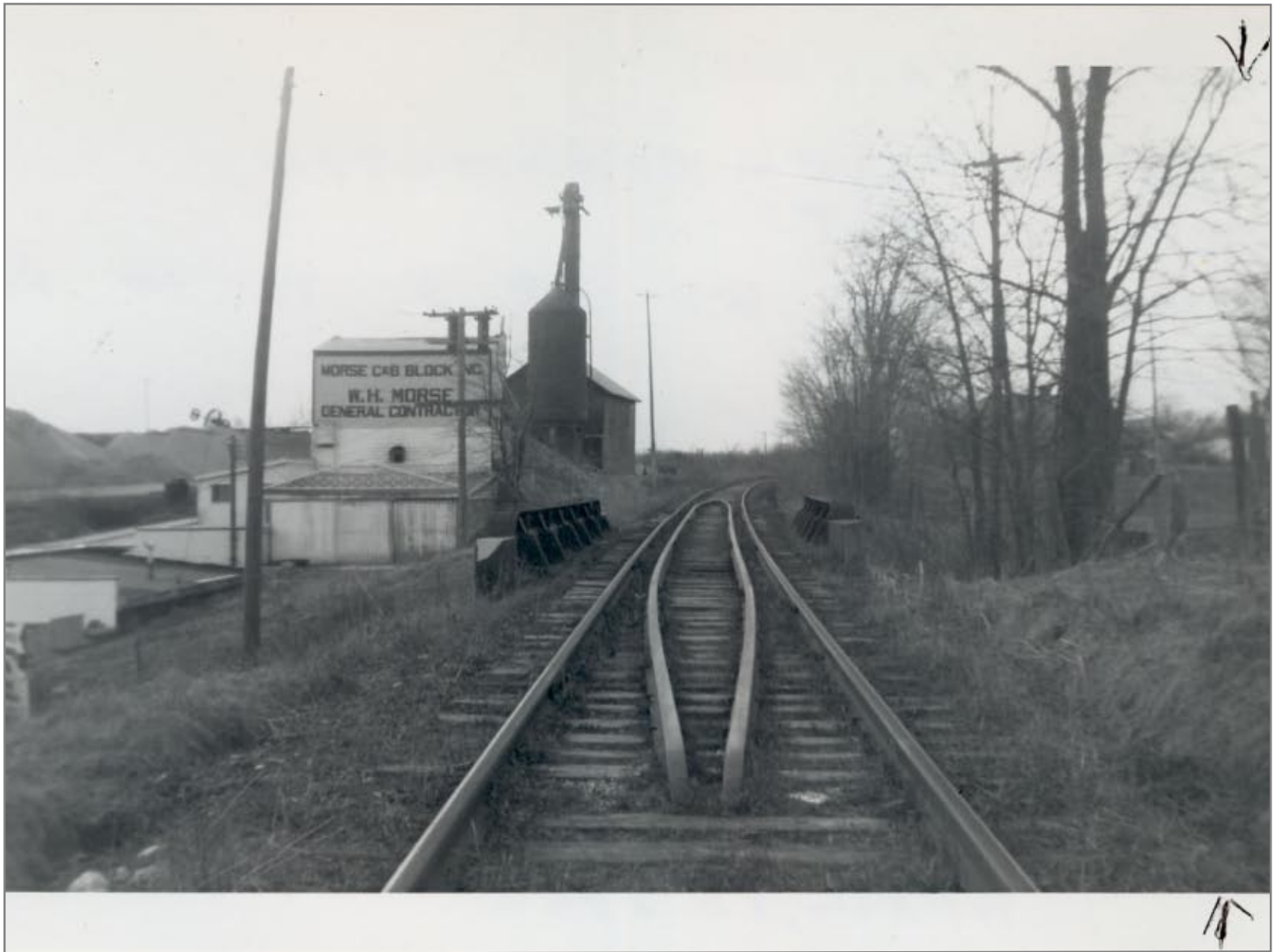
Morse Block, Bridge over Route 7 in foreground 4/15/1962
