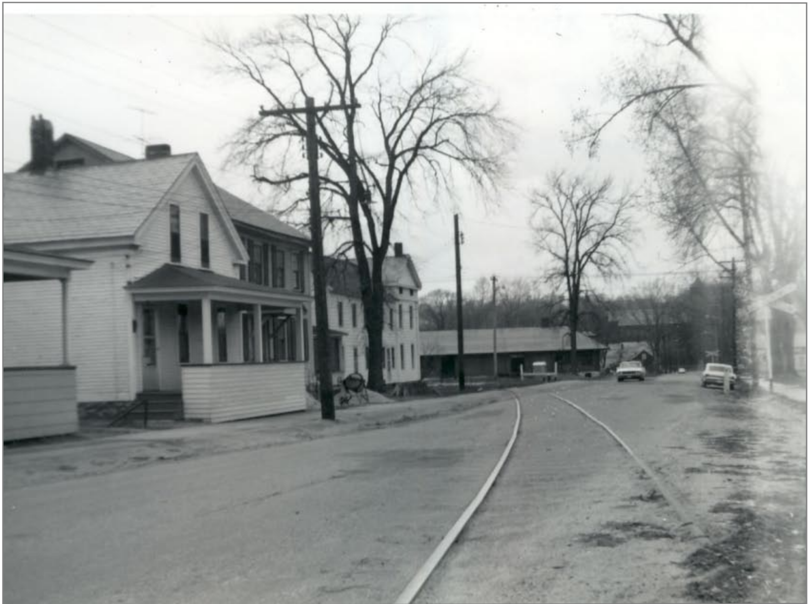
Branch Crossing County Street Looking West Freight House in Distance 4/20/1962
