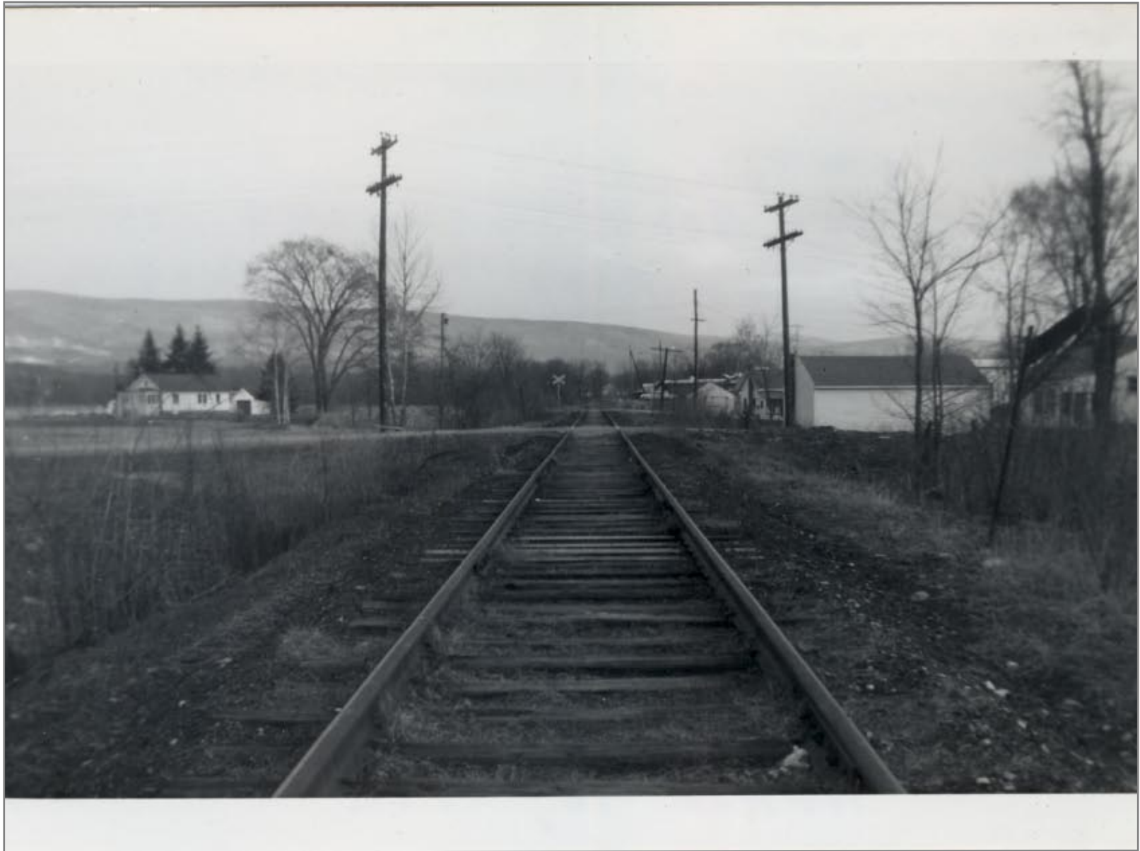
Looking South at Willow Road Crossing with Hick's Crossing in Distance 4/15/1962
