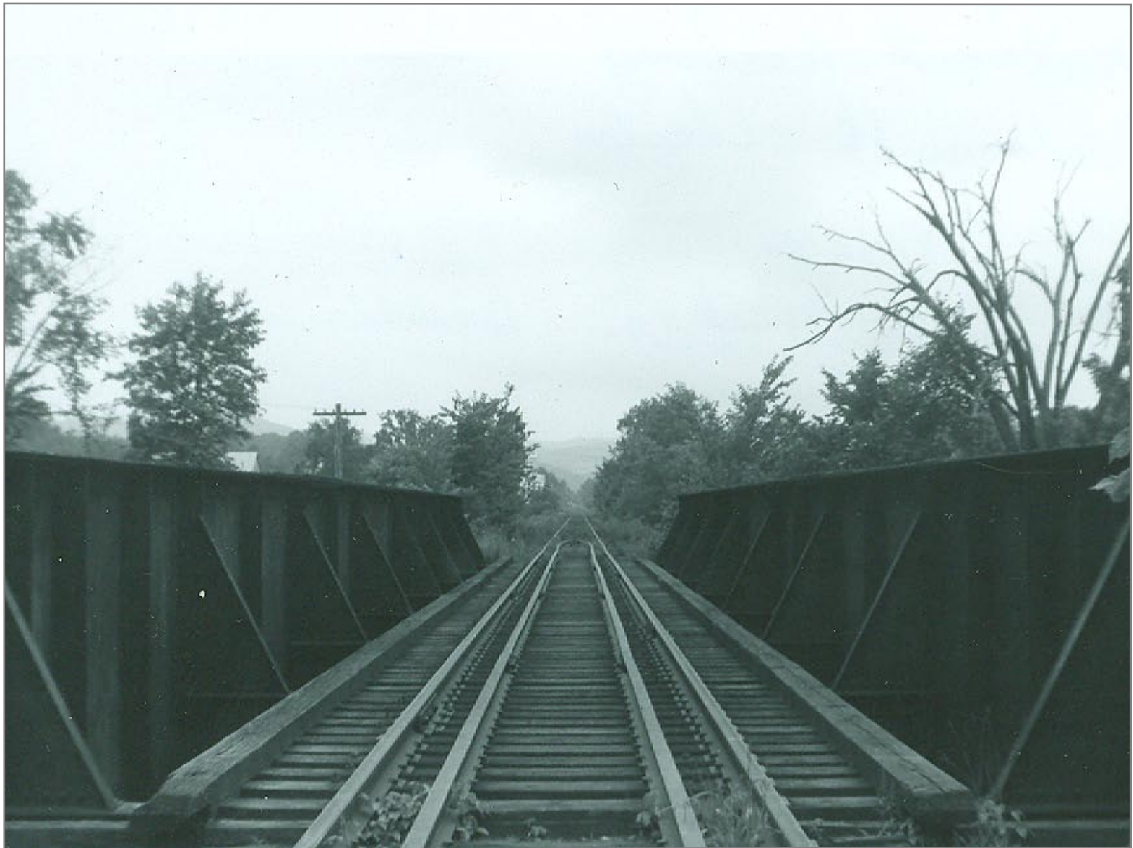
Bridge 119 Northbound over Williams River
