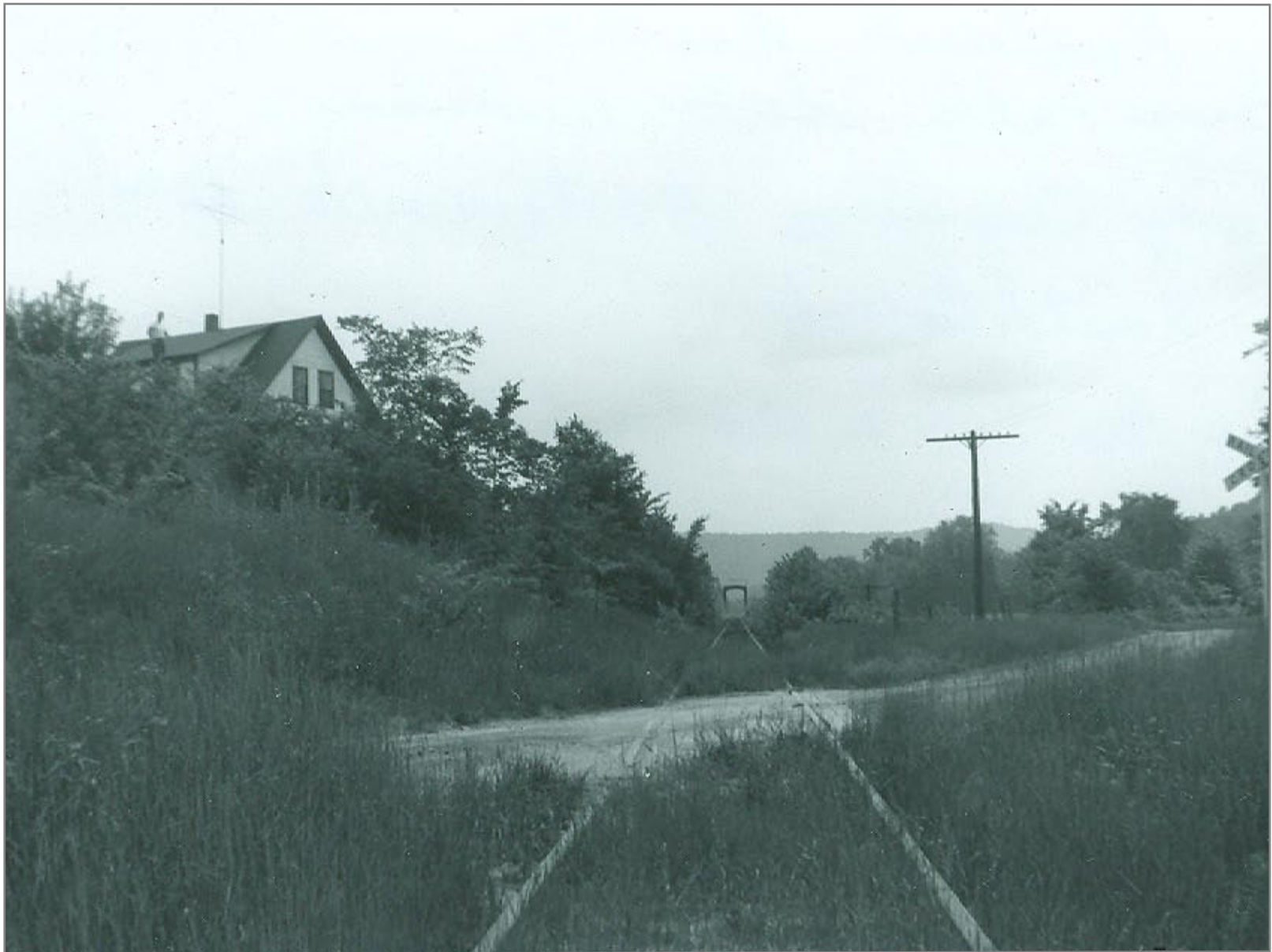
Southbound Bridge 114 in distance
