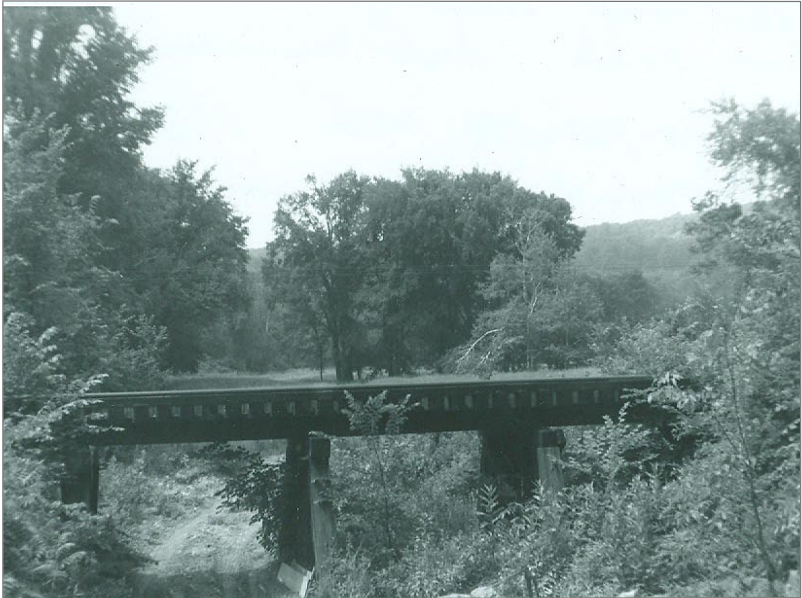
Bridge 115 BLT 1936 44 feet long
