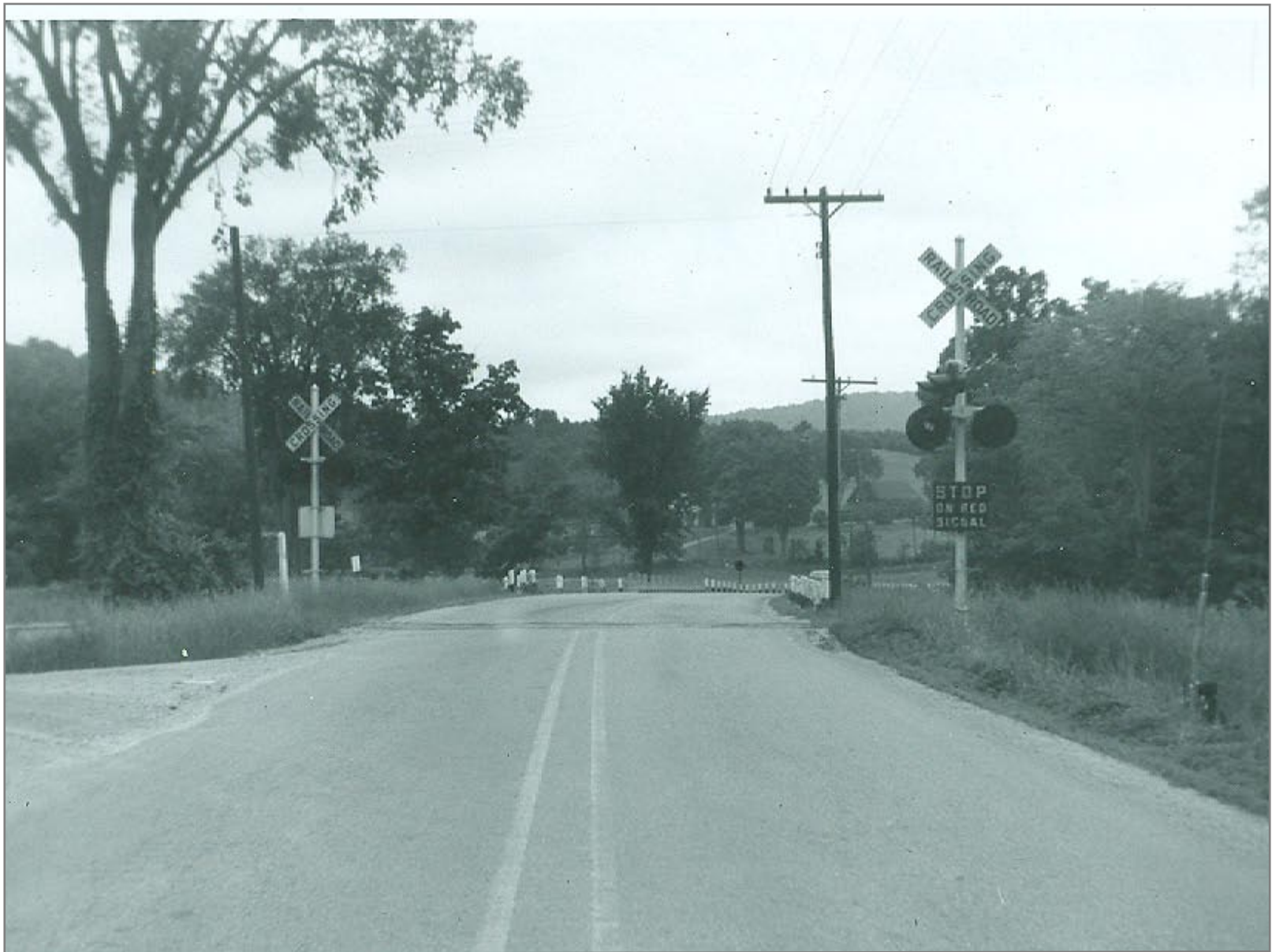
Mile post 13 on left - looking west
