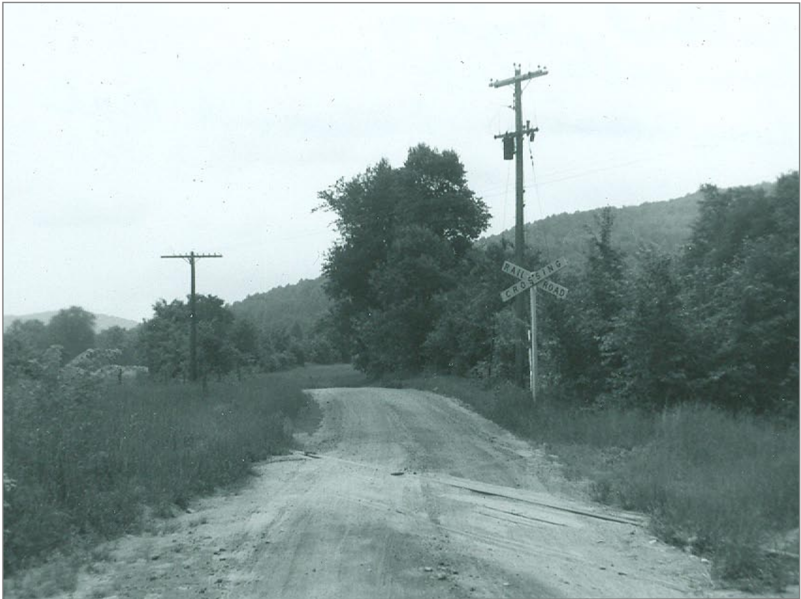
Looking East at 2nd crossing south of Chester
