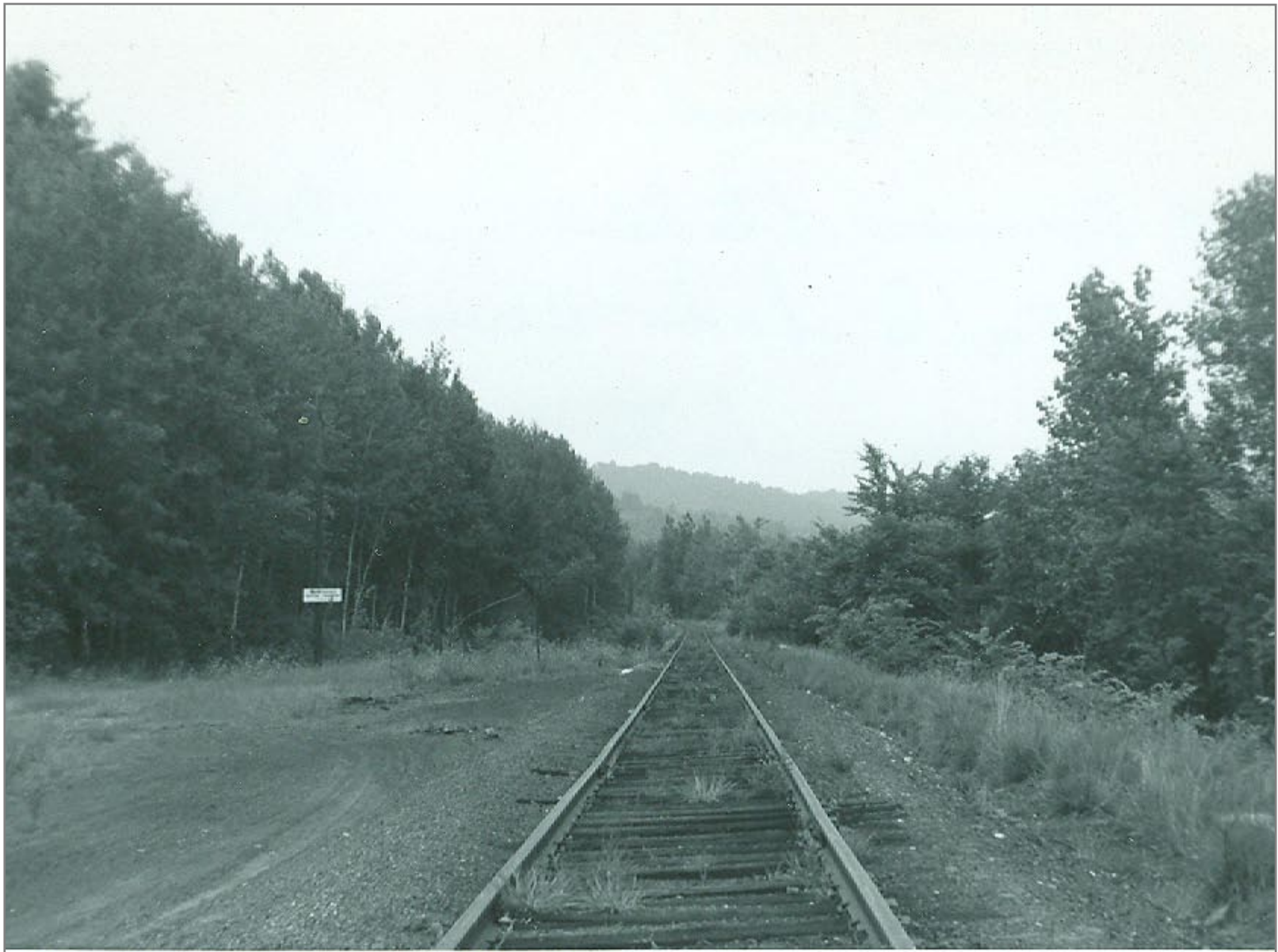
Nothbound at Bartonville Station site on left
