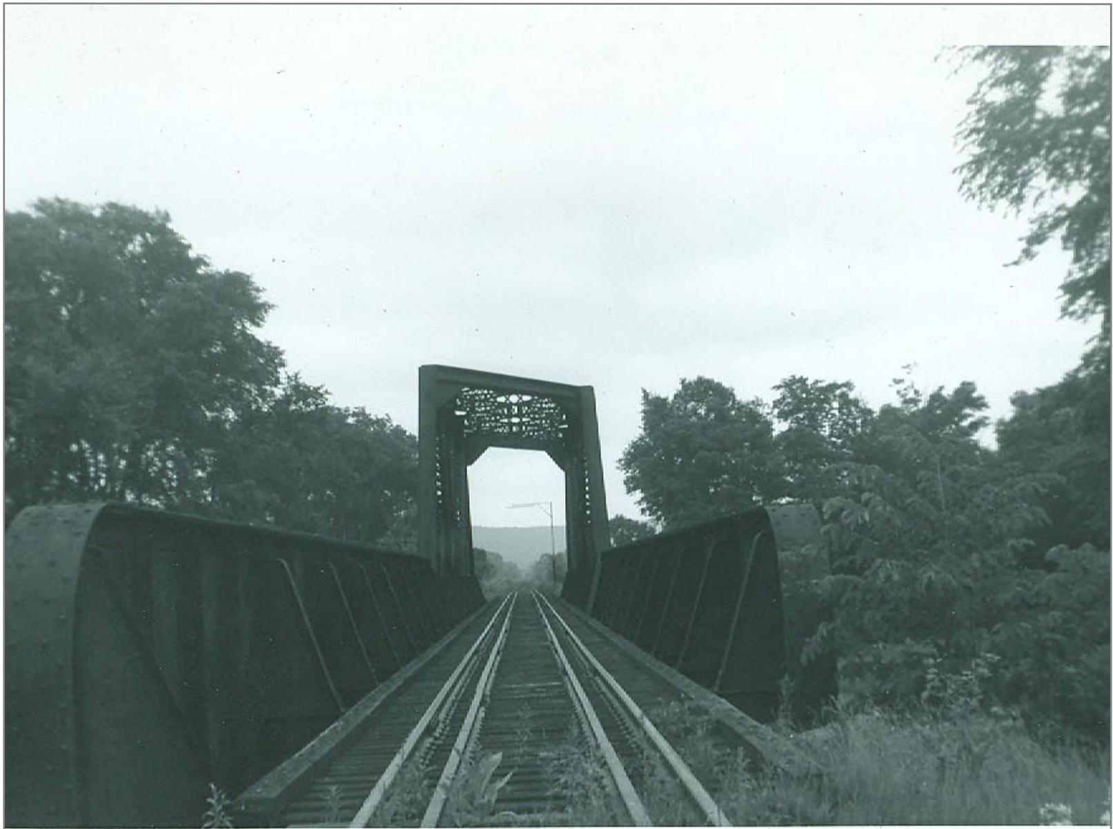
Southbound @ Bridge 118 BLT 1903
