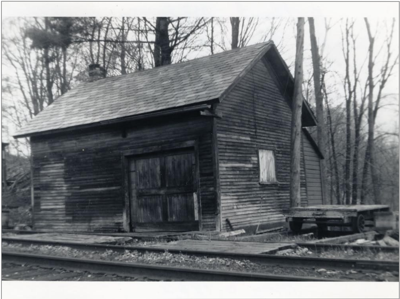
Section House At North End of Arlington Yard 5/6/1962
