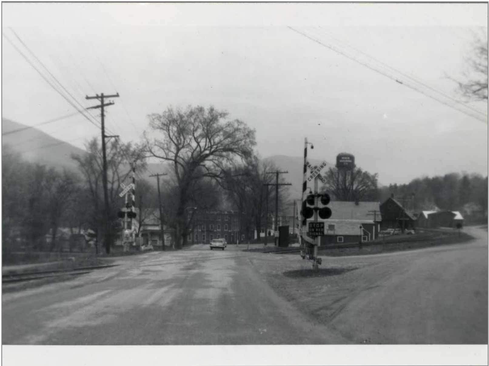
Northbound in Arlington 4/29/1962
