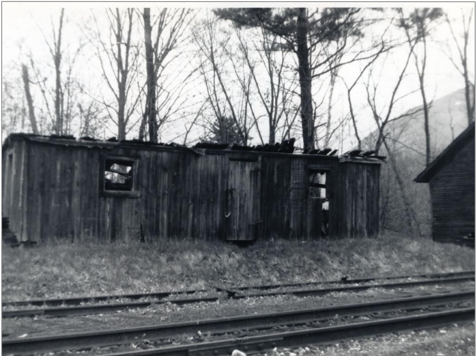
Former O & LC Boxcar Used For Tool Storage 5/6/1962
