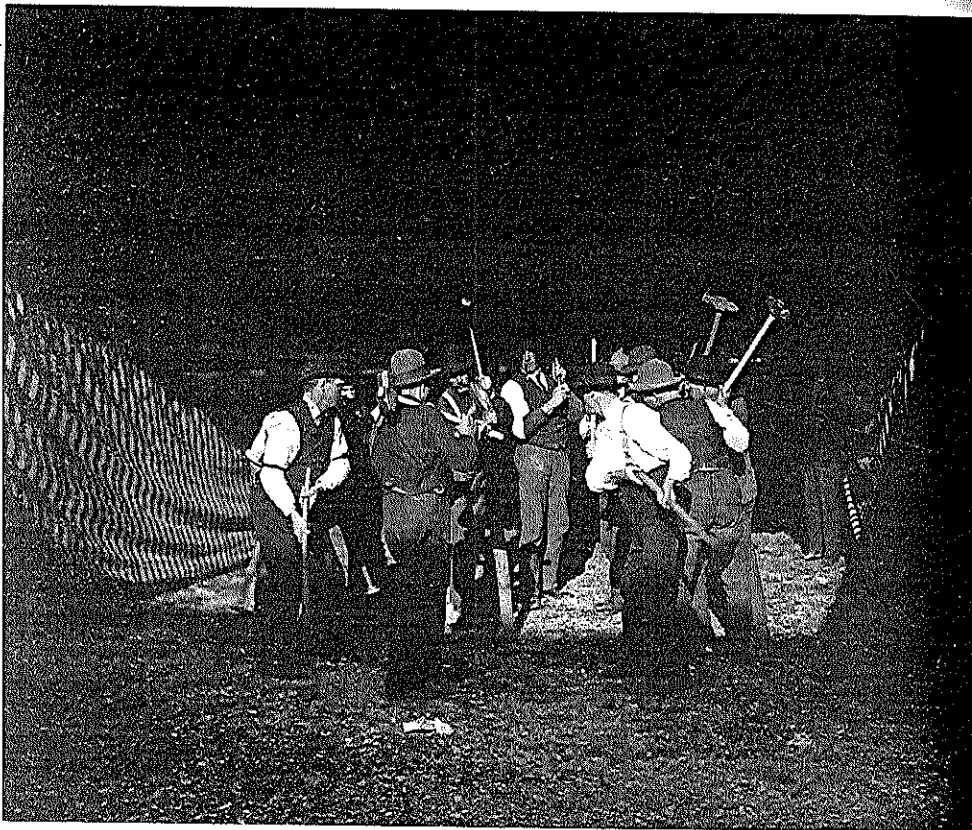
Figure 8. "Sledging Gang," Barnum & Bailey, Brockton, Mass., 1903. With near military precision, stake drivers singing sea shanties and other songs rhythmically pounded into the ground the heavy stakes used to secure the fifty-foot center poles. (Frederick Glasier Collection, neg. no. 1319; black-and-white photograph, copy from glass plate negative, 10 × 8 in., museum purchase, Collection of the John and Mable Museum of Art Archives, Sarasota, Fla.)
