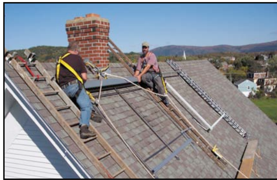
Solar thermal panels being installed at the Shannon St. house.
