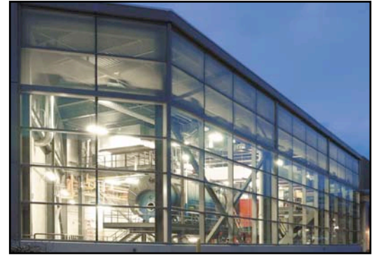
New biomass facility at Middlebury College
