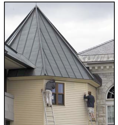
Renovation of McCullough included much needed insulation.
