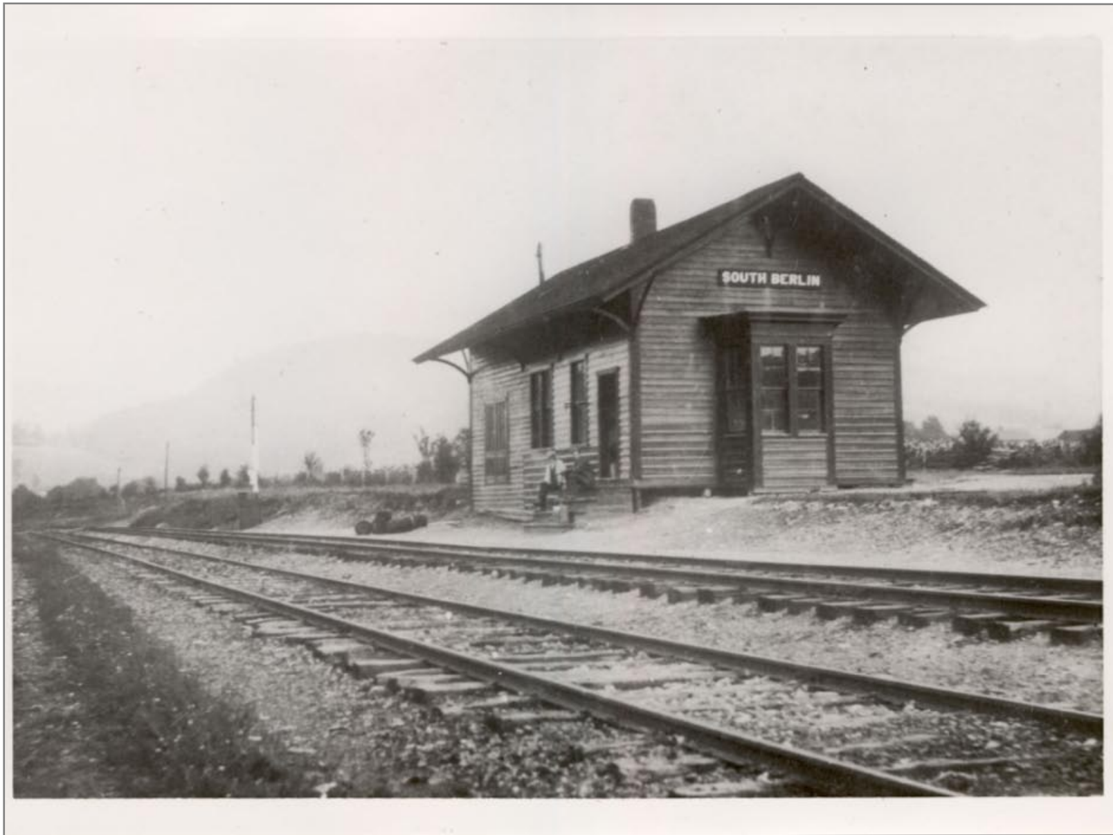
South Berlin Station - The name of this station was changed to Cherry Plain because of confusion on train orders with Berlin Station
