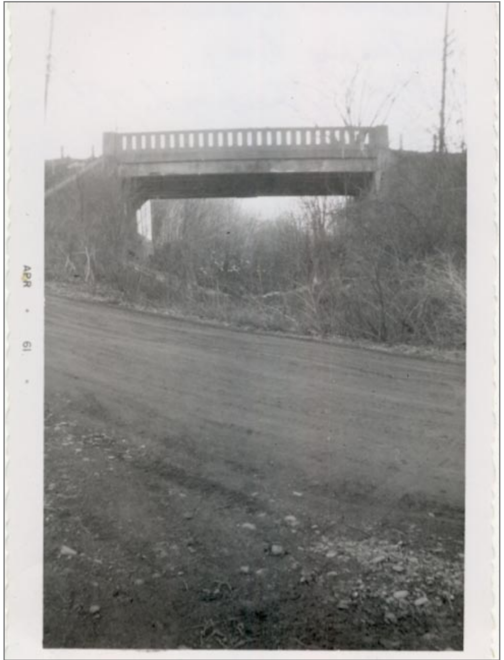
Highway Bridge over Rutland RR looking North from Petersburgh Station site 4/2/1961
